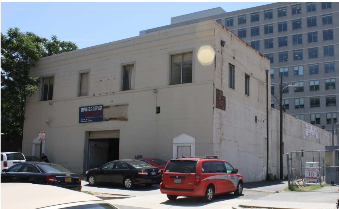
Figure 2: The north and west façade of 37 L St., SE (Commercial). Photograph by Lisa P. Davidson, 10 June 2016.
