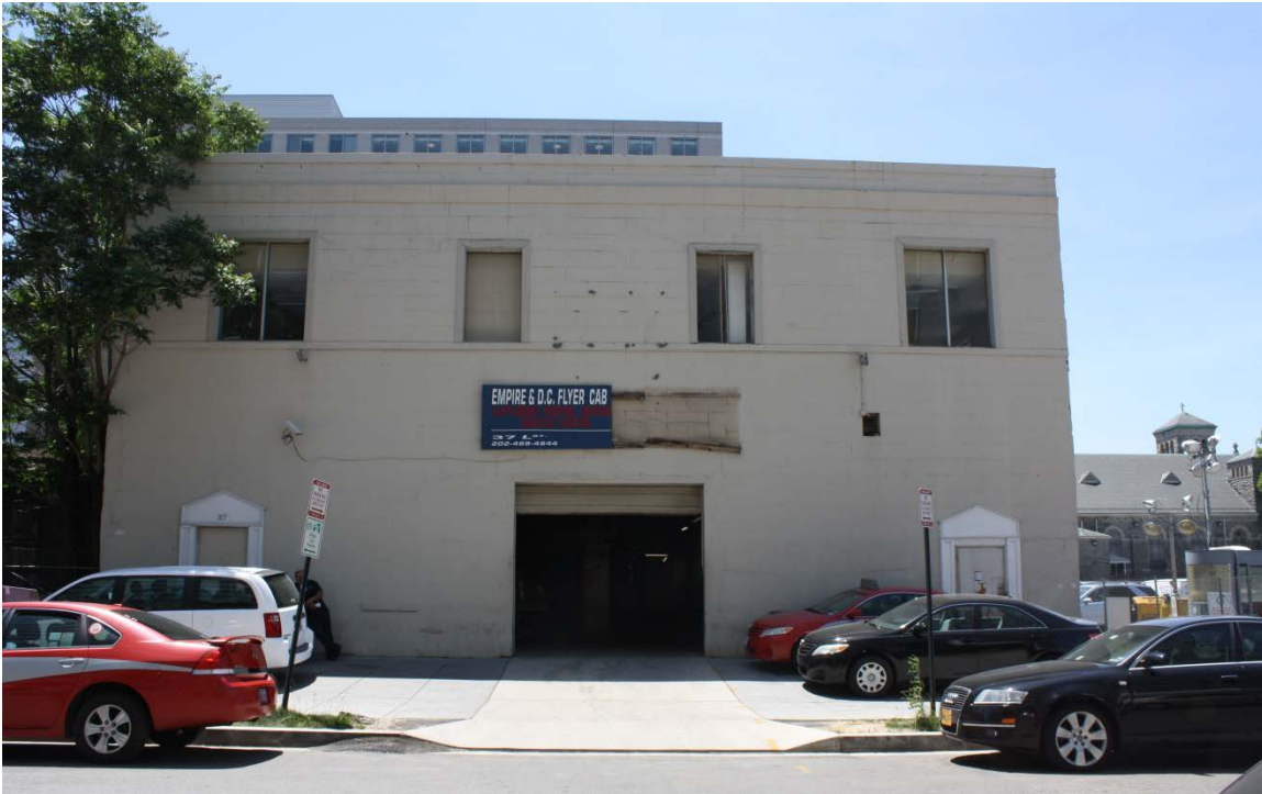
Figure 1: The north façade of 37 L St., SE (Commercial). Photograph by Lisa P. Davidson, 10 June 2016.
