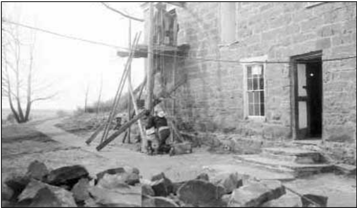
104. Scaffolding erected on south side of fort, January 19, 1959 ( Photograph by Leonard Heaton, Pipe Spring National Monument, neg. 51 ).
