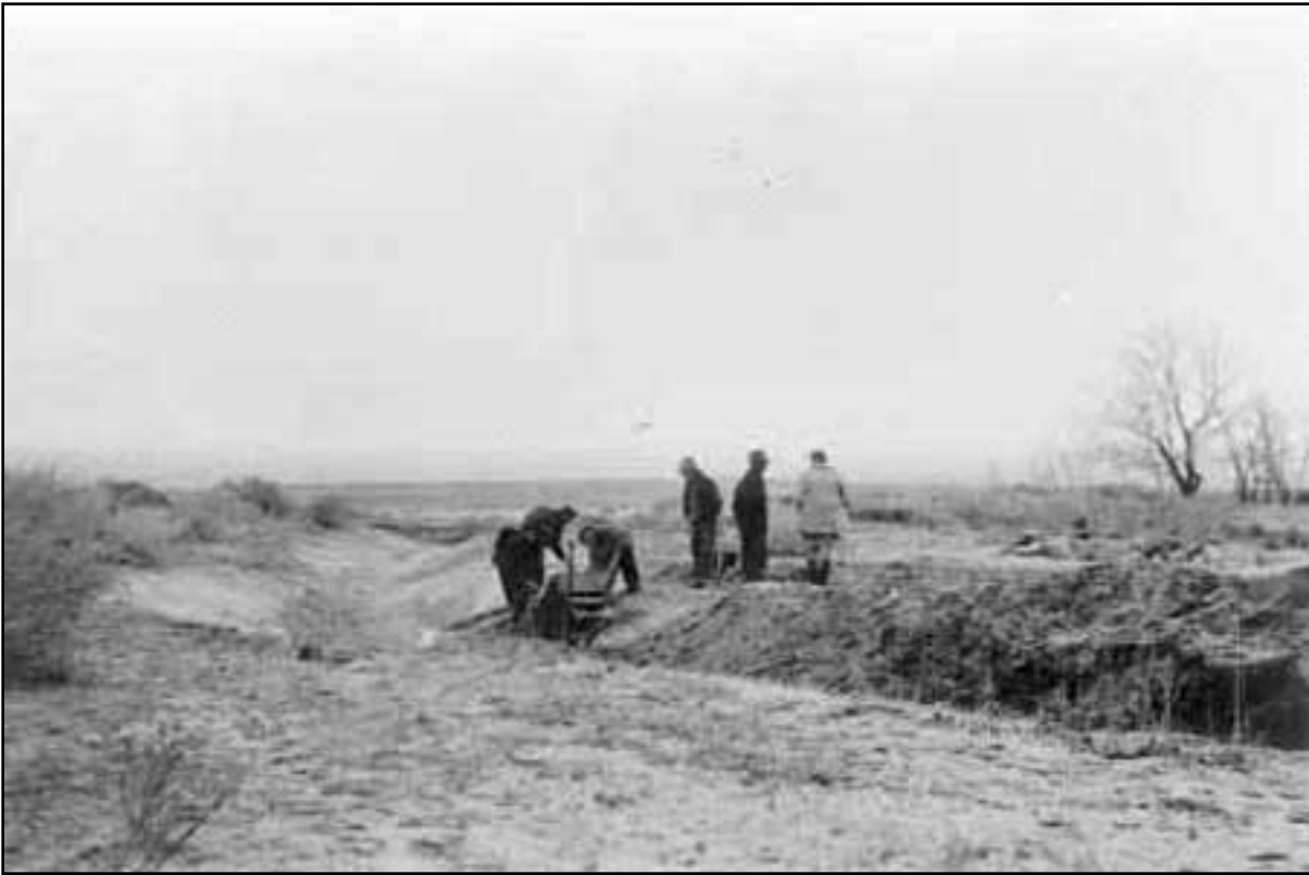
75. Diversion ditch under construction by CCC enrollees to prevent flooding of campground, probably 1936
