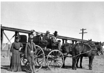
Homesteaders and train trestle
