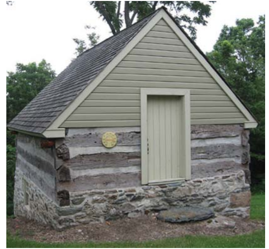
Thornton Poole House, Montgomery County, Maryland. NPS Photo.
