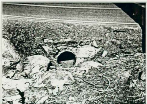
Culvert on downslope side of road – Mileage, 15.10
