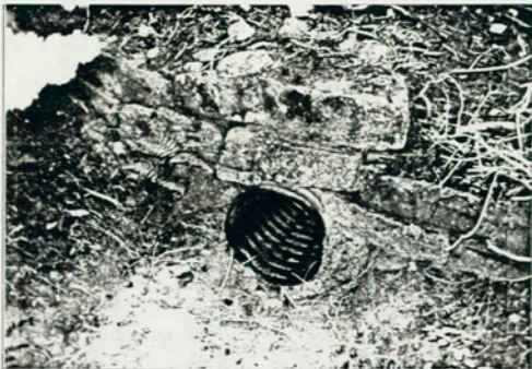
Culvert on upslope side of road - Mileage 14.65
