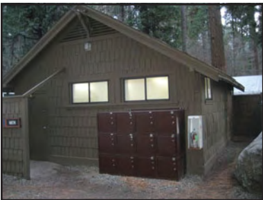
Figure 51. The 1935 500’s comfort station features an undressed concrete foundation and frame construction. This building is identical in design to the 1936 600’s comfort station.
