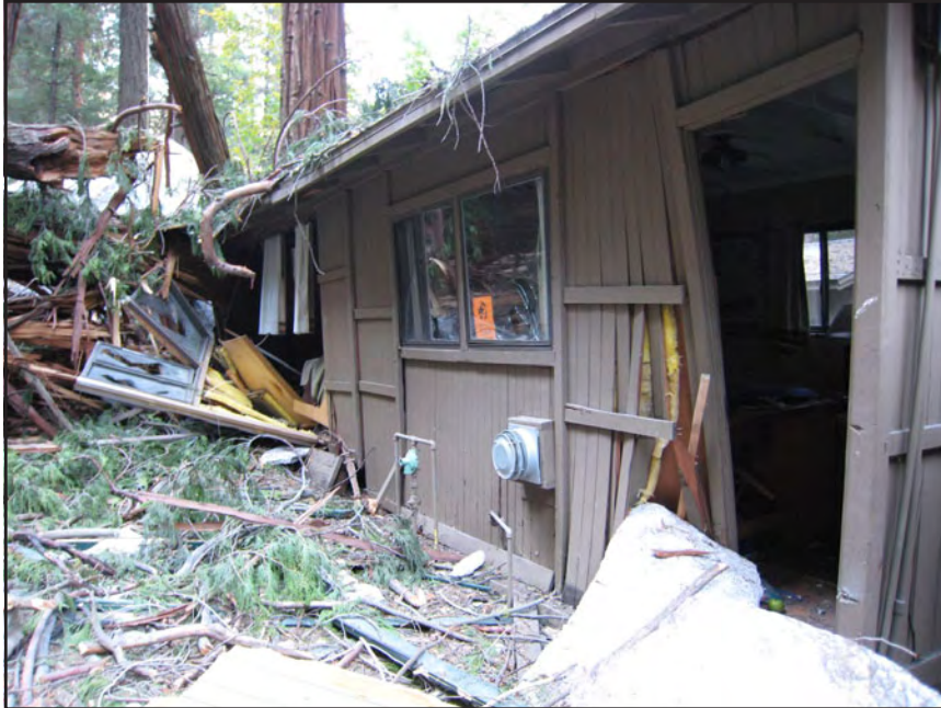
Figure 63. Both hard-sided and tent cabins suffered extensive damage during the October 2008 rock falls at Camp Curry.
