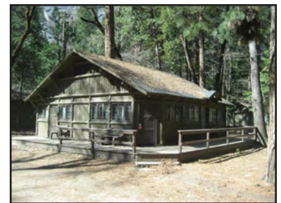
Figure 39. View of fourplex bungalow #1. This is one of the few bungalows that retain log rafter and lookouts.
