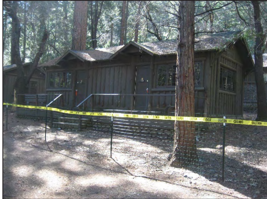
Figure 38. One of the historic bungalows that are within the rock fall hazard zone. This bungalow features board-and-batten siding, with half-log battens.
