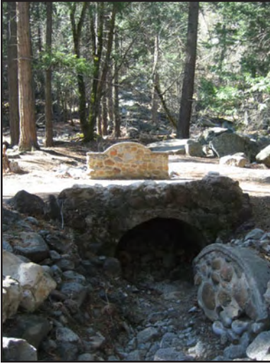
Figure 24. Staircase Creek Drainage Channel as it flows through the bungalows. The far culvert headwall remains intact, while the near culvert headwall has collapsed.
