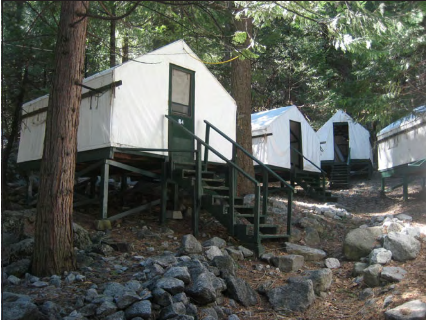
Figure 48. Cluster of four tent cabins in the area determined to be uninhabitable due to rock fall danger. Due to the steeper terrain and the presence of boulders, the majority of cabins within the rock fall zone are characterized by elevated platforms and irregular groupings and configurations.
