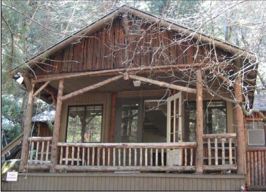
Figure 35. Primary entrance and porch to the Foster Curry Bungalow. Incompatible repairs made to the building include the use of textured plywood around the foundation, dressed lumber for the stairway railing, milled landscape timbers for the right lookout and knee brace, false divided light aluminum windows and the use of modern-appearing light fixtures on the porch.
