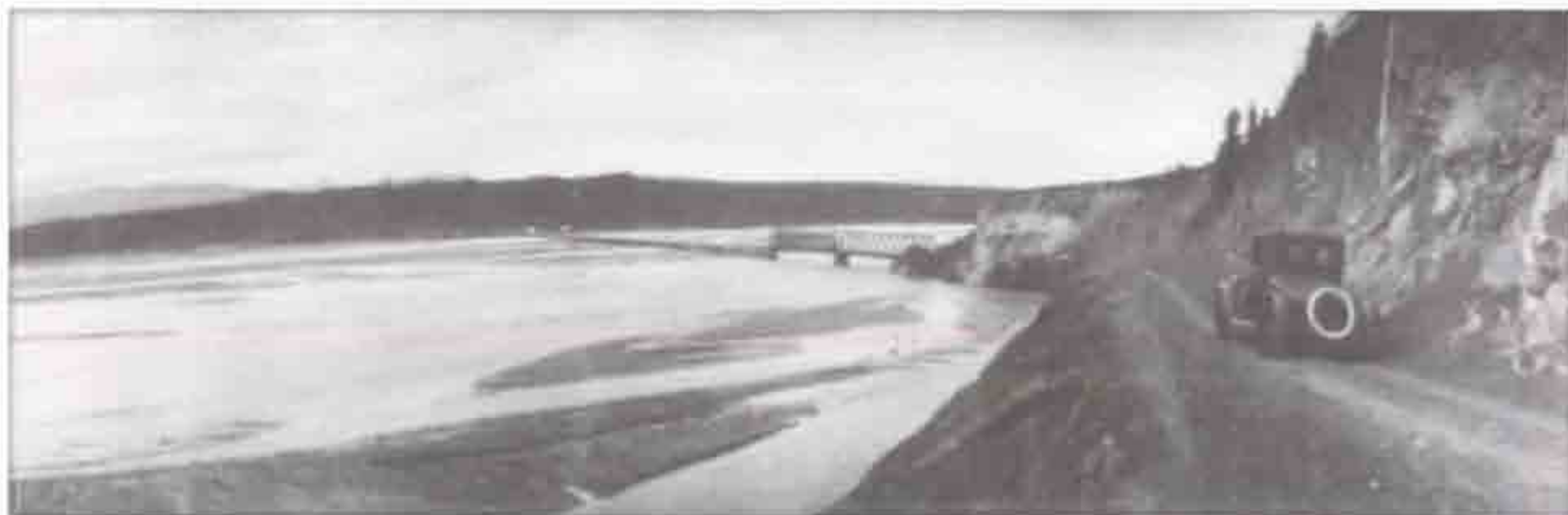
Nizina River Bridge.
