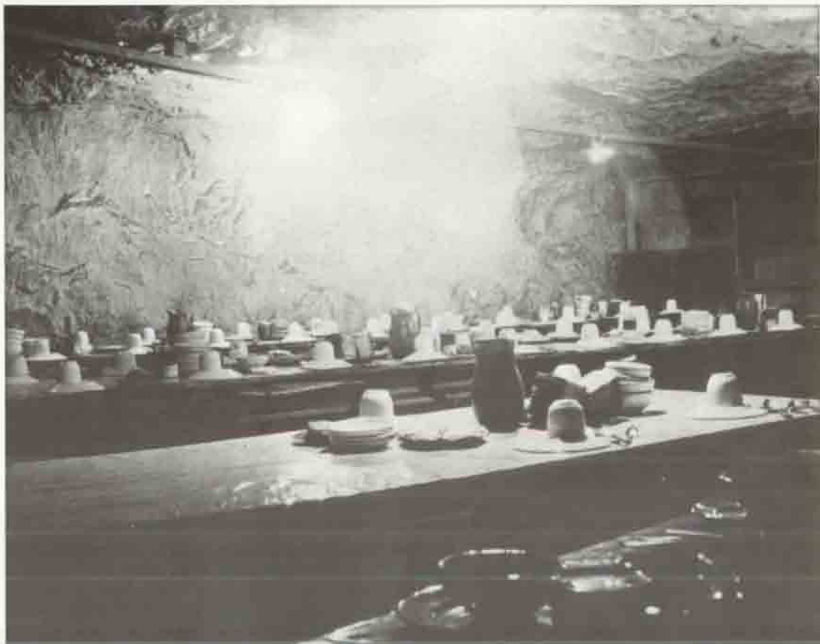
Bonanza dining hall, 500 feet below ground level.
