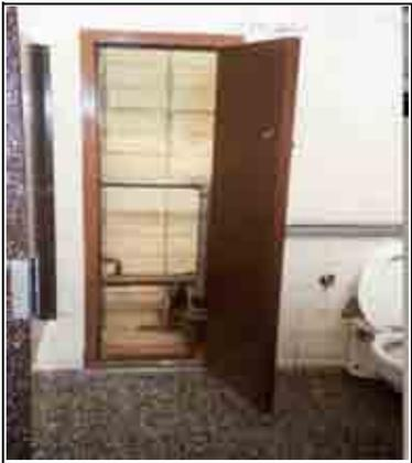
**Deficiency:** Water closet designated for handicapped is not mounted at proper height for handicapped accessibility.
