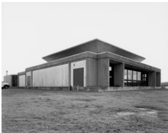
**Figure 25** Above, view of northwest corner of building showing modern window system at right, white "Shadowform" panels and infilled window bays on north side of building at left (National Park Service, 2000)
