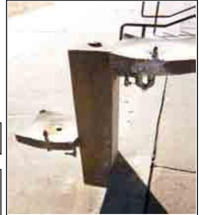
**Deficiency:** Working parts are missing, concrete parts are cracked and broken out.
