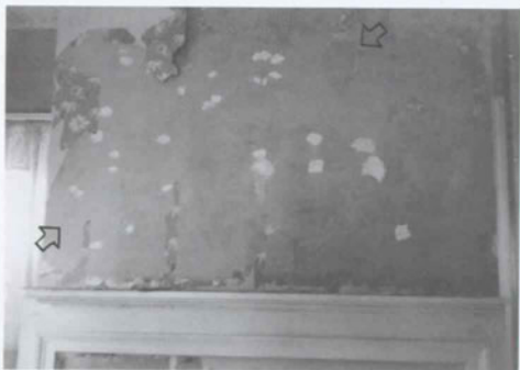
Figure 92. M'Clintock House: Room 104 (Kitchen/Dining Room), Chimney Breast; arrows indicate stovepipe patch and wallpaper note shown below [1988].
