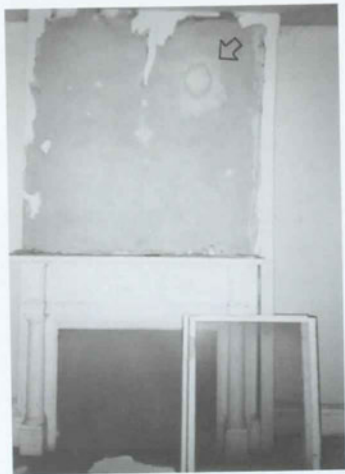
Figure 77. M'Clintock House: Room 102 (Parlor), Patch in Chimney Breast at Former Stovepipe Hole [1988].
