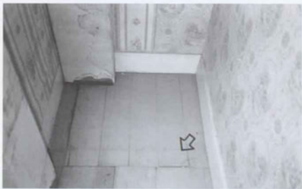
Figure 87. M'Clintock House: Room 103 (Southeast Room), Closet Floor at West End, Showing Location of Earlier Wall [1988].
