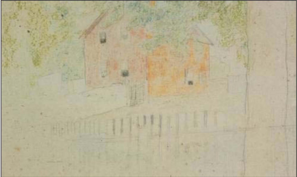
**Figure 1.4.** Drawing by Julian Alden Weir, showing north and west elevations of caretaker's house (circa 1885). Noticeably absent are the east kitchen ell and window #W109, neither of which had yet been built.
