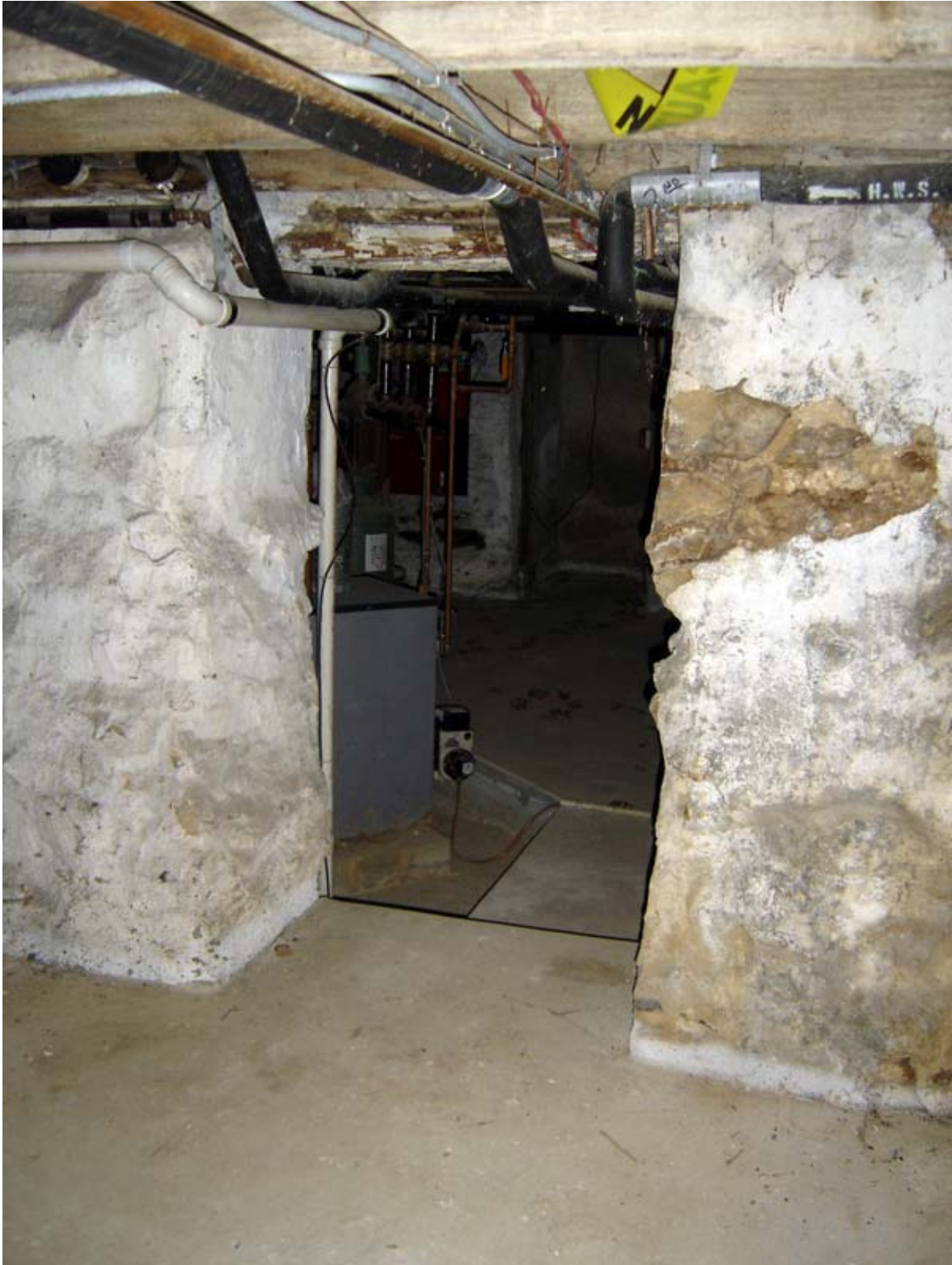
Photo 001b - Masonry opening between Rooms 001 and 002, looking west. Rough character of stonework suggests that the opening was added after original construction. This opening was likely formed at the time of the east addition, c.1830.
