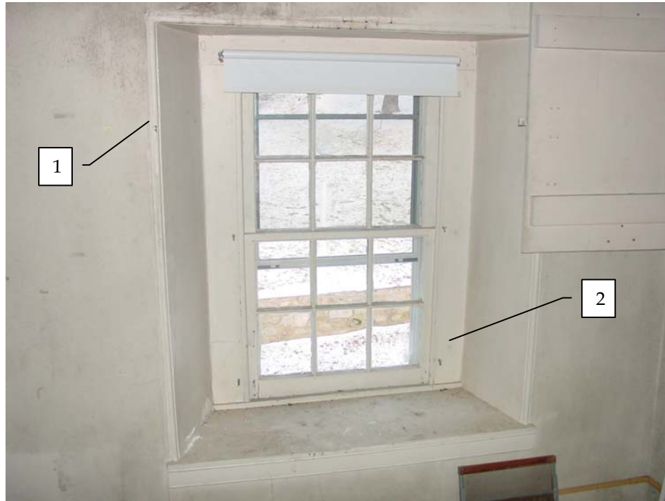
Photo 201c - Interior view of Window 223, looking north.
