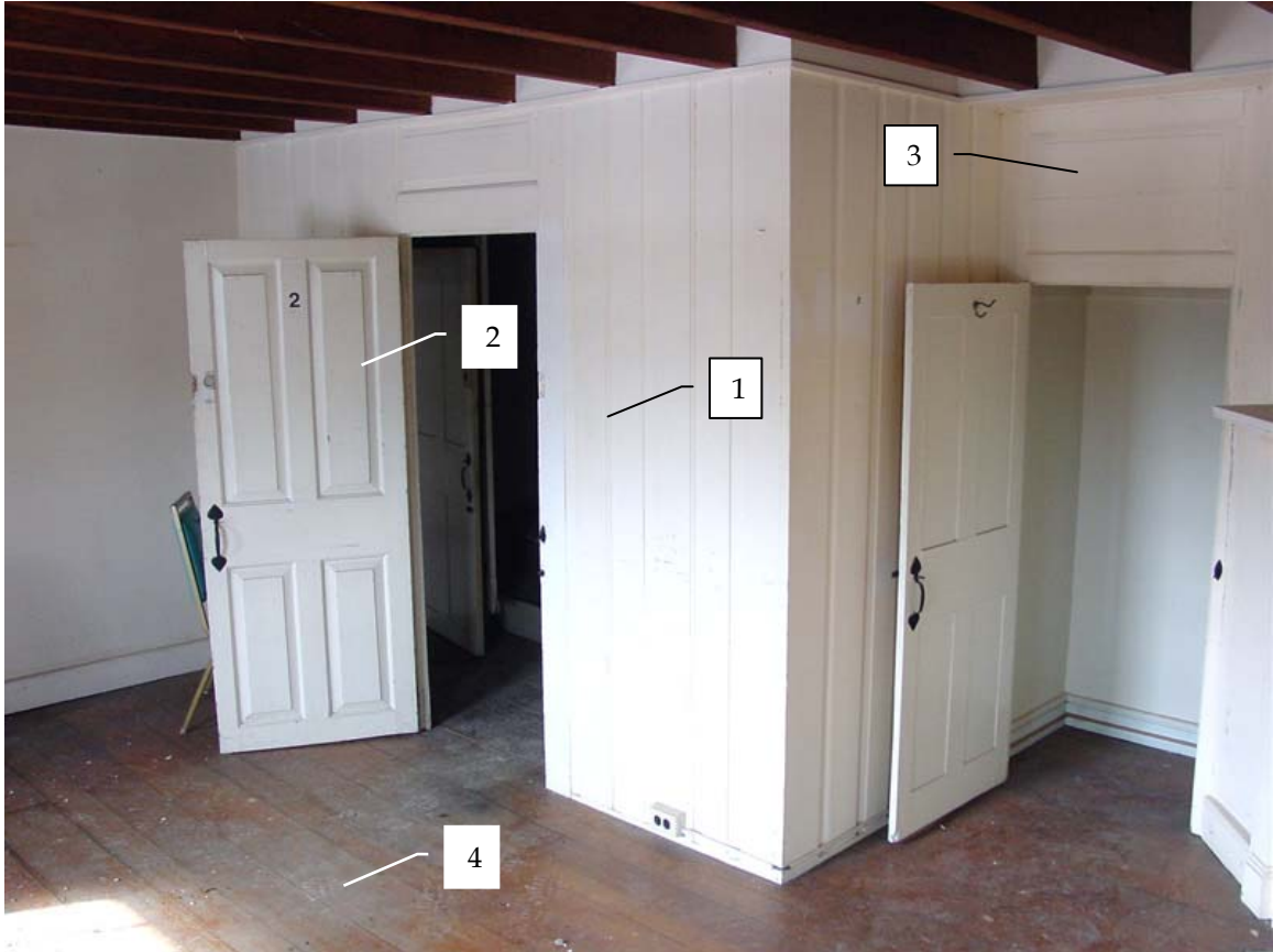
Photo 205a - View of north wall of Room 205, looking northwest.
