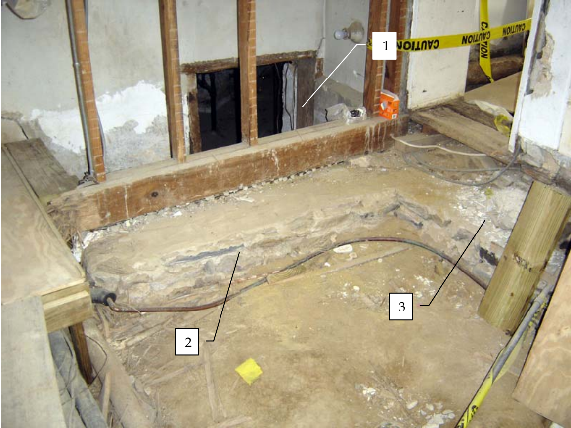
Photo 106c - General view of floor in Room 106, looking southeast.
