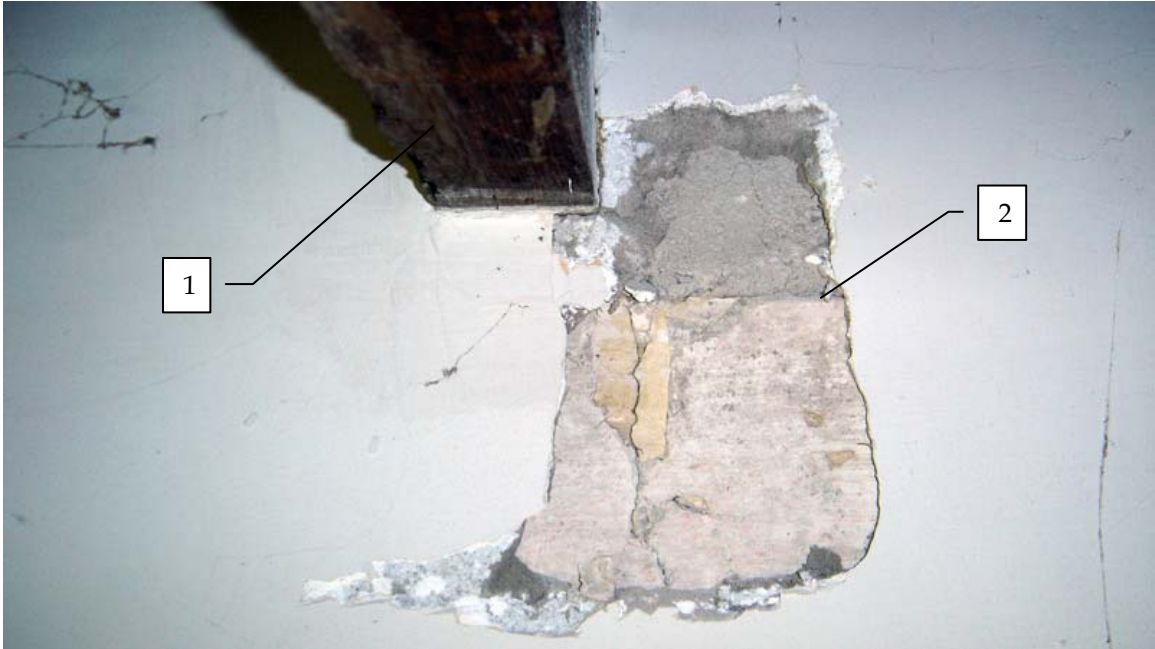
Photo 101a – Detail of plaster evidence below ceiling joist, south wall, Room 101, looking south. 1. Nail holes for lath at underside of joist. 2. Line of original c. 1830 plaster indicating intersection of wall and former ceiling plaster.
