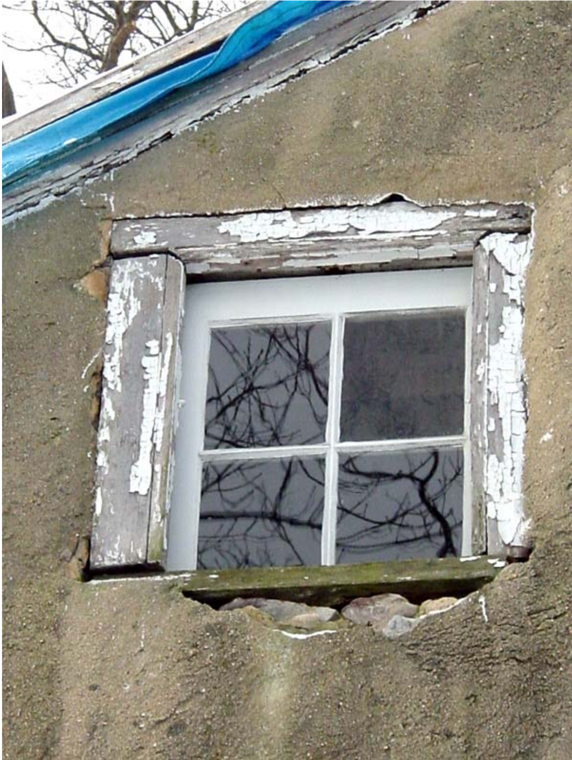
Photo EEe – Exterior view of Window 302, looking west.
