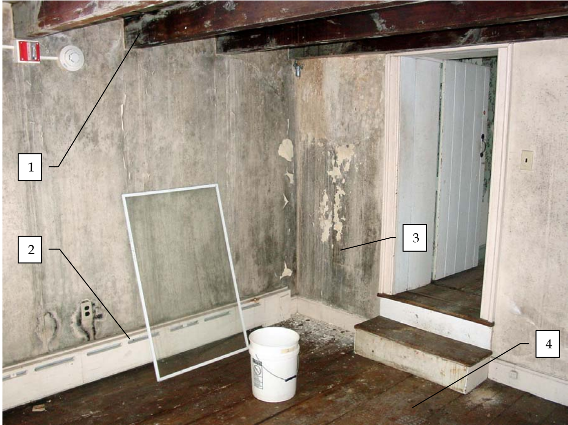
Photo 201a – Interior view of Room 201, looking southwest.
