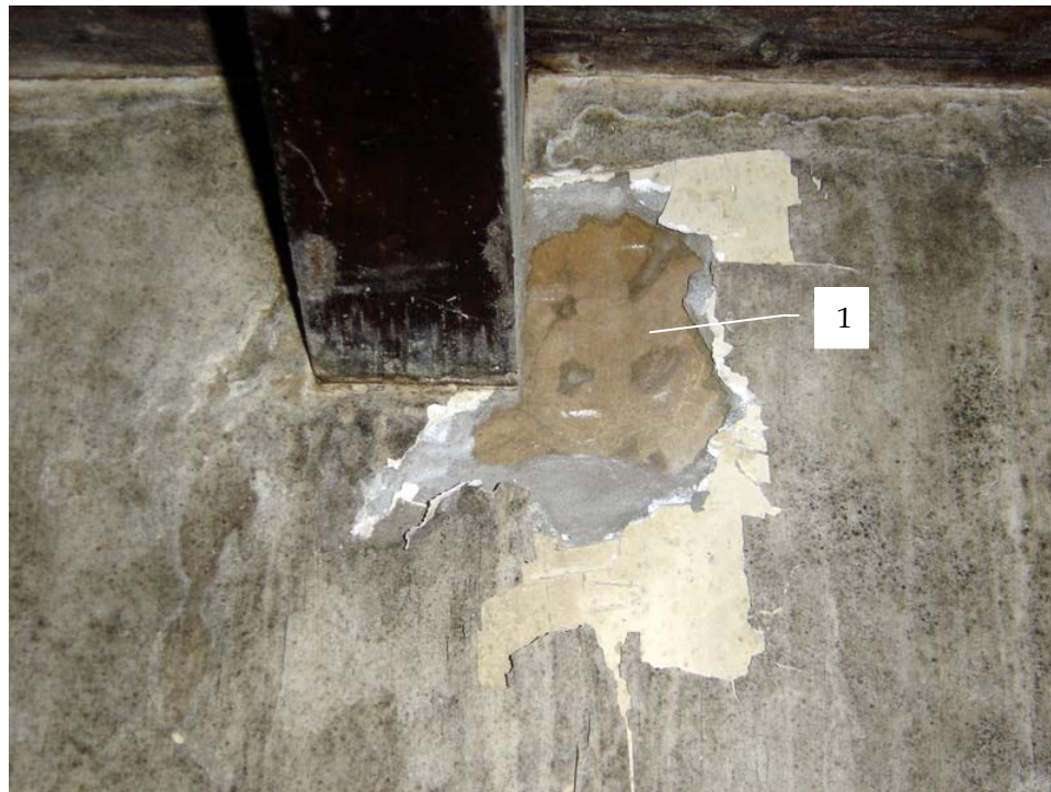
Photo 201d - Detail view of plaster at south wall, Room 201, looking south.
