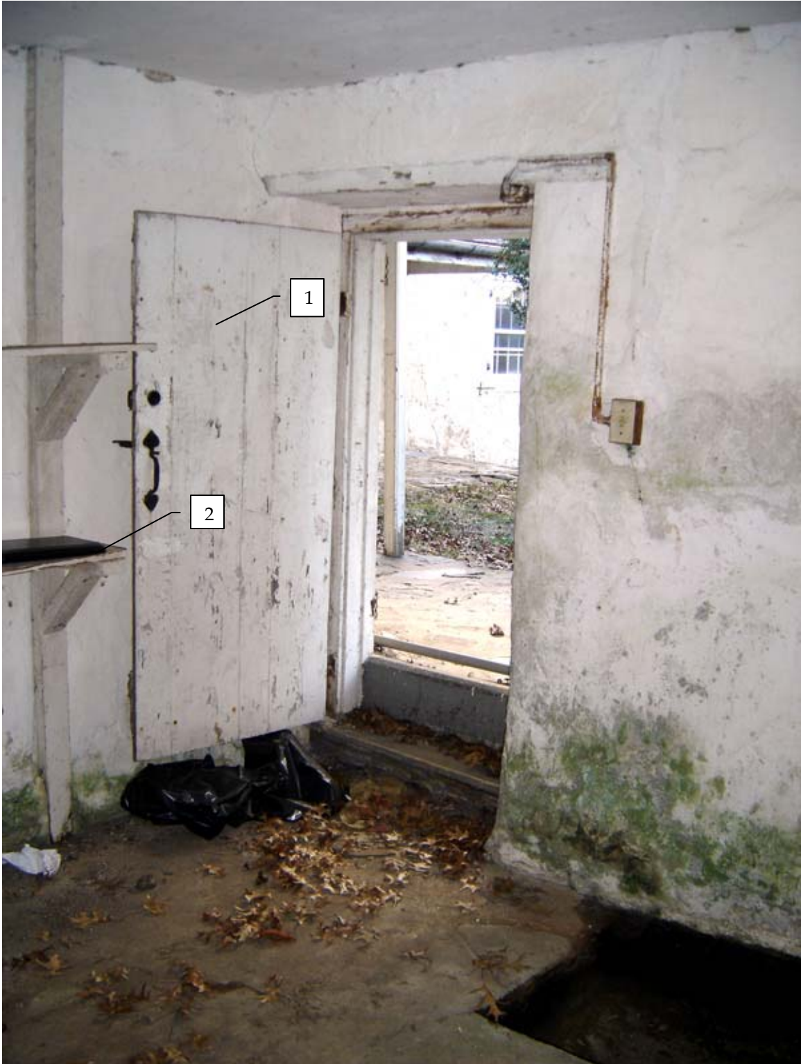
Photo 109c - Segment of springhouse interior, Room 109, looking southeast.
