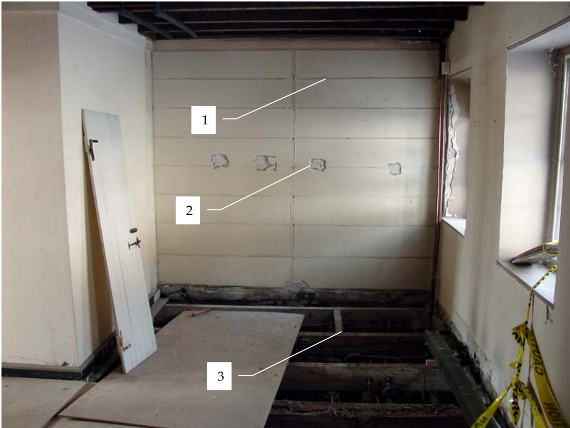
Photo 102a – View of west wall, Room 102.
