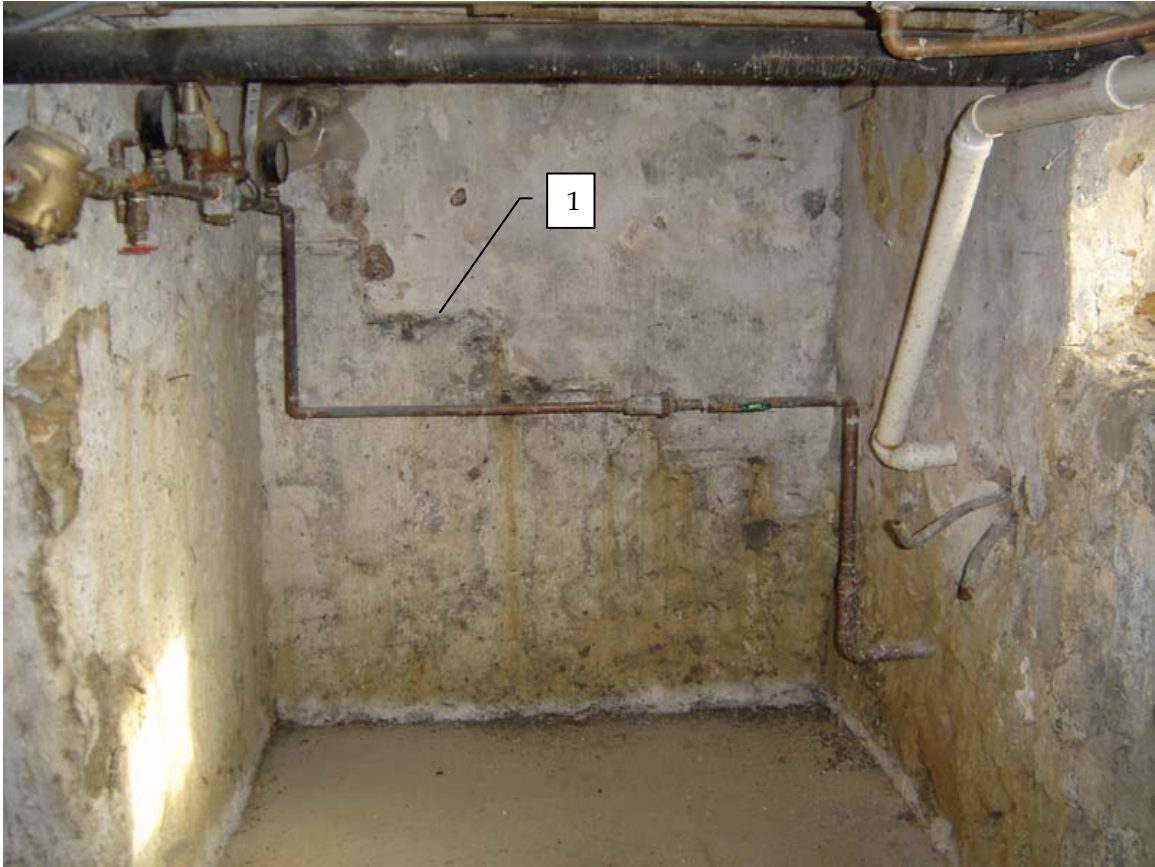
Photo 001a - View of segment of east wall to the south of the chimney vault, Room 001, looking east.
