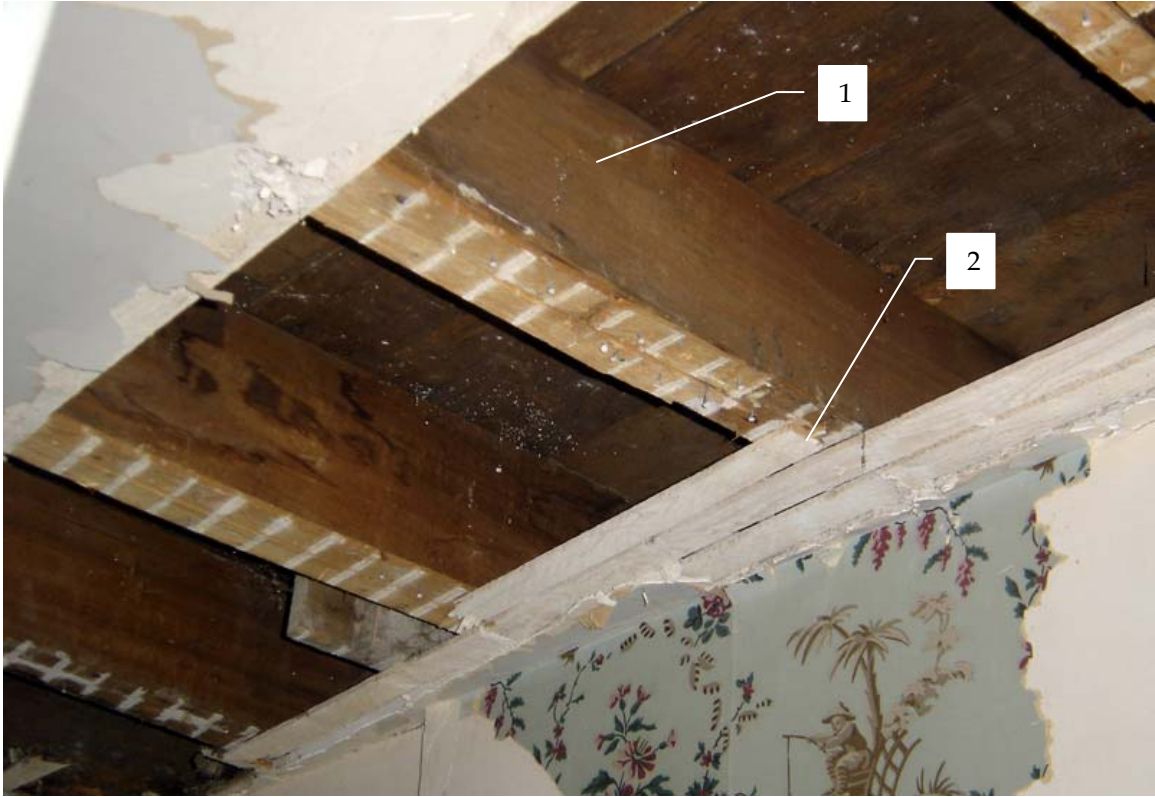
Photo 204b – View of exposed ceiling joists, Room 204A, looking southeast.
