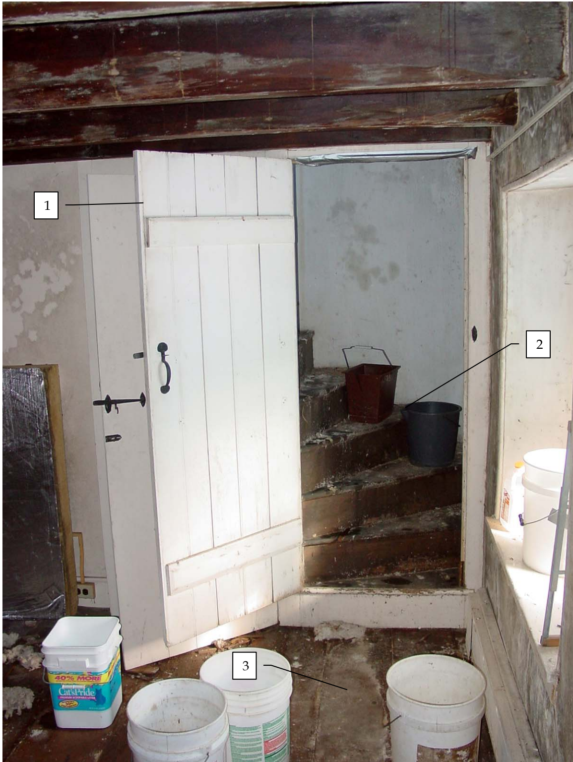
Photo 201b – Winder stair (c. 1830) at southeast corner of Room 201, looking east.
