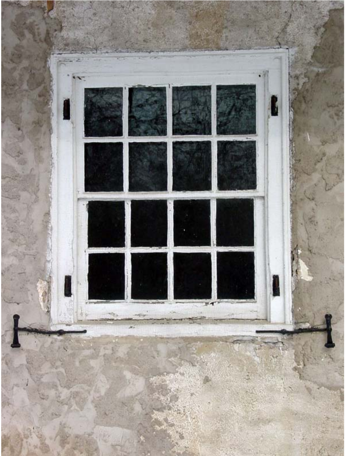
Photo SEg - Exterior view of Window 105, looking north.
