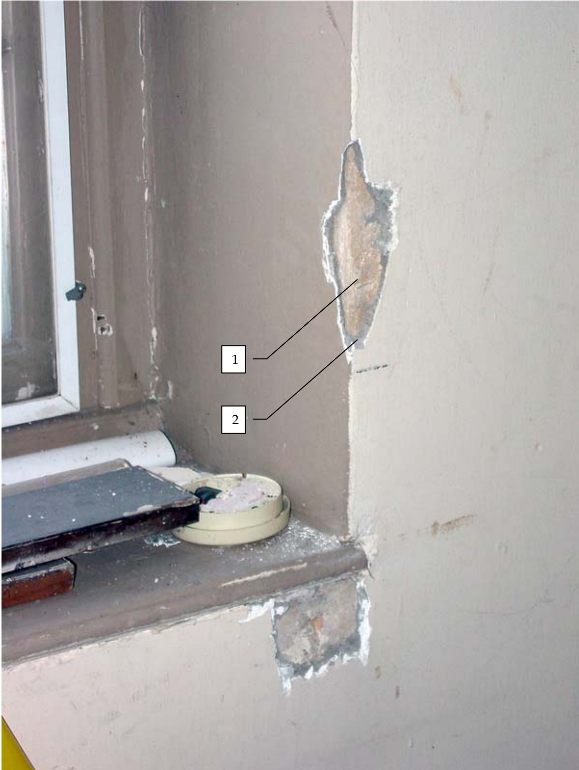
Photo 102c - Detail view of plaster at interior jamb, Window 118, looking northeast.
