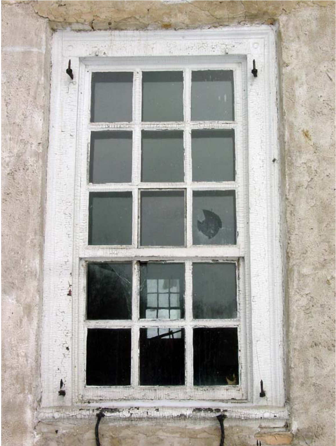
Photo SEf - Exterior view of Window 104, looking north.
