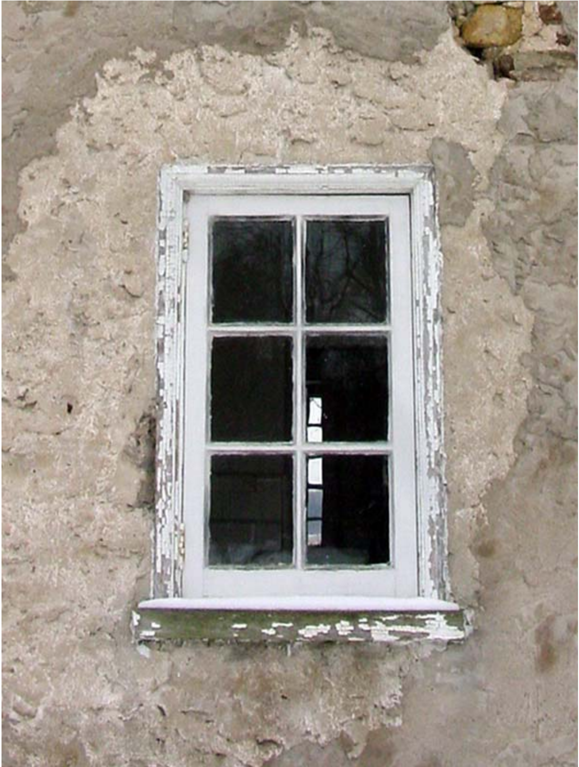
Photo WEe - Exterior view of Window 106, looking east.
