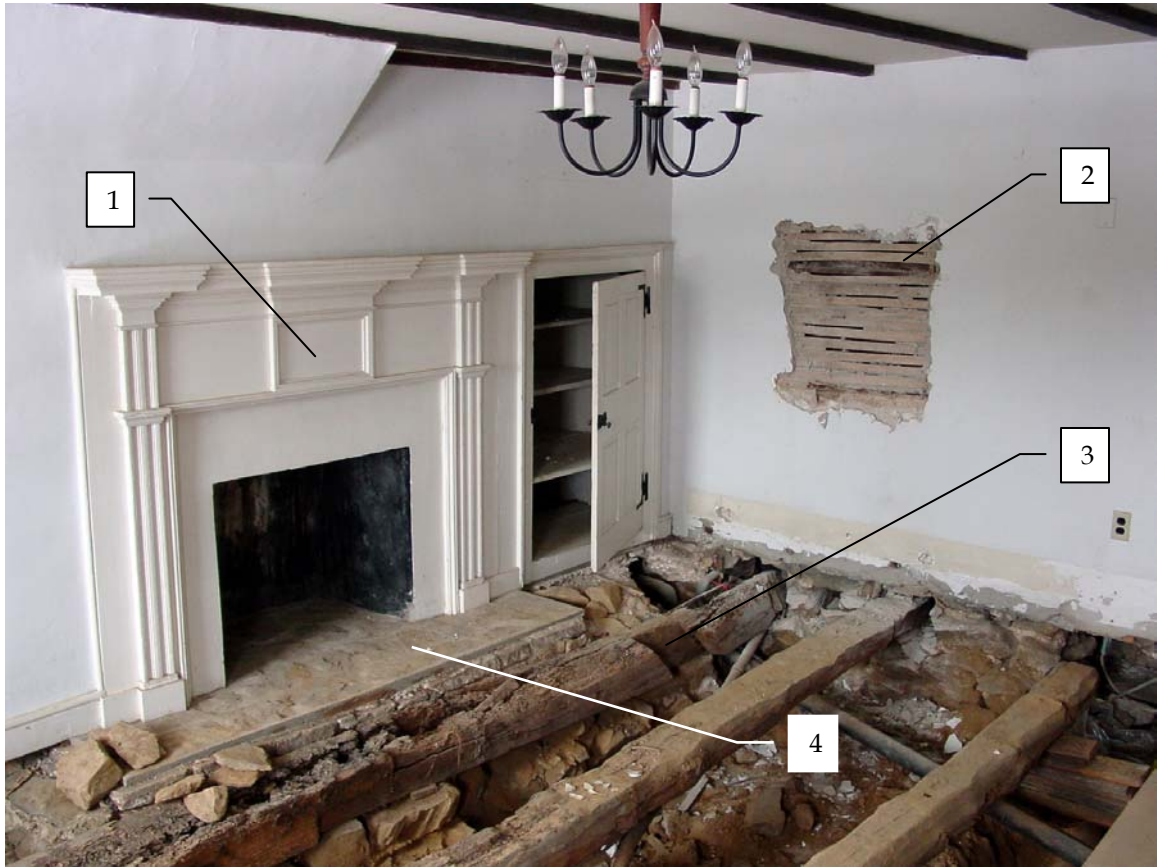
Photo 104a – Interior view of Room 104, looking northwest.
