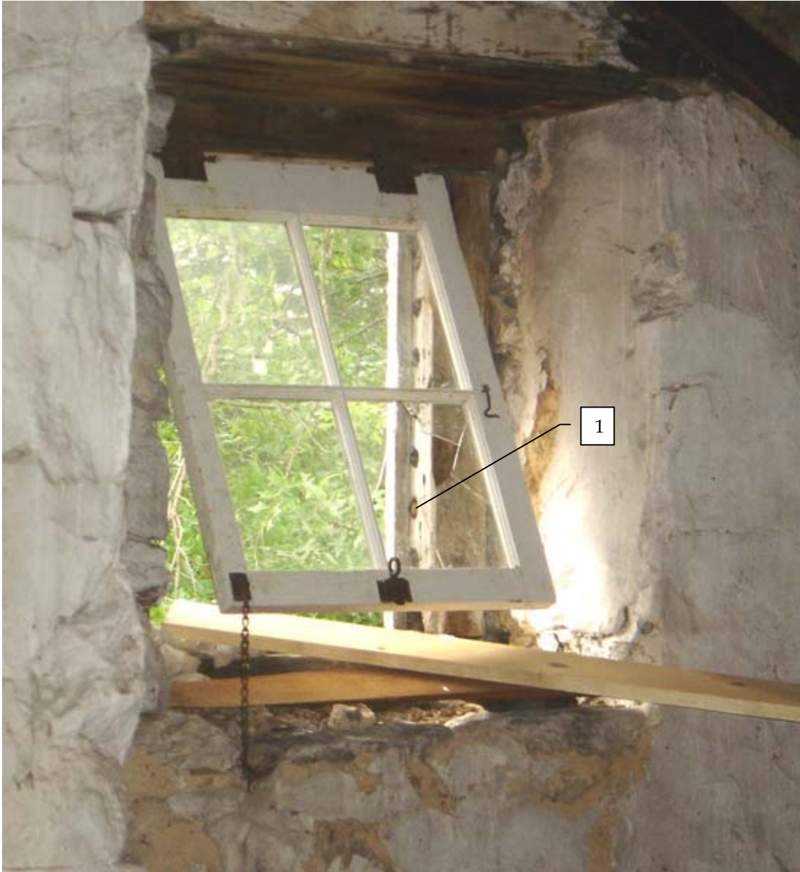
Photo 302a – Interior view of Window 302, looking southeast.
