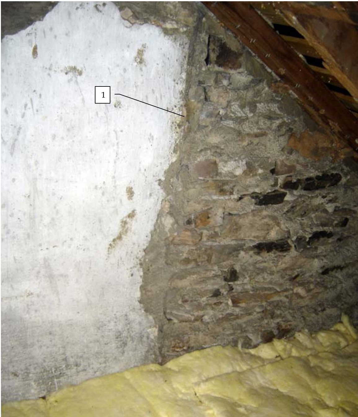
Photo 303a – West wall, north end, Room 303, looking west.
