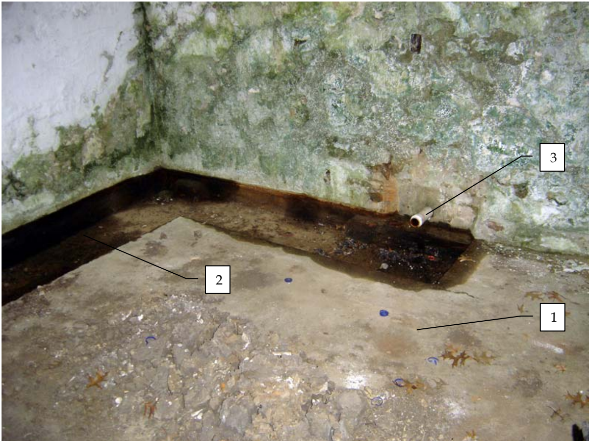
Photo 109a - Segment of springhouse interior, Room 109, looking northwest.
