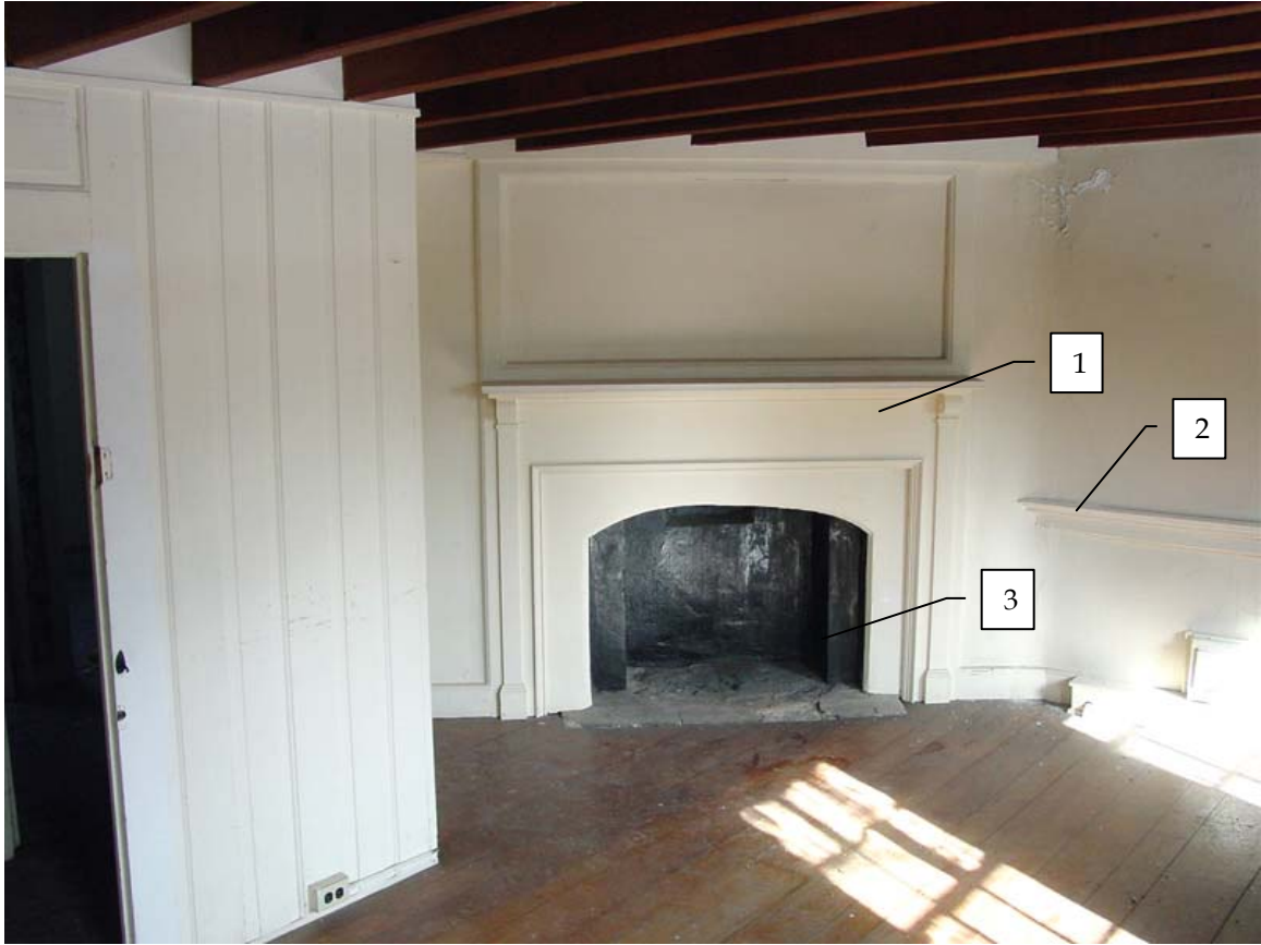
Photo 205c – View of east wall of Room 205, looking northeast.
