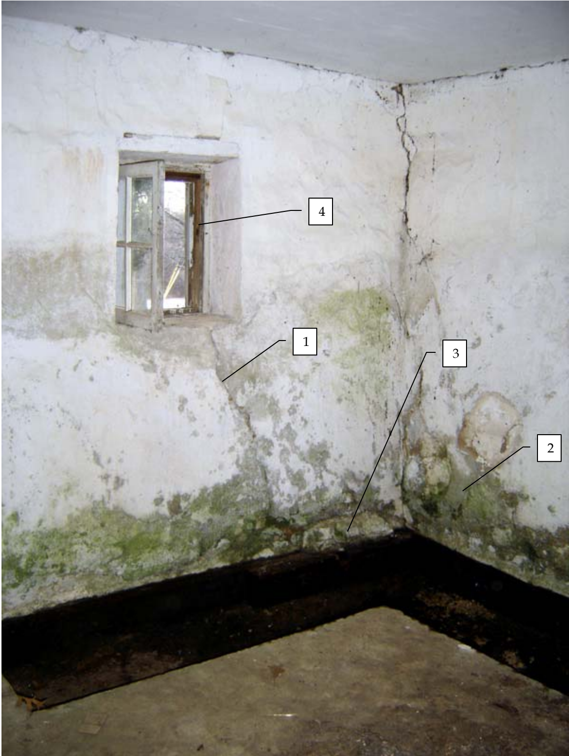
Photo 109b – Segment of springhouse interior, Room 109, looking southwest.
