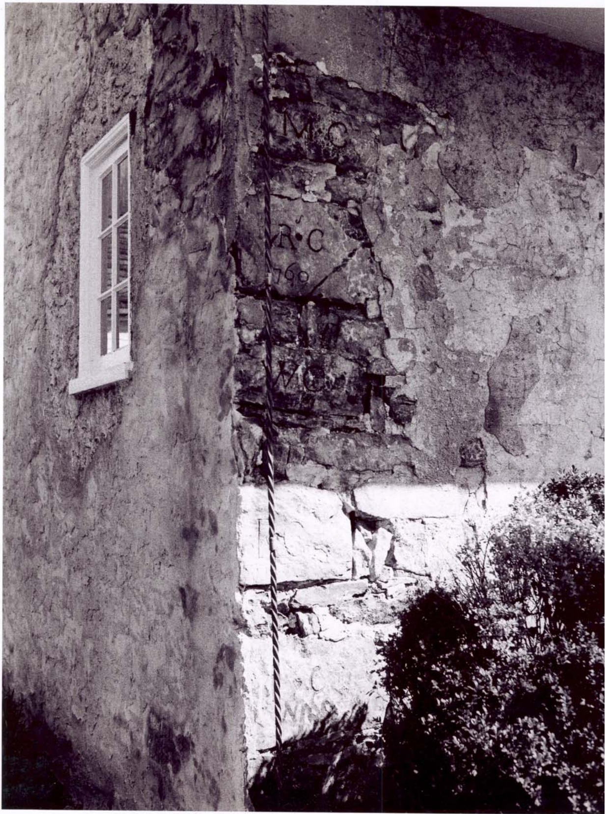
Archive Photo 1 Corner stones with inscribed initials and dates at southeast corner of west block.
