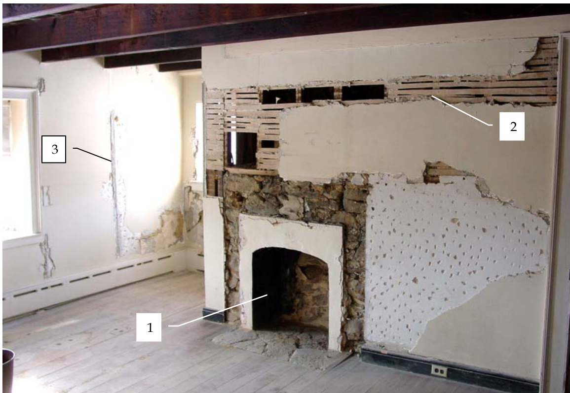
Photo 206a – Interior view of Room 206, looking southwest.
