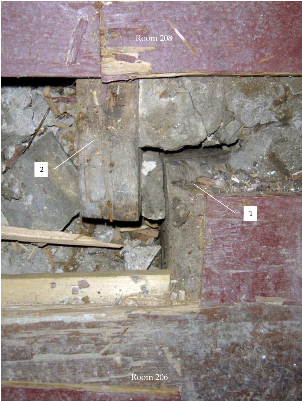
Photo 206d – Detail view of floor and framing (over masonry wall), between Room 206 (bottom) & Room 208 (top), looking down.
