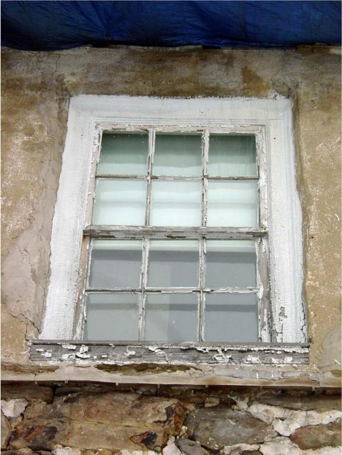
Photo SEh - Exterior view of Window 204, looking north.
