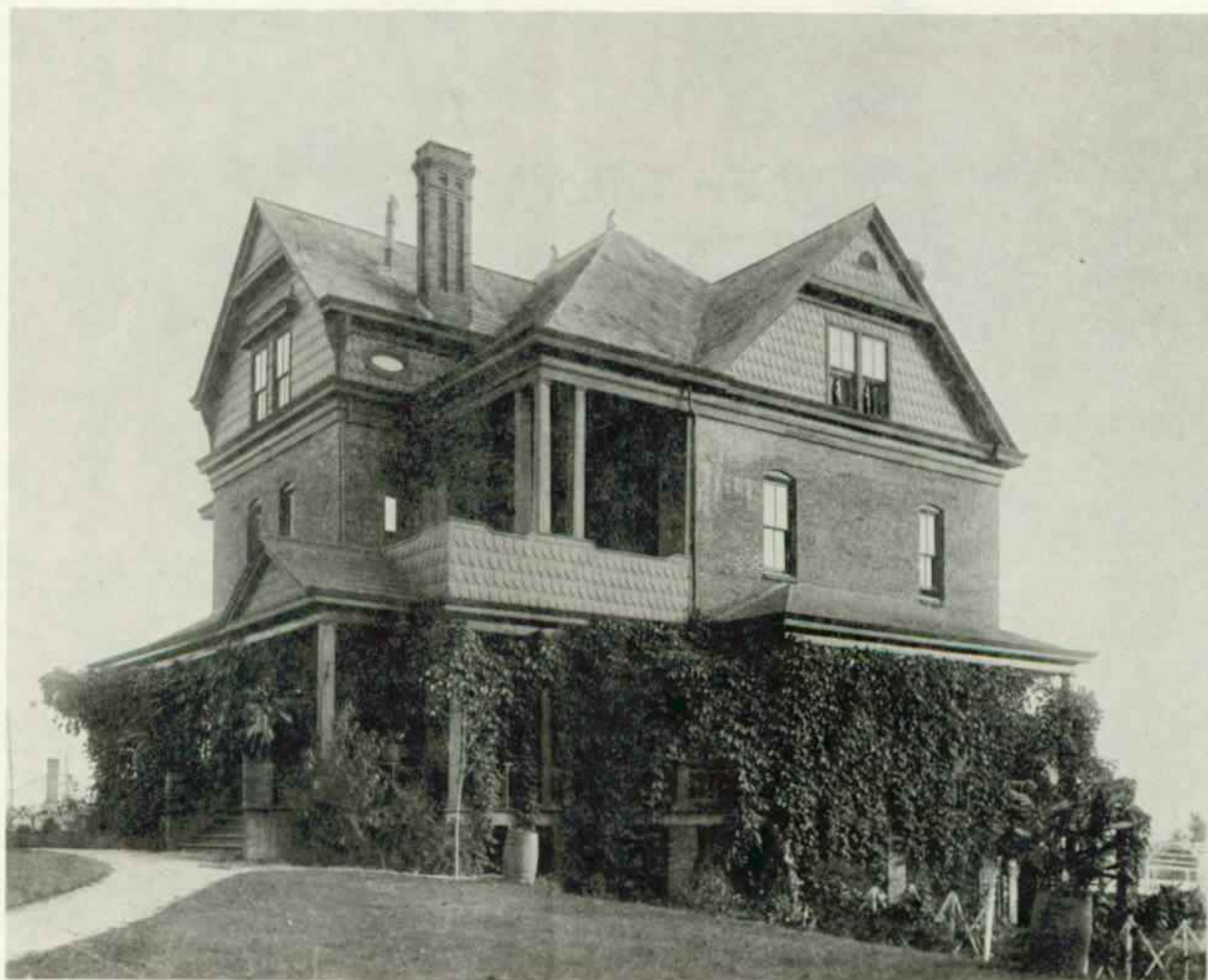
Figure 3. Northwest Corner of the Oaks, 1902. Note the construction of the veranda and porches, the interior window shutters, and the stovepipe for the third-floor north bedroom. (Frances Benjamin Johnston Collection, Library of Congress)
