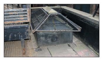
Detail of the corroded skylight and deteriorated mortar joints around terracotta pavers, JMI, 2006.
