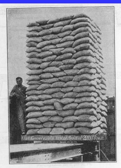
FIG. 2.—ARBITRARY TEST LOAD. SAND IN BAGS ON 4-IN. SLAB, 36 IN. WIDE AND 6 FT. LONG.
