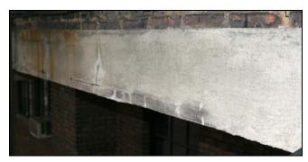
Detail of cracking, iron staining, and efflorescence on the reinforced concrete lintel (Room 308), JMI, 2006.
