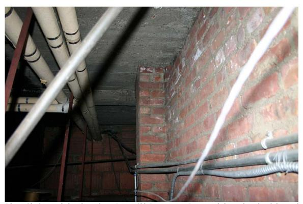
Photo 12. Suspended ceiling above Room 403 Preparation Room and the underside of the roof slab
