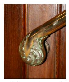
Detail of brass handrail and areas of green corrosion, JMI, 2006.
