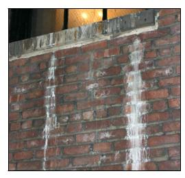
Areas of efflorescence under the window sill, JMI, 2006.
