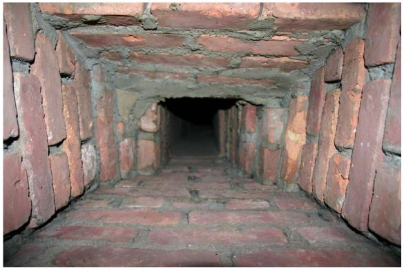
Photo 47. Chimney flue lined with clay masonry in Room 103 Front Parlor
