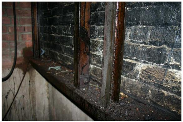
Photo 32. Brick masonry in the dumb waiter shaft above the Ground Floor
