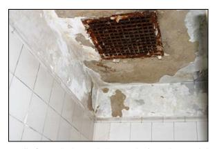
Detail of severely damaged plaster and paint and a corroded ceiling vent, JMI, 2006.
