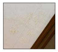
View of deteriorated plaster ceiling, JMI, 2006.
