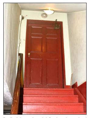
Detail of the metal paneled fire door, the metal and concrete staircase, and the wood hand rail, JMI, 2006.
