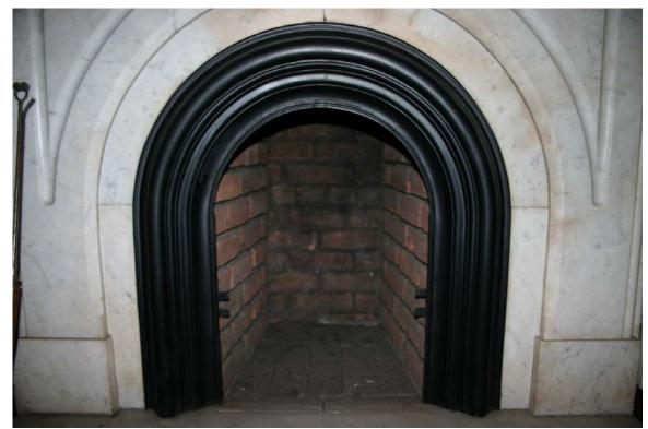
Photo 51. Chimney flue constructed of brick masonry and lined with clay tile in Room 104 Family Parlor
