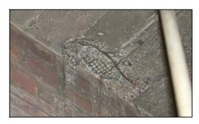
Area of the exposed metal lath and reinforcement at concrete ceiling, JMI, 2006.
