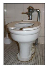
Detail of a toilet showing staining and deteriorated seal around the base, JMI, 2006.
