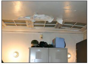
Deteriorated paint and plaster ceiling to the right of the ajar skylight, JMI, 2006.
