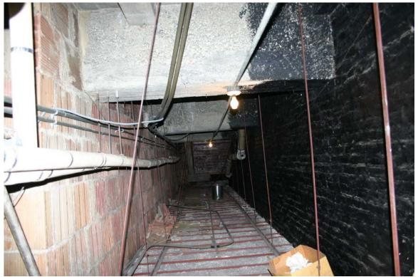
Photo 11. Suspended ceiling above Stair S-4 and the underside of the roof slab
