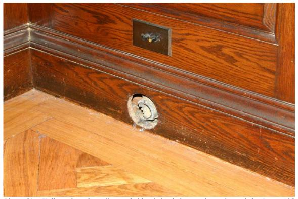
Photo 64. Hollow clay tile walls are hidden behind the wood paneling of the Room 405 Auditorium
