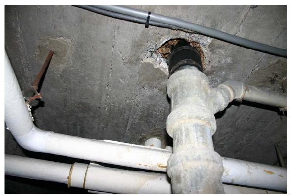
Photo 20. Typical floor penetration in the underside of the Ground Floor seen in the under floor space
