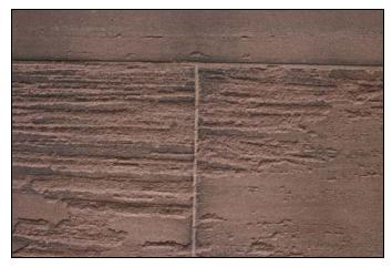
Detail of deteriorated brownstone units on the museum portion of complex of the north elevation, JMI, 2006.
