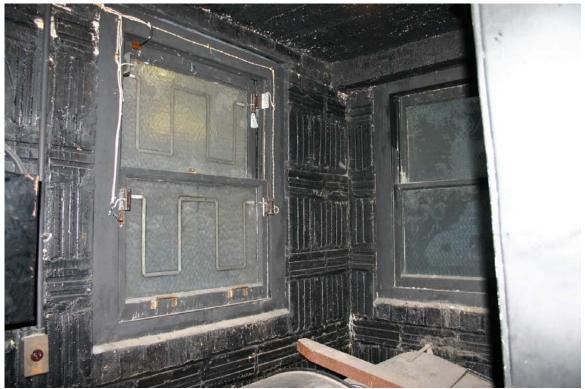
Photo 25. Hollow clay tile used in Room 503 Vent Room
