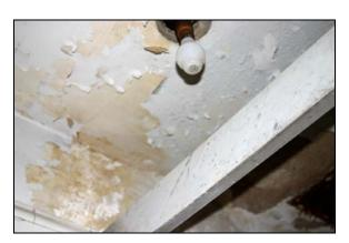
Detail of plaster and paint deterioration, JMI, 2006.
