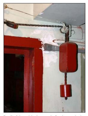
Detail of the weighted automatic fire door mechanics, JMI, 2006.
