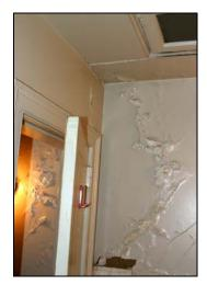
Detail of the east wall showing deteriorated paint and plaster, JMI, 2006.
