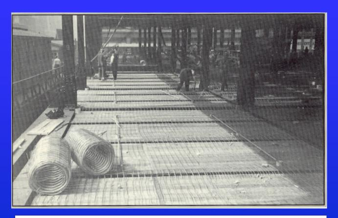
Slab forms with mesh and conduit
