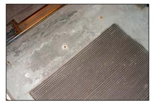
Detail of the metal floor grate and corroded ferrous remnants, JMI, 2006.
