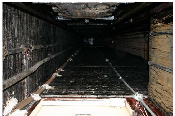
Photo 33. Brick masonry in the dumb waiter shaft above the Ground Floor
