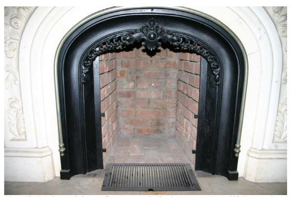
Photo 46. Fireplace and chimney flue constructed of brick masonry in Room 103 Front Parlor
