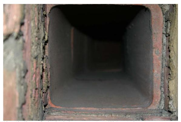
Photo 48. Chimney flue lined with clay masonry in Room 103 Front Parlor
