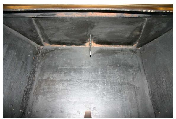
Photo 54. Chimney flue in Room 310 Archive Storage concealed by metal lining with closed vent
