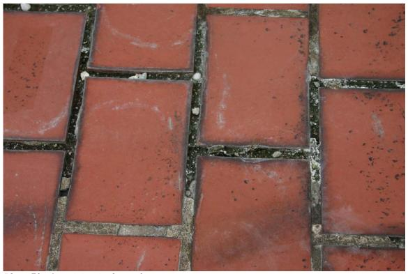
Photo 70. Open joints in the roof top terrace pavers
