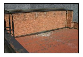
View of roof deck looking west showing areas of efflorescence, staining, and soiling, JMI, 2007.
