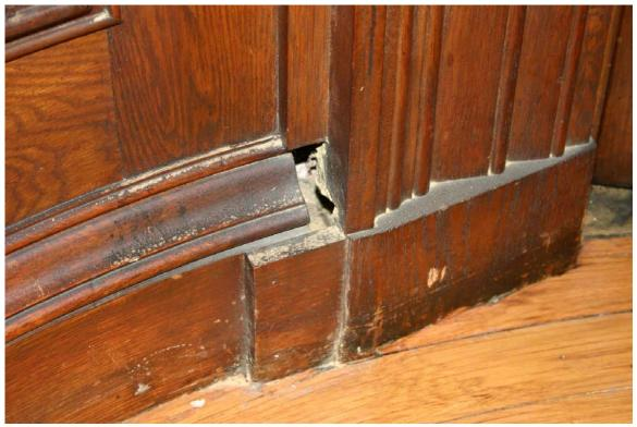
Photo 63. Hollow clay tile walls are hidden behind the wood paneling of the Room 405 Auditorium
