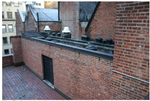
Photo 71. Open joints in the exterior brick masonry of the roof top penthouse with repointing near the top of the wall
