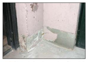
Detail of damaged paint and stucco at base of the walls in the entrance vestibule, JMI, 2006.
