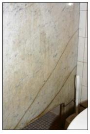
Detail of cracks and staining along wall of the marble stall, JMI, 2006.
