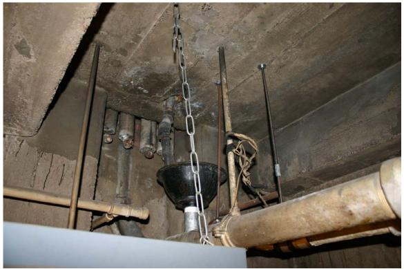
Photo 27. Abandoned piping and conduit in the pipe chase in Room B-05
