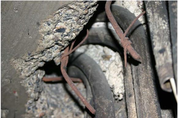
Photo 7. Floor penetration in the ceiling above Stair FS-0 with exposed wire reinforcement in the slab with wire oriented in the north-south direction (wire measures 0.238 to 0.240 inch in diameter and spaced at 4-1/2 inches on center)
