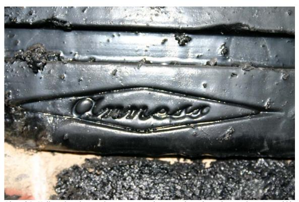
Photo 24. Hollow clay tile manufacturer seen in the space above the archive vaults in Room 309
