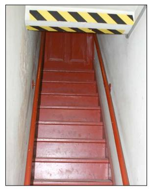
View of the metal paneled fire door, the metal and concrete staircase, and the metal hand rails, JMI, 2006.
