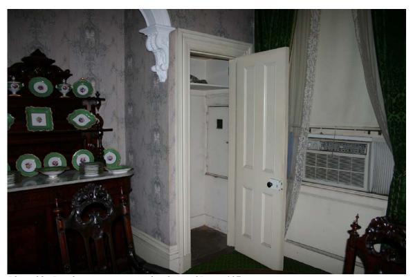
Photo 38. Dumb waiter access in the closet of Room 107
