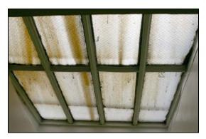
Deteriorated metal and glass in the skylight, JMI, 2006
