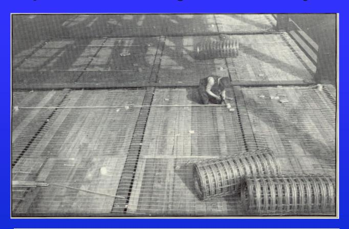
Slab forms with mesh and conduit
