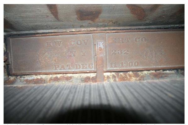
Photo 56. Chimney flue in Room 306 Office concealed by metal lining and closed vent
