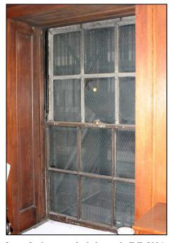
Loss of paint on steel window sash, JMI, 2006.
