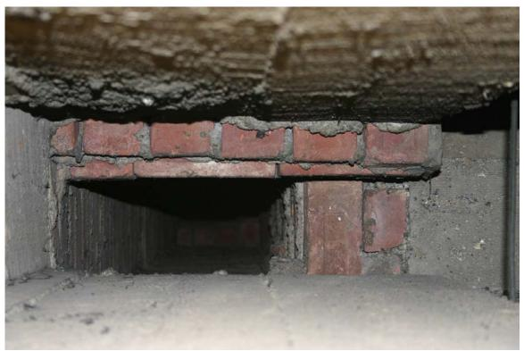
Photo 29. Empty pipe chase in the east foundation wall adjacent to Room B-03 Restroom
