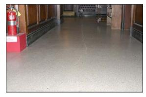
Detail of a major crack in the terrazzo floor extending the length of the hall, JMI, 2006.
