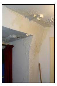
Detail of paint and plaster deterioration on walls, JMI, 2006.
