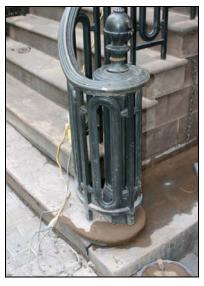
**Figure 25:** Jahn mortar patches on the entrance brownstone stairs, JMI, January 2007.
