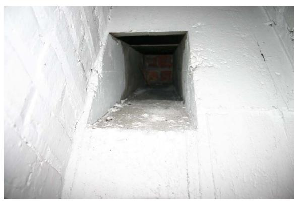
Photo 6. Formed opening in the concrete foundation wall at the ceiling with brick closure in the fireplace clean out shoot in Room B-01 Hallway
