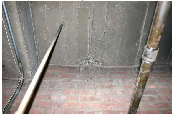
Photo 8. Floor penetration in the ceiling above Room B-06 with exposed wire reinforcement in the slab with wire oriented in the north-south direction
