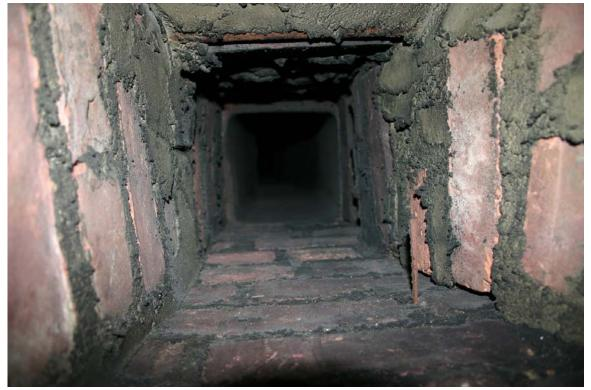
Photo 52. Chimney flue constructed of brick masonry and lined with clay tile in Room 104 Family Parlor
