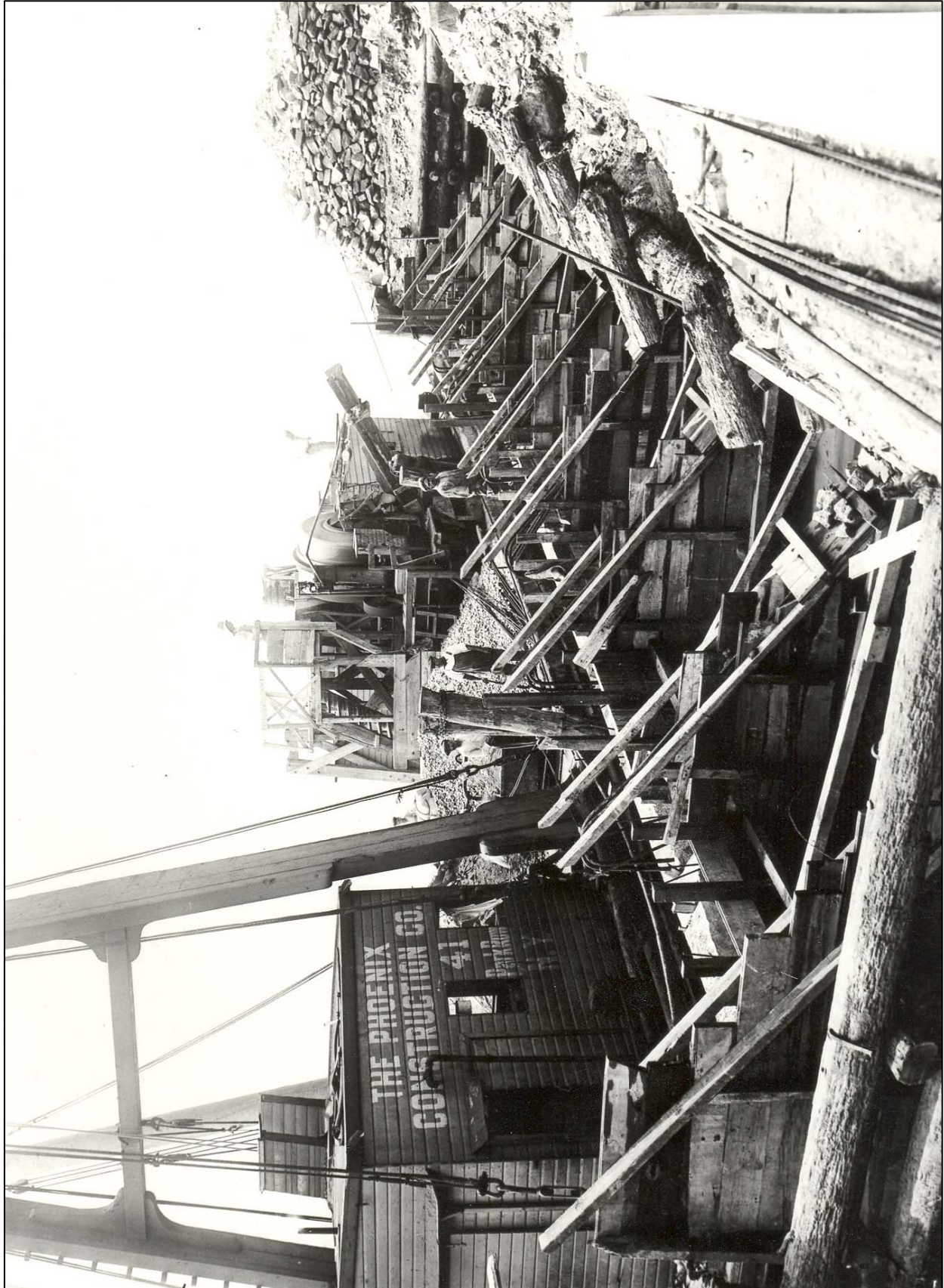
Figure 28. Construction of concrete counterforts on top of Island Two or Three cribwork, 1917.
