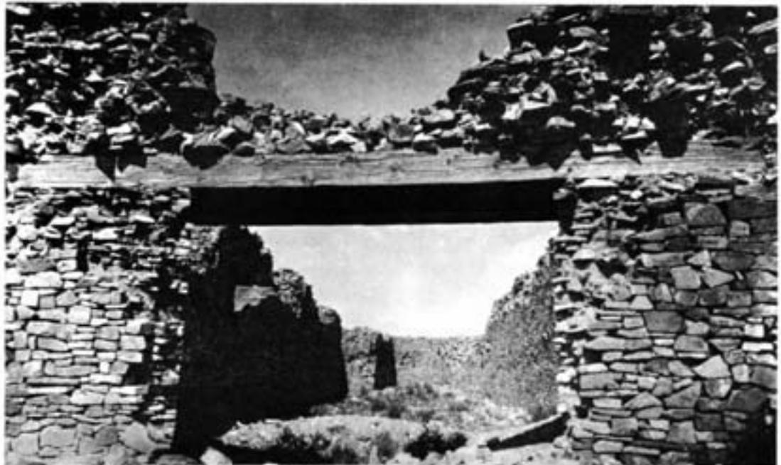
FIGURE 26 San Buenaventura in 1890 when the lintels remained over the entrance at the east, and one of the corbels under the choir loft was in place in the south wall. (Southwest Museum.)
