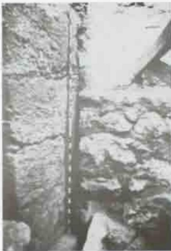
Figure 26. Photograph of the Construction Seam Between the ca. 1002 Ocellus Corner and the Filled Ocellus Area.
