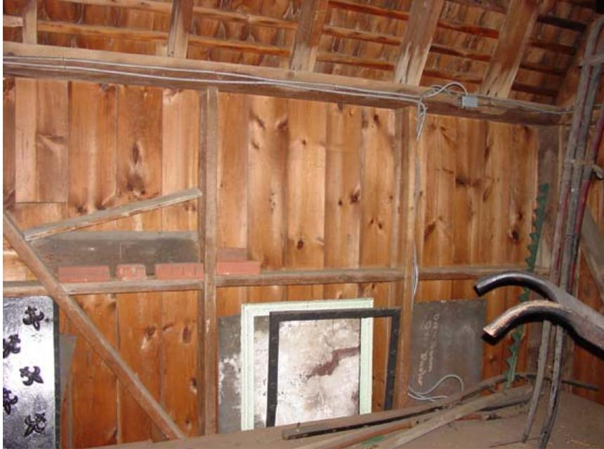
**Figure 21.** New Barn, north- elevation framing, interior view of northeast section showing 2 by 6 studs, blocking and bracing, plate, and corner post (2005).
