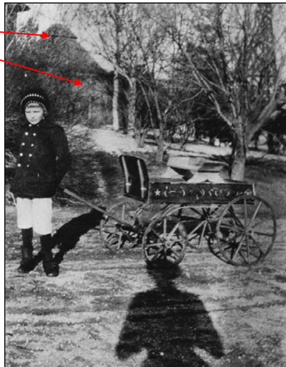
Figure 69. Archie Roosevelt with wagon, Ice House and lattice in background, 1901.
