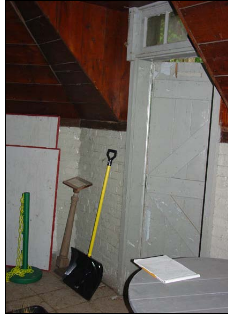
Figure 81. Ice House: South room looking southeast, 2007.
