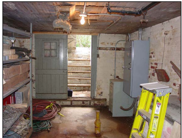
Figure 94. Pump House: South room and bulkhead entry, looking south, 2007.
