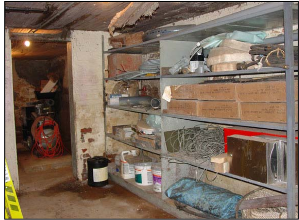
Figure 95. Pump House: Interior south room looking north, 2007.
