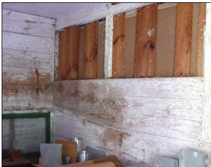
Figure 49. Chicken House: Room 102, east partition wall and evidence of roost on both the north and east walls, 2007.
