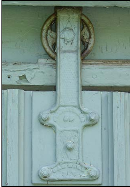
Figure 28. Gardener's Shed: Door roller and track, 2007.
