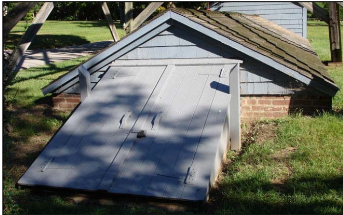
Figure 93. Pump House: South elevation with new bulkhead cover, 2007.
