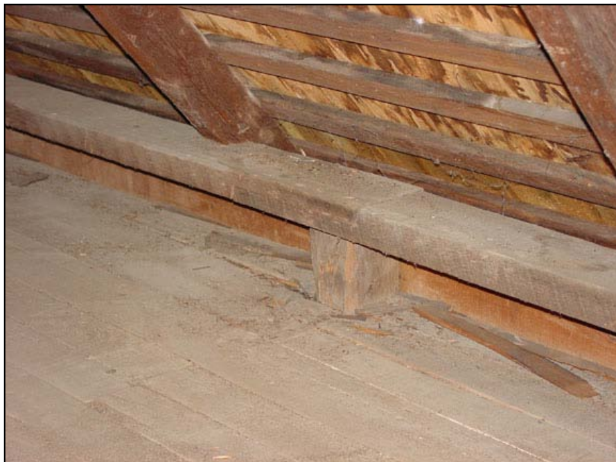
Figure 67. Chicken House: Loft, south elevation post, plate and common rafter, 2007.
