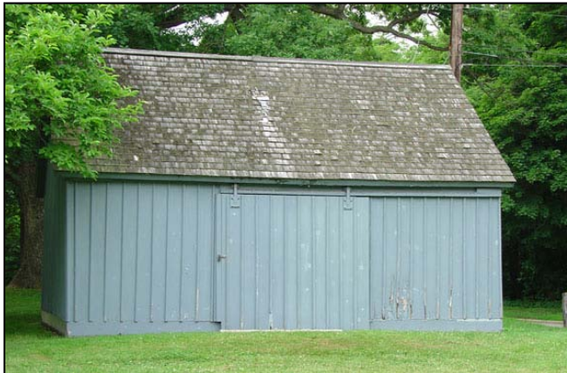
Figure 26. Gardener's Shed: East elevation, 2007.
