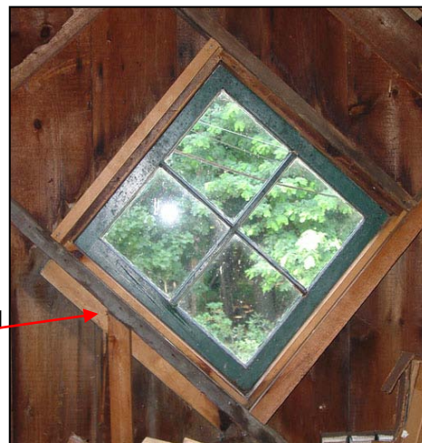
Figure 30. Gardener's Shed: Interior of north gable window and sash, 2007.
