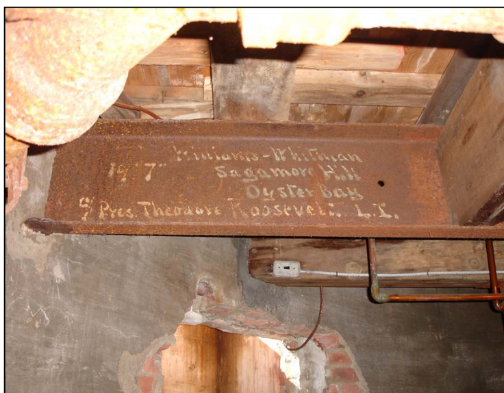
Figure 72. Steel beam in the basement/cistern of the Ice House, inscribed with the address and date, 2007.
