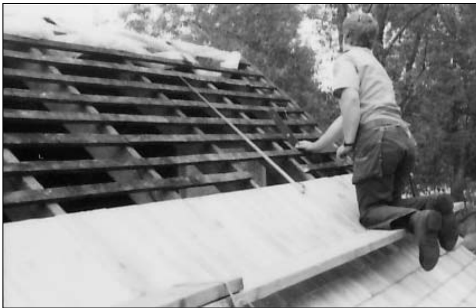
Figure 57. Chicken House: Repairs to roof, including replacement of wood lath and installation of wood shingle roof, 1986.
