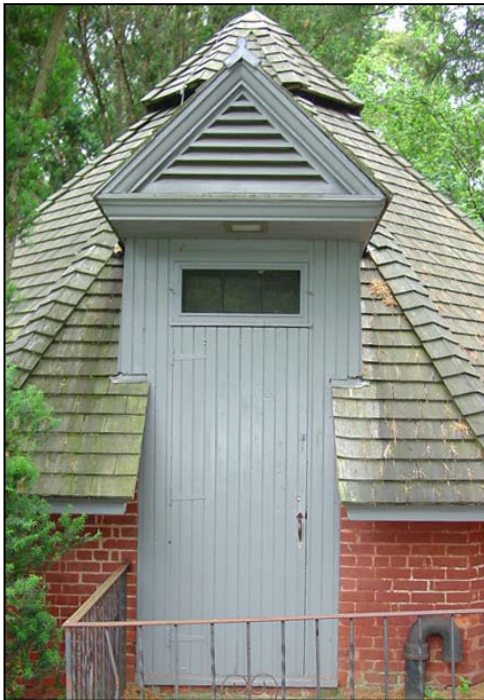
Figure 77. Ice House: North Entry Doorway, 2007.
