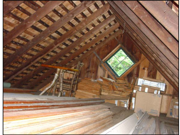
Figure 32. Gardener's Shed: Interior of loft looking north, 2007.
