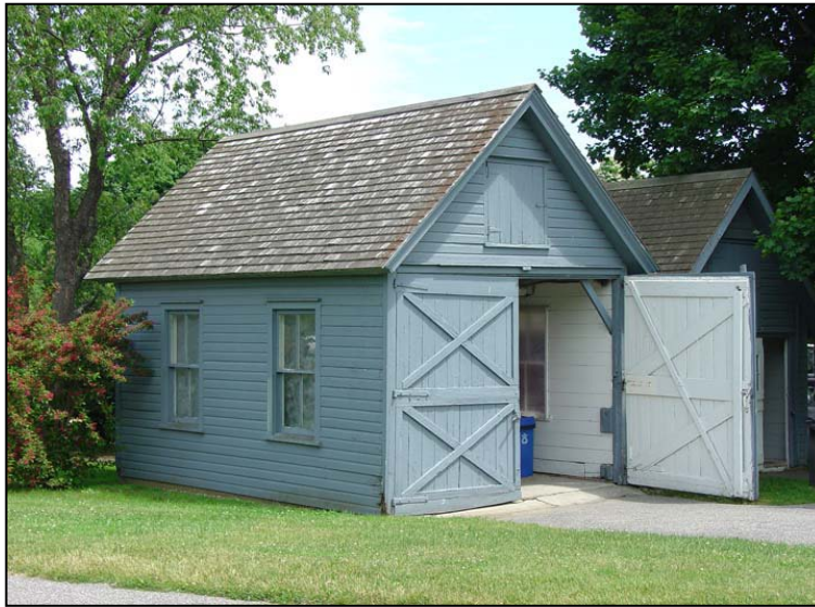
Figure 5. Farm Shed: North and West elevations, looking southeast, 2007.
