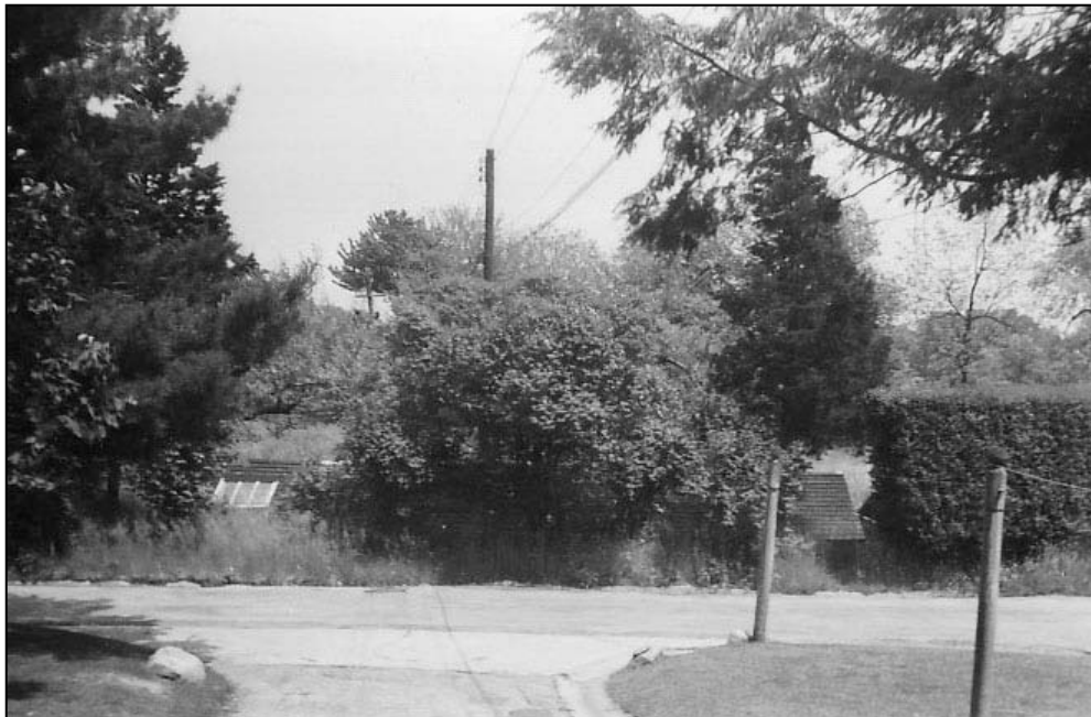
Figure 85. Pump House: Looking east, 1950. Note green-house type window on west side of roof and absence of windmill.
