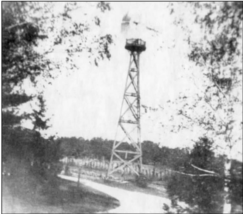
Figure 84. Windmill at Sagamore Hill with pump house at base of structure, ca. 1905.
