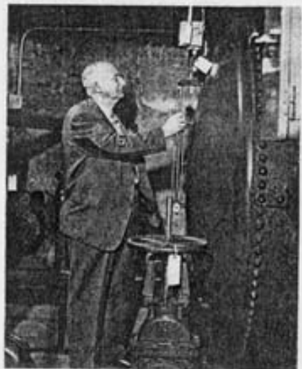
Interior of Pump House
