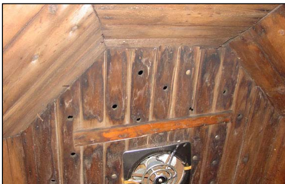
Figure 71. Ice House: Ceiling near peak of roof, original tongue-and-groove boards with vent holes (modern fan), 2007.
