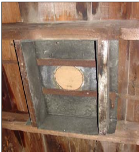
Figure 33. Gardener's Shed: Framed stovepipe opening, 2007.
