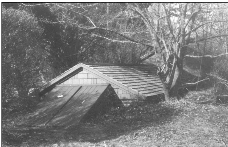
Figure 88. Pump House: Looking northwest, 1969. Hose Reel House depicted at north end of Pump House.
