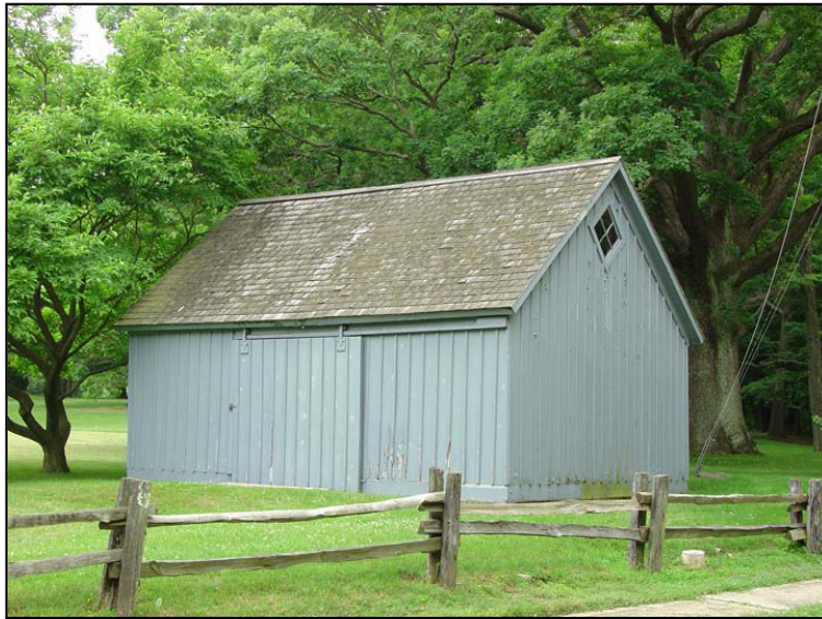
Figure 4. Gardener's Shed: East and North elevations looking southwest, 2007.
