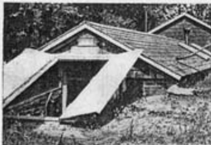
Pump House Used for Water Supply and Fire Protection Control Equipment
