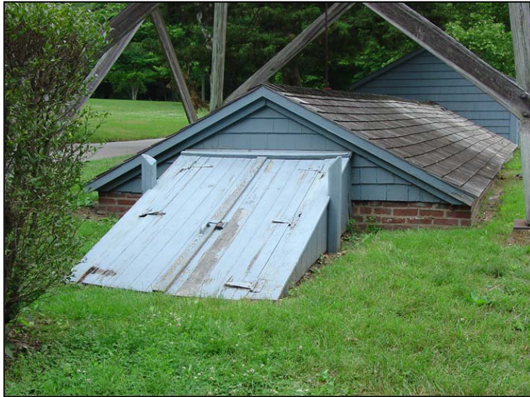
Figure 8. Pump House: South elevation, looking north, 2007.
