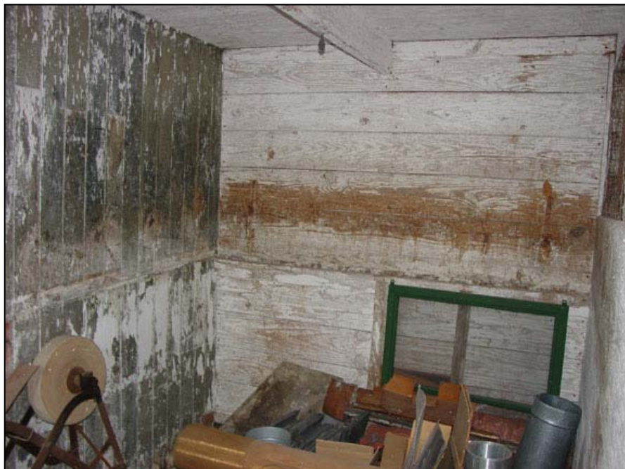
Figure 63. Chicken House: Room 102, looking northwest, 2007.
