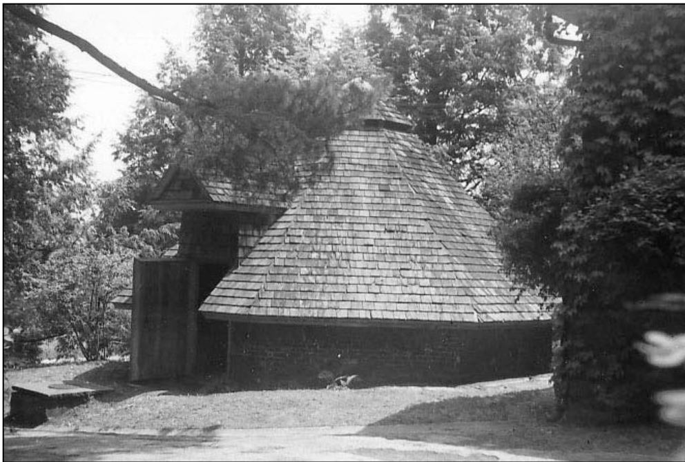
Figure 68. Ice House at Sagamore Hill: Looking southeast, June 1950.
