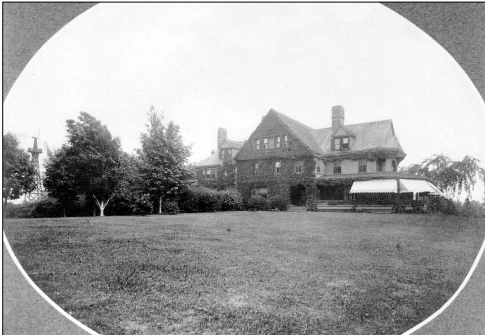
Figure 82. Sagamore Hill: Prior to 1905 North Room addition. Note early windmill on left side of image.
