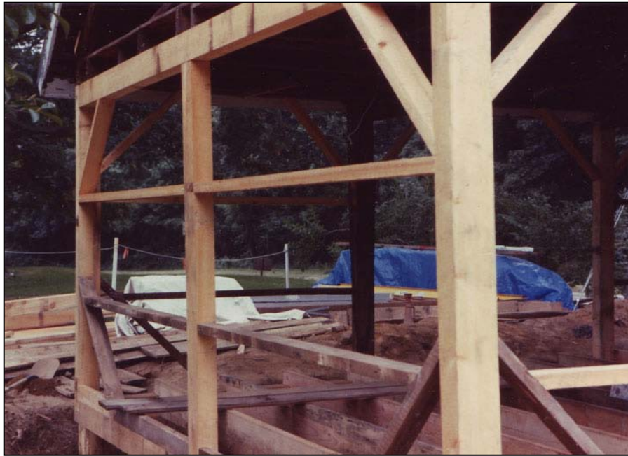
Figure 25. Gardener's Shed: South elevation showing in-kind replacement framing, 1986.
