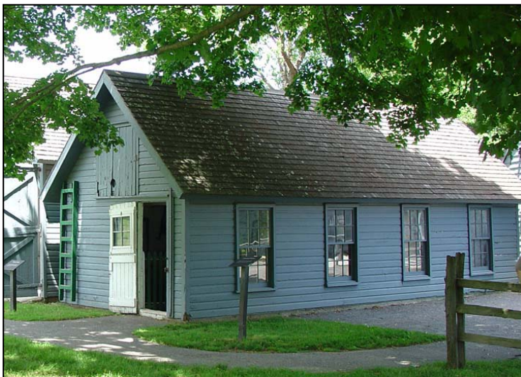
Figure 6. Chicken House: South and West elevations, looking northeast, 2007.
