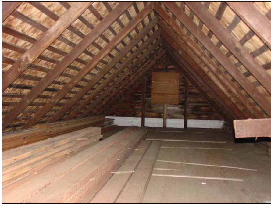
Figure 66. Chicken House: Loft, looking east, 2007.
