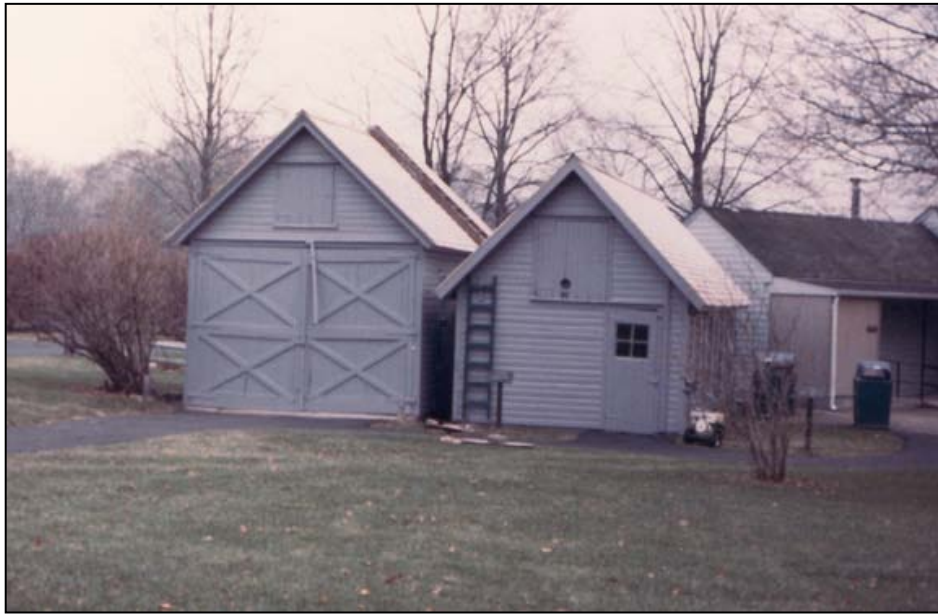
Figure 58. Chicken House and Farm Shed: Completion photograph of west elevations, 1986.
