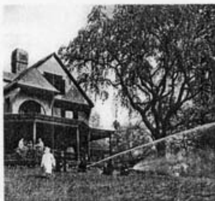
Test of Fire Streams at Sagamore Hill
