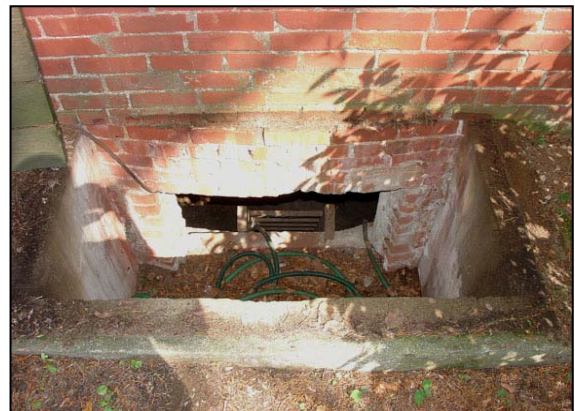
Figure 76. Ice House: Window well on southeast elevation, 2007.
