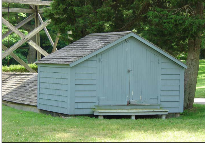
Figure 96. Hose Reel House: North elevation, 2007.
