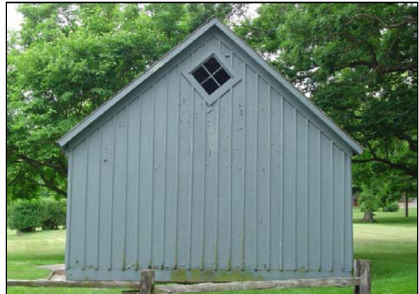
Figure 27. Gardener's Shed: North elevation, 2007.
