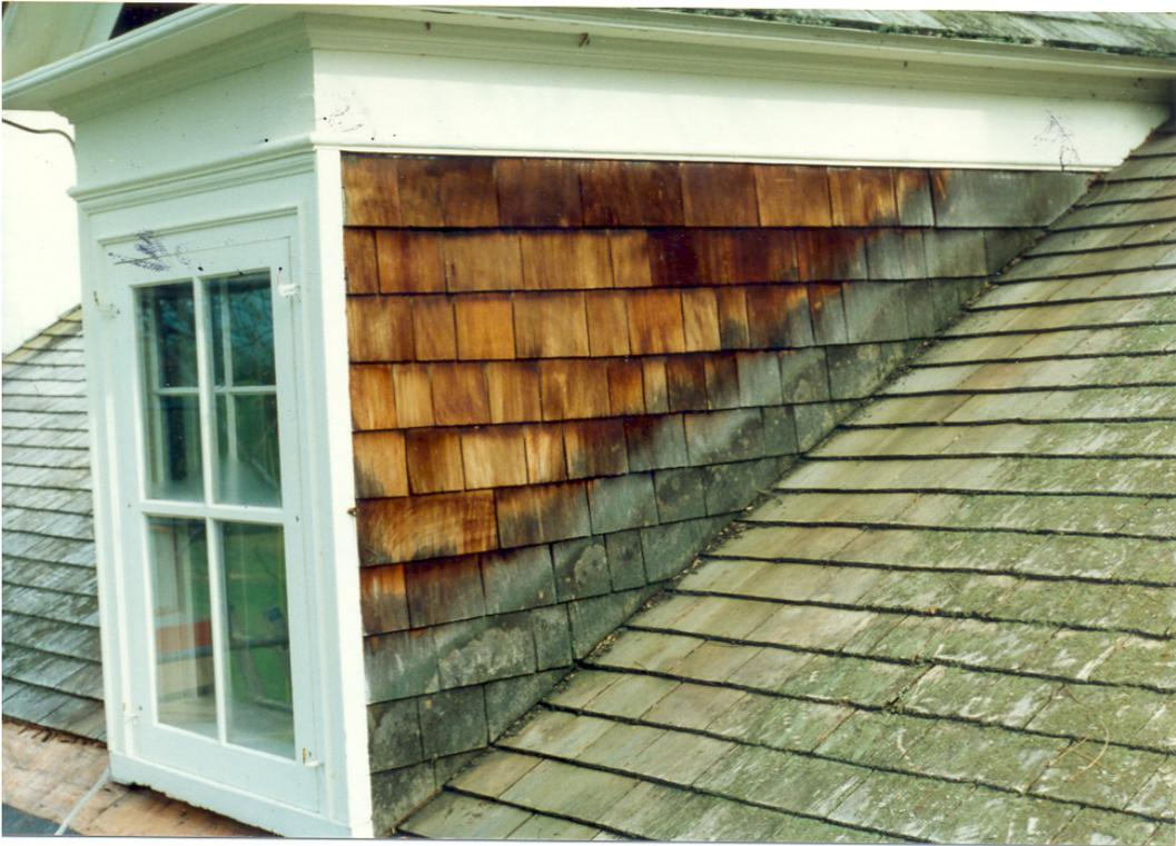
Figure 59. Aspet, dormer showing mold and water damage to shingles; mold and moss also covers adjacent roof shingles, 1993.
