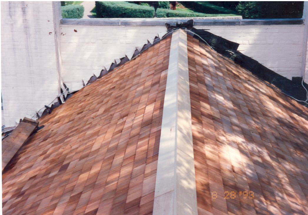
Figure 60. Aspet, new roof ridge, flashing, and shingles, 1993.
