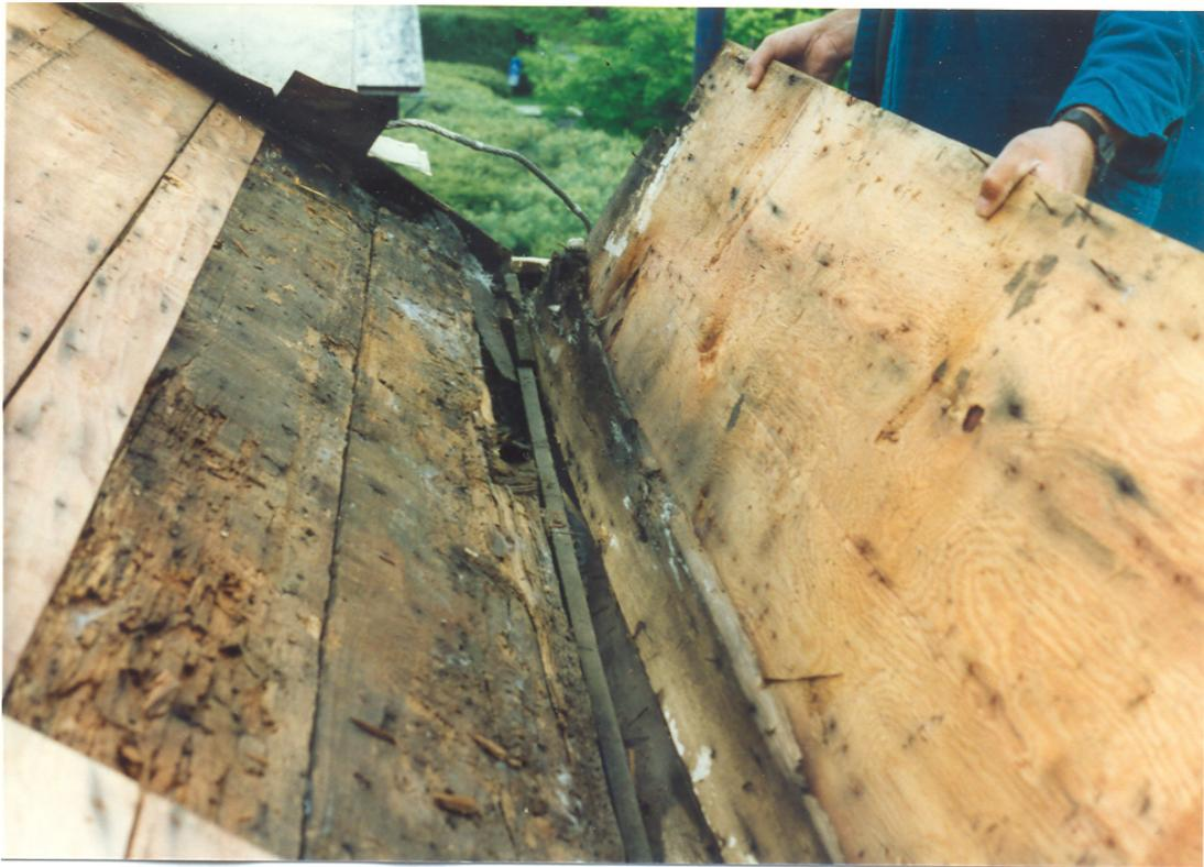
Figure 57. Aspet, rotten sheathing boards exposed, 1993.
