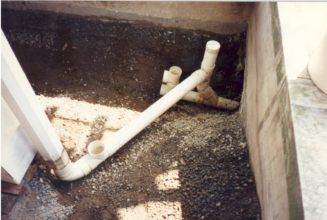
**Figure 106.** Little Studio, drainage project: new PVC pipe for downspout connection at southwest corner of pergola, 1994.
