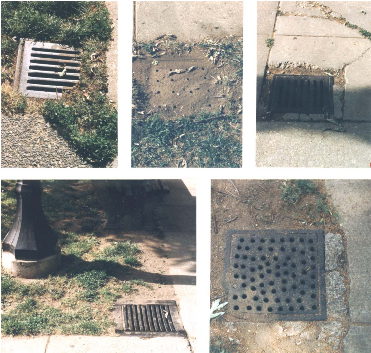
These pictures illustrate the diversity of non-original catch basin inlet covers found in the park. The one located in paving (obscured by the light fixture shadow) is an original location for a catch basin, but has had paving added around it. The steel plate inlet covers with holes are apparently expedients to replace the original brass covers, which have been stolen.
