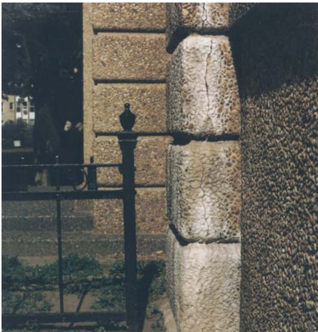
(above left) An example of cracks and efflorescence, on the northern wall of the park, looking west from the children's play area. This fence finial is the only one still in place on the fence at this play area.
