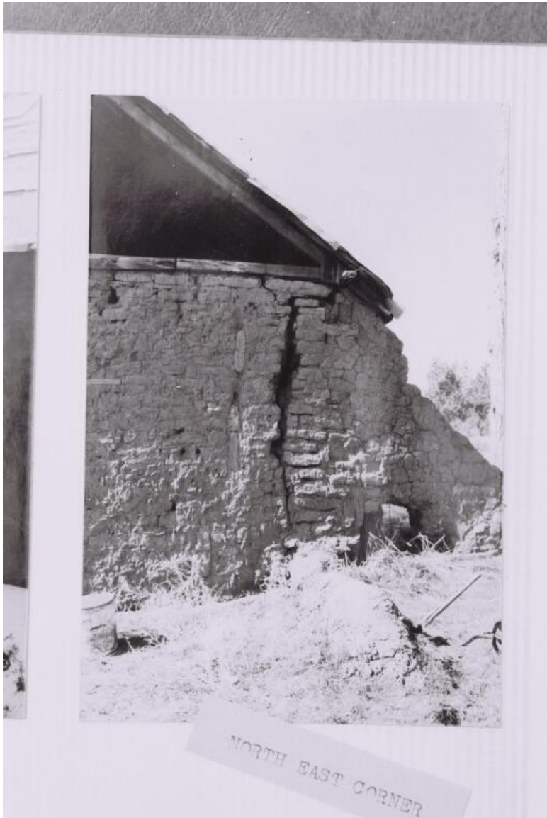
Northeast corner before collapse showing separation of wall from main building, February 23, 1983.
