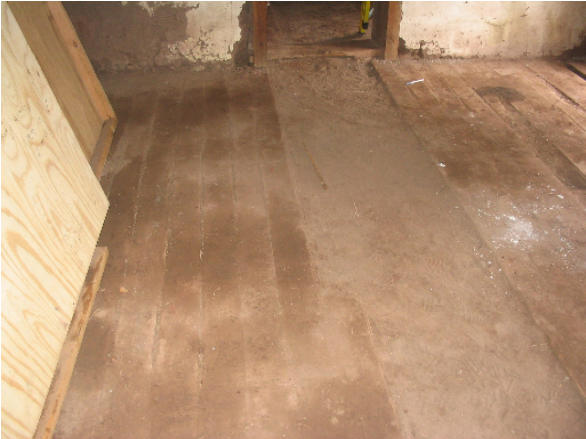
Floor finishes, west room.
