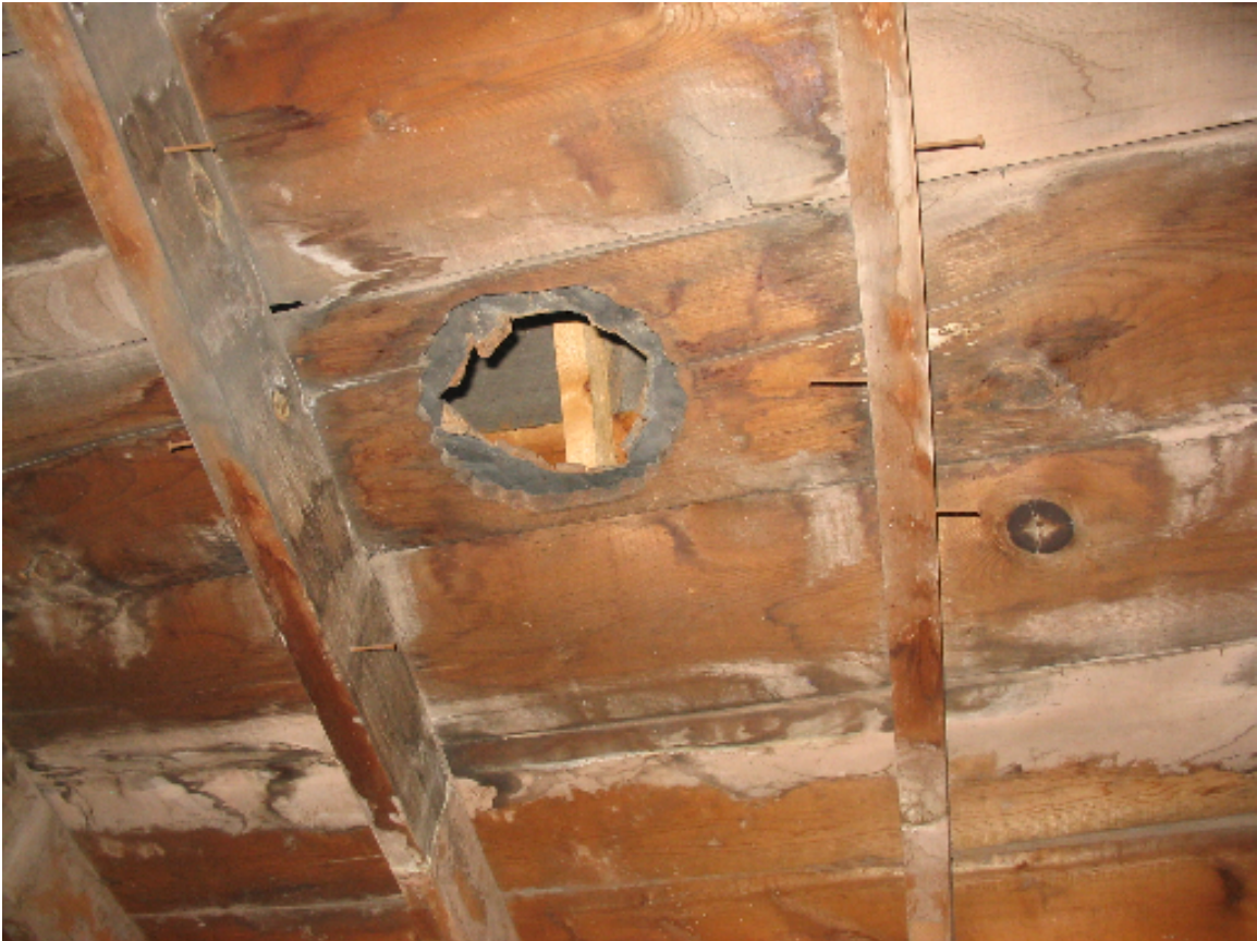
Ceiling stove chimney hole, west room.
