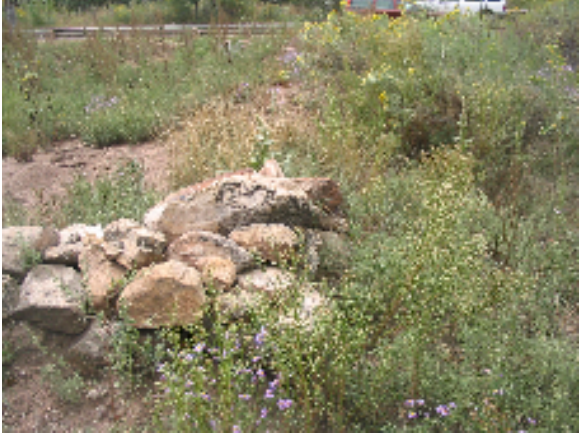
West wall from corner looking south
