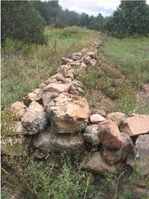
North wall from corner looking east
