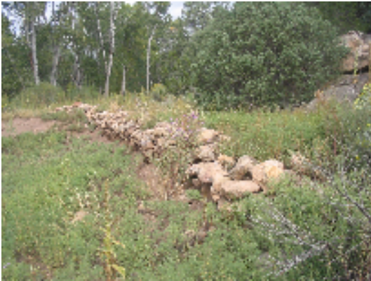
North wall looking west
