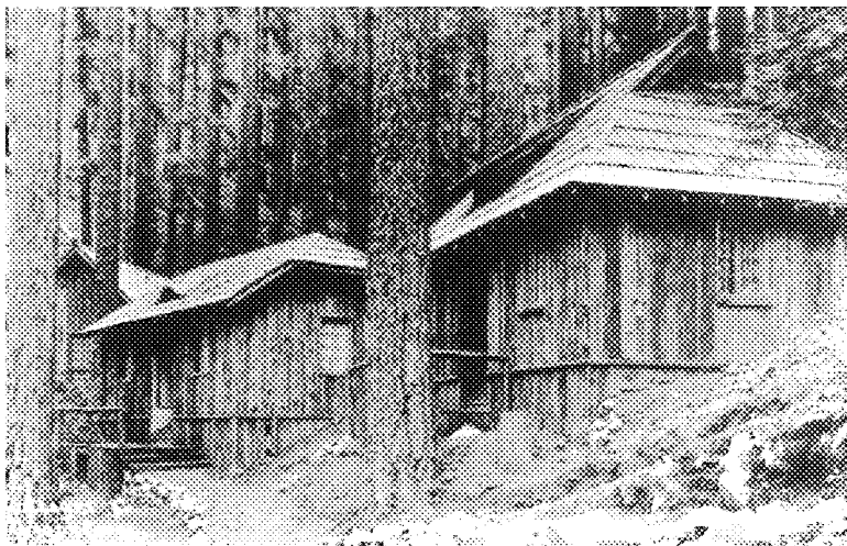
FIGURE 38. Resort cabins or “cottages” at Oregon Caves. (Photo by Frank Patterson, OCNM Museum and Archives Collections.)
