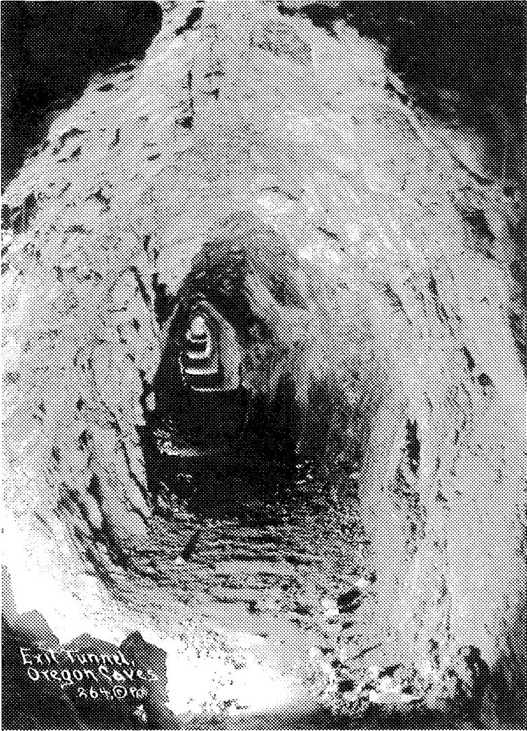
FIGURE 39. Newly completed exit tunnel, 1931. (Photo by Frank Patterson, OCNM Museum and Archives Collections.)
