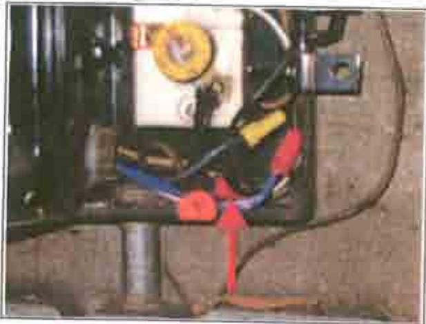
**Component:** Load side red wire nut connection on purple wire below fused disconnect switch.
