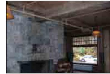
**Figure 5.2:** Exposed Sprinkler Piping in Main Lobby
