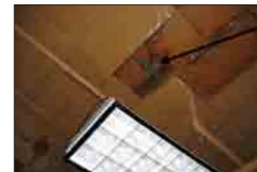
**Figure 4.9:** Missing Ceiling Panels Exposing Framing at First Basement
