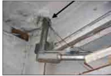
Figure 4.2: Third Basement Stairway Fire Separation Deficiencies
