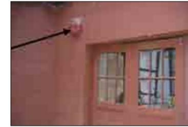
**Figure 4.19:** Sprinkler Water Motor Gong (Note: This is the only sprinkler activation alarm.)
