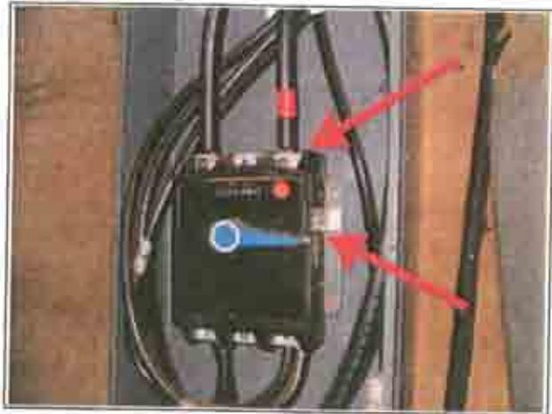
**Component:** Right phase line side wire lug connections or internal problem in circuit breaker
