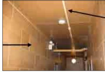
**Figure 4.13:** Non-fire rated fiberboard panel wall and ceiling finish throughout First Basement through Third Floor
