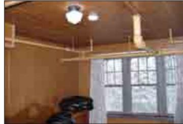
Figure 4.22: Exposed Sprinkler Piping in Guest Room
