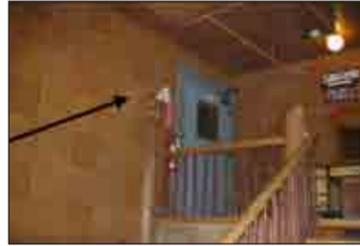
**Figure 4.14:** Non-fire rated walls around Fire Doors
