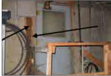
Figure 4.3: Close Proximity of Propane HW Heater and Boiler Burner
