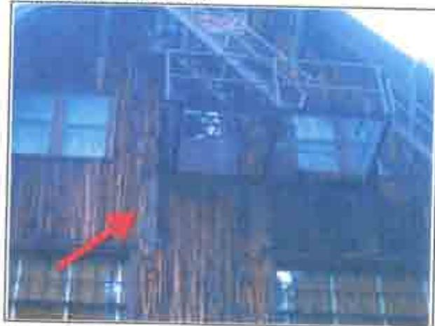
**Component:** Small temp difference around north 2nd floor mounting bracket of fire escape, possible moisture problem or other anomaly.
