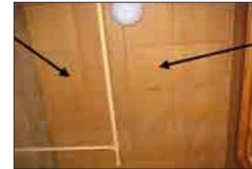
**Figure 4.8:** Gaps at Ceiling Fiberboard Panels (Typical Throughout at First Basement through Third Floor)
