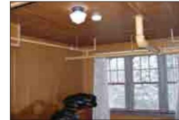
**Figure 5.3:** Exposed Sprinkler Piping in Guest Room
