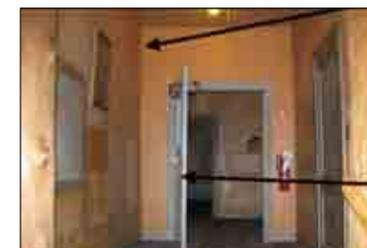
**Figure 4.12:** Fire Door to Guest Wing at First Floor held open, Non-fire rated wall
