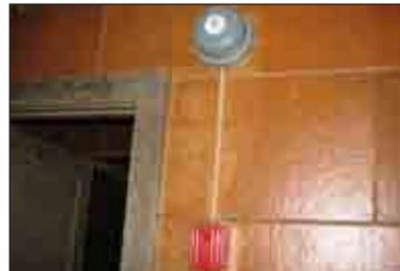
**Figure 4.16:** Typical Alarm Bell and Manual Alarm Station
