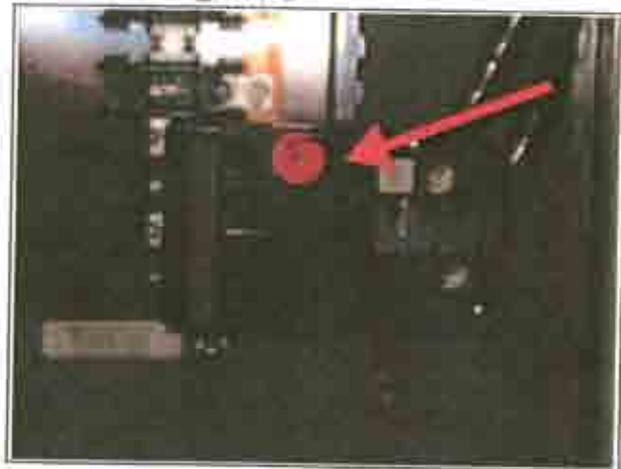
**Component:** Upper phase heating possible internal problem in circuit breaker #24,26,28,30 sub pnl upstairs.
