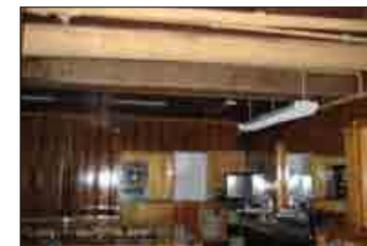
**Figure 4.10:** Lack of Fire Separation between Kitchen and Coffee Shop at First Basement
