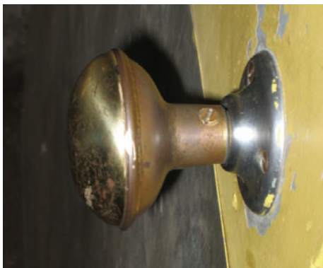
Figure C-79. Chrome, Type U escutcheon from 1950-51 era and replacement doorknob.
