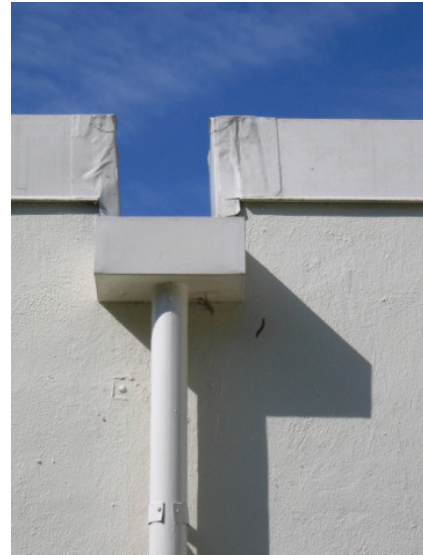
Figure C-5. Scuppers and external Downspouts added 1999.
