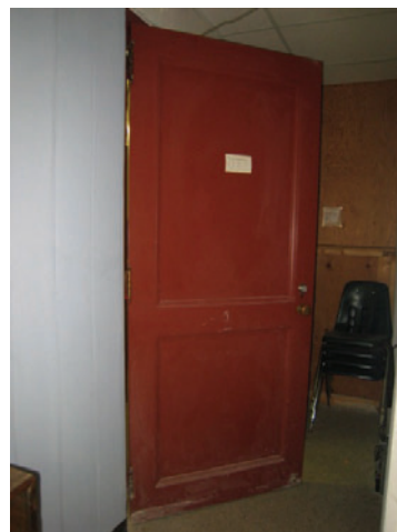
Figure C-17. 1938-41 metal-clad door.
