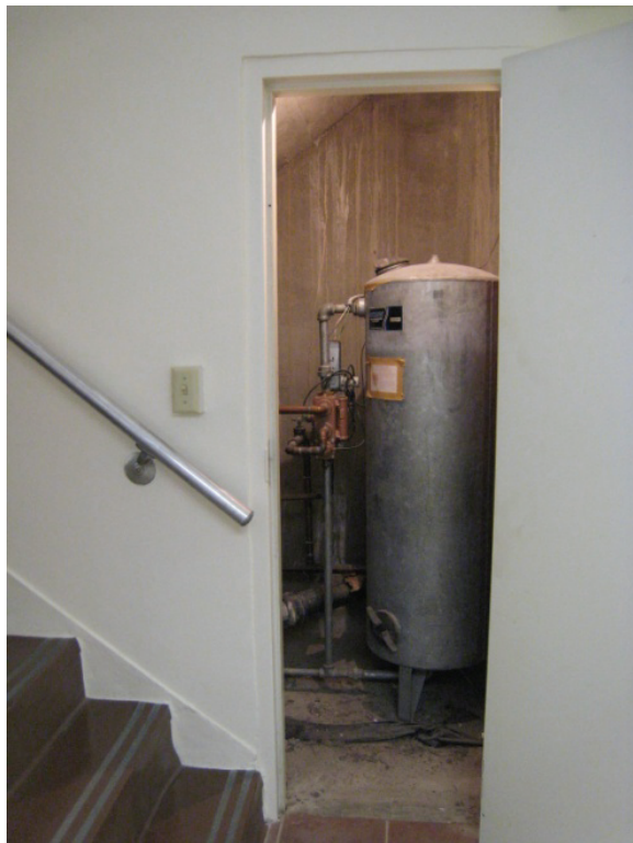
Figure C-63. Abandoned back-flush tank for solar panels.
