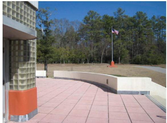
Figure C-6. New pavers at east terrace.
