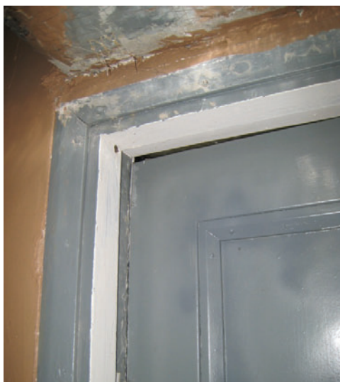
Figure C-91. Beveled molding of door and door casing dating to 1938-41.
