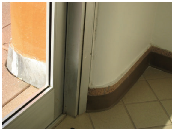
Figure C-100. Vinyl baseboard applied over original terrazzo baseboard.
