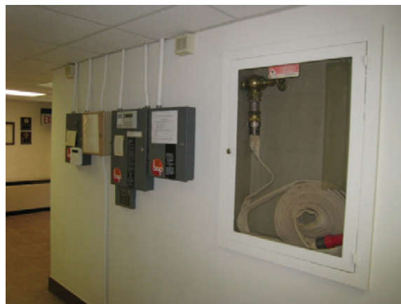
Figure C-56. Security control panels and 1950-51 fire hose cabinet at west wall.
