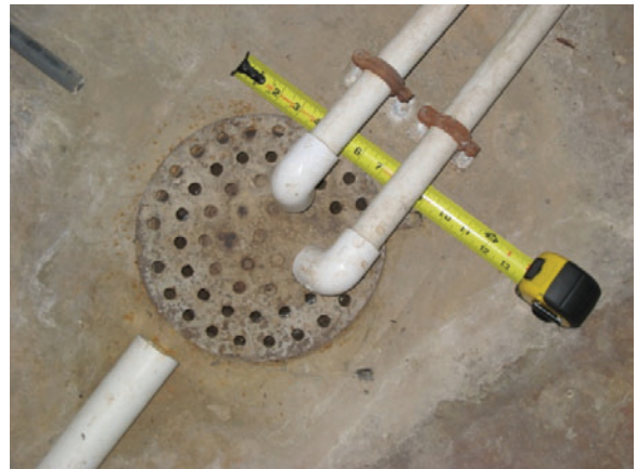
Figure C-20 Typical 10" floor drain.
