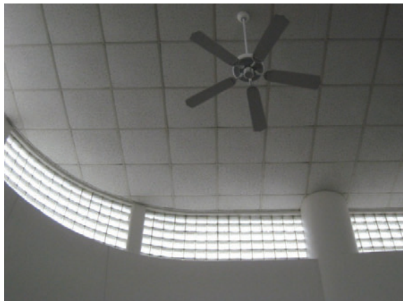
Figure C-103. A band of glass blocks.
