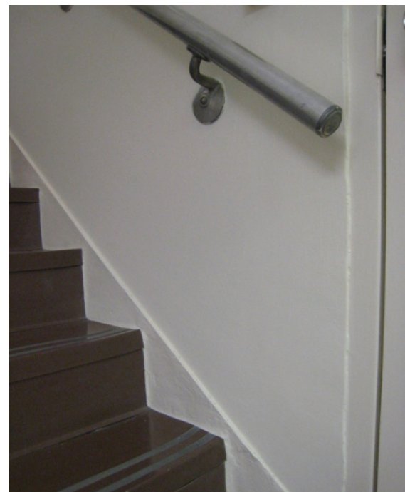
Figure C-62. Original 1950-51 aluminum handrail.
