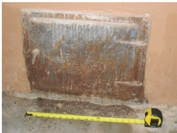
Figure C-96. Hatch for Chimney.
