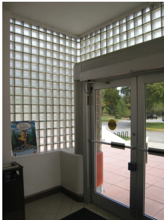
Figure C-99. Replacement doors in original door frames of main entrance.
