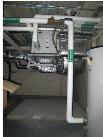
Figure C-35. Mechanical room (Room 007B) looking north. Gas hot water heater at right.
