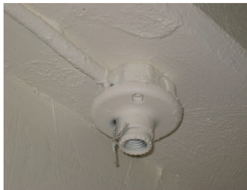
Figure C-87. Typical ceramic base lighting fixture for an incandescent light bulb.
