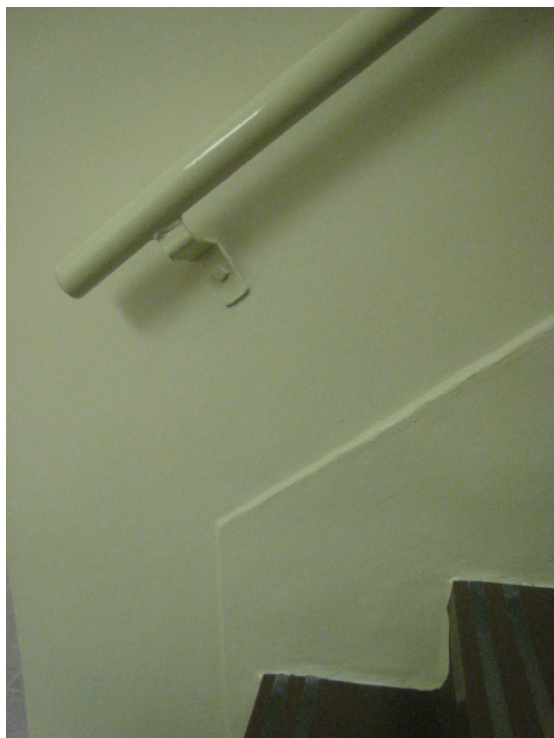
Figure C-43. Cast-cement baseboard and painted steel handrail.
