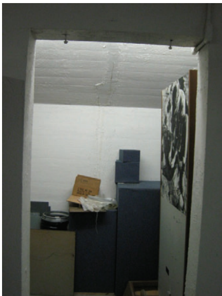
Figure C-21. Doorway to Room 002 with header bolts still present and formwork imprints in the concrete.
