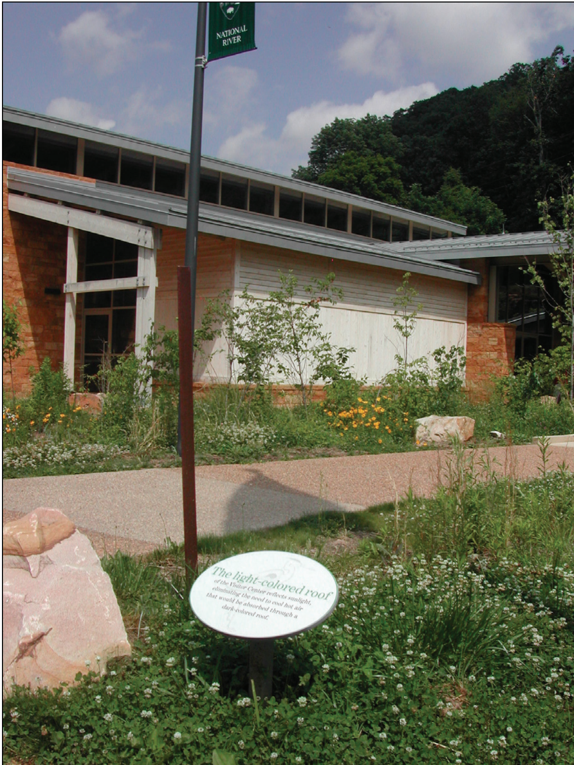
Figure 57. Sandstone Visitor Center is a "green building," including the reflective roof, locally sourced materials, certified wood, and careful attention to storm water runoff, 2004. Photograph by Gregory A. Good.
