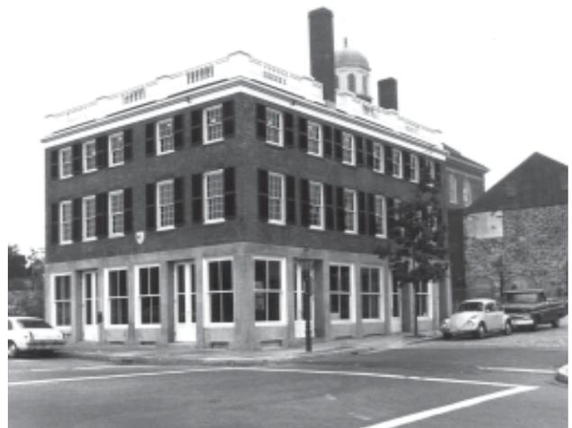
Figures 133 (left) and 134 (right): The Sundial Building, Union and North Water Streets, 1977 and 1980. WHALE restored the Federal-style building to its 1850 appearance after fire destroyed the roof and a portion of the walls.
