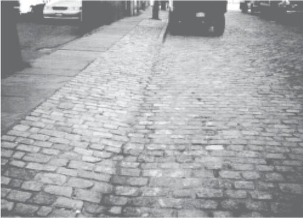
Figure 141: Typical curb cut for driveway and parking lot entrances paved in Belgian block, 1997.
