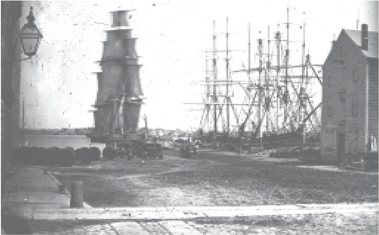
Figure 33: Waterfront, mid-nineteenth century. The granite runners in the foreground facilitated moving large casks of oil from the whaling ships at the docks to local processing plants.
