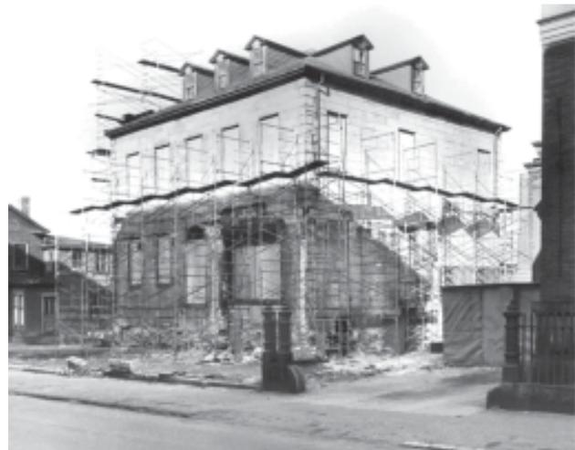
Figure 120: Benjamin Rodman House, North Second Street, ca. 1966. Restoration in progress on the Rodman House, the only one of three remaining waterfront mansions still standing on its original foundation.
