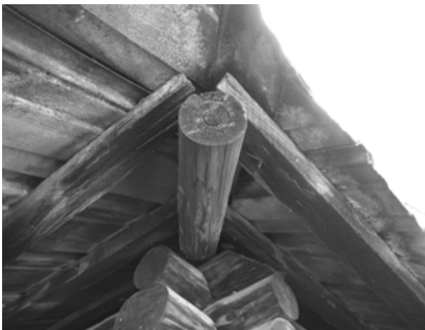
FIGURE 33. View of southwest corner of roof.
