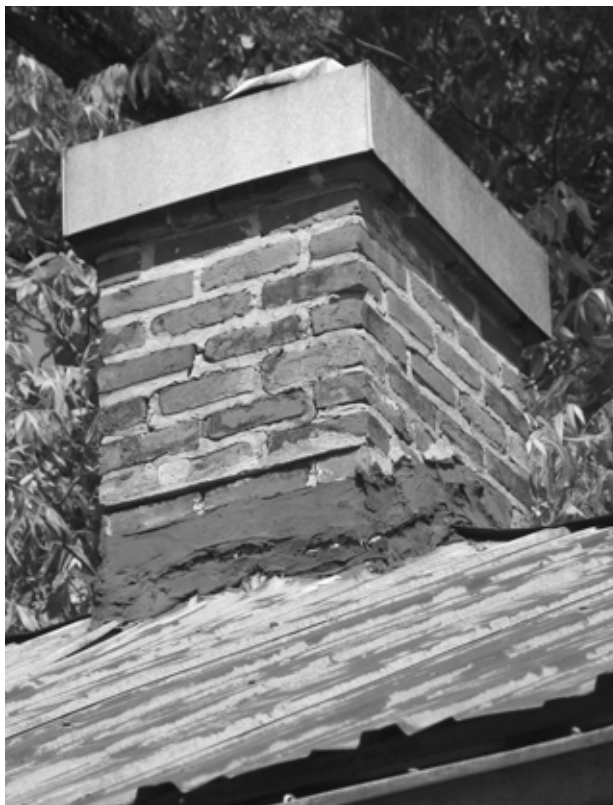
FIGURE 40. View of chimney.
