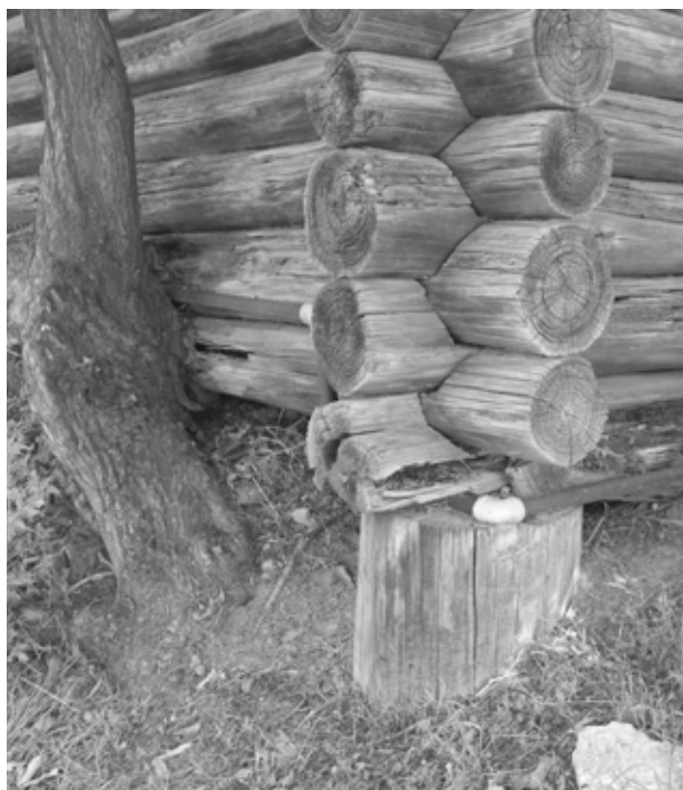
FIGURE 22. View of south corner of building.
