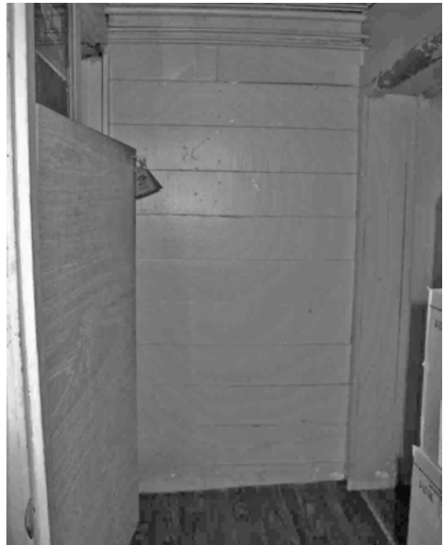
FIGURE 42. View of board walls in hall, typical of original wall finishes in the small pen.
