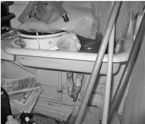
FIGURE 46. View of cast-iron sink in original Kitchen.
