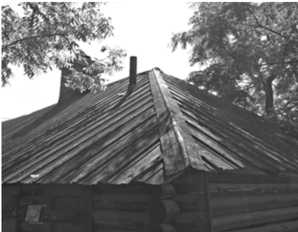
FIGURE 32. View of western hip of roof, showing typical metal roofing.
