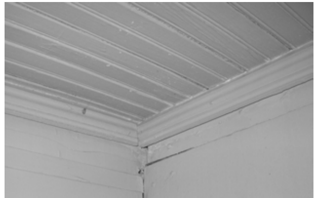
FIGURE 43. View of a corner of the hall showing what was probably the typical ceiling finish in the building's smaller pen.
