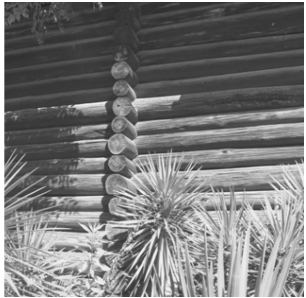
FIGURE 28. View of ends of logs forming the building's crosswall.
