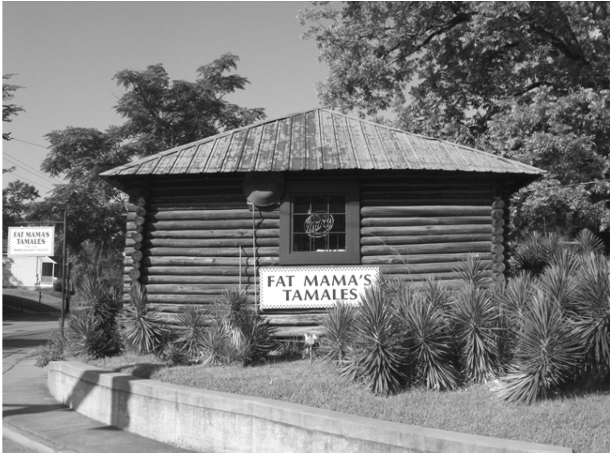
FIGURE 27. View of northeast end of building.
