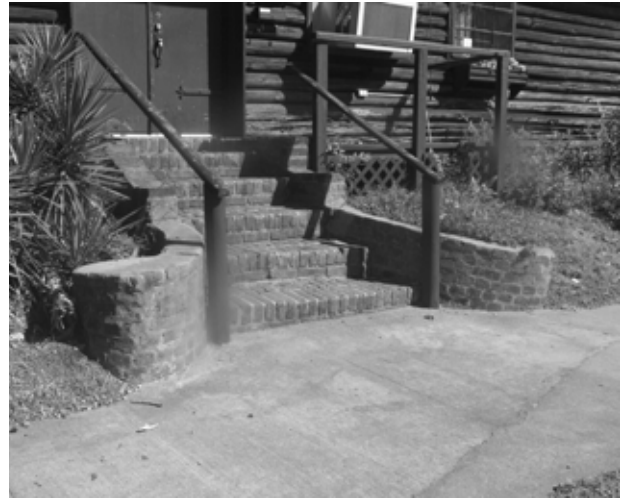
FIGURE 21. View of front steps.
