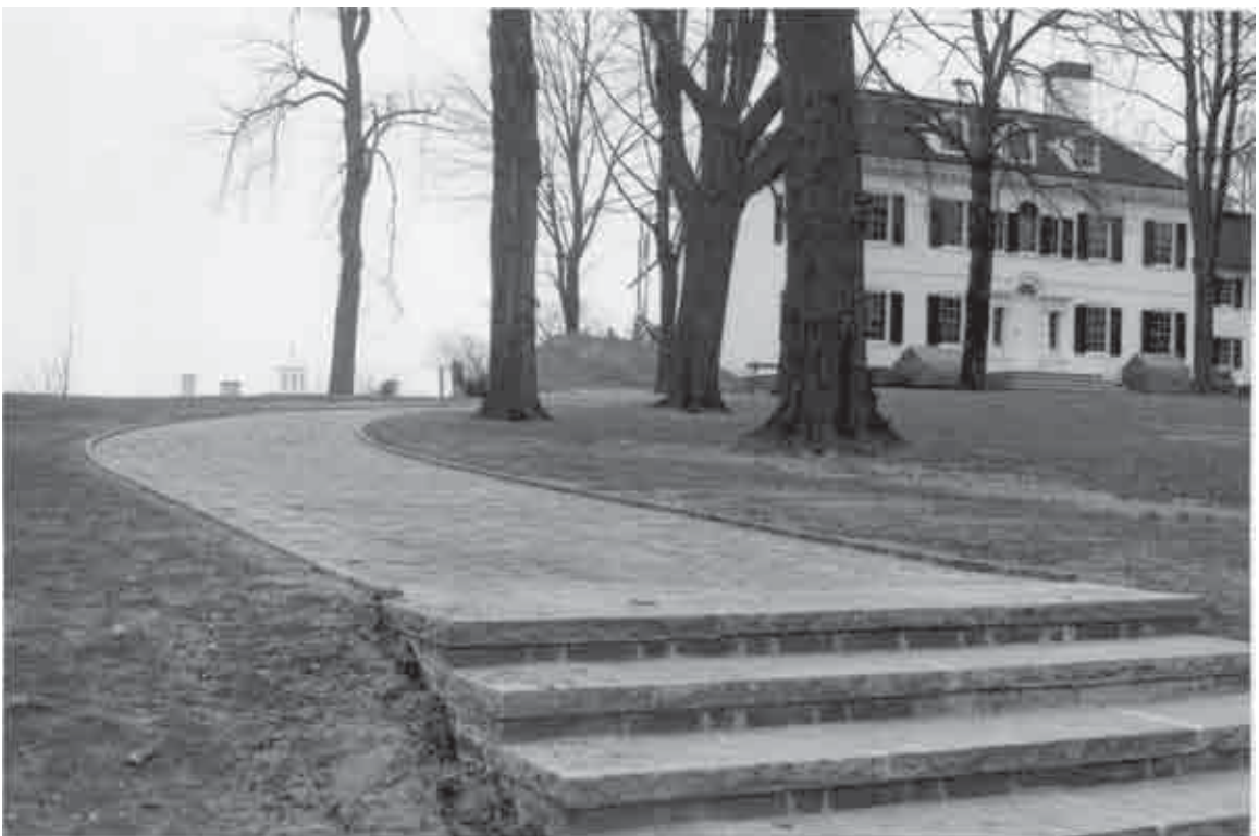
Figure 176. Southwestern end of semicircular front walkway after construction prior to privet shrub planting, 1935 (Morristown NHP CRM Archives).
