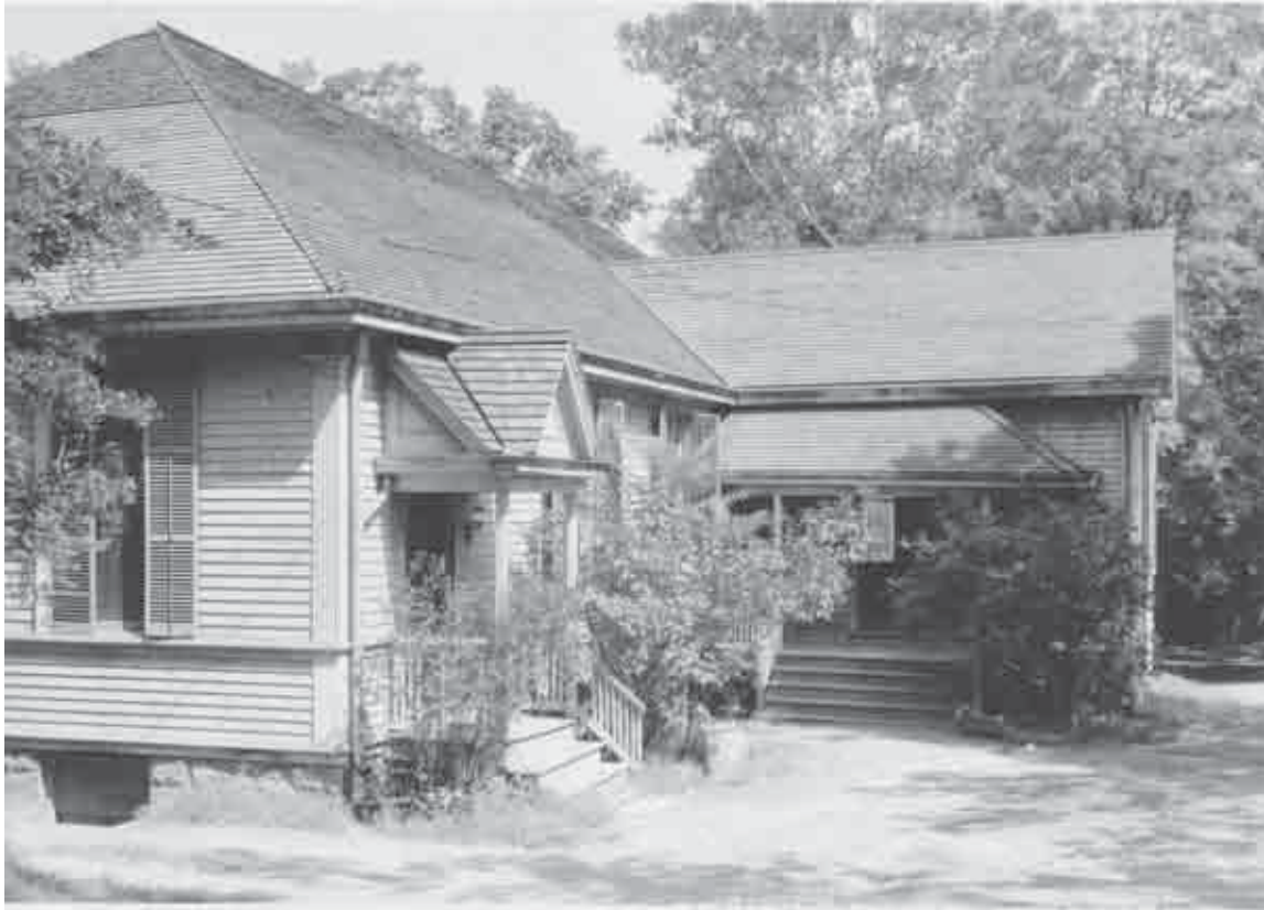
Figure 60. Lafayette Hall prior to demolition, c.1940 (Morristown NHP CRM Archives).
