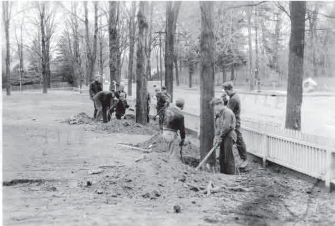
Figure 69. CCC grading the front lawn, 1938 (Morristown NHP CRM Archives).
