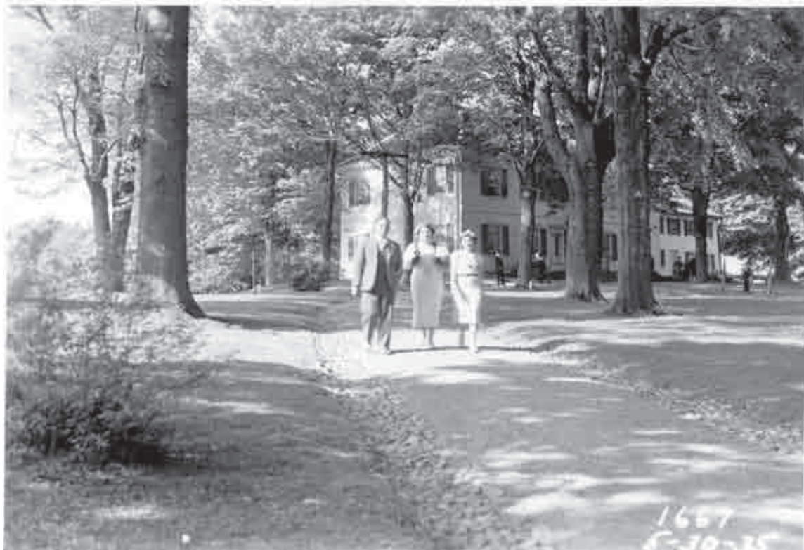
Figure 174. Southwestern portion of semicircular front walkway, 1935 (note gravel surface and cobbled gutters) (Morristown NHP CRM Archives).
