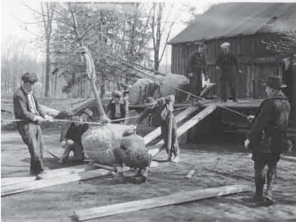
Figure 82. CCC foreman Layton directing the unloading of white oak trees, 1939 (Morristown NHP CRM Archives).
