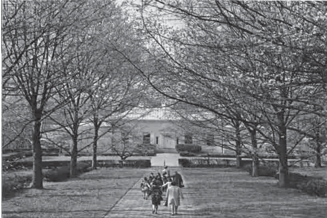
Figure 114. View of allee with brick walkway to museum with a group of touring school children, 1967 (Morristown NHP CRM Archives).
