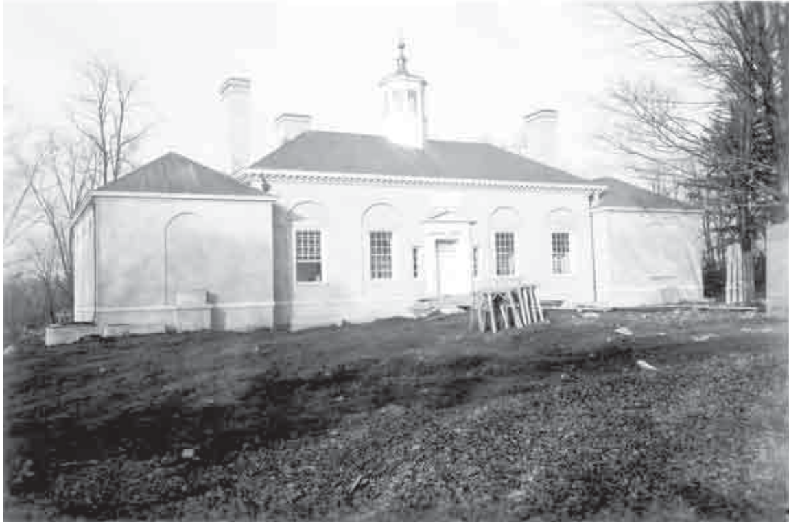
Figure 65. Grading the parterre in front of the new museum, 1937 (Morristown NHP CRM Archives).
