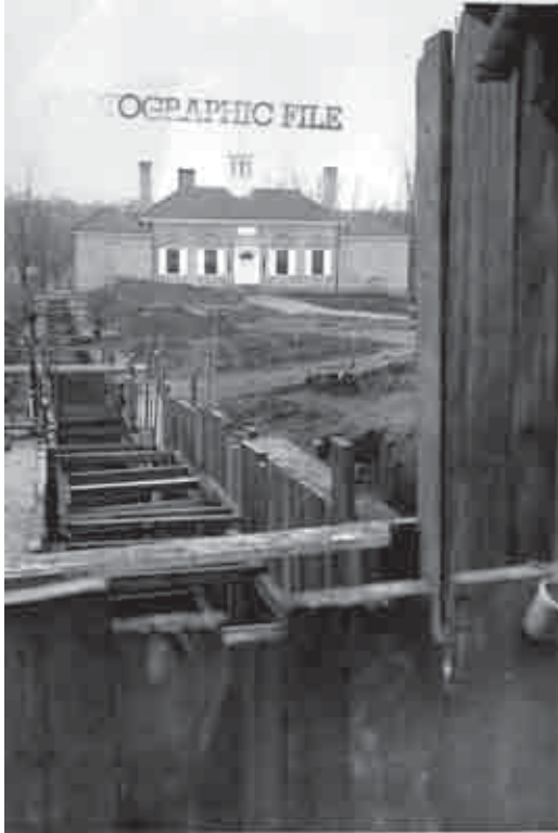
Figure 87. Installation of the steam/utility tunnel by the CCC, 1938 (Morristown NHP CRM Archives).
