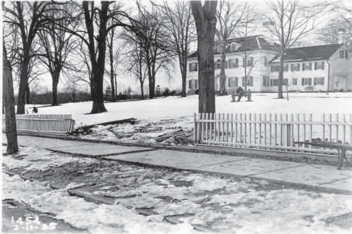
Figure 49. Fence damaged by automobile, 1935 (Morristown NHP CRM Archives).
