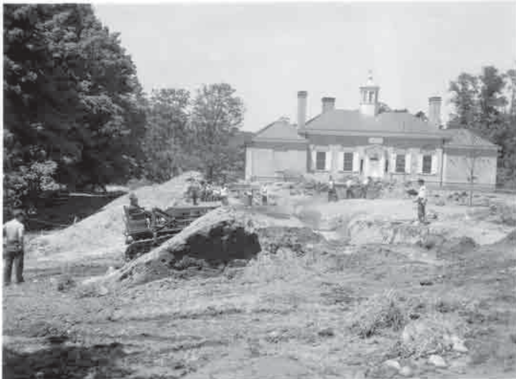
Figure 88. Covering over the completed steam/utility tunnel, 1939 (Morristown NHP CRM Archives).
