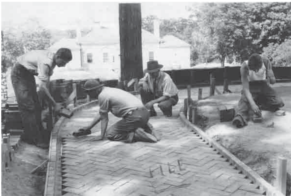
Figure 75. CCC installing the brick rectilinear walkway by the mansion, 1938 (Morristown NHP CRM Archives).
