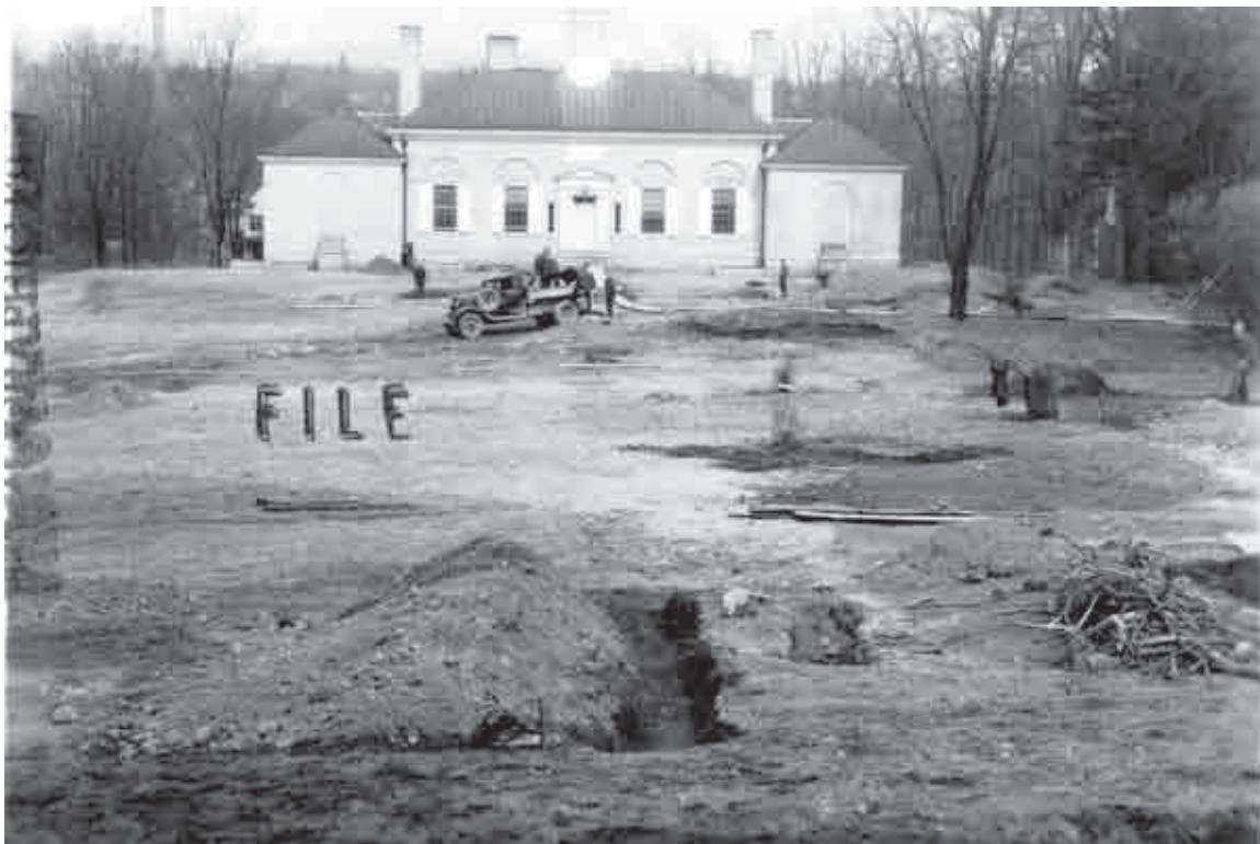
Figure 66. CCC grading the central lawn, 1938 (Morristown NHP CRM Archives).
