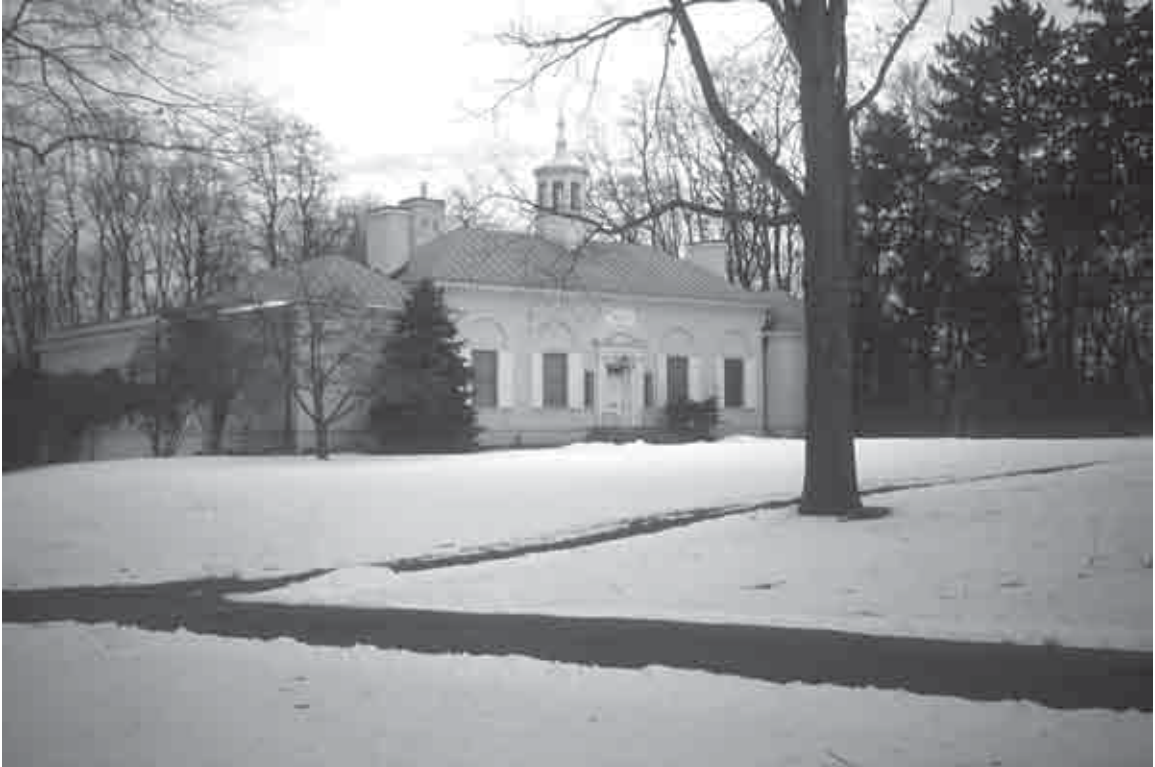
Figure 153. The point where the asphalt circuitous path from the north façade of the museum branches and leads east along the south façade and south to the Ford mansion (OCLP, 2001).
