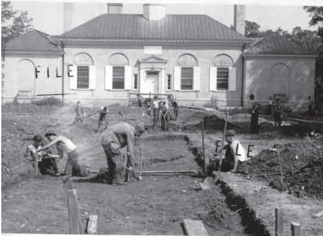
Figure 70. CCC building the brick axial path, 1938 (Morristown NHP CRM Archives).
