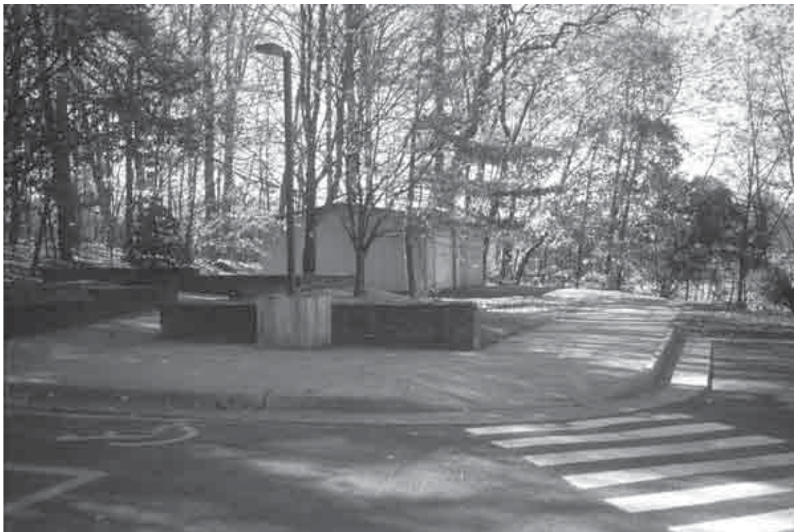
Figure 140. Maintenance shed at southwest corner of visitor parking lot (OCLP, 2001).
