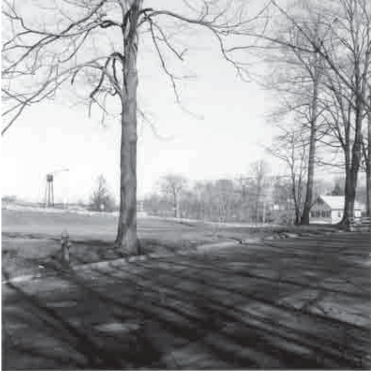
Figure 129. Division Street looking toward Washington Place and new Lafayette Avenue, 1974 (note the street trees from the former homes) (Morristown NHP CRM Archives).
