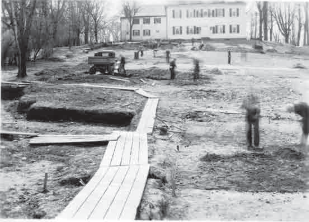
Figure 67. CCC grading the central lawn, 1938 (Morristown NHP CRM Archives).
