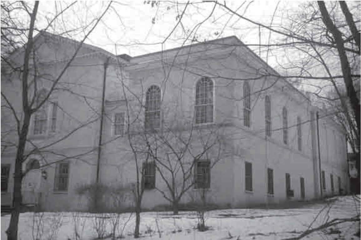
Figure 137. View of the northwest corner of the museum showing the 1957 library addition (OCLP, 2001).
