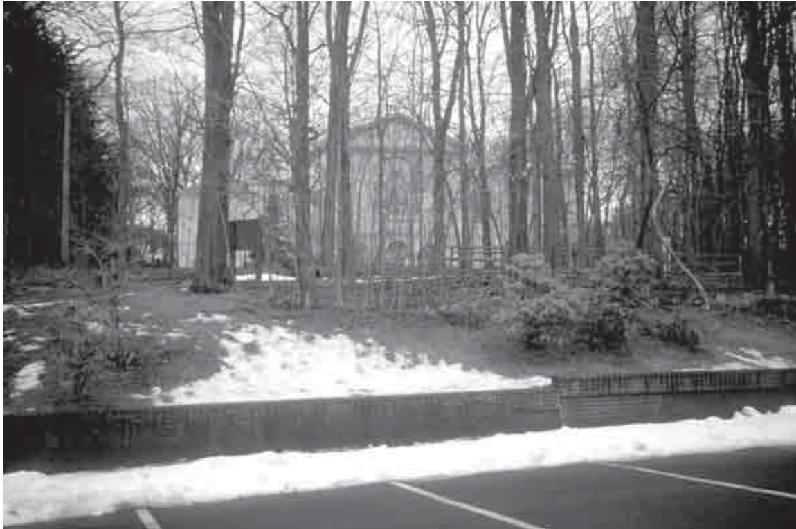
Figure 147. The brick retaining wall along the south side of the visitor's parking lot and the asphalt winding path that leads up the slope to the museum (OCLP, 2001).
