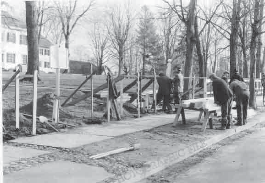
Figure 79. CCC installation of new fence, 1939 (Morristown NHP CRM Archives).
