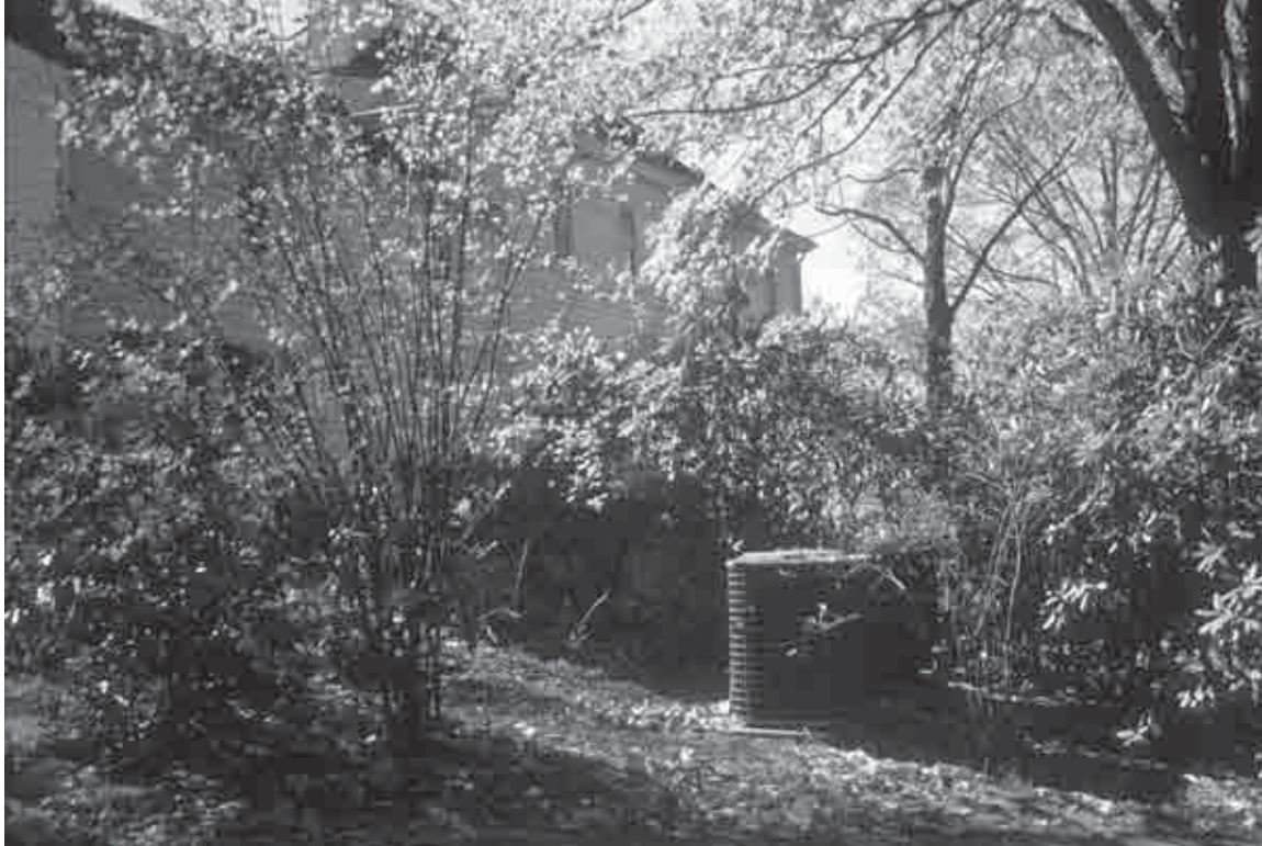
Figure 161. HVAC unit behind northeast corner of Ford mansion screened by shrubs including rhododendron (OCLP, 2001).
