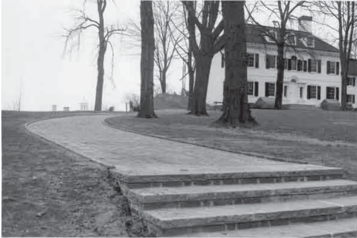
Figure 77. Southwest end of the semicircular walkway just after construction, 1938 (Morristown NHP CRM Archives).
