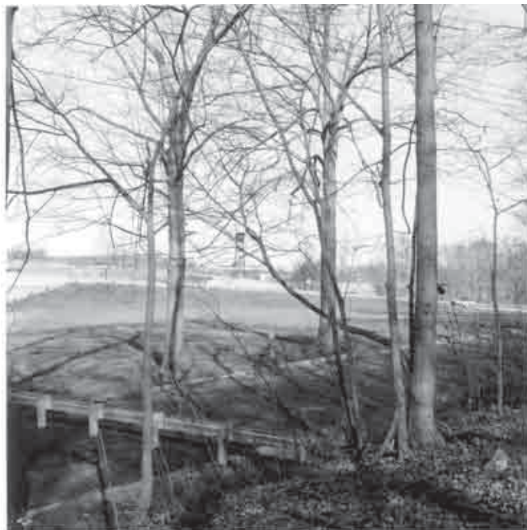
Figure 132. View across parking lot under construction toward new Lafayette Avenue, 1974 (Morristown NHP CRM Archives).
