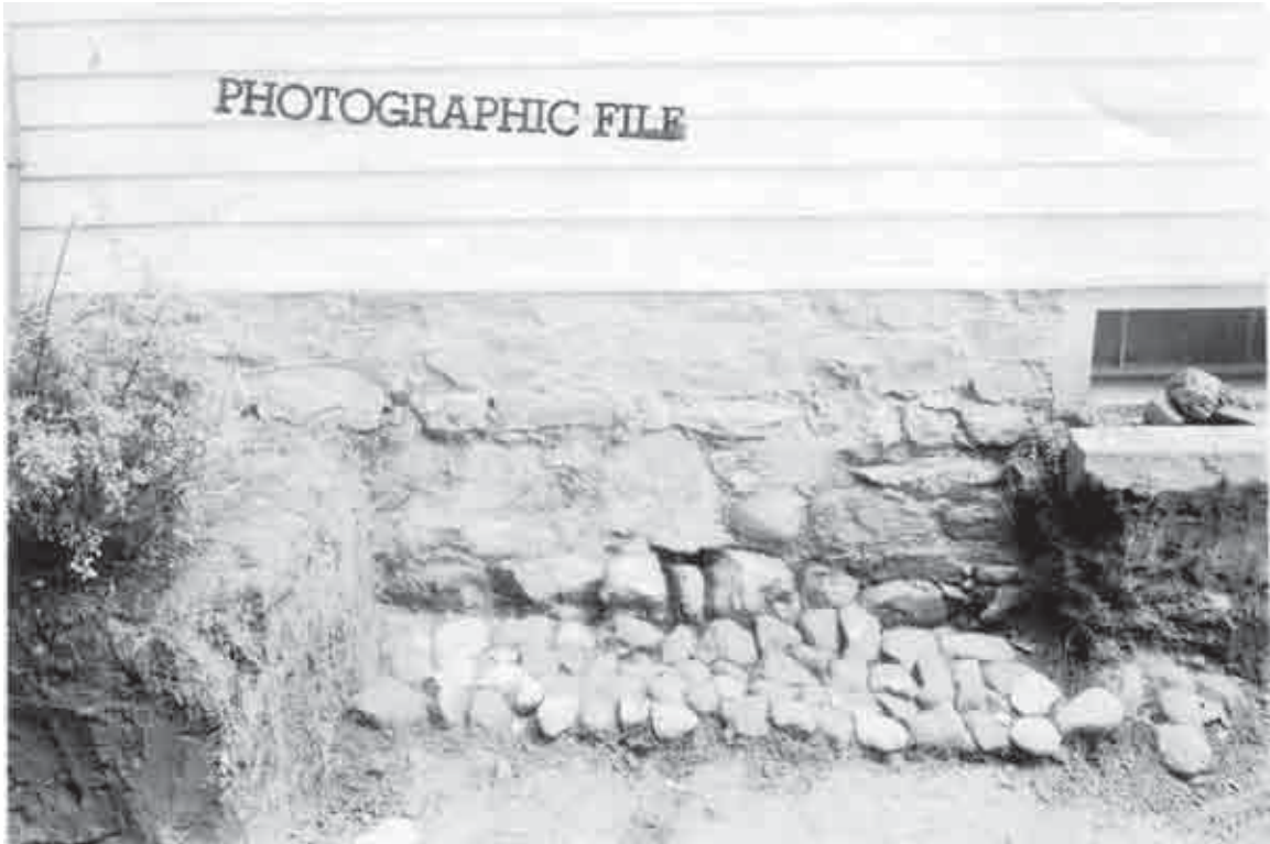
Figure 100. CCC archeology showing that original grade around mansion was two feet lower, 1937 (Morristown NHP CRM Archives).
