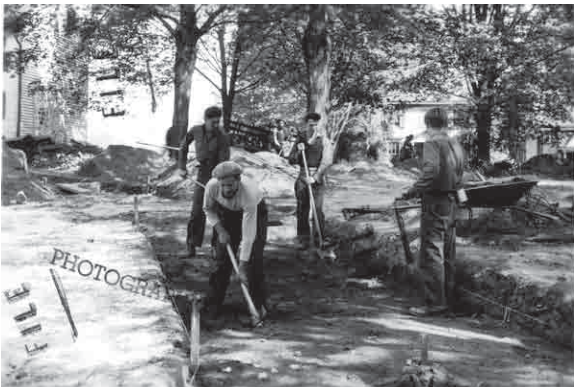
Figure 76. CCC installing the brick rectilinear walkway by the mansion, 1938 (Morristown NHP CRM Archives).
