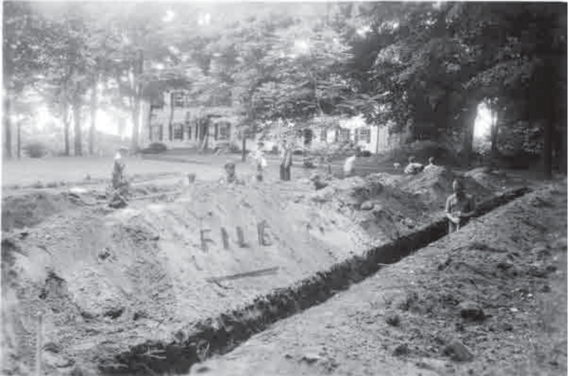
Figure 96. CCC archeological grid trenching of front lawn, 1937 (Morristown NHP CRM Archives).
