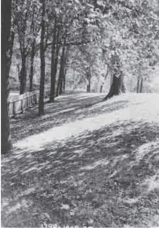
Figure 45. Southeast corner of property along Washington Place, 1935 (Morristown NHP CRM Archives).
