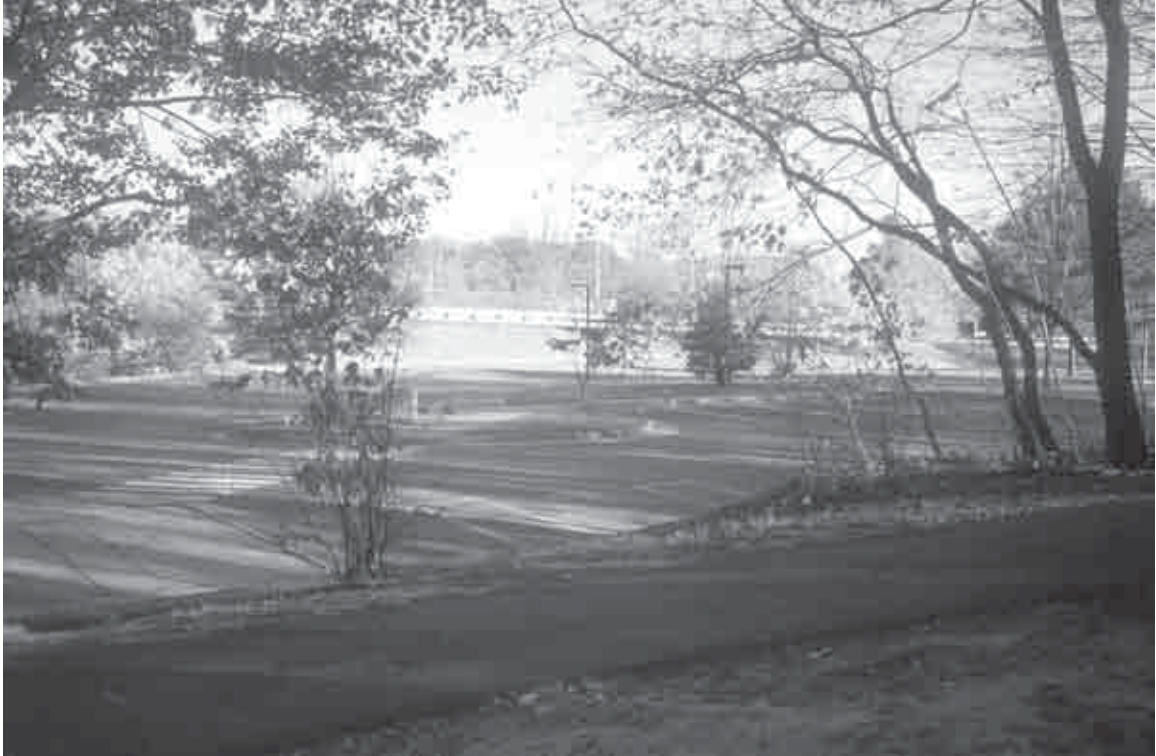
Figure 148. Northern view of the visitor's parking lot from the asphalt winding path (OCLP, 2002).
