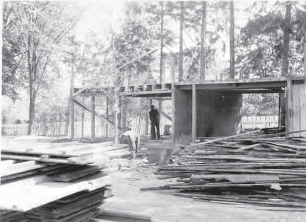
Figure 63. CCC razing the barn, 1939 (Morristown NHP CRM Archives).
