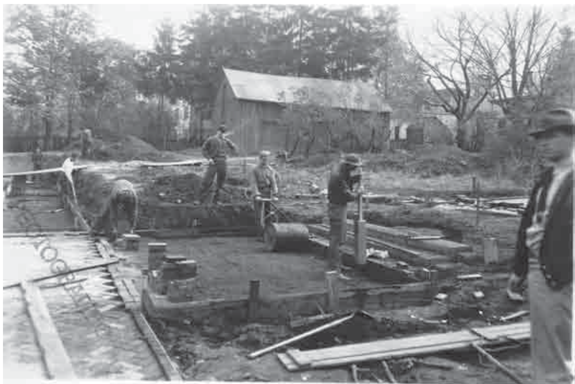
Figure 72. Norman Newton directing the CCC's installation of the parterre's brick rectilinear path, 1938 (Morristown NHP CRM Archives).
