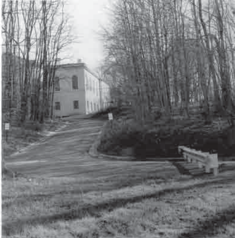
Figure 130. Division Street and entrance drive intersection truncated for I-287 construction, 1974 (Morristown NHP CRM Archives).
