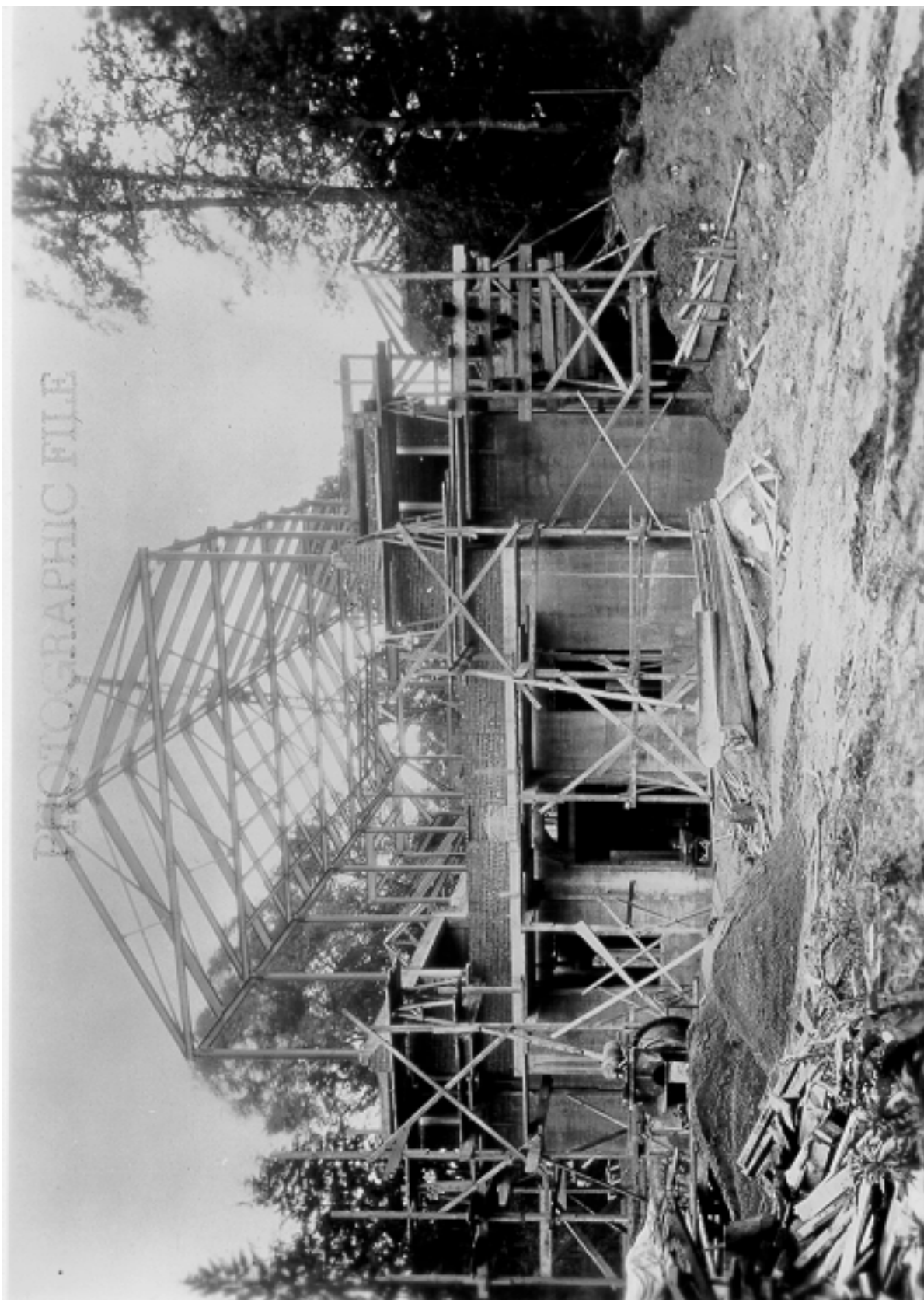
Figure 11. Morristown Museum Building: north elevation, poured- concrete foundation and steel framing (June 1936).
