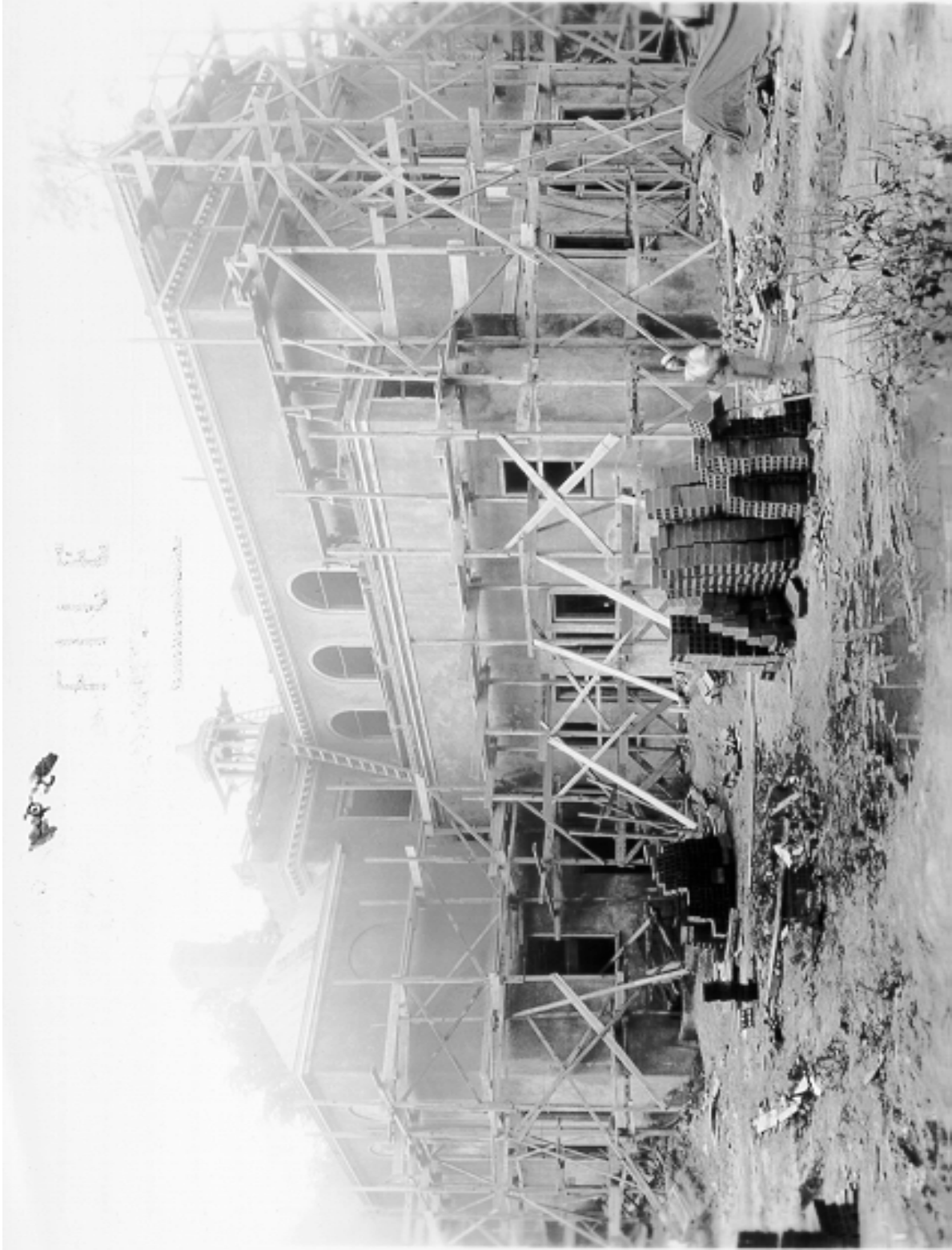
Figure 13. Morristown Museum Building: east and north elevations, stucco application. Note stacks of terra- cotta blocks (1936).
