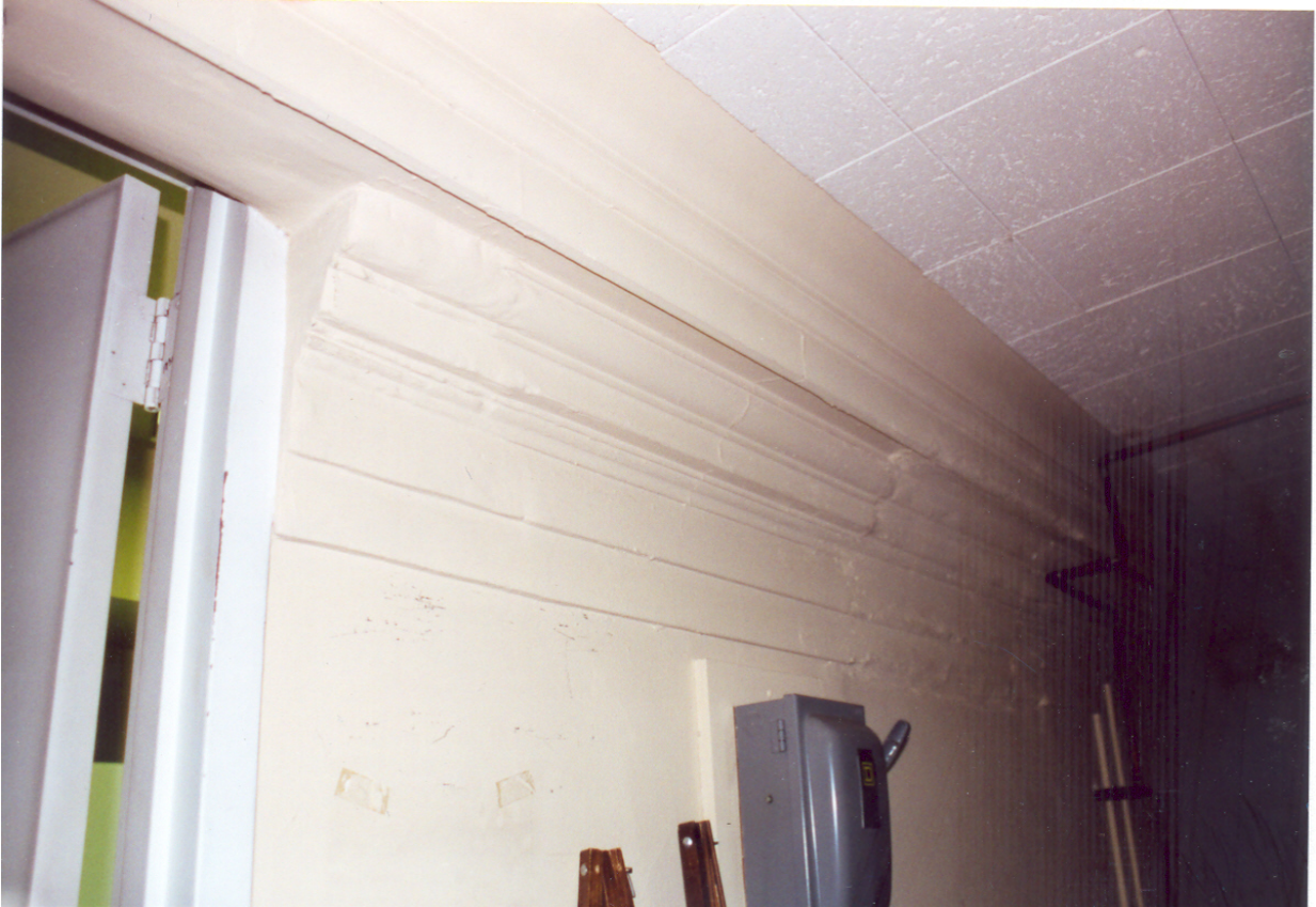
Figure 157. Room 203 – second- story mechanical room: south wall, 1937 auditorium plaster cornice with 1975 patching (2001).
