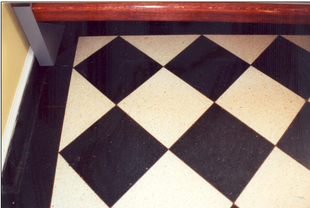
Figure 115. Room 101 – vestibule: terrazzo tile flooring (2001).
