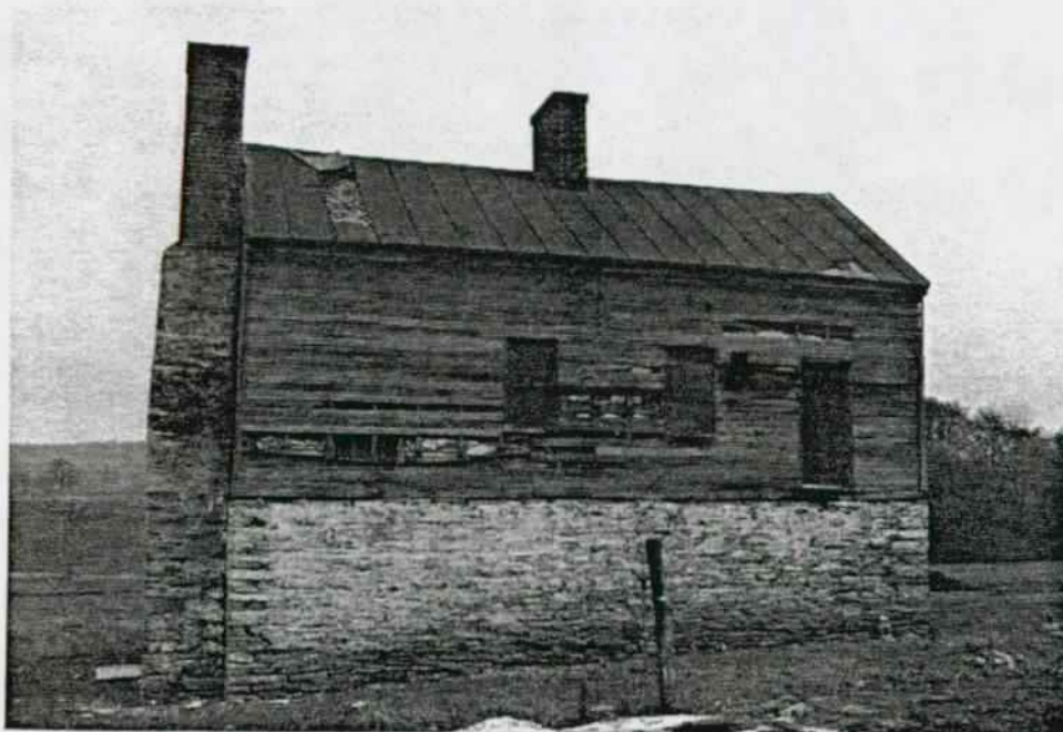
The Hermitage. Secondary dwelling, west elevation stone section, ca. 1760s-1770s, log addition ca. 1790s. Note door on left in log section, closed in. P. Reed 4/98.
