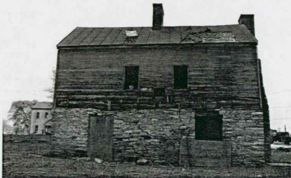
The Hermitage. Secondary dwelling, east elevation, ca. 1760s-1770s, with 1790s log top story. P. Reed 4/98.
