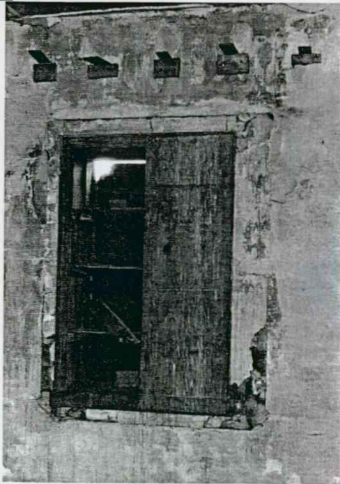
The Hermitage. Secondary dwelling. South room, second floor, window. Note change of size. P. Reed 4/98.
