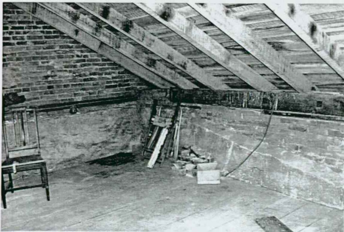
The Hermitage. Attic, 1820s addition. Note parged wall remnants from former shed-roofed extension. P. Reed 2/99.
