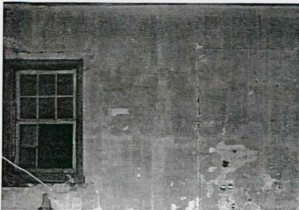
The Hermitage. Secondary dwelling. Second floor, north room, west wall, window. Note outline of door, filled-in, change in size of window, and marks in plaster indicating a peg rail between window and door. P. Reed 4/98.
