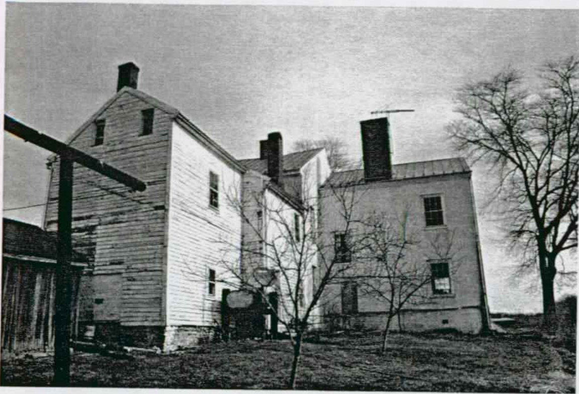
Hermitage (Best Farm). Rear elevation showing five components of the house. From left, one story sided log room with frame second story; two story frame section; two story 1820s stuccoed brick section; and two story stuccoed brick 1790s section with watertable. P. Reed 2/99.
