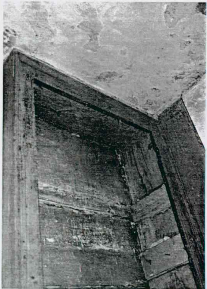
The Hermitage. Secondary dwelling. South room, second floor, cupboard. Note 1790s ovalo trim. P. Reed 4/98.
