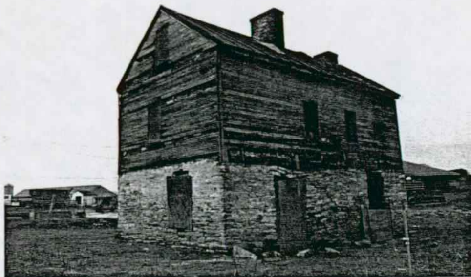
The Hermitage. Secondary dwelling, northwest view, ca 1760s-1770s with 1790s log top story. P. Reed 4/98.
