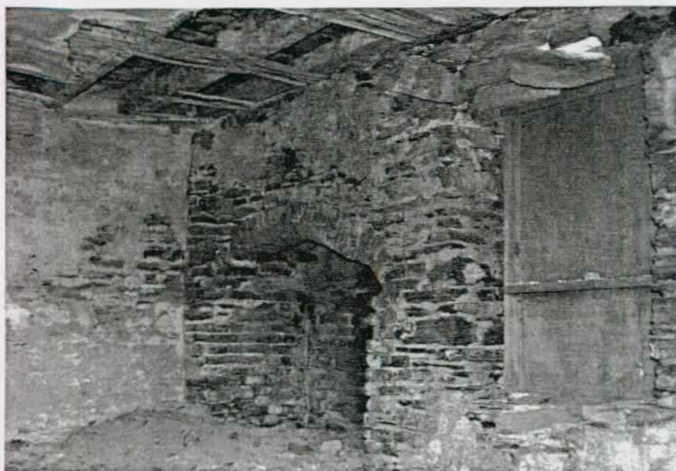
The Hermitage. Secondary dwelling. North room ground level, ca. 1760s-1770s. Note arched fireplace opening. P. Reed 4/98.
