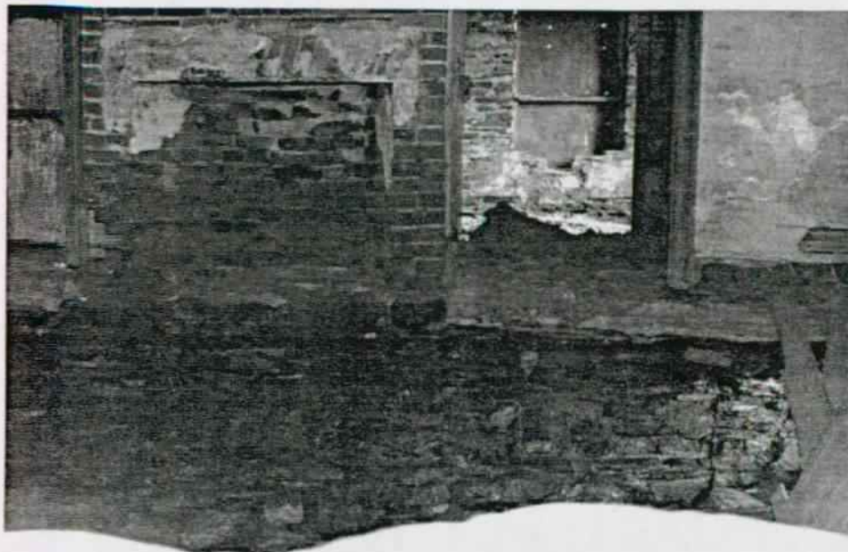
The Hermitage. Secondary dwelling. South room, ground level. Note added fireplace, ca. 1790s. P. Reed 4/98.
