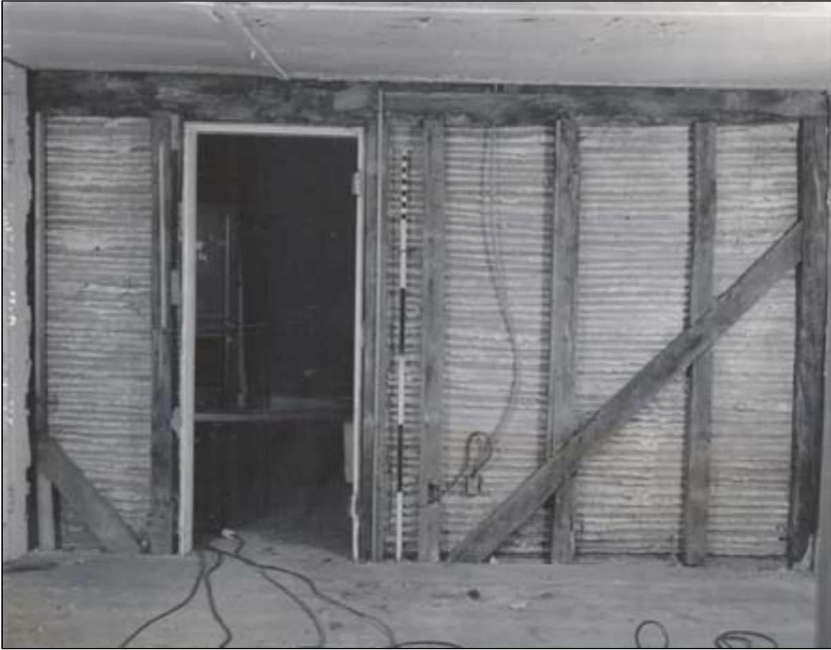
Figure 42. Main House: West gable end, after removal of ca.- 1956 clapboards during architectural investigation; window opening is not original.
