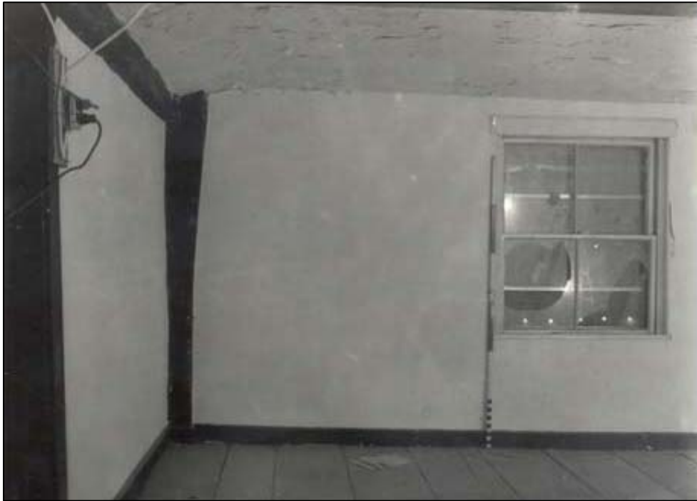
Figure 62. Main House: East Chamber, northeast corner, showing plaster cove ceiling.
