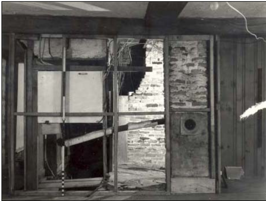
Figure 56. Main House: East Parlor, west wall after removal of ca.- 1956 paneling, showing space originally occupied by central chimney.
