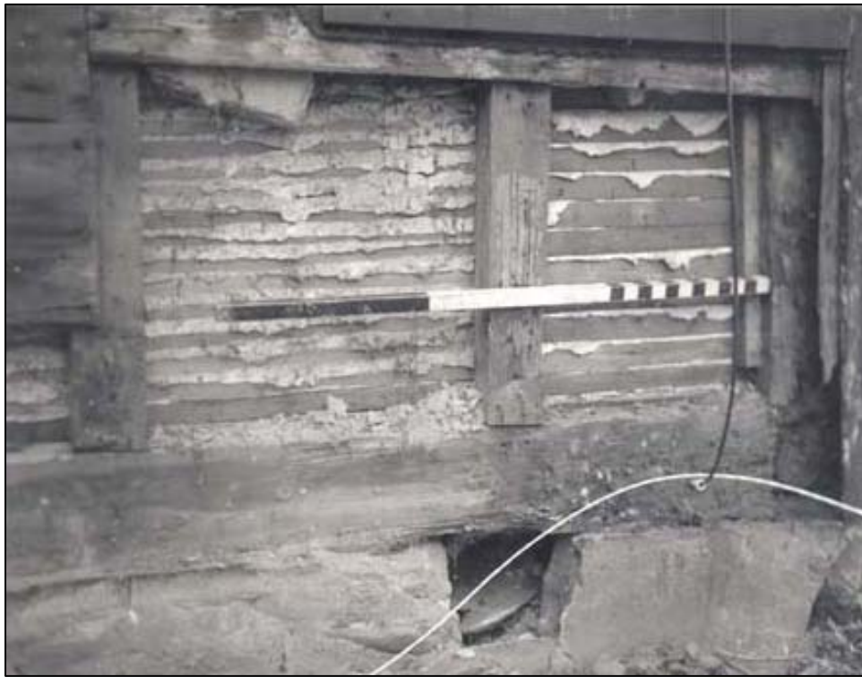
Figure 78. Main House: West wall, south corner, showing west sill replaced ca. 1825.
