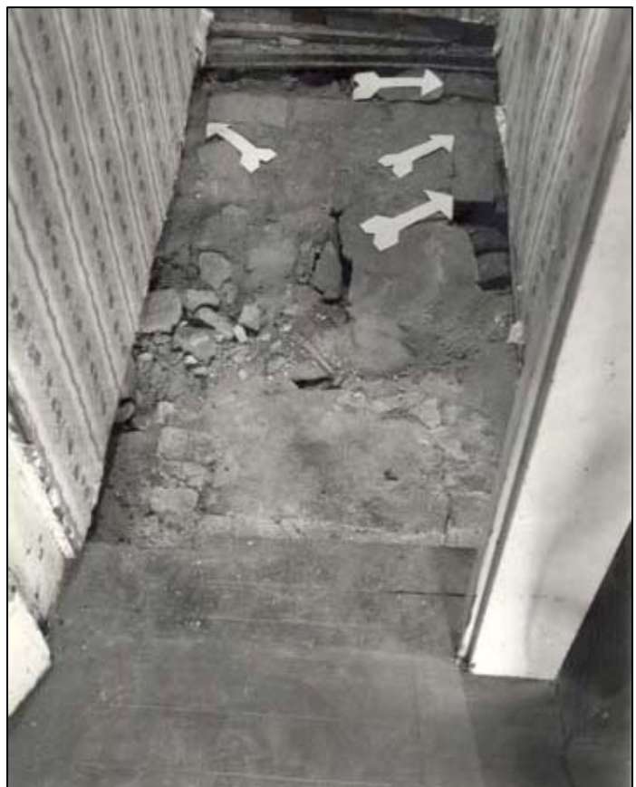
Figure 58. Main House: East Parlor, remains of north jamb of ca.- 1692 fireplace (left arrows), and of east side of ca.- 1750 fireplace in lean- to (right arrows).
