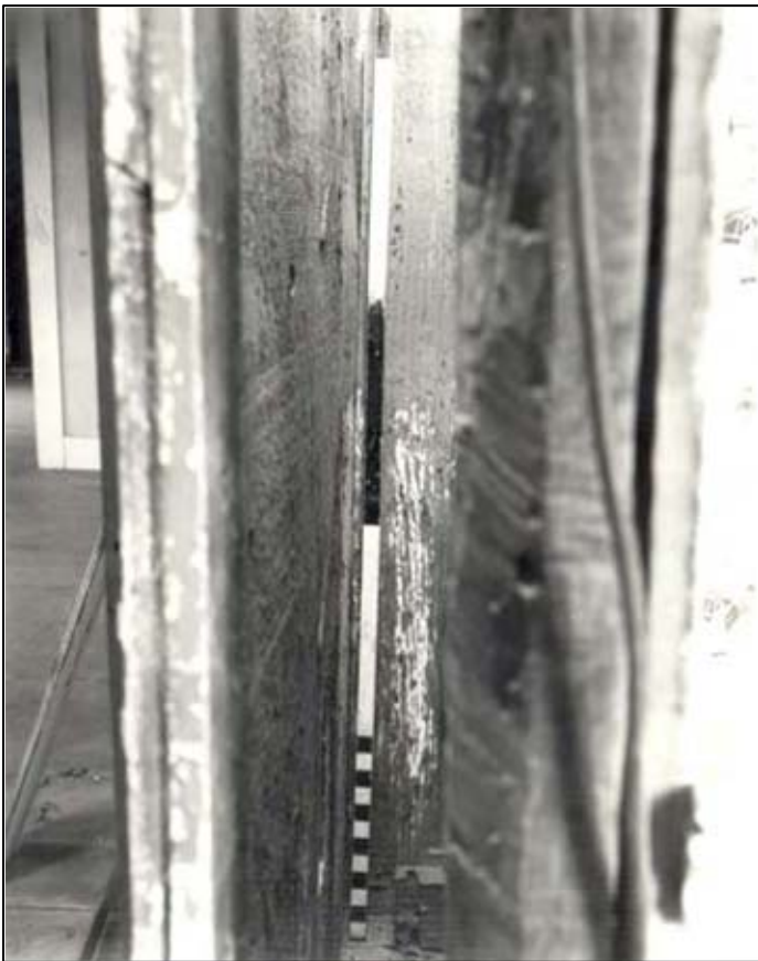
Figure 71. Main House: Front Hall, looking northwest into West Chamber, showing cut- out for first step of original attic stairway (removed ca. 1750).
