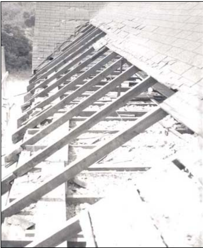
Figure 91. Ca.- 1900 Addition: East roof slope, after removal of reused ca.- 1692 wall boards.
