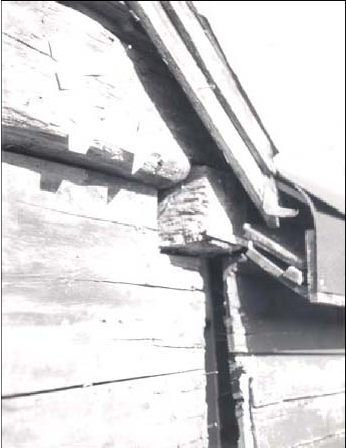
Figure 35. Main House: North corner of east gable end, showing end of north wall plate overridden by east overhanging girt; arrows point to pin connections of rafter and posts tenons.
