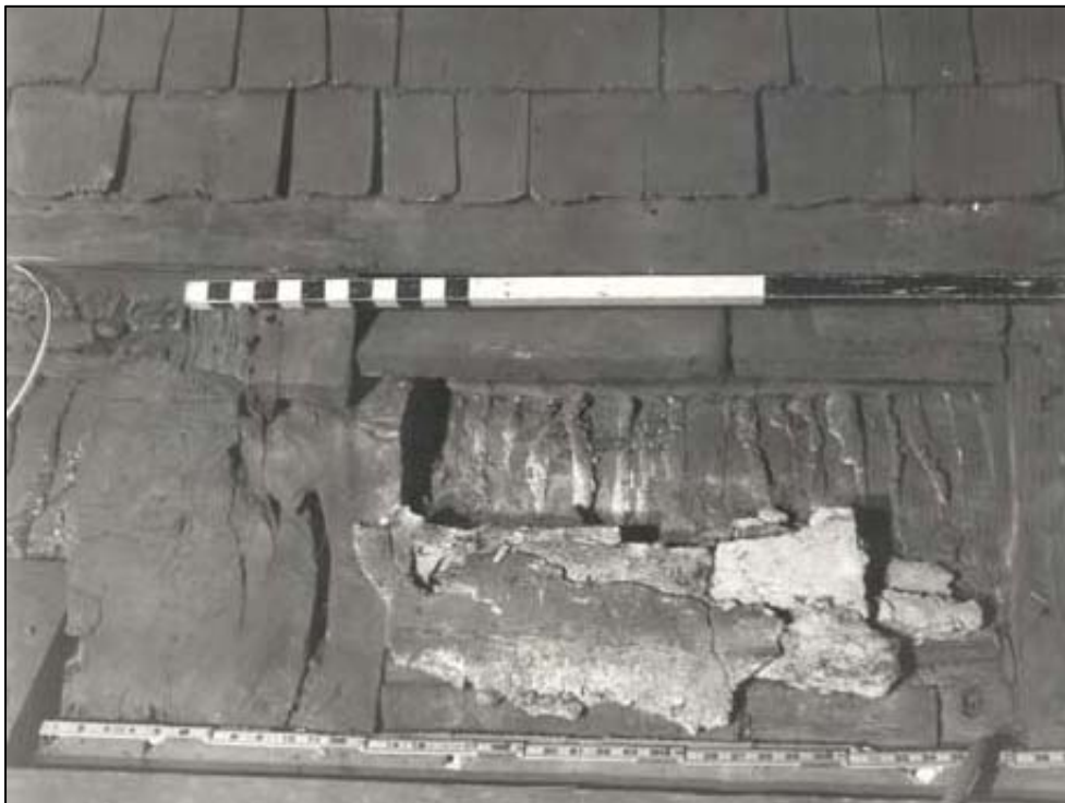
Figure 63. Ca.- 1900 Addition: Attic, looking south at backside of lath- and-plaster cove ceiling along north wall of West Chamber.
