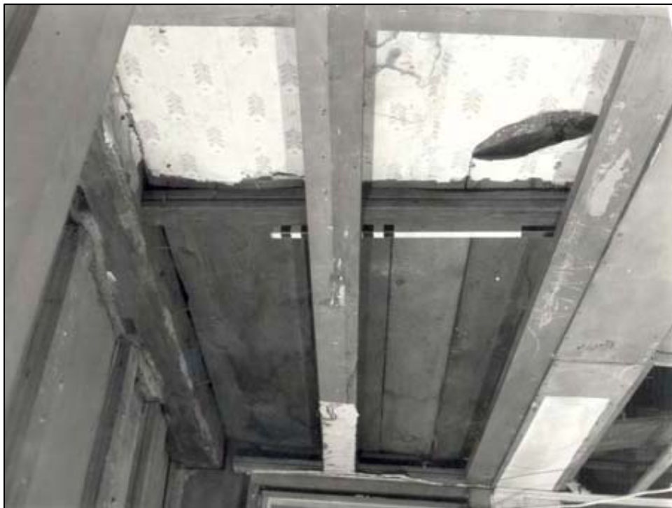
Figure 70. Main House: View of central chimney area, second story, looking east after removal of plasterboard walls and ceiling; scale stick rests on reused piece of ca.- 1692 handrail.
