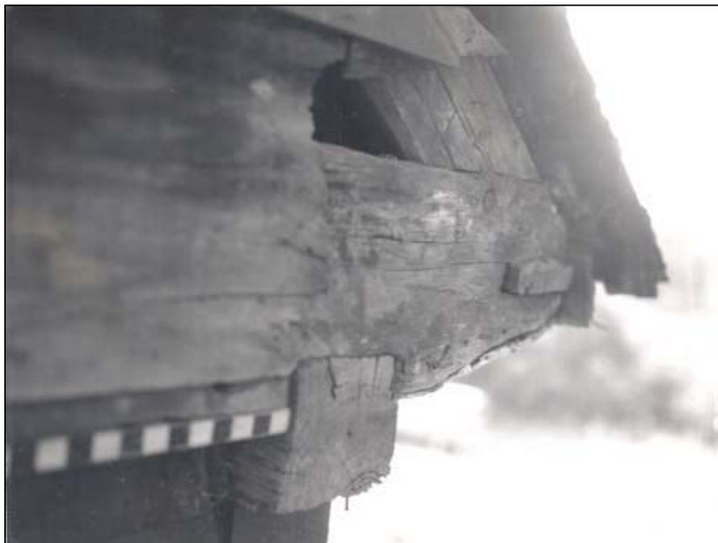
Figure 34. Main House: South corner of west gable end, showing overhanging plate and girt.
