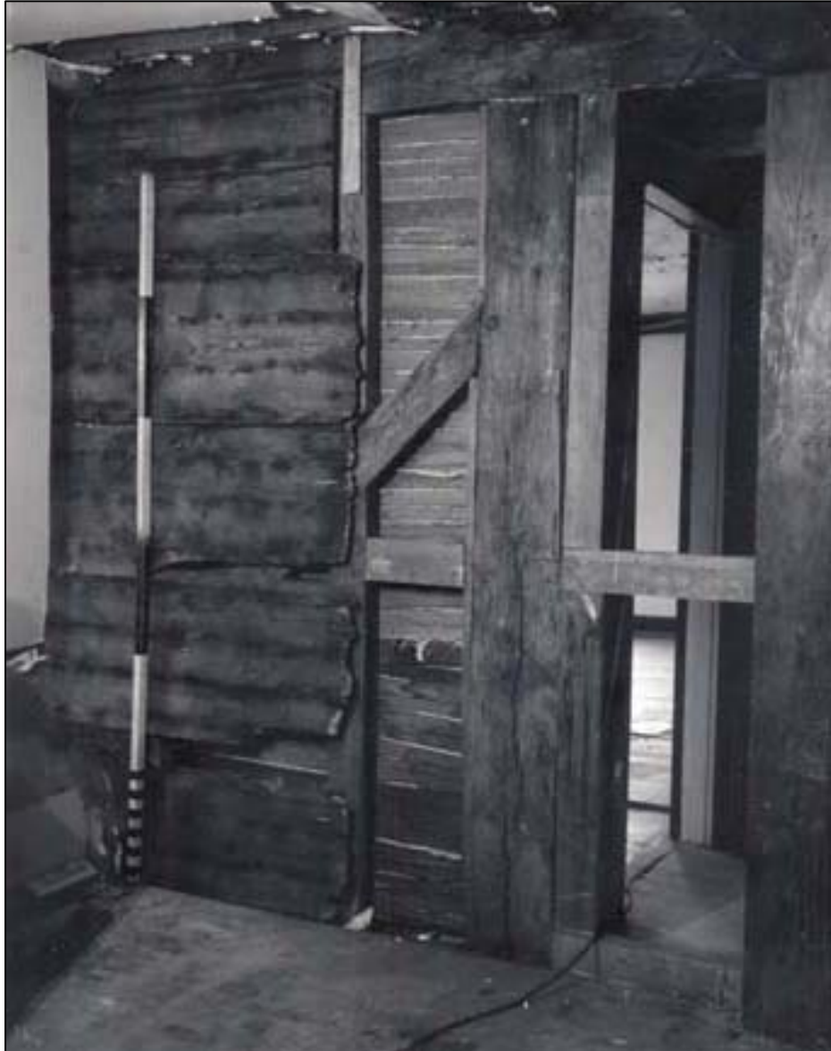
Figure 45. Ca.- 1900 Addition: Second- story center room, looking south at north (formerly exterior) wall of main house, showing original wall boards with lapped ends, removed ca. 1900 and replaced in 1980.
