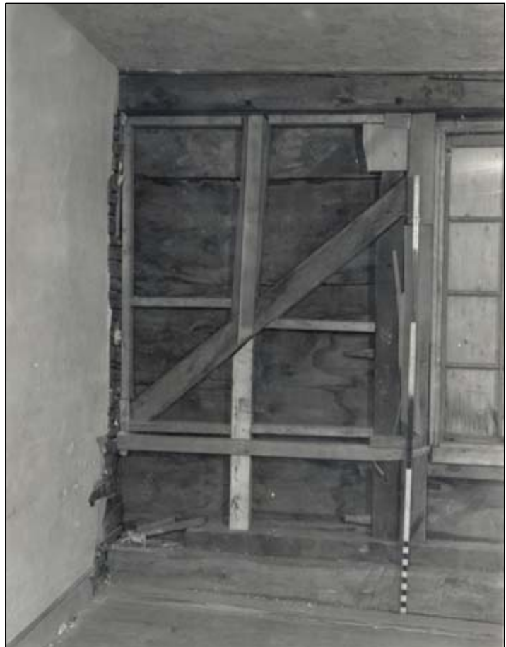
Figure 38. Ca.- 1900 Addition: Looking east from first- story center room along north (formerly exterior) wall of main house (at right), after wall covering was removed.
