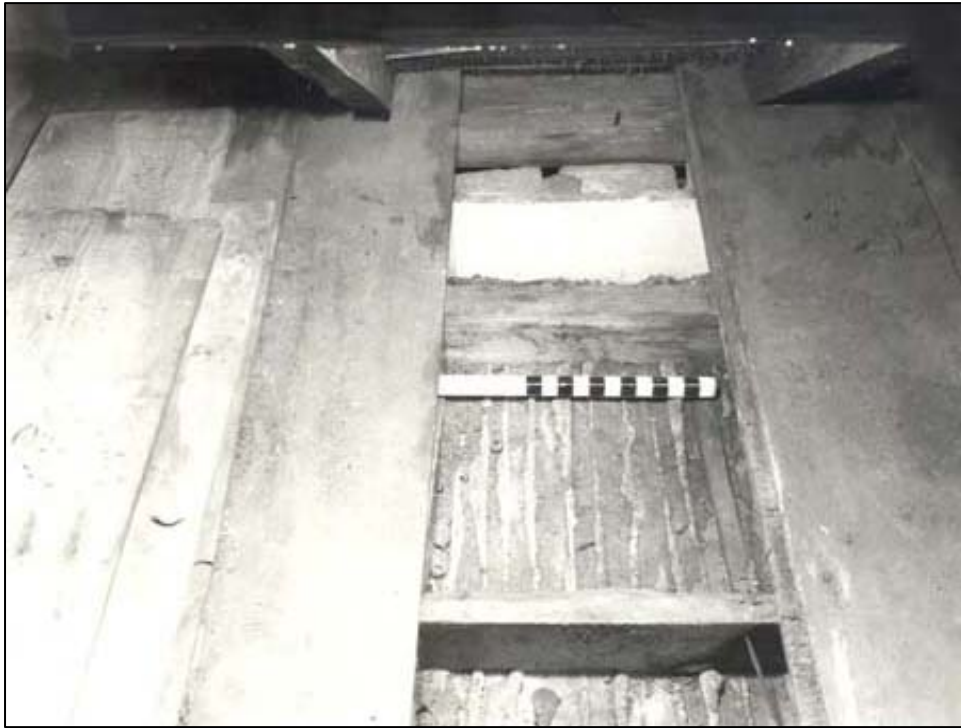
Figure 69. Main House: Attic, plaster over bricks between south plate and floorboards above West Chamber.
