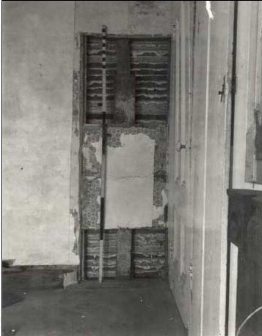
Figure 55. Main House: West Parlor, north wall, former doorway to ca.-1730 lean- to.
