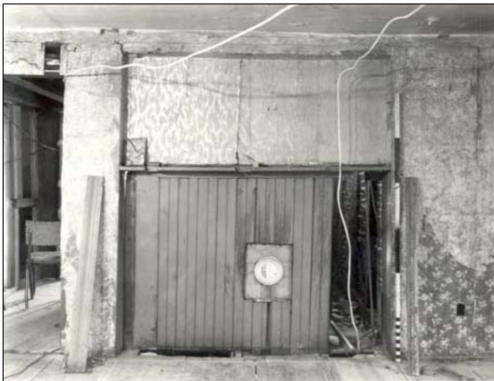
Figure 81. Main House: West Chamber, east wall, showing ca.- 1825 mantel elements and ca.- 1910 wainscot infill and flue thimble.
