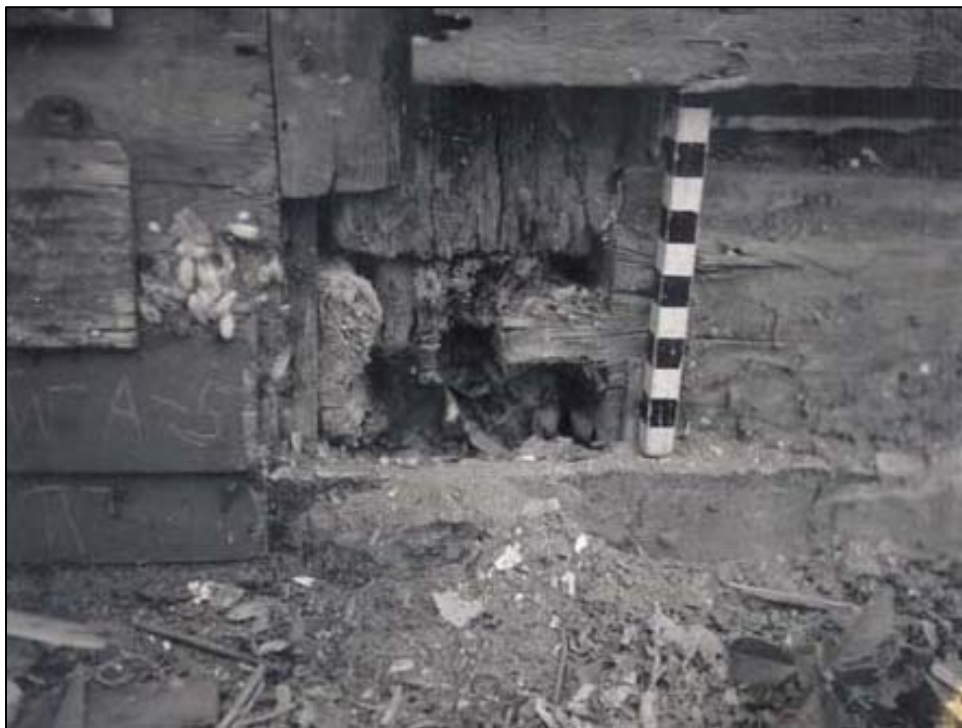
Figure 79. Main House: West wall, north corner, showing west sill tenoned into north sill.
