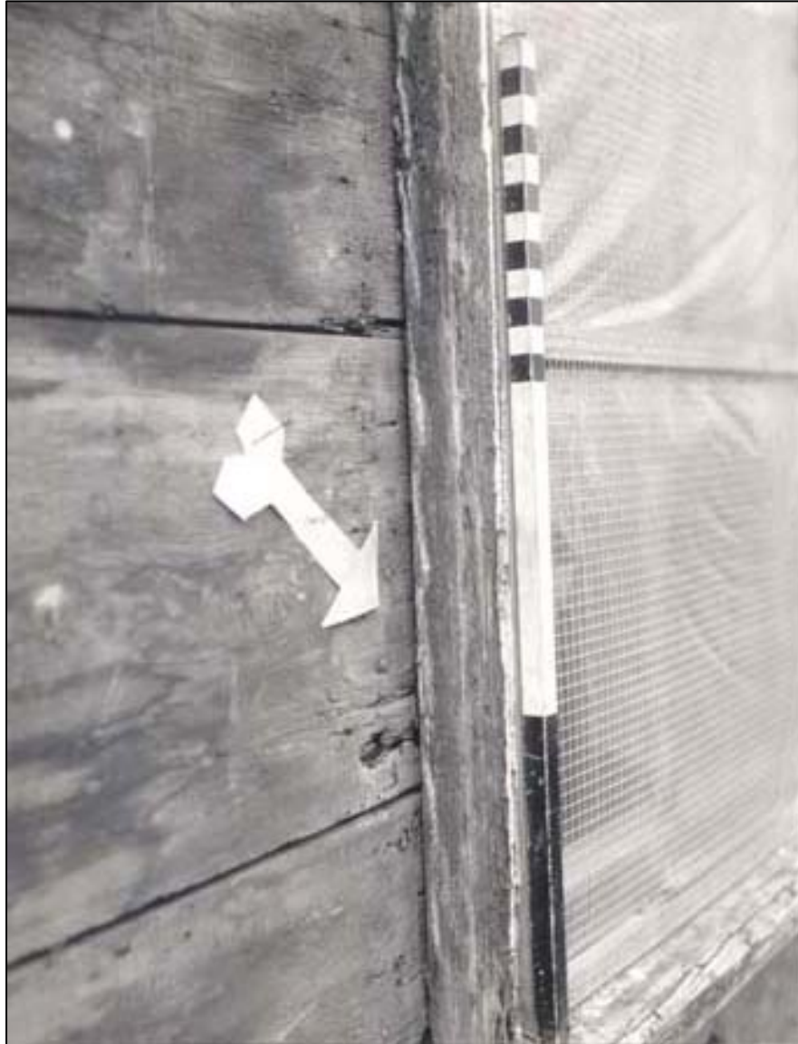
Figure 50. Main House: East exterior wall, showing East Chamber window; arrow points to outline of ca.- 1692 window sill, jamb.
