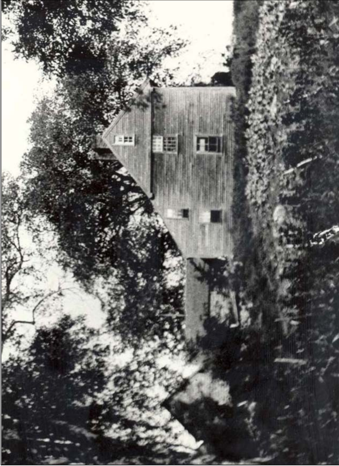
Figure 7. Captain William Smith House: View of west elevation, showing shed ell of ca. 1825 attached to kitchen lean-to. Photographer unknown; date of photograph 1895- 1897.
