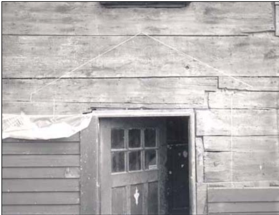
Figure 73. Main House: South exterior wall, outline of ca.- 1750 entrance pediment.
