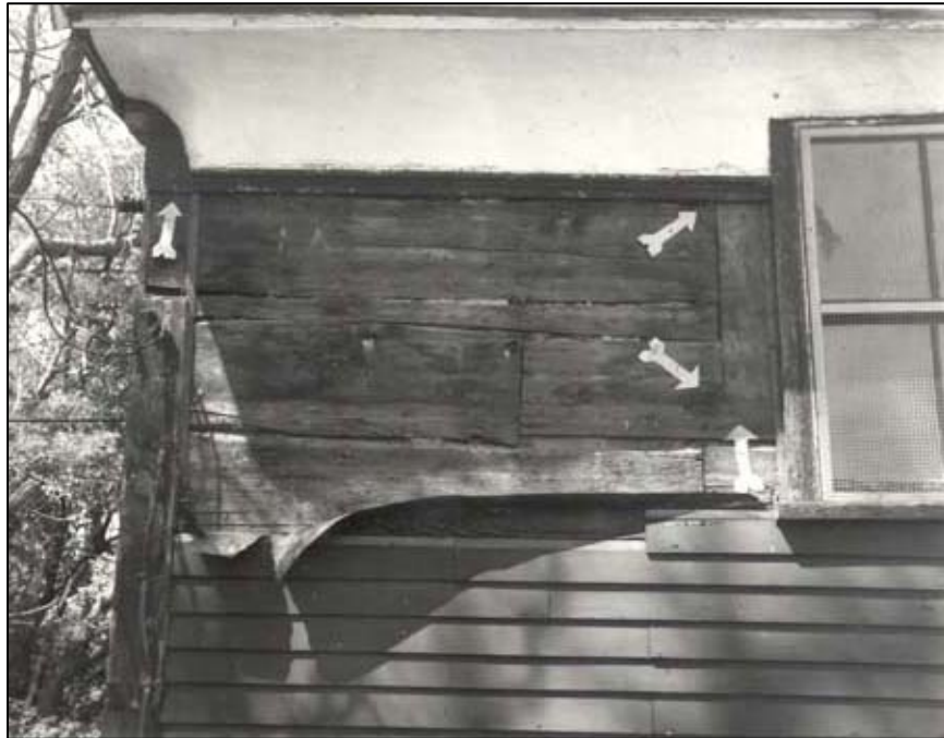
Figure 51. Main House: South exterior wall, west end, showing cove cornice and West Chamber window; left arrow points to former location of original bed molding; right arrows point to head, jamb, sill locations of ca.- 1692 window opening.
