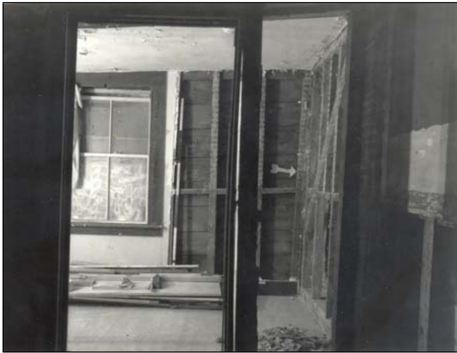
Figure 38. Ca.- 1900 Addition: Looking east from first- story center room along north (formerly exterior) wall of main house (at right), after wall covering was removed.
