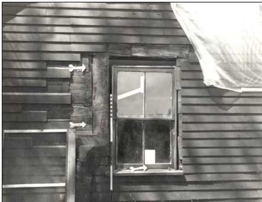
Figure 52. Main House: South exterior wall, showing West Parlor window; arrows point to head, sill locations of ca.- 1692 window opening.
