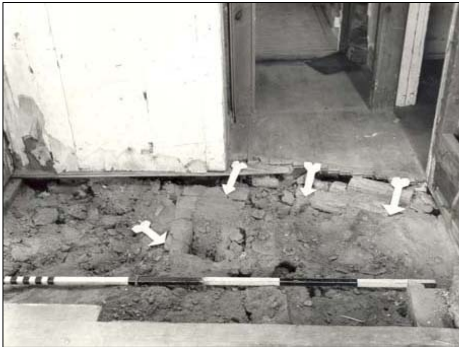
Figure 58. Main House: East Parlor, remains of north jamb of ca.- 1692 fireplace (left arrows), and of east side of ca.- 1750 fireplace in lean- to (right arrows).
