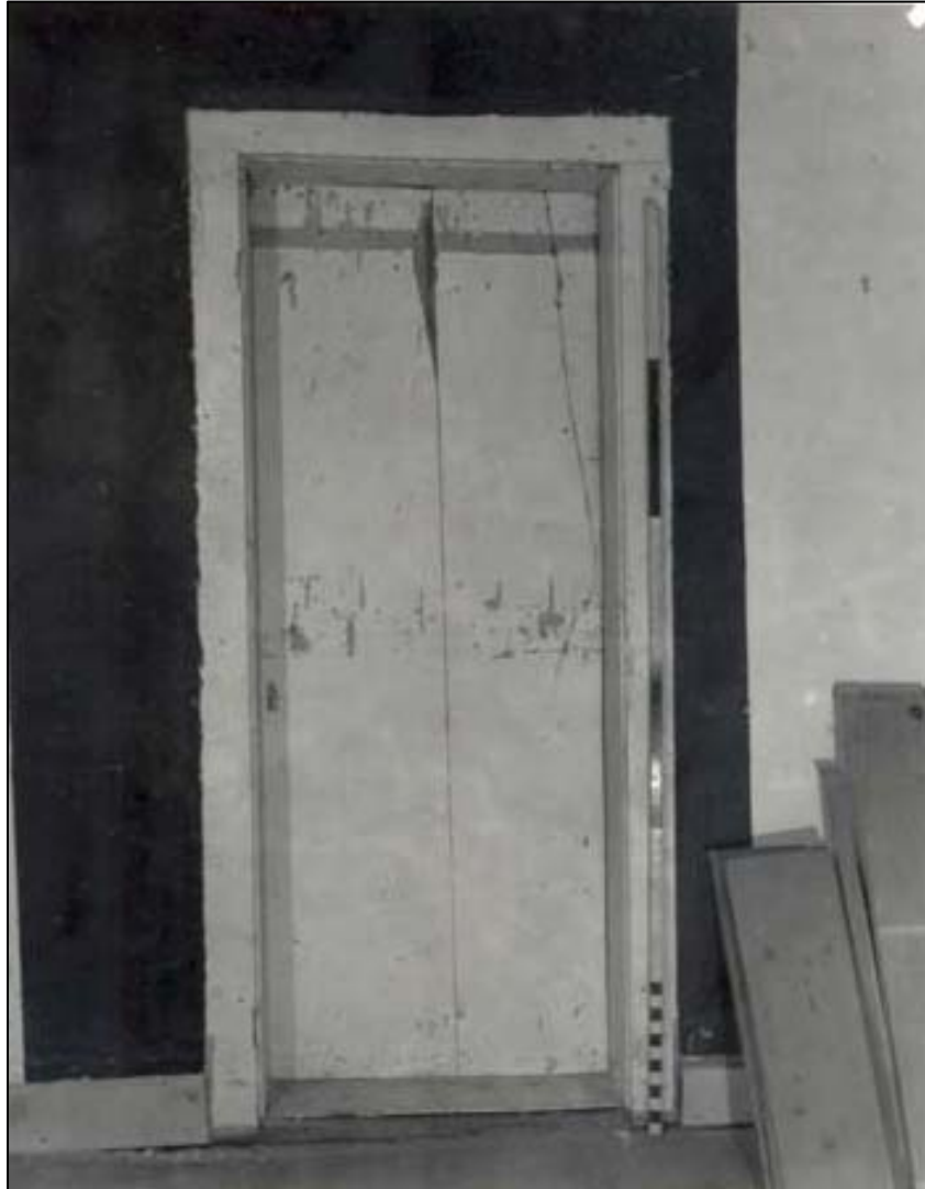
Figure 77. Main House: East Parlor, north wall, ca.- 1810 doorway to ca.- 1730 lean- to (after removal of ca.- 1956 paneling and shelves).
