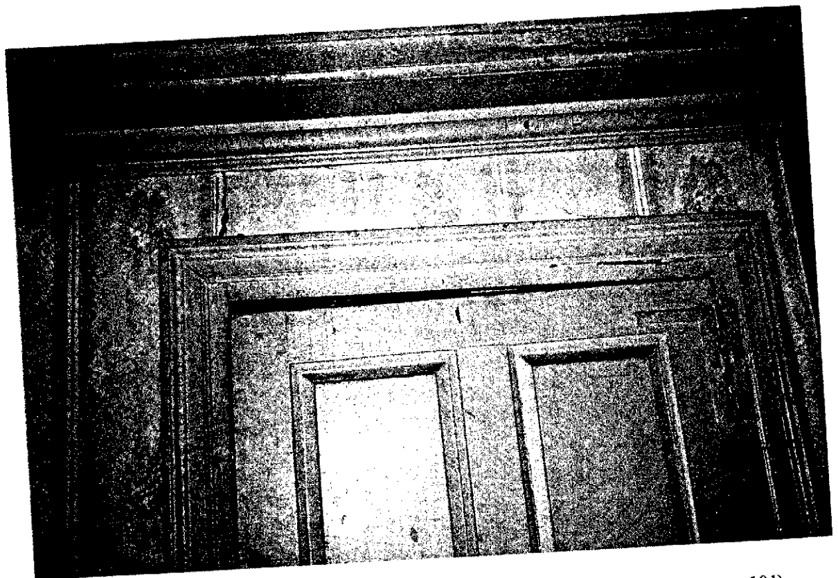
Figure F-9. Out-of-level door frame, east doorway of the southwest room (Room 101).
