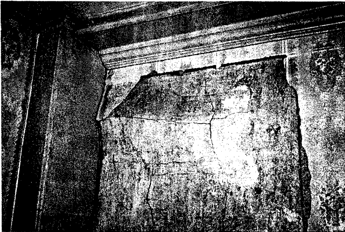
Figure F-6. Buckling plaster wall, northeast corner of the southwest room (Room 101).
