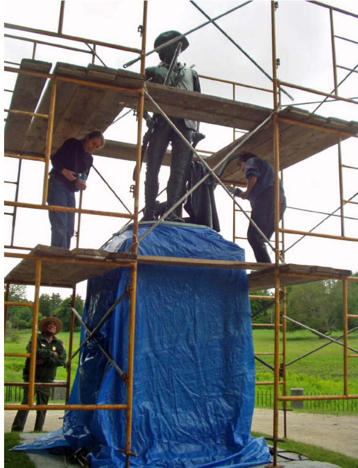
During treatment, CCB conservators apply heat with propane torches to drive off moisture before applying Incralac coatings.
