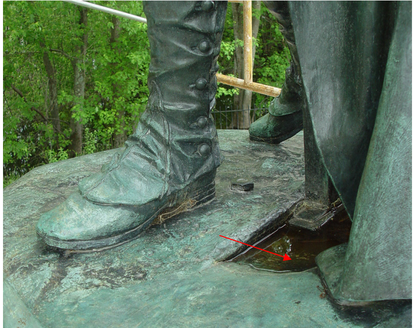
Standing water in recess of base.
