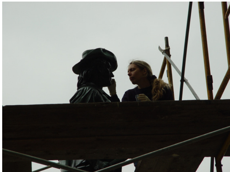
After brush coat of Incralac was applied, weathered areas in the patina are toned with pigmented Incralac.
