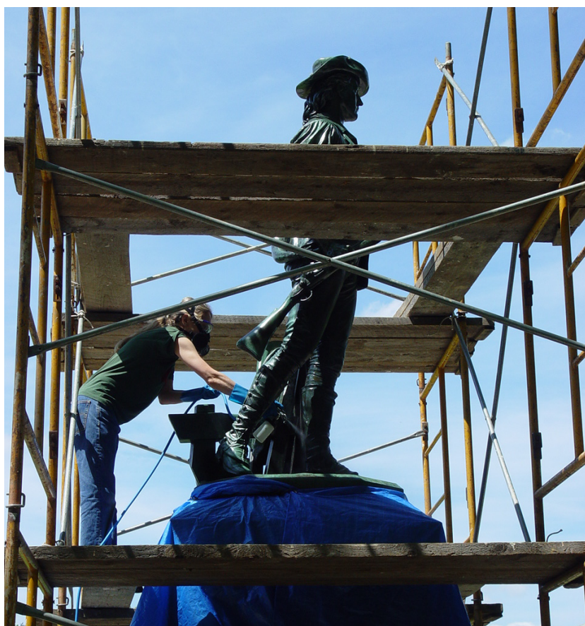
CCB Conservators Carol Warner and Margaret Breuker apply spray coats of Incralac.
