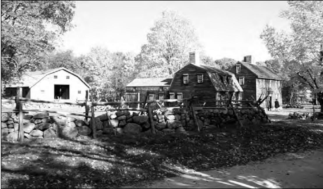
Figure 106. Thrown stone wall restored by the NPS along the Battle Road Trail at Hartwell Tavern, 2004. (OCLP)
