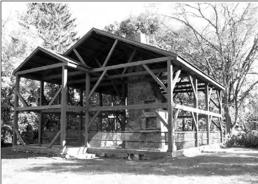
Figure 137. View east of the Samuel Hartwell chimney and the NPS constructed protective frame structure, built on the footprint of the Samuel Hartwell house, 2002. (OCLP)
