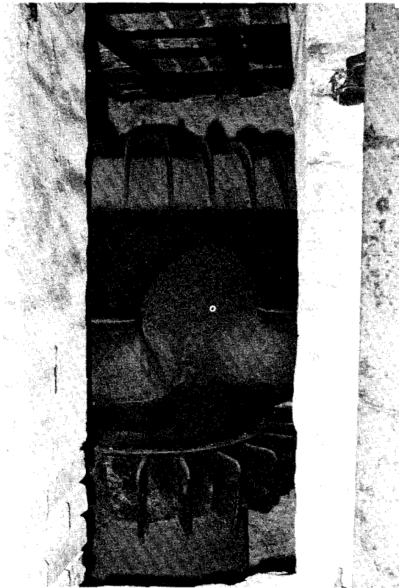
IP082, N010-07. Boynton's patent cast-iron furnace.
