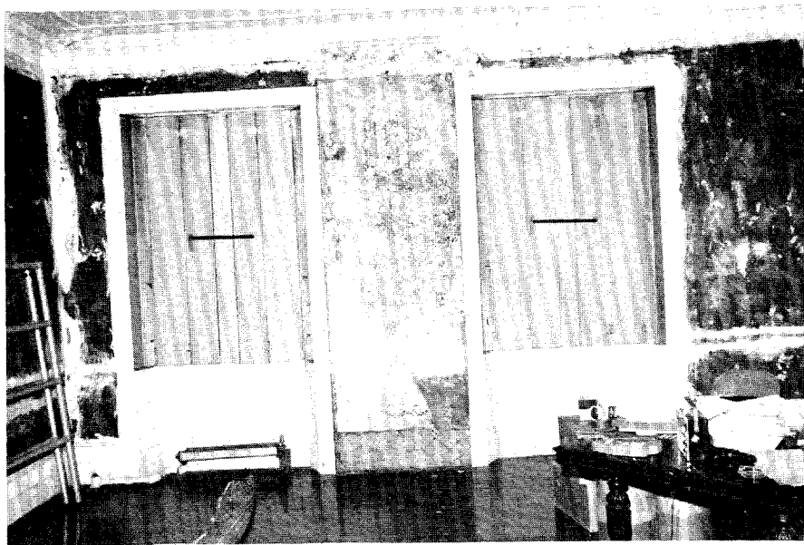
IP030, N023-24. Room 106, east wall. Note historic wallpaper revealed by removal of mirror between windows 101 and 102.
