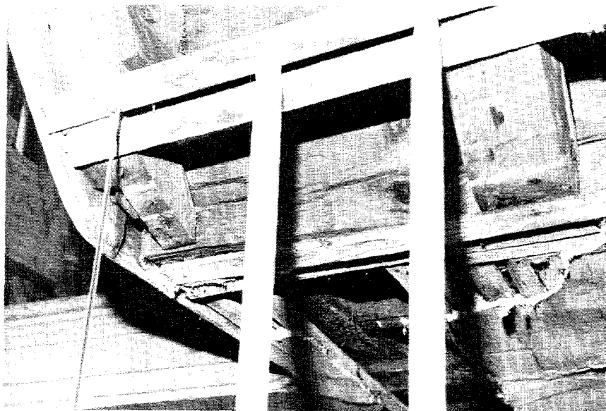
IP075, N041-06. Same area as IP069 (above), looking northwest and slightly up. Note stair stringers at top of picture. Horizontal joist is cantilevered from east wall. Tenon of previously mentioned stub joist appears at west end of cantilever above stair stringer.
