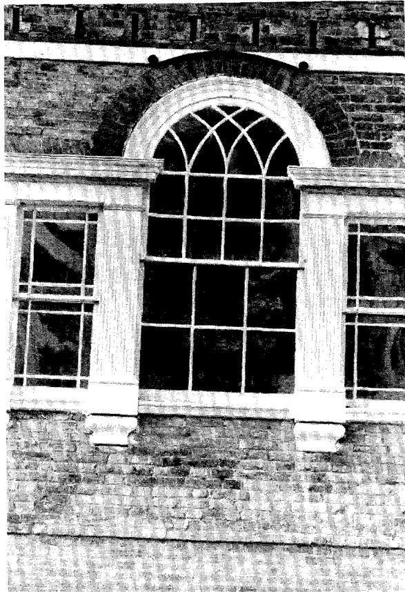
IP013, N013-05. Window 204, ca. 1797 "Gothick" sash above ca. 1840 six-light sash.
