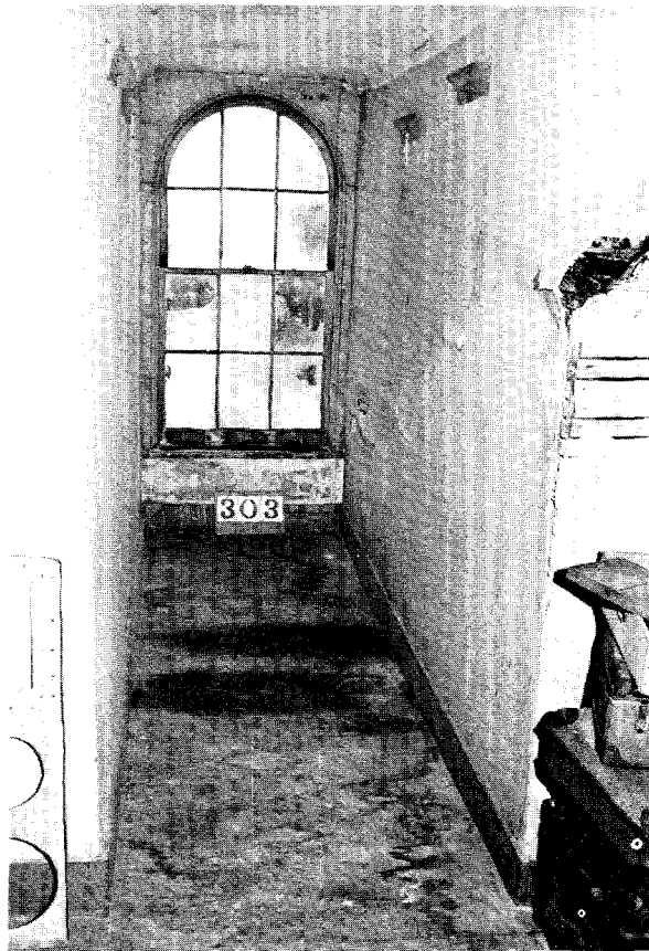
IP062, N008-15. Room 303 eastward dormer extension and window 303.
