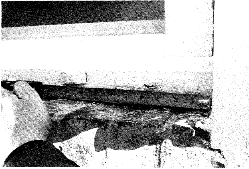
IP137, N034-04. Wrought-iron pintle for exterior shutter blinds.
