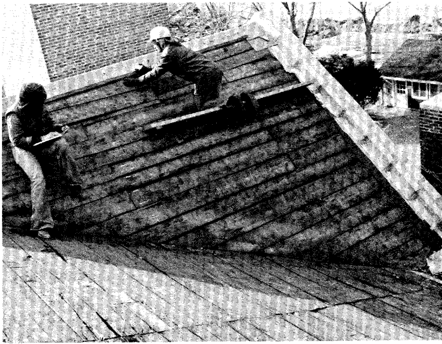
IP007, N039-14. Gable sheathing.
