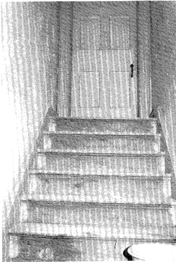
IP065, N032-09. Room 307, looking east up stairs to door 307.
