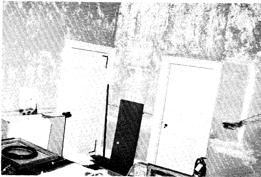
IP052, N030-11. Room 210 north and east walls, doors 215 and 216.
