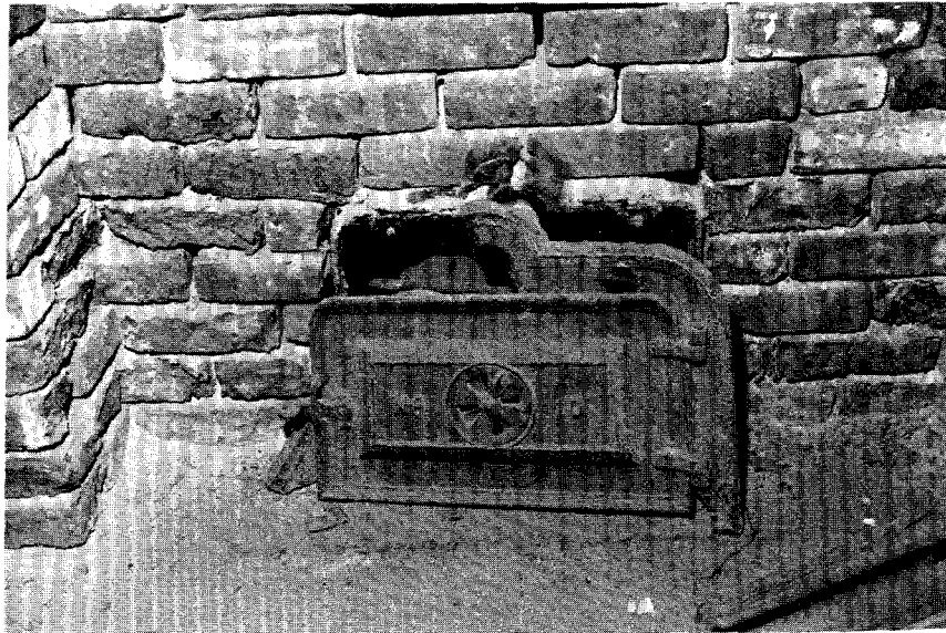
IP084, N010-10. Cast-iron ash cleanout door.
