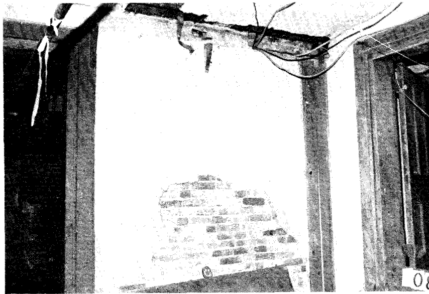
IP101, N009-20. Room 009, northeast corner. Note remains of wooden pipe chase.
