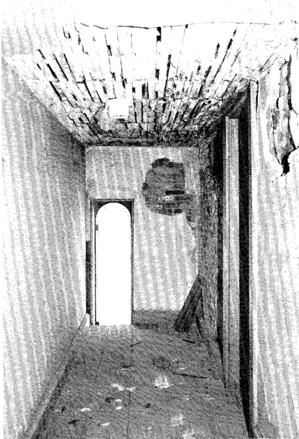
IP064, N032-6. Room 307, looking south past door 309 to window 315.
