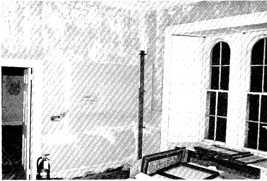
IP053, N030-10. Room 210, east and south walls, door 216, and windows 215 and 216.
