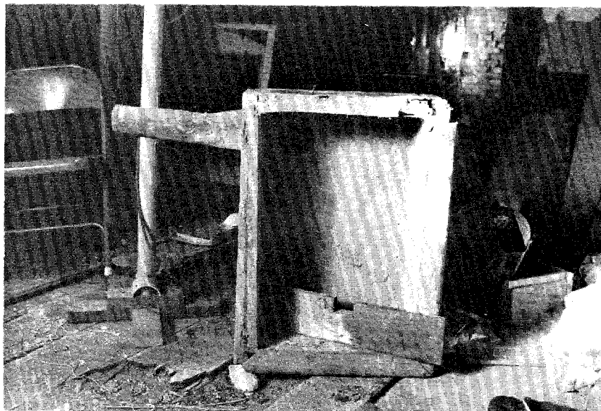
IP092, N001-08. Laundry room, room 007, sink.
