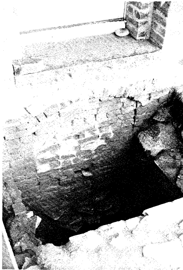
IP009, N004-19. Exterior view of door 010, probable entrance to cold storage area.
