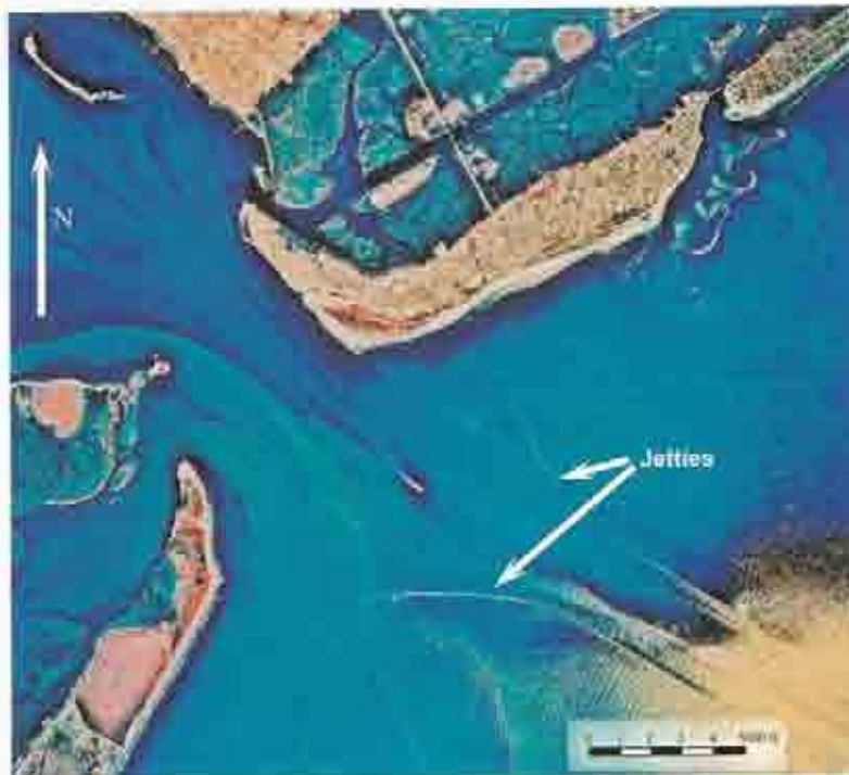
Figure 8.24. Aerial photograph of the Charleston Jetties (courtesy USGS).
