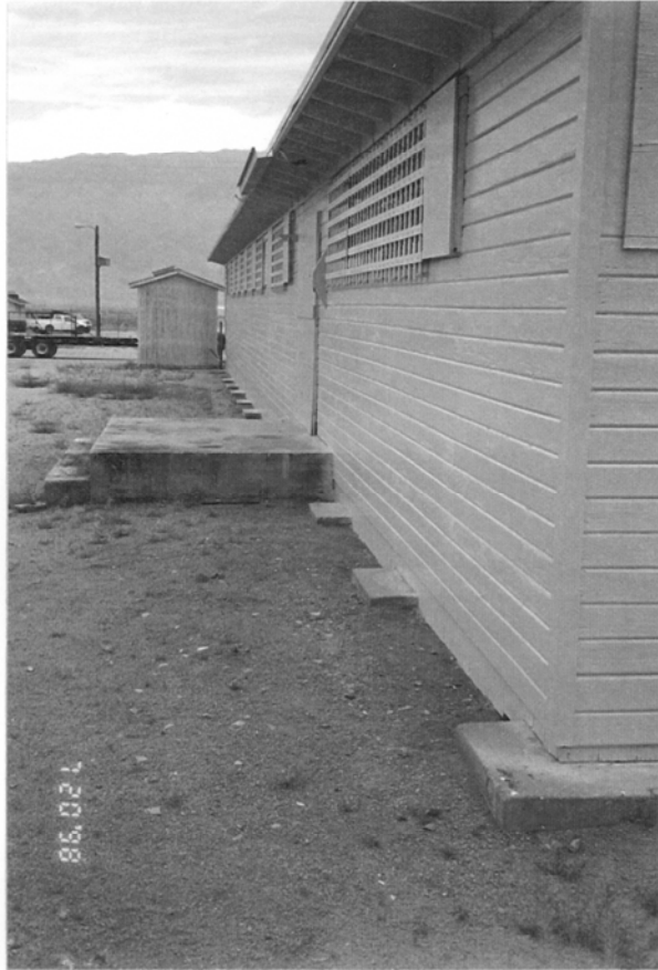
Photo No. 9 Exposed Footings on North Wall of North Wing
