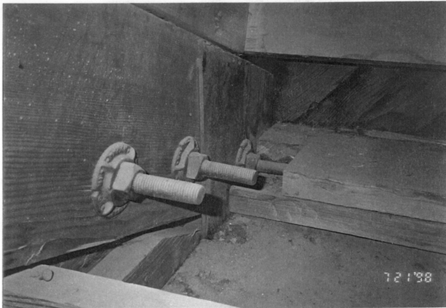
Photo No. 19 Two 2x Top Wall Plate Discontinuous at Truss to Column Connections
