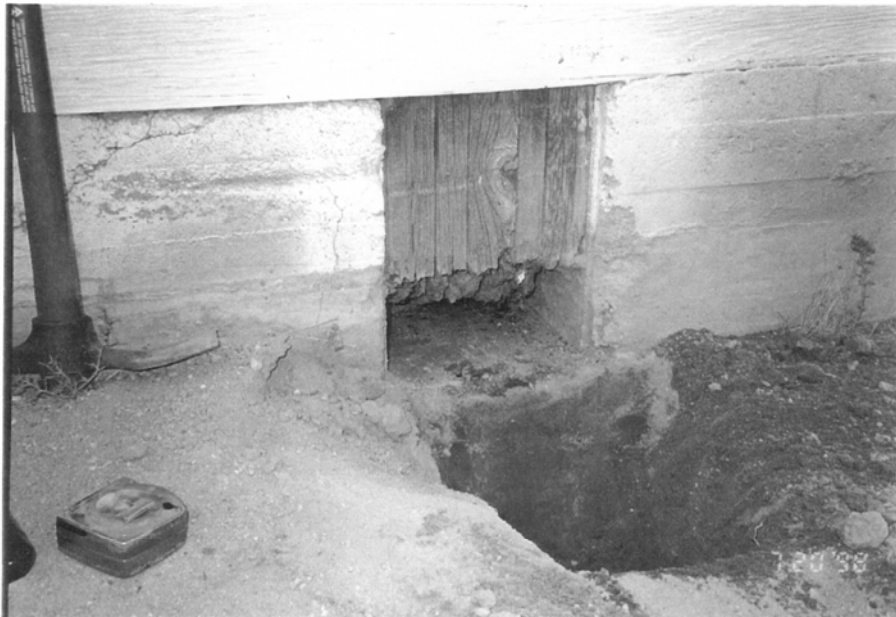
Photo No. 14 Decayed Bottom of Column
