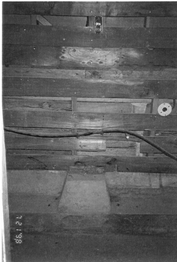
Photo No. 21 Auditorium East Wall with Remnant of the Original Wood Floor
