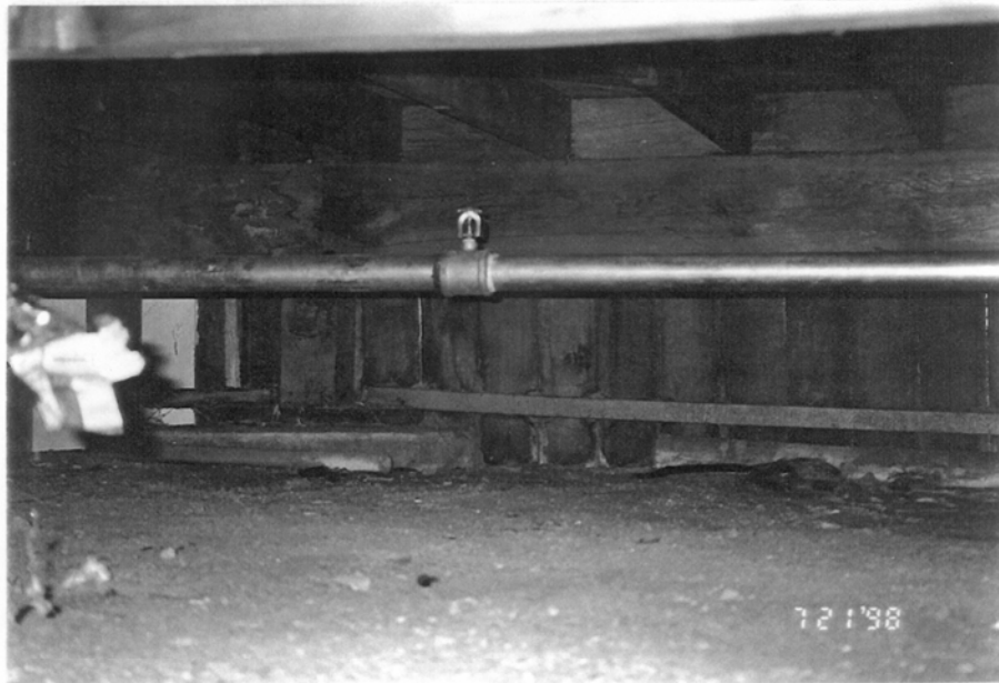
Photo No. 17 Unbraced Cripple Wall at North Wing
