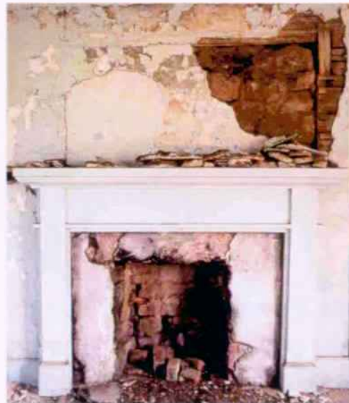
The over mantle area in Room 202 shows evidence of multiple layers of finishes as well as the original plaster over lath construction. No fewer than 5 layers of finishes have been discovered in this area.
