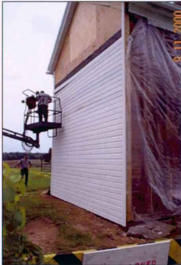
Figure 11. New exterior siding being installed over felt paper underlayment over \frac{3}{4} inch CDX plywood wall sheathing. 09/11/2000
