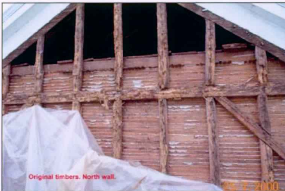
Figure 7. North Elevation Gable End with Exterior Siding and Sheathing Boards Removed. 07/26/2000
