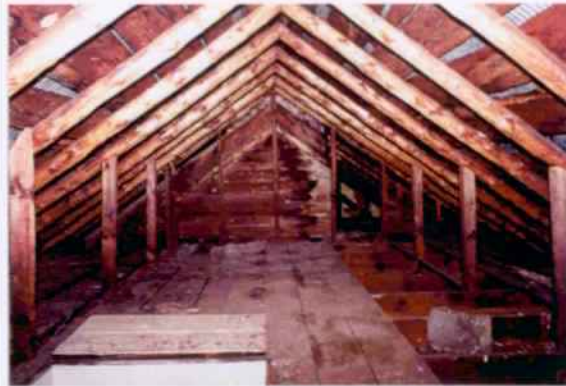
South attic, view of north gable wall, attic hatch and attic floorboards. North gable is first period construction exterior wall.
