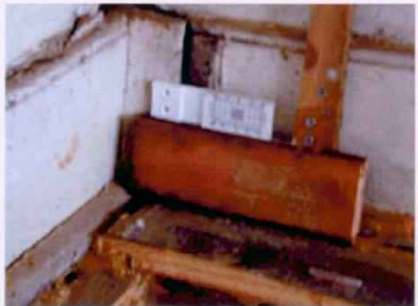
Crack 2 at SE corner of room supported by wood blocking to measure at bottom of wall to track floor width movement.
