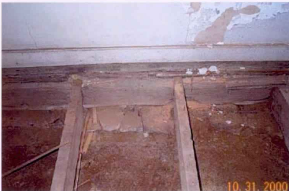
Figure 18. WSW Quad, north of SW corner, view of west wall sill plate and joists.
