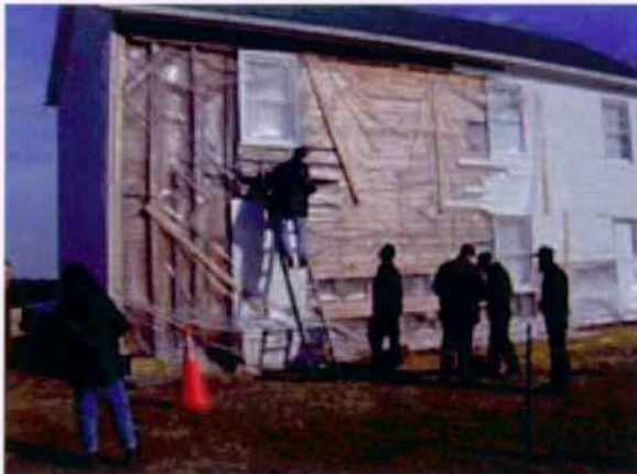
Fabric Investigation and Structural Evaluation of Exterior Wall Frame System at North Block.
