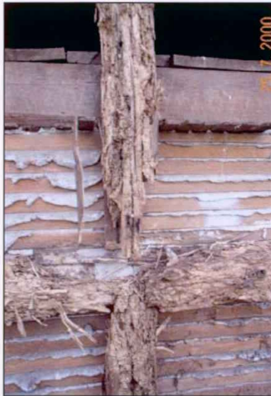
Figure 9. North Elevation Gable End, vertical stud and horizontal wall plate exposed. Attic floor planking and top wall plate seen above wall lath with plaster keys exposed.
