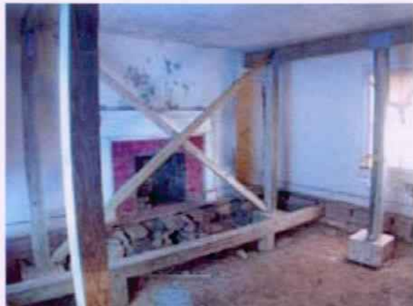
RM 102 with beginning of temporary emergency structural stabilization system installed. This system was designed to relieve the load of the building from the building frame.
