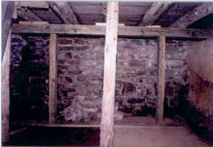
East stone foundation wall in north cellar represents typical mortared construction for this part of the house.
