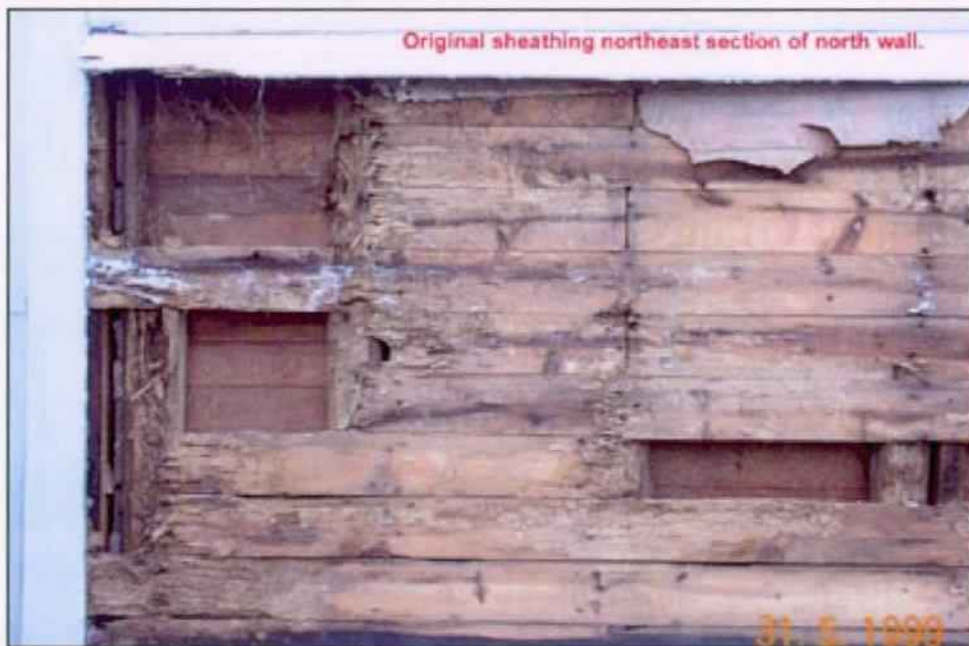
Figure 6. North Elevation at NE corner – wall sheathing exposed after exterior siding has been removed.
