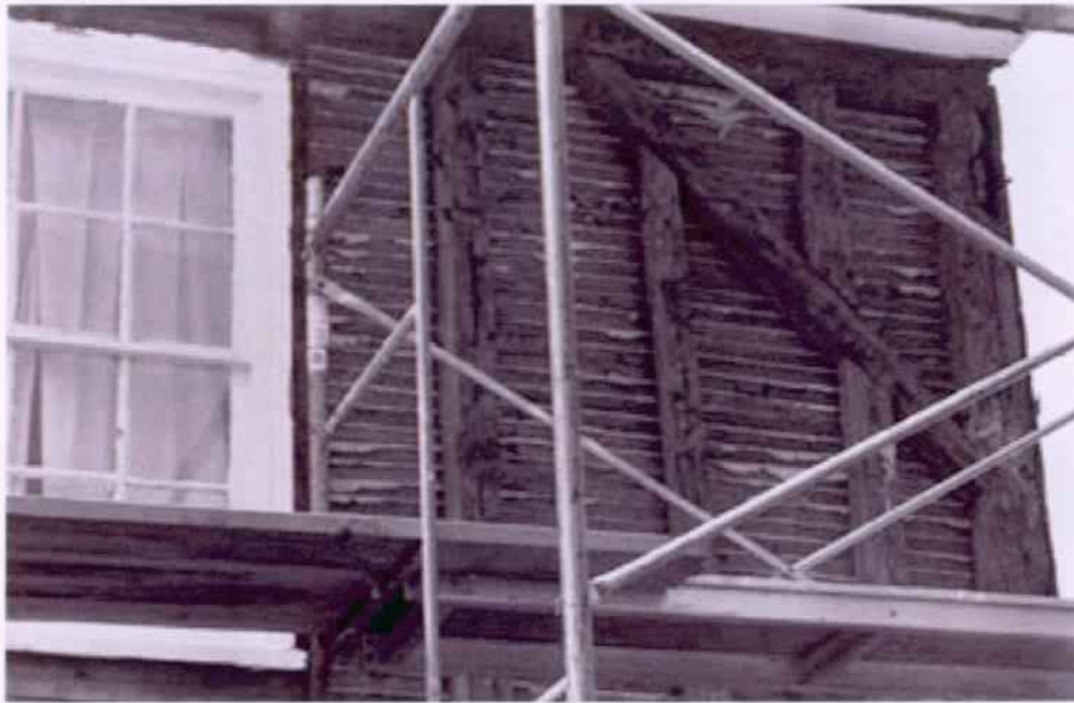
Figure 7. View of upper section of NE (north block) corner reveals diagonal corner post as part of braced frame construction method. Brace is notched (mortise & tenon) into corner post and top of wall frame. Note exposed lath and plaster marks historic interior wall surface.
