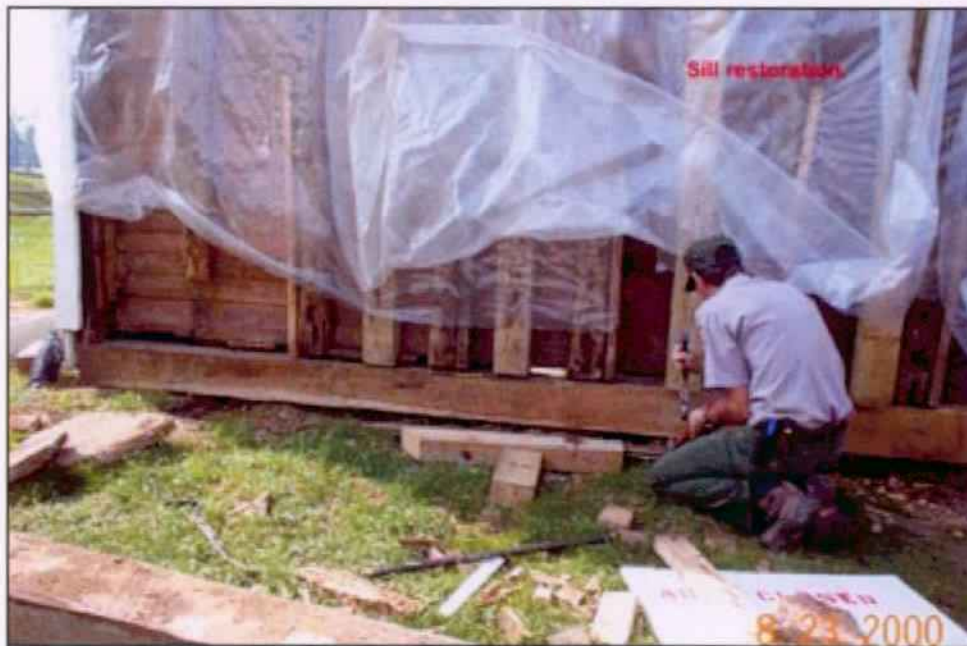
Figure 8. North Elevation Gable End replacement sill installed. 08/23/2000
