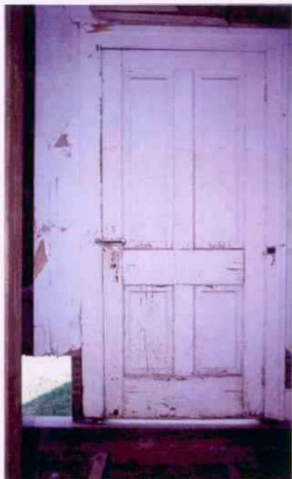
Typical plain 4-panel door used throughout the south block for the first period on construction. D106 at R103. 08/01.
