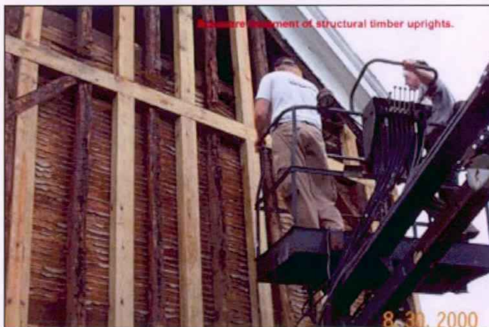
Figure 4. Boracare treatment of structural framing members at north elevation gable end. 08/30/2000.
