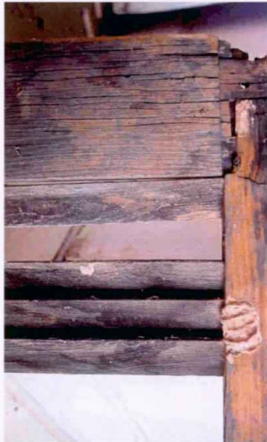
Shutter in inverted position to view mortise and tenon construction of frame, note pegged connection and thru tenoned detail.
