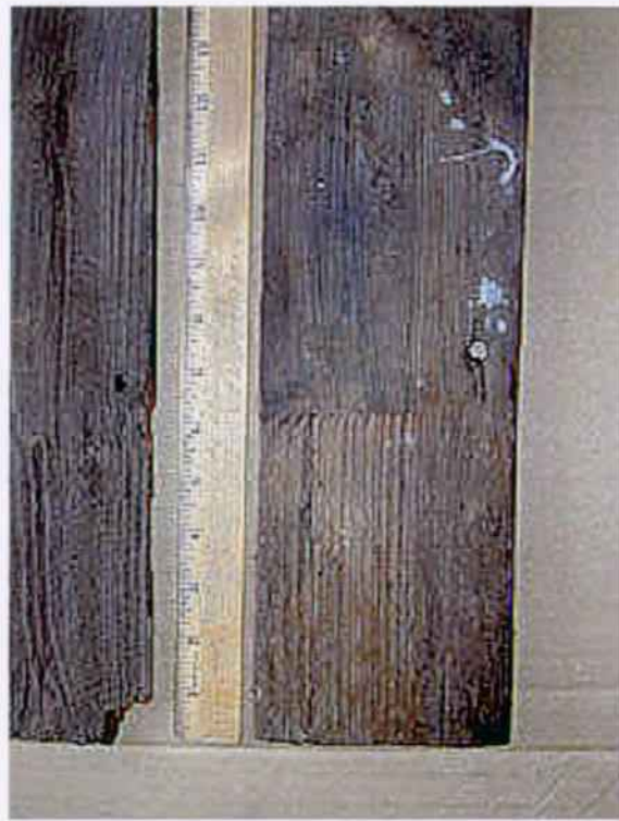
Detail showing exposure pattern, shown with 18 inch ruler. Note exposure area at lower edges of the shingles, this is the 5 inches to the weather described in the text.
