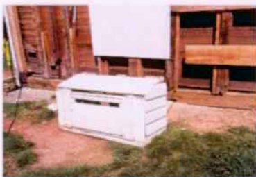
Wood frame cellar vent hood, exterior vent slats are covered with plywood.
