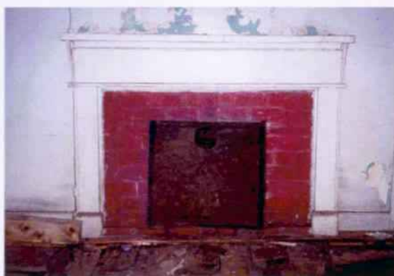
Firebox and mantle on north wall of R102. Center view shows braced mantle shelf and plain frieze and pilasters of the mantle casings.
