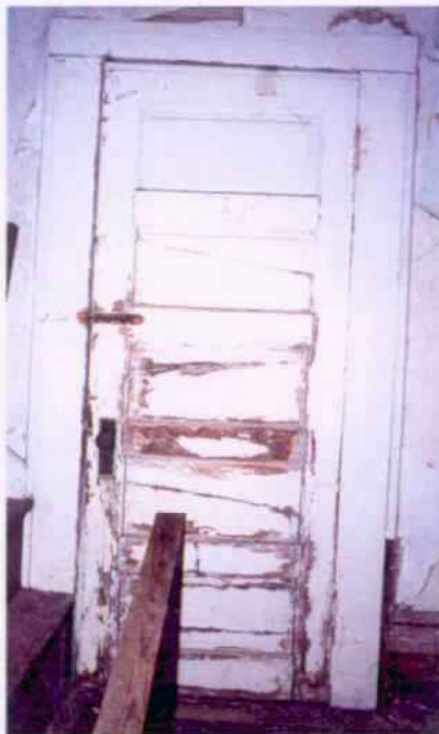
Later period door installed at south elevation during remodeling of entry hall, D105 at R103 in the south block of the house. 08/01.
