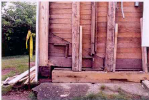
NORTH ADDITION: Lower West Elevation; sill plates, corner post, wall studs and interior sheathing exposed.
