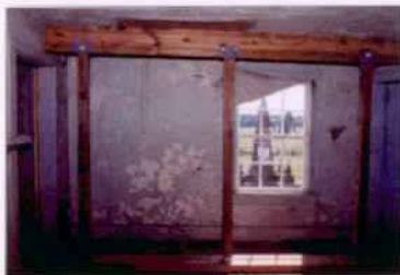
R202, East wall, W202. Temporary emergency structural system bracing seen along wall.
