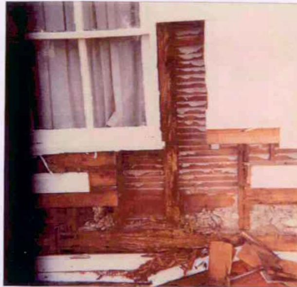
W102, SE portion of south wall, deteriorated sill plate and structural wall frame components exposed.
