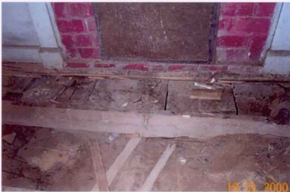
Figure 10. North Wall with Fireplace and Hearth Framing at center.
