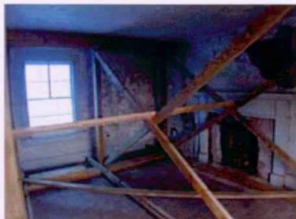
RM 202, Northwest quadrant. The Temporary emergency structural stabilization system provides lateral and longitudinal support for the house frame through a series of diagonal cross-braced vertical trusses using floor, ceiling and wall supports shimmed tight against the existing wall surfaces or fastened to the historic structure.
