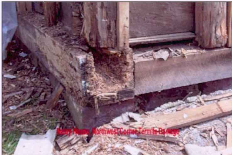
Figure 10. Northwest corner of building with north sill plate exposed with damage.
