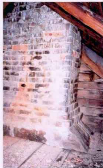
Stone chimney base with brick throat extending through roof line
