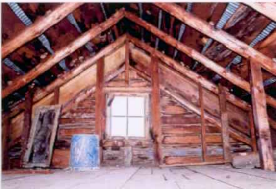
South attic, view of south gable interior, W310 at center. Note 10 inch wide frieze boards at top of gable and post and pole framing.
