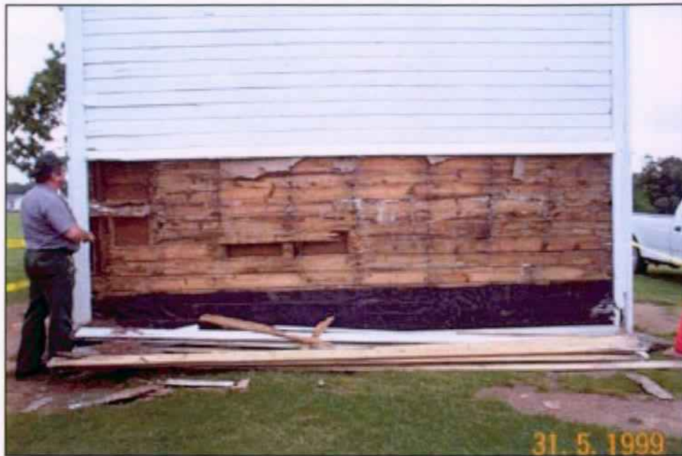
Figure 1. North Elevation Gable End – Exterior Siding Being Removed. 05/31/1999
