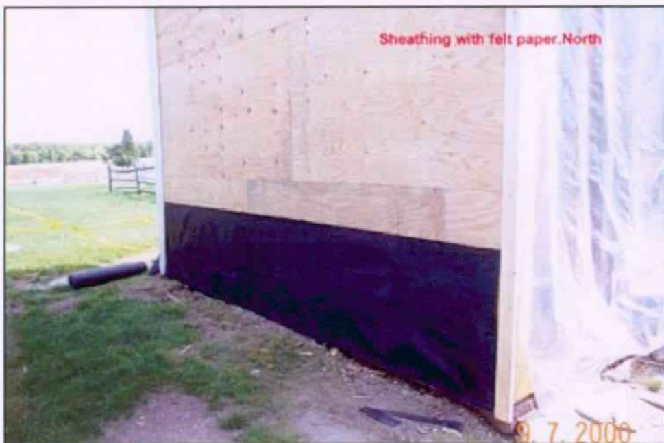
Figure 10. North Elevation Gable End – \frac{3}{4} inch CDX plywood sheathing installed over new pressure treated wall framing members, felt paper installed over plywood.
