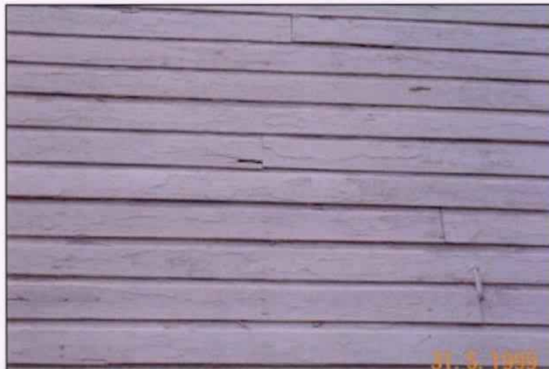
Figure 2. Detail exterior "German Style" ship-lap weatherboard siding, prior to 1999/ 2000 north elevation repair project. 05/31/99
