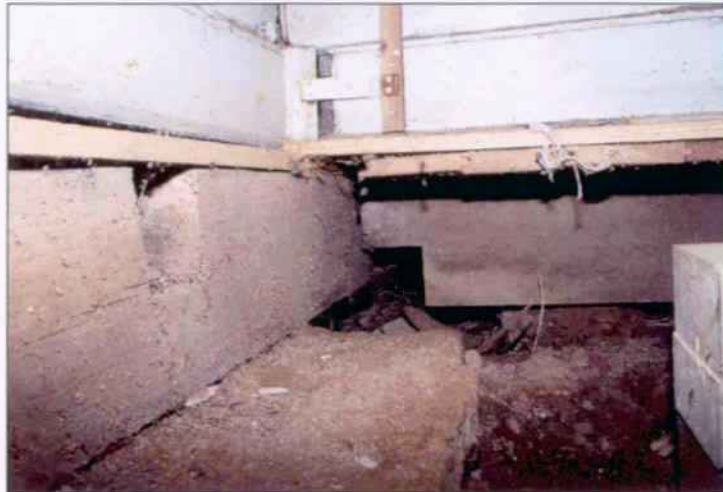
East wall sawn sill plate is notched for floor joists. Sill plate sits on shallow stone foundation. Floor joist is not connected to sill plate at this location.
