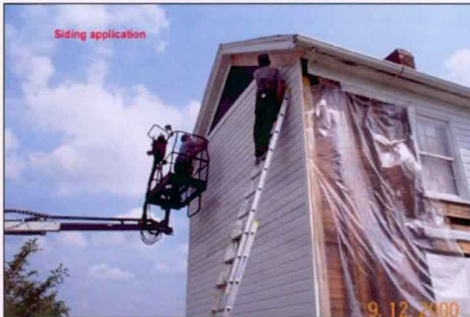
Figure 12. Installation of third generation replacement exterior siding at north elevation gable end almost completed, 09/12/2000.
