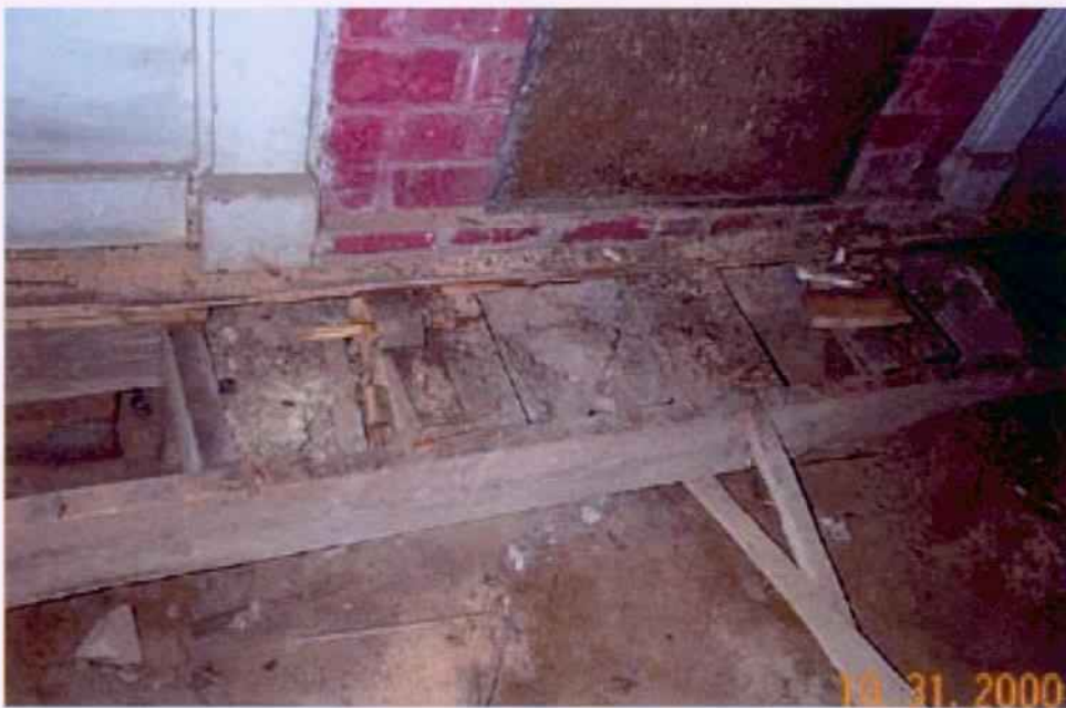
Figure 8. NNW Quad with Fireplace Hearth Framing.
