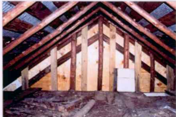
North attic, view to largely reconstructed north gable wall.
