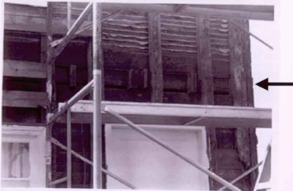
Figure 8. The horizontal ribbon board used to support the second floor joists is clearly visible in this view (arrow). This method of construction helps date the house frame and provides information about the sequence of construction. The ribbon board (riband) is attached to the continuous vertical framing members and the floor joists are notched over it and face nailed to the vertical framing member.
