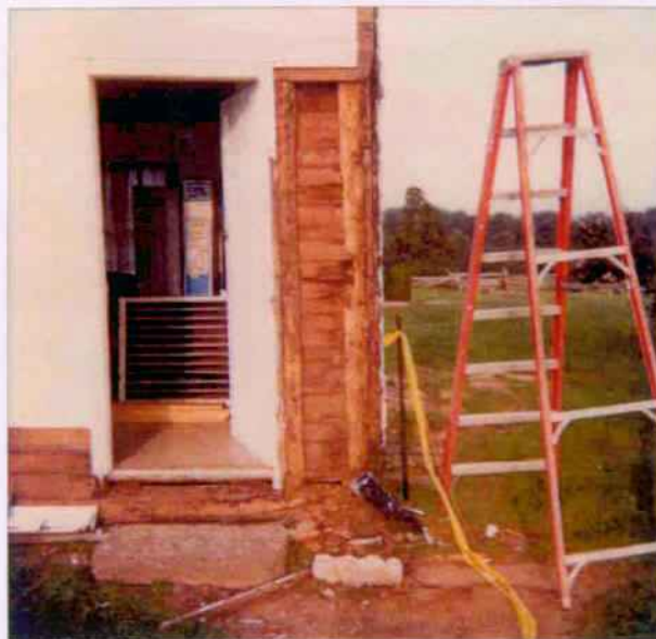
D101 @ East Elevation, Siding Removed to Reveal Severely Deteriorated NE Corner Post.
