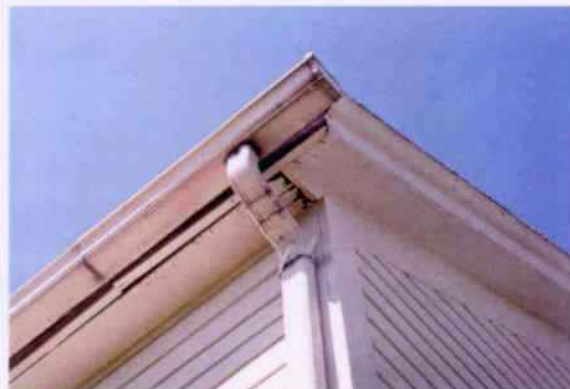
SW corner detail of cornice, gutter and downspout.
