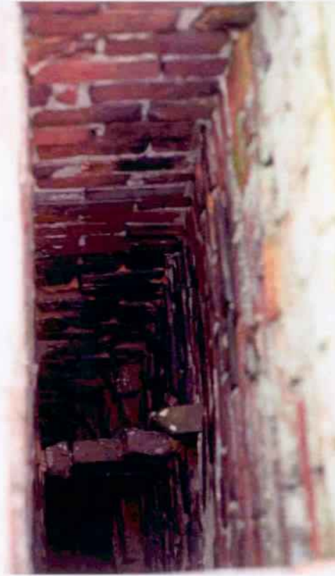
View down throat of chimney showing one wythe brick flue divider.
