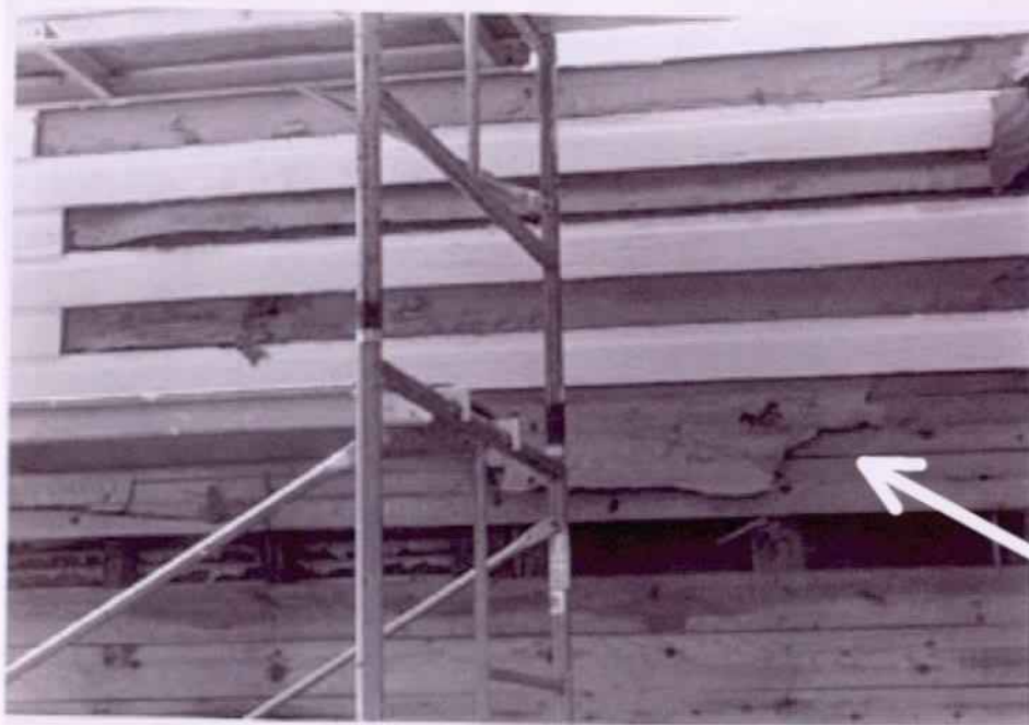
Figure 6. This view of the east wall construction reveals the use of a building paper (at arrow) between the exterior "German Style" shiplap weatherboard siding and the tongue & groove sheathing boards. Overlap pattern of siding boards dates to installation c. 1930's when it was installed to replace the 19 th century non-tapered lapped weatherboard siding. Lath and plaster visible at interior of south block. North block is to right of scaffold brace in foreground.
