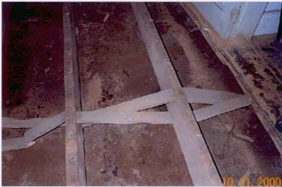
Figure 16. SSE Quad with Joist Bridging at D103.
