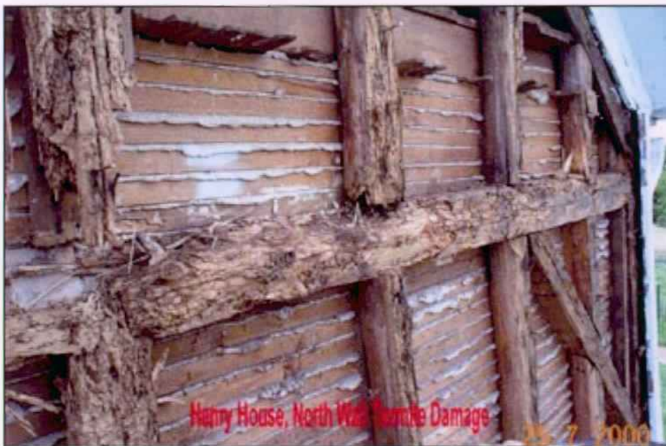
Figure 8. North Elevation Gable End timber frame exposed after removal of exterior siding and wall sheathing boards. 07/25/2000
