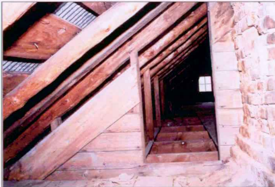
View from north attic through wall opening in north gable wall into south attic. Note 10 inch wide first period frieze board and exterior siding boards – all unpainted. Note also transition of chimney construction from stone to brick just above the finished floor.
