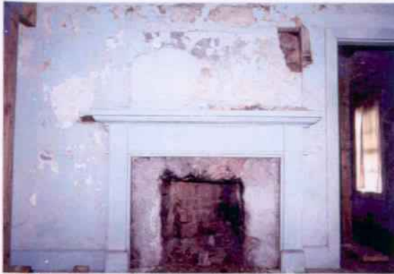
R202, plaster lined stone firebox at chimney and wood mantle centrally placed on north wall of room. 07/01.
