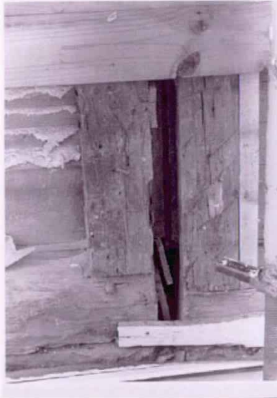
Figure 5. Detail photo documenting two outside corner posts at middle of current east elevation marking addition of north block to south block of house. Left post is first period of construction (south block); right post is from second period of construction (north block).
