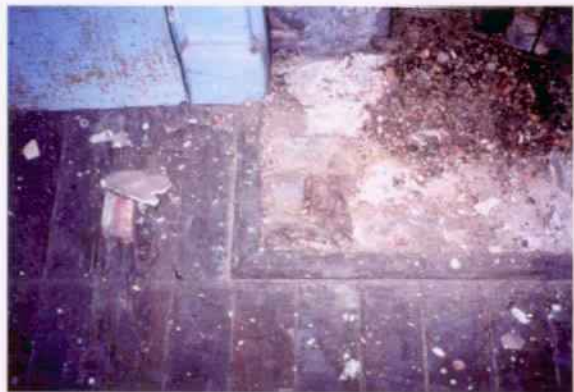
R202. Hearth area located at mouth of firebox. Bricks are laid out into room and area is trimmed with elongated quarter round wood trim. Floor in room is wood strip flooring.
