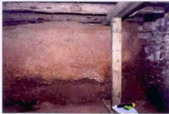
North Cellar, southwest interior view of earth embankment that supports chimney at juncture with west foundation wall.
