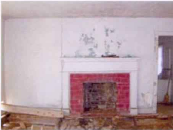
RM 102. Floor to ceiling crack is seen to west of mantle on north wall of room. Note missing floor joists. Monitored as Crack 1.
