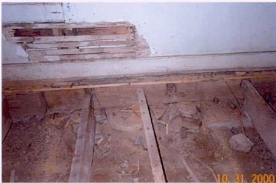
Figure 6. East Wall Near Center, further north, showing empty joist pocket.
