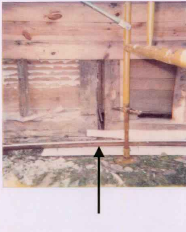
Double posts indicate location of south and north block point of adjoining structures.
