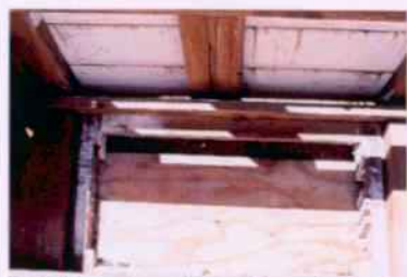
Interior of well vent hood, note mortised grooves for missing vent slats at inner frame.
