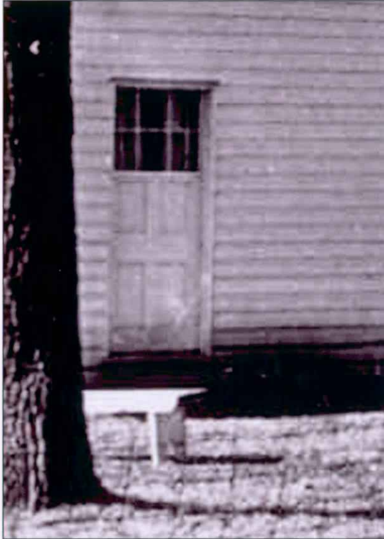
Figure 30a. Electronic (non-photographic) enlargement of HFC HPC MANA 430 (Figure 30). The east cross hallway door with a large 6 light transom window (possibly actually a window sash given its proportion) is seen in this rare rear view of the house. This door was later removed and converted to a window (W103) as labeled on the drawings associated with the HSR.
