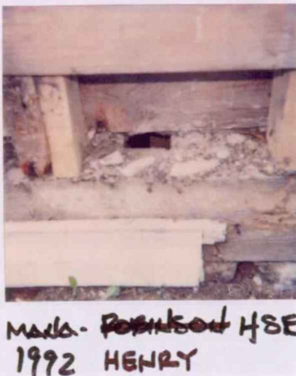
East Elevation Sill Plate with Termite Damage Prior to Repair
