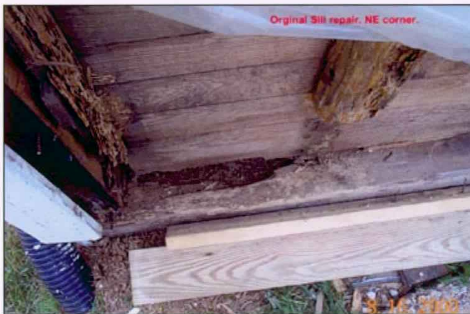
Figure 6. View of NE corner of building showing damage to original sill plate and vertical framing members. 08/16/2000.
