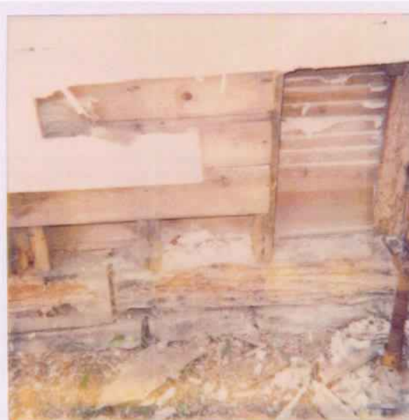
W201 & NE corner reveal braced frame construction and balloon frame at north block.
