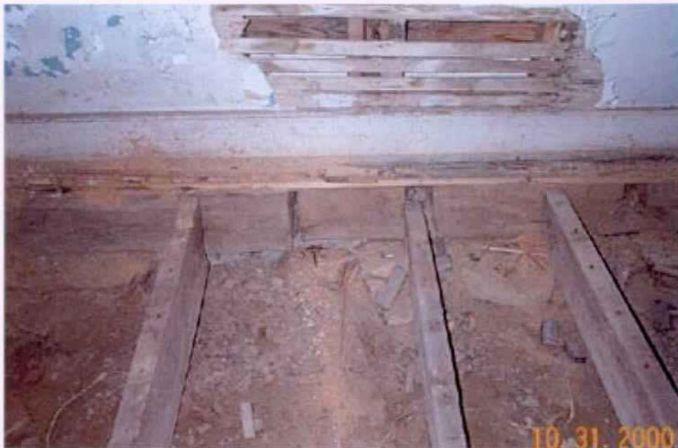
Figure 5. East Wall Near Center, note split in sill plate between joists.
