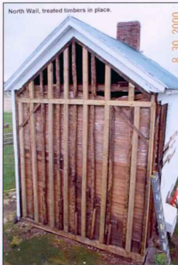
Figure 3. North Elevation Gable End – treated timbers in place. 08/30/2000.
