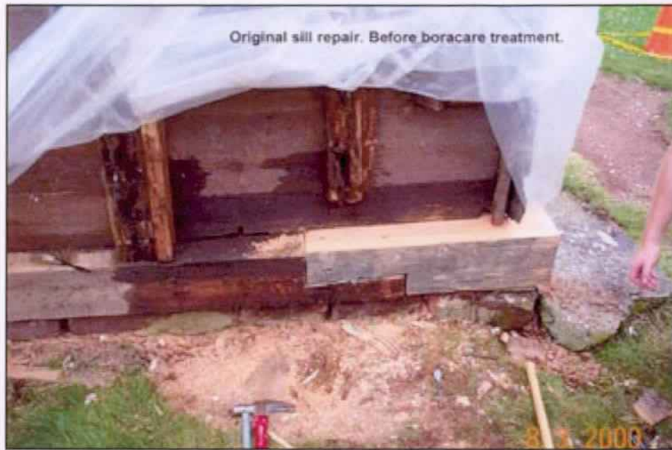
Figure 7. Repairs made to original sill of north elevation gable end at NW corner. Note corner post is not seen in this view. 08/03/2000
