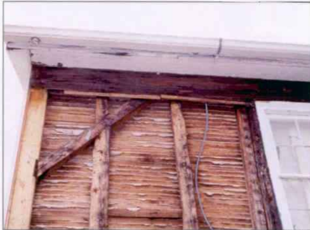
Corner Brace at northwest corner post in north addition.
