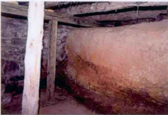
North Cellar, southeast interior view of earth embankment that supports chimney at juncture with east foundation wall.
