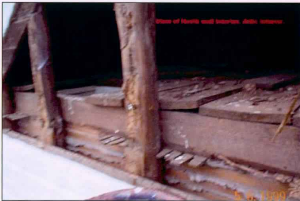
Figure 12. North Elevation Gable End framing exposed, note attic floor planking and top of wall plate over ceiling lath. 05/06/1999
