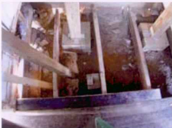
RM 103, Stair Hall at South Block with Temporary emergency Structural Stabilization system partially constructed. New floor joists and vertical posts provide load bearing capacity for historic framed structure of house.
