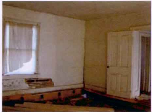
RM 102. SE quadrant of room. Floor to ceiling crack is at corner. Monitored as Crack 2.
