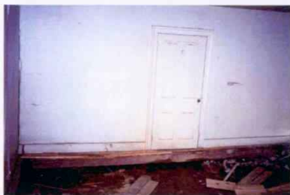
R102 south wall. Features baseboard, door casing for D103 and telephone shelf. Floor framing system has been removed. 03/01.
