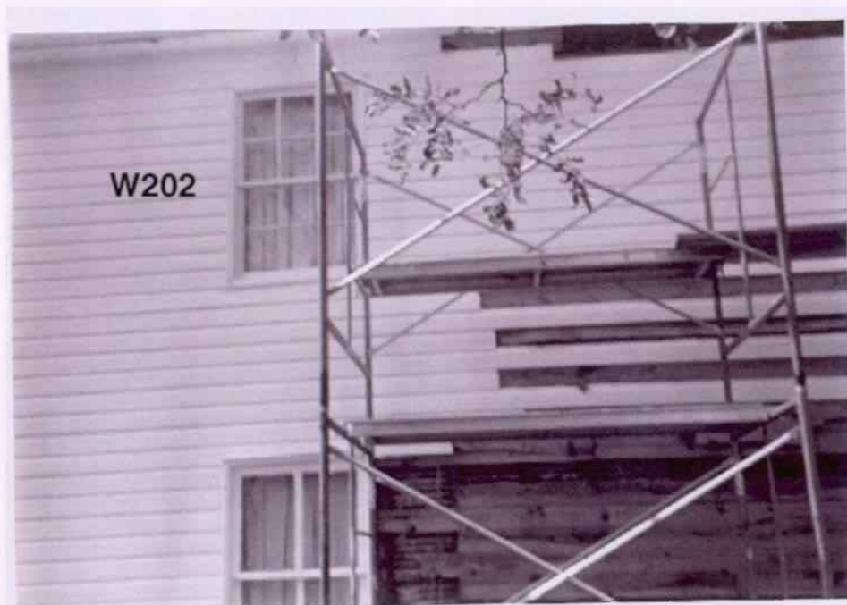
Figure 3. Documentation of extent of removal of exterior siding to investigate condition of wall structure and range of termite damage.
