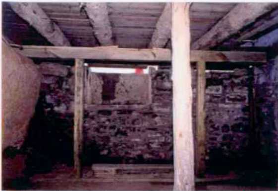
North Cellar, west foundation wall with cellar vent well cut into stone wall. Well is concrete.
