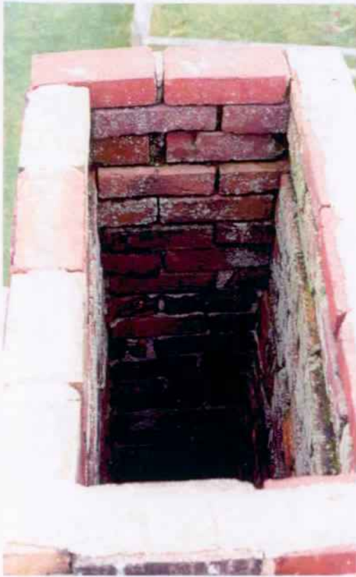
Birdseye view of top of chimney stack with thin mortar wash.
