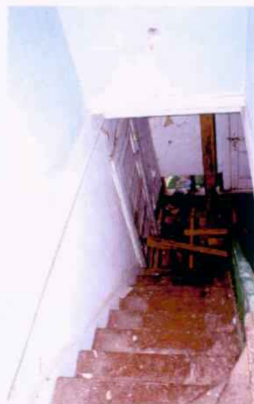
South stair S101 with R103 at bottom of stair. Note wall trim featured at south wall and bulkhead trim overhead.
