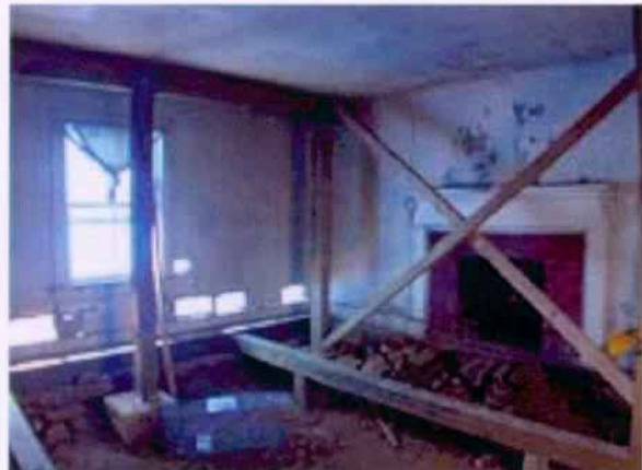
Temporary Emergency Structural Stabilization brace in place on 1 st floor. Note lack of exterior wall structure.
