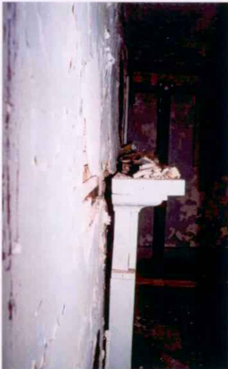
Profile view of west side of fireplace mantle in R202. Mantle is mounted against plaster wall (installed after wall was plastered).
