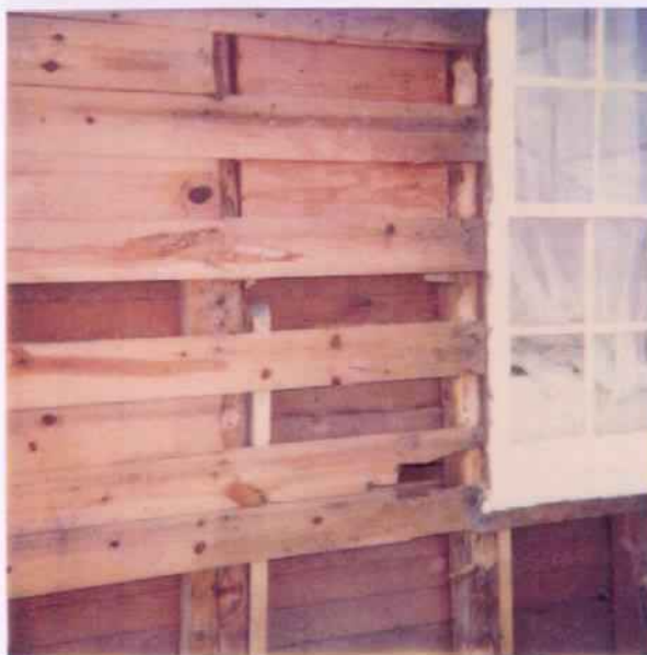
W101 @ North Block exposed window frame and subsheathing revealed after removal of exterior wall covering.
