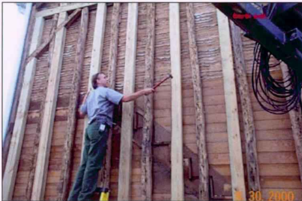
Figure 2. North Elevation Gable End – Pressure Treated framing Members in place to supplement insitu historic framing components. 08/30/2000
