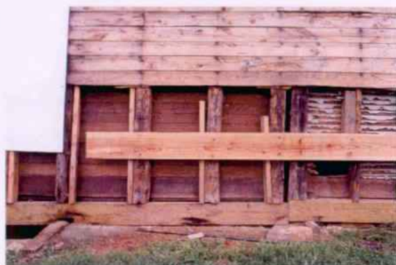
MEETING POINT between south block (right) and north addition (left), tow corner posts are visible in the center of the photo.
