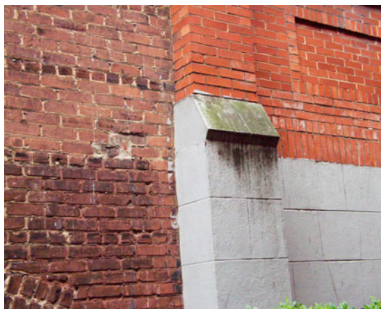
Detail of brick wall on east side. At right are red face brick and stucco used on primary elevations; at left is common brick used on secondary elevations. (NPS, 2000)
