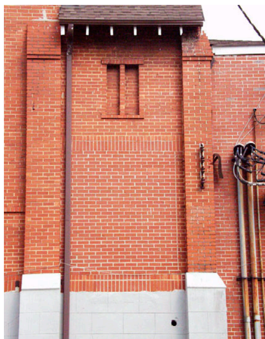
Detail from south end of west side, showing infilled door opening below blind niches. (NPS, 2000)
