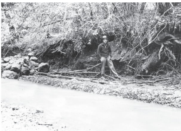
Figure 4.38 (below): Erosion around old basket-type revetment, photographed 1937. The identity of the person is not known. J. Barton Herschler, April 1937 monthly report. National Archives II, College Park, Maryland, RG 79, PI 166, E7, Central Classified Files, 1933-1949, Muir Woods, box 2293.
