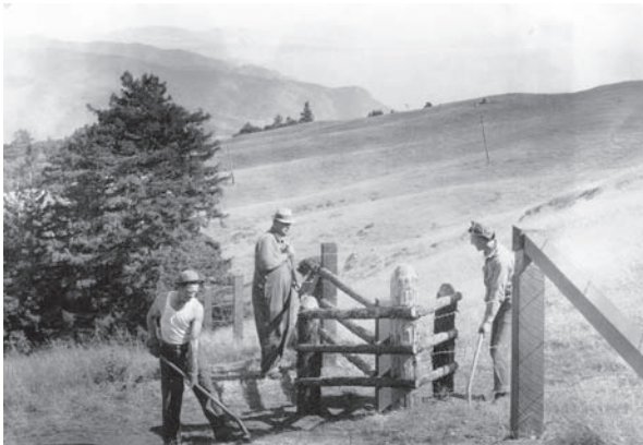
Figure 4.35: Looking southwest across Ranch X showing the west boundary fence and "V" stile under construction by CCC crews, June 1934. J. Barton Herschler, June 1934 ECW report. National Archives II, College Park, Maryland, RG 79, PI 166, E7, Central Classified Files, 1933-1949, Muir Woods, box 2293.
