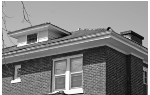
FIGURE 48. View of front dormer and capped chimney.
