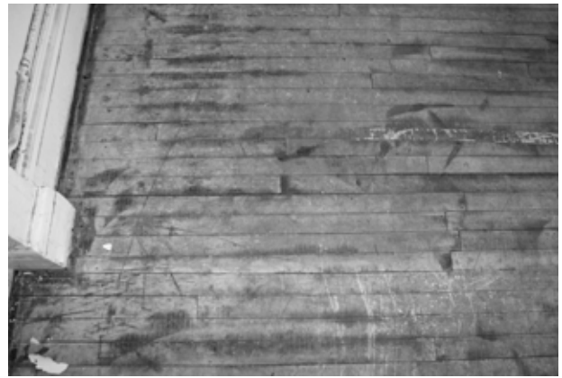
FIGURE 52. Oak flooring at location of former wall between Rooms 101 and 104.
