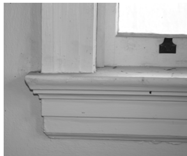
FIGURE 62. View of typical window casing and stool.
