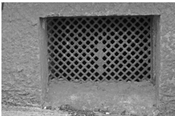
FIGURE 29. View of typical porch foundation vent.
