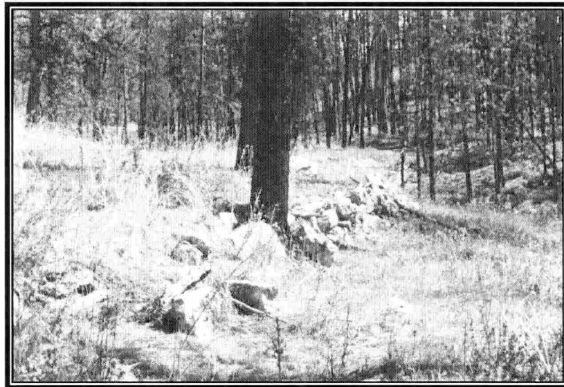
Figure 5-7. Stone foundation of Michaud log house, May 2004. Photo by Gail Evans-Hatch, Courtesy of Jewel Cave National Monument, deposited at Mount Rushmore National Memorial.
