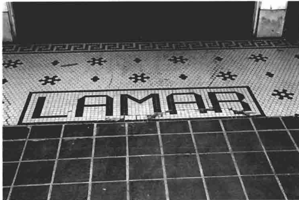
IC-12: West Site. Front entry tile at alcove and at stair entry platform (quarry tile). 11/2003
