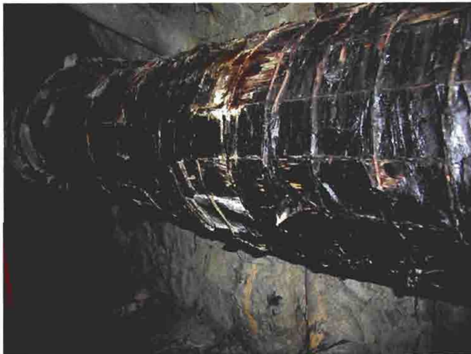
CA-5: The Creek Arch. The hot springs collection pipe.
