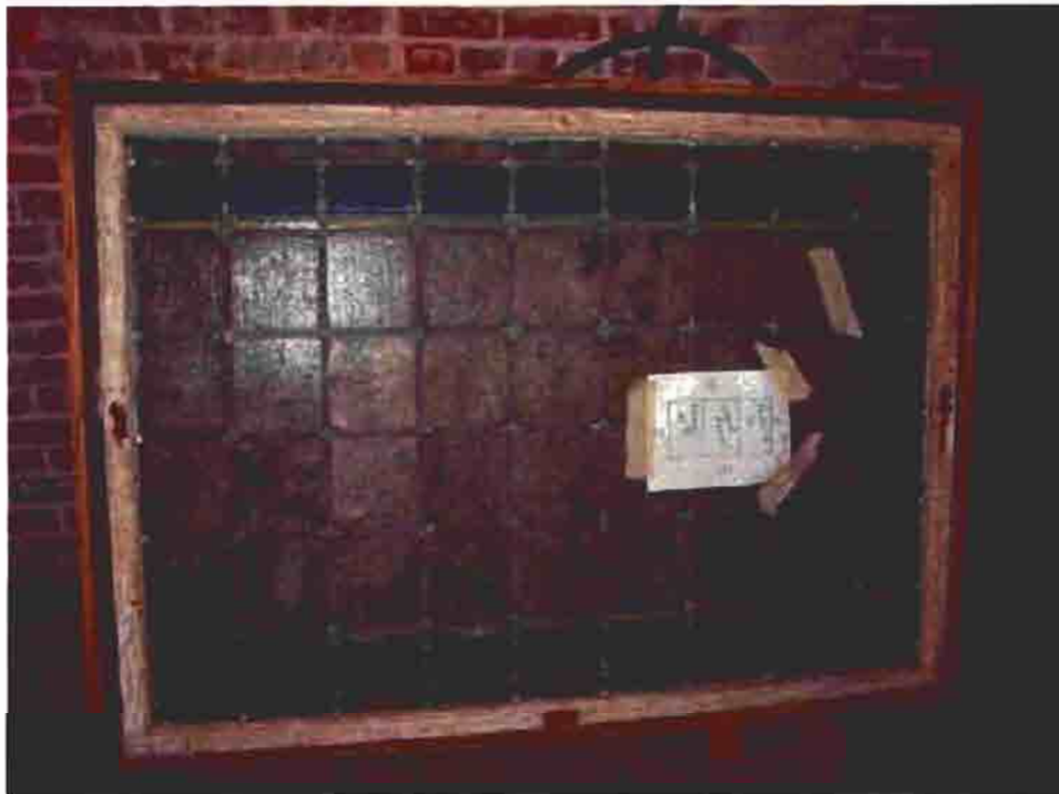
WOOD FRAMED PANEL: NOTE THAT THIS IS AN END PANEL, & EXHIBITS A TYPICAL LAYOUT DIAGRAM TAPED TO THE PANEL. THIS IS AN EXAMPLE OF A REPAIRABLE PANEL; IT IS IN GOOD CONDITION.
