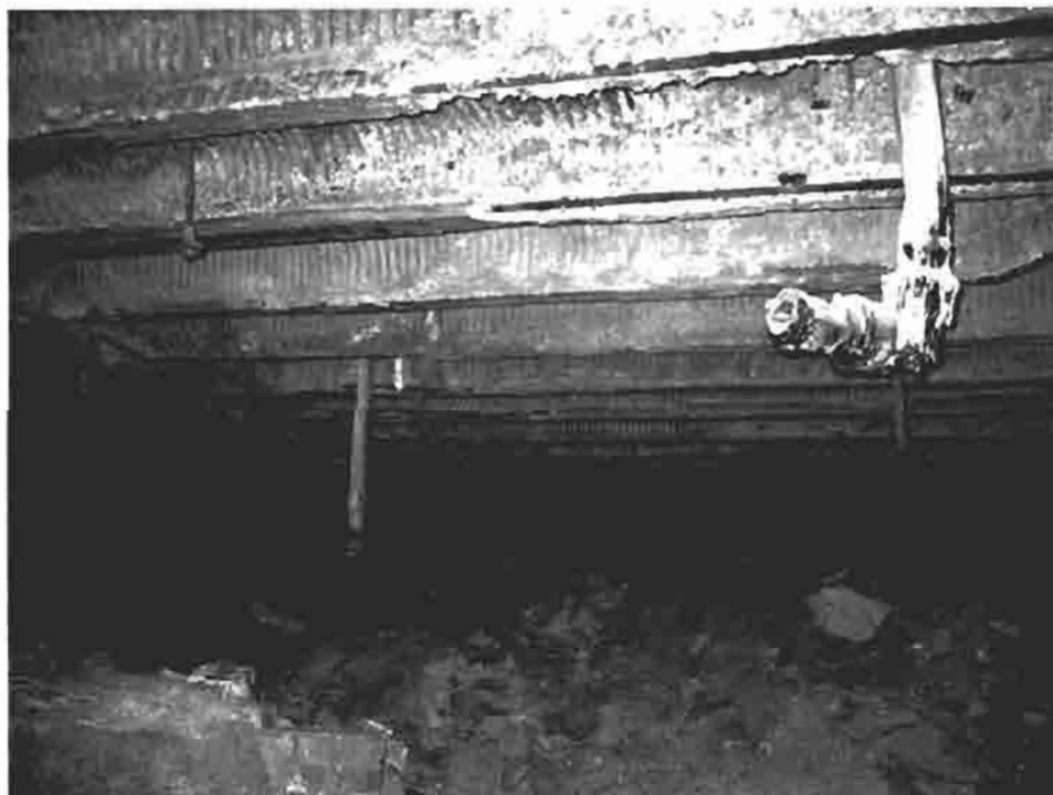
1C-55: Crawl Space: Northeast view: from Fuel Room 01: Note: Exposed rebar in beams. 11/2003
