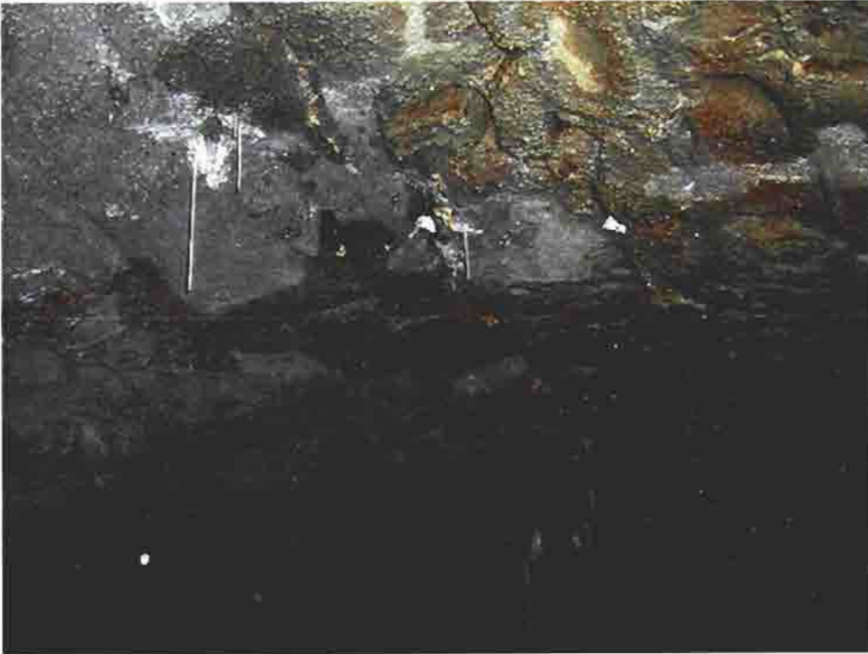
CA-8: The Creek Arch. A building up of stalactites from the arch surface. This is evidence of a steady drip.
