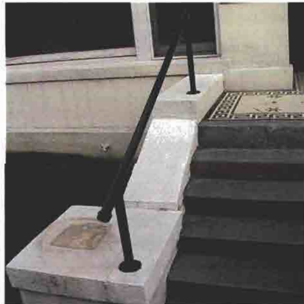
Figure CLA-6: Repair of degraded stairs and walls should replicate the existing profiles and finish. (Shapins Associates, 2003)
