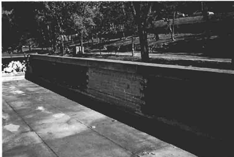
IC-43: Roof. The east parapet wall is mostly covered by roofing tar except where the differently colored brick is present. 11/2003
