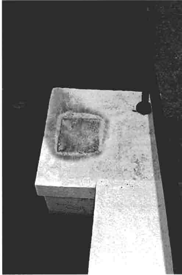
1C-49: Missing element from the west elevation. Historic photos show a garden urn at this loca- tion. 11/2003
