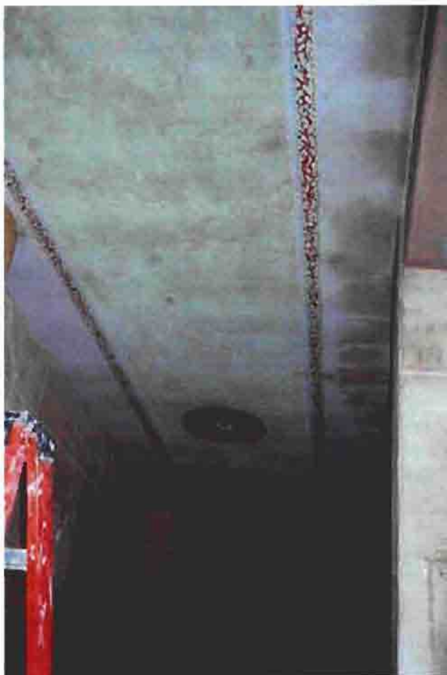
DECORATIVE PAINT: EXTENSIVE STAINING AT EDGE OF EAST CEILING PANEL.
