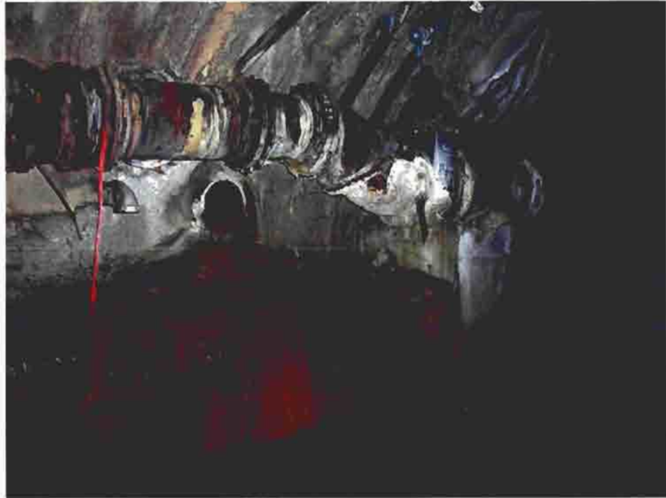
CA-10: The Creek Arch. The end of the hot springs collection pipe, with valves
