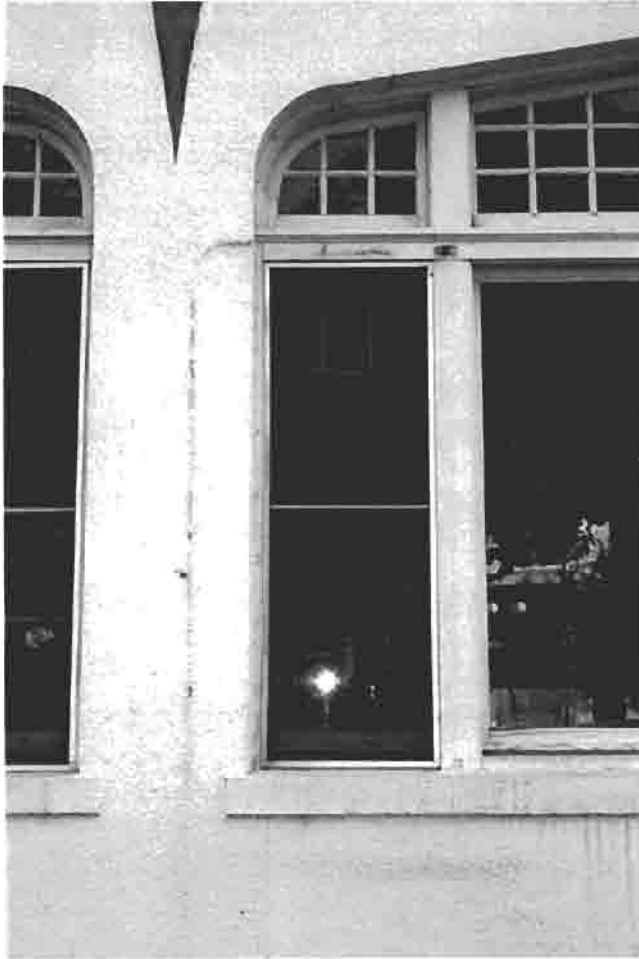
1C-27: West Elevation. Note the ghost of a conduit on the stucco. 11/2003
