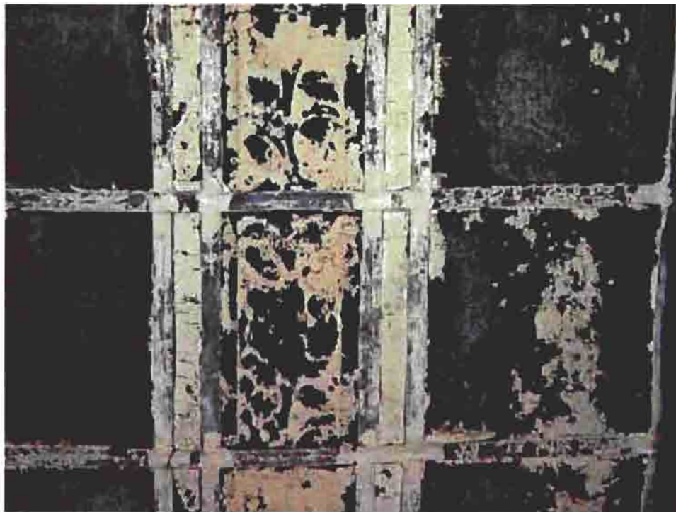
DETAIL OF PAINTED FINISH LOSS
