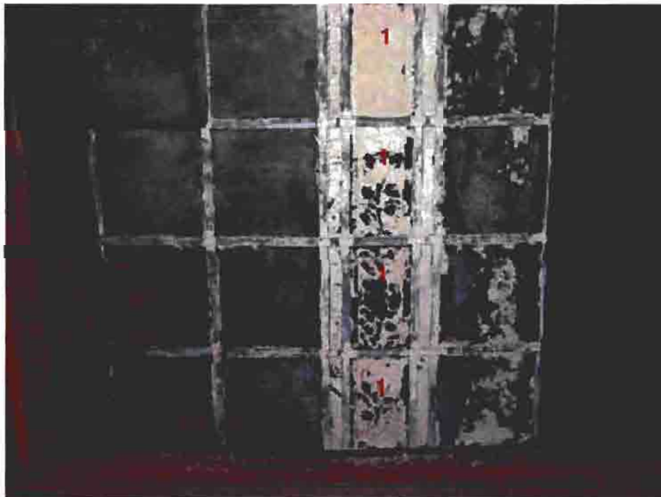
SOME TYPICAL CONDITION PROBLEMS: LOSS OF PAINTED FINISH (1), LOOSE CAME (2); CORROSION OF CAMES (TYPICAL).
