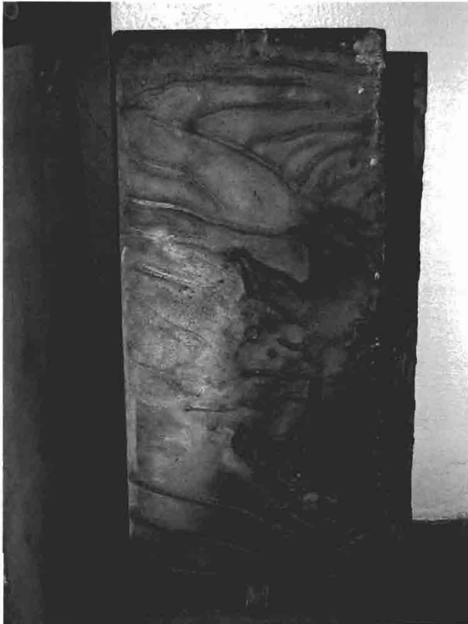
1C-89: Room 109, Women's Pack Room, Marble Panel. Deterioration due to exposure to spring water and steam. 11/2003
