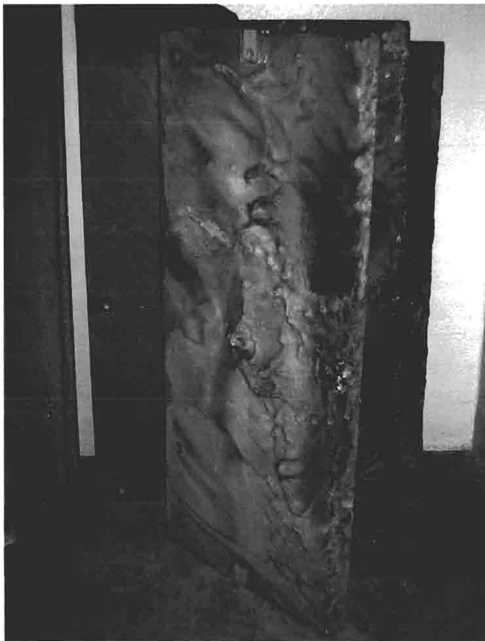
1C-88: Room 109, Women's Pack Room: Marble panel found stored in room 109. Deterioration due to exposure to spring water and steam. 11/2003
