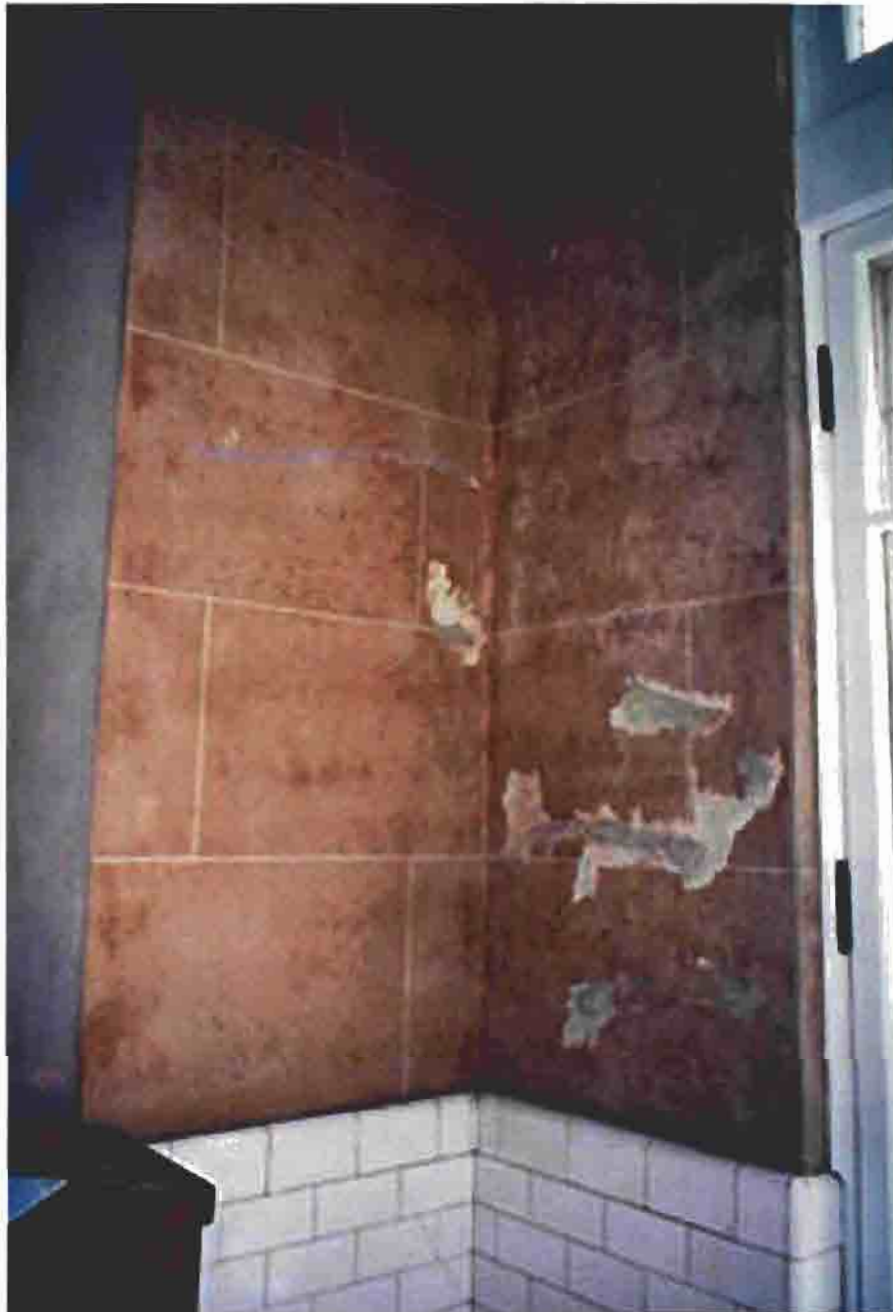
PLASTER/DECORATIVE PAINT JUNCTION: EAST & SOUTH WALLS AT SUN PORCH, LOCATION WHERE LOOSE PAINT WAS REMOVED TO REVEAL UNDERPAINTING.
