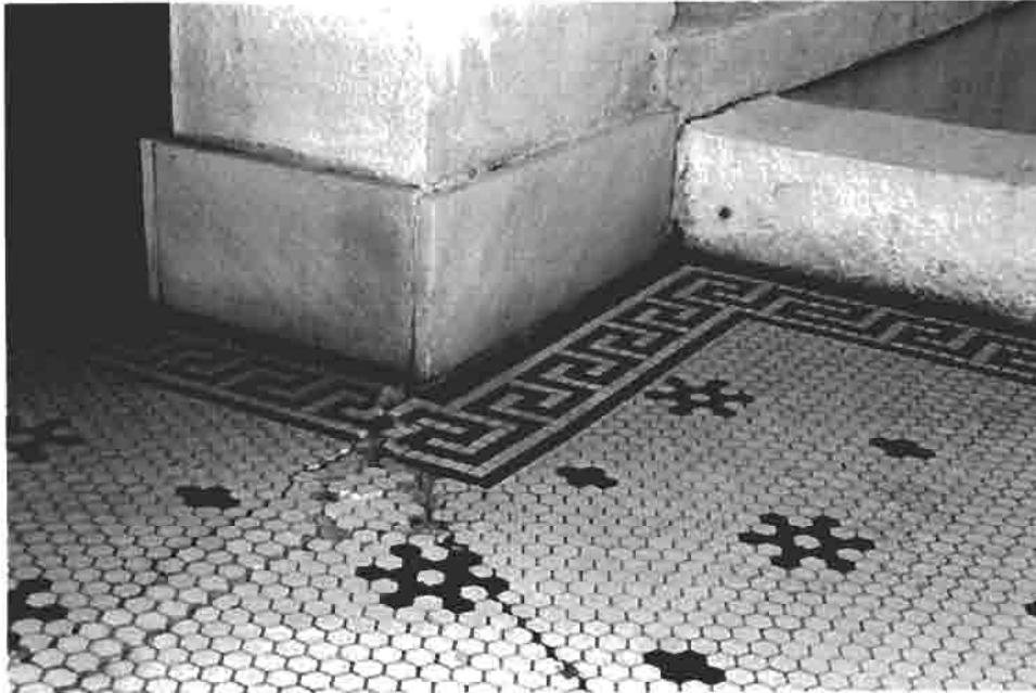
1C-11: West Site. Typical damage to the tile at the front entry alcove. 11/2003
