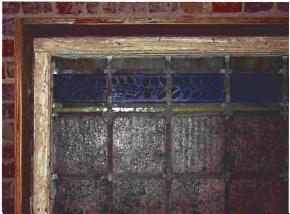
WOOD FRAMED PANEL: DETAIL OF RUN PANEL FROM THE OUTER EDGE; OPALESCENT, PAINTED BLUE, GREEN, & OBSCURED GLASS.
