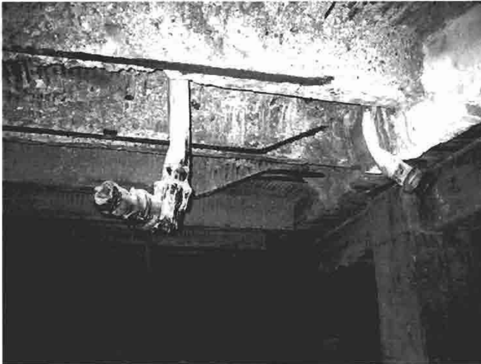
1C-56: Crawl Space: Southeast view from Fuel Room 01: Note: Exposed rebar & substantial loss of material at the south end of the third beam. 11/2003
