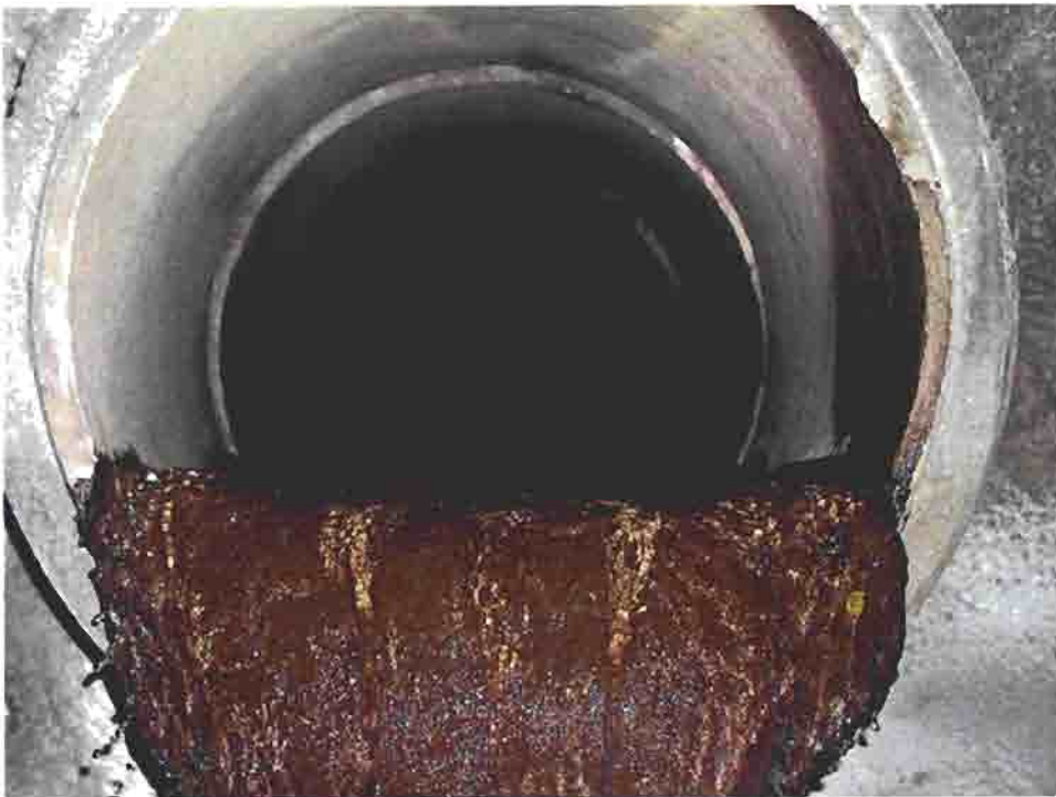
CA-13: The Creek Arch. The lower one-third to two-thirds of the pipe's diameter has been blocked by hot springs mineral deposits which can build up quite rapidly.
