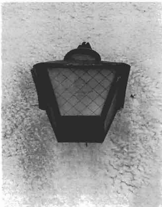
1C-29: West Elevation. Note oxidation in the metal of the light adjacent to the front entry. 11/2003
