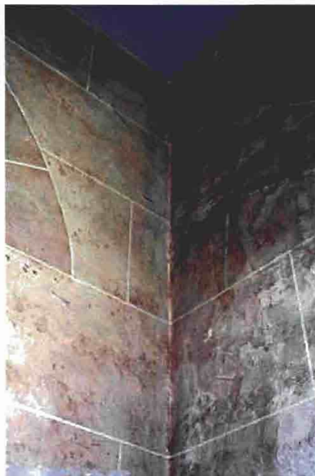
PLASTER: DISCOLORATION OF RIGHT HAND WALL, WITH POWDERED PLASTER, EVIDENTLY MOISTURE RELATED.
