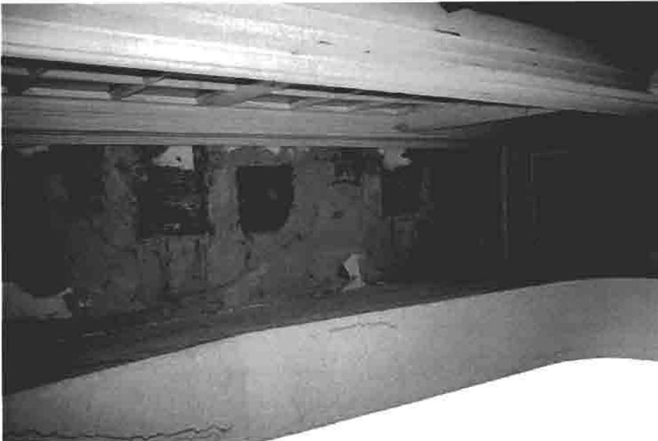
1C-28: West Elevation. The ceiling of the alcove has lost most of its plaster. Comprehensive restoration is required. 11/2003
