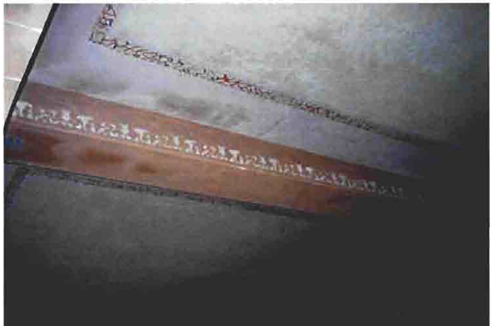
DECORATIVE PAINT: MOISTURE STAINING OF DECORATIVE PAINT AT PANEL EDGE & UNDERSIDE OF BEAM.
