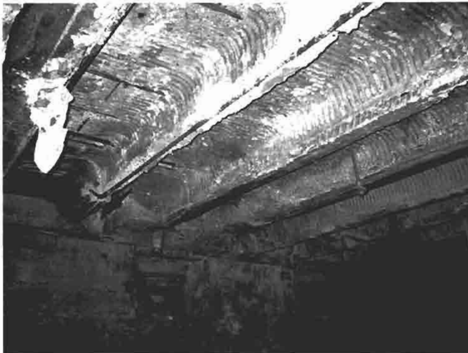
1C-54: Crawl Space: North view: from Fuel Room 01: Note: Exposed underside of the first floor structure & exposed rebar. 11/2003
