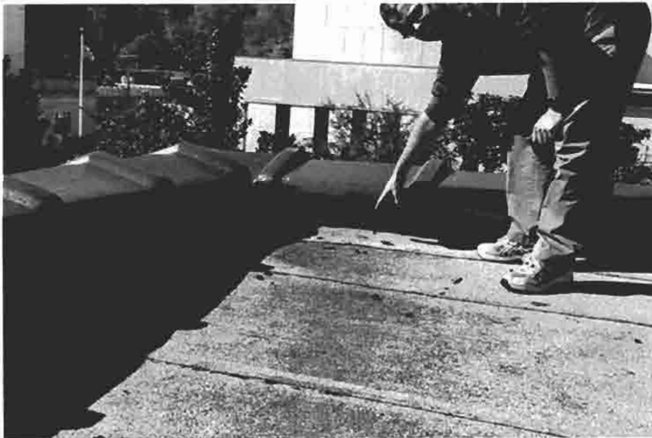
IC-38: Roof. Roofing, flashing (pointed out), and vitrified clay parapet coping tile. 11/2003
