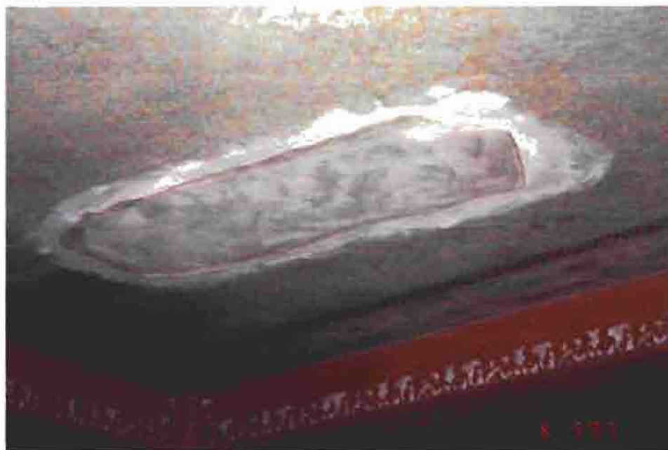
PLASTER: PATCH IN CEILING SECTION C, CENTER OF LOBBY. ALSO, NOTE MOISTURE DISCOLORATION SPOTS.
