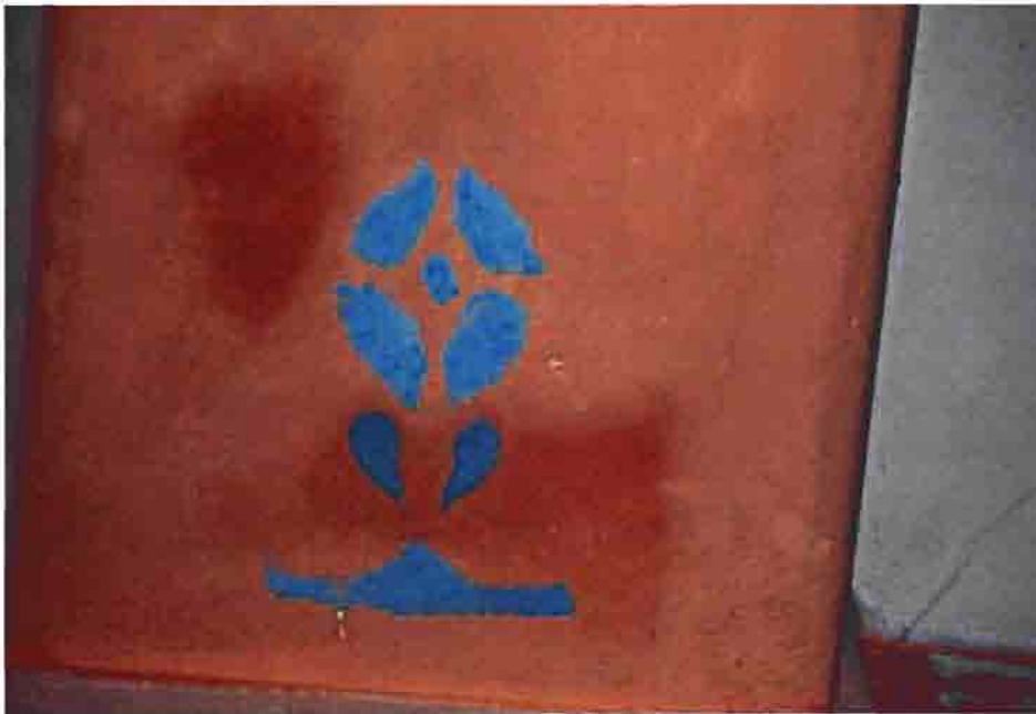
DECORATIVE STENCIL APPEARS ON BOTTOM OF BEAM AT EACH END OF BEAM. NOTE: DARKENED AREAS ARE DUE TO WATER DAMAGE.
