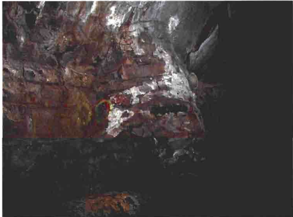
CA-11: The Creek Arch. Note the abundance of faded and overlaid markings on the wall beside this part manhole. These markings make location of problems difficult.
