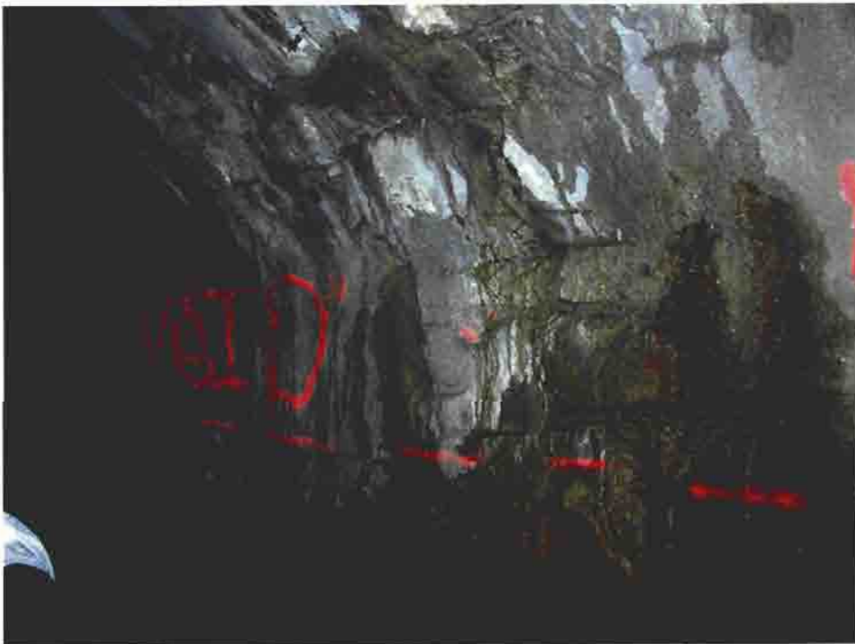
CA-9: The Creek Arch. The "void" designation was the only one found, but it did coincide with areas of mortar loss deep within the joints.
