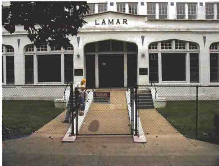
Figure CLA-5: Original entry's rigidly symmetrical ramps emphasize the building's symmetry. The lawn on the left is planned to be sloped toward the new accessible ramp. (Shapins Associates, 2003)
