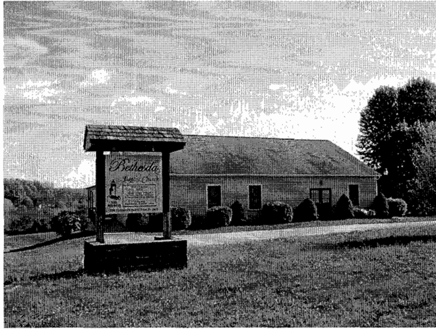
Figure 5.12 The new Bethesda Baptist Church, Harmonyville Road, St. Peter's.
