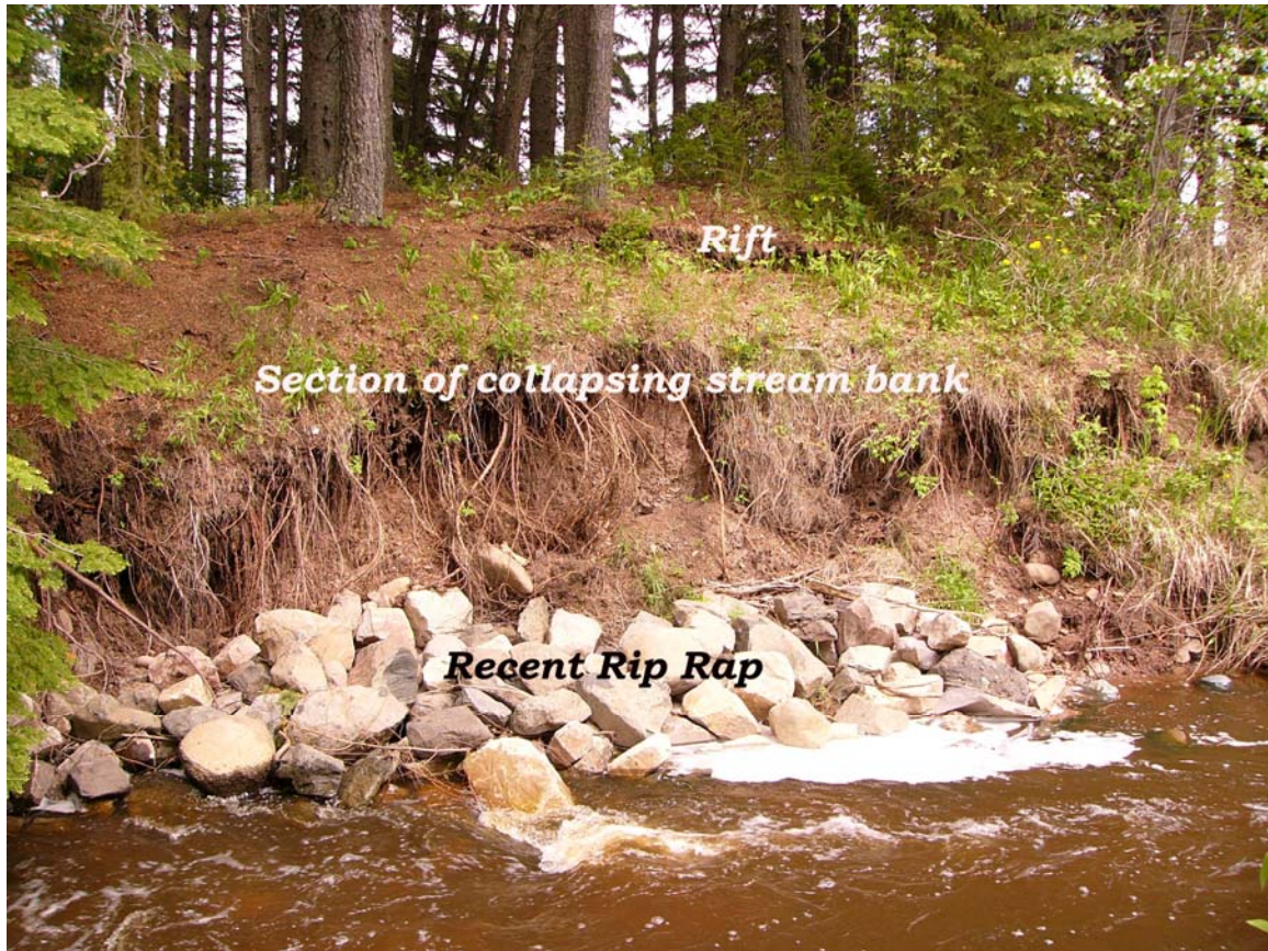
Figure 12. This east view shows a collapsing section of stream bank, recently riprapped, just below the old ford on the east side of Grand Portage Creek (Digital photo by the author, 6 June 2005).
