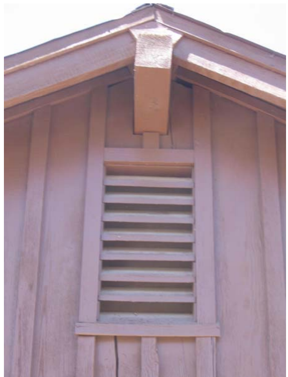
Vertical Board and Batten Siding 0090 - 113
