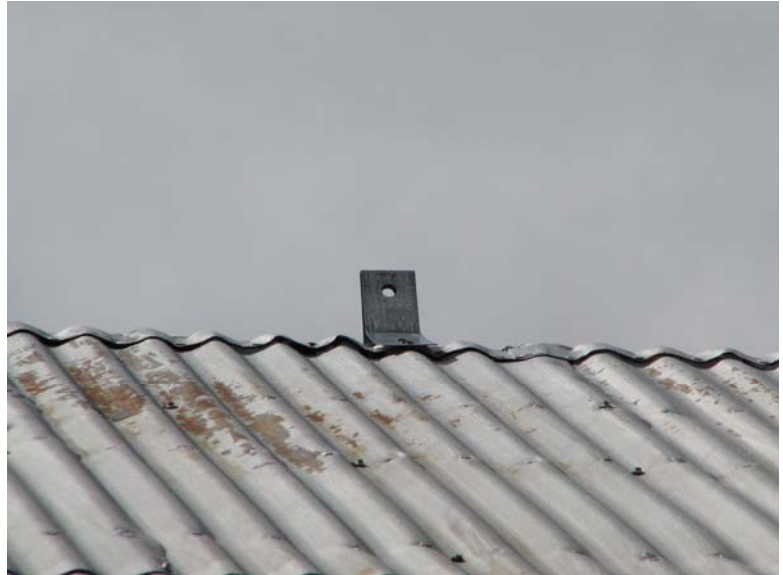
Steel Brackets at Ridge 0078-105
