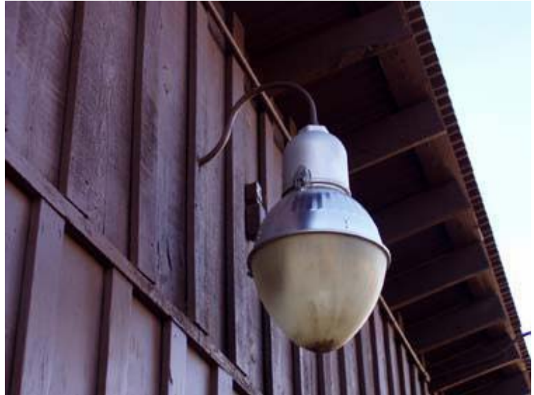
Mercury Vapor Fixture 0074-139
