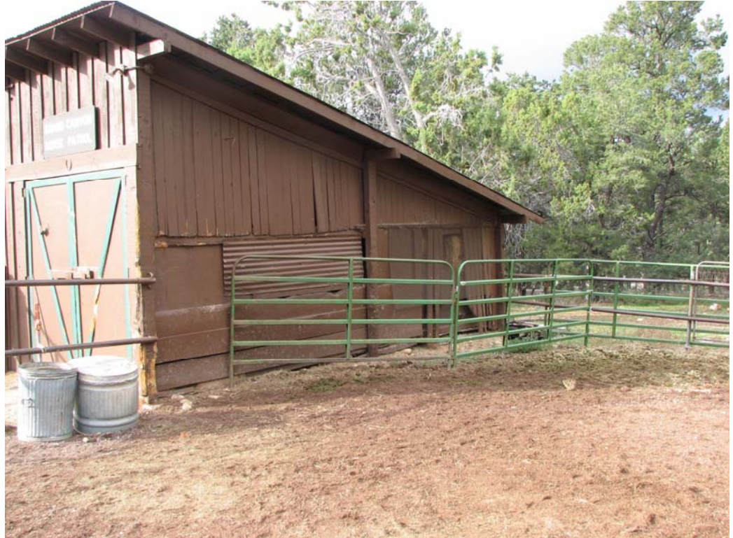
Mixed Rough Sawn Siding on North Elevation 0074-109
