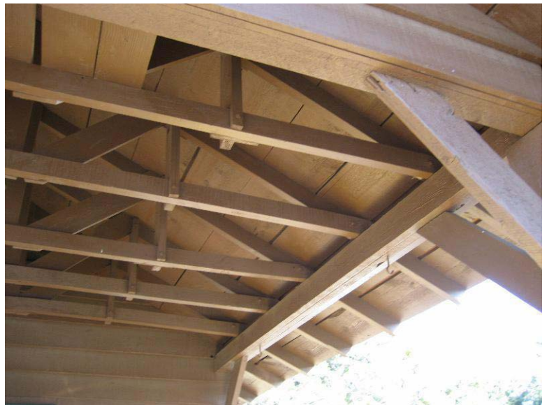
Exterior Girder Supporting Trusses 0079-124
