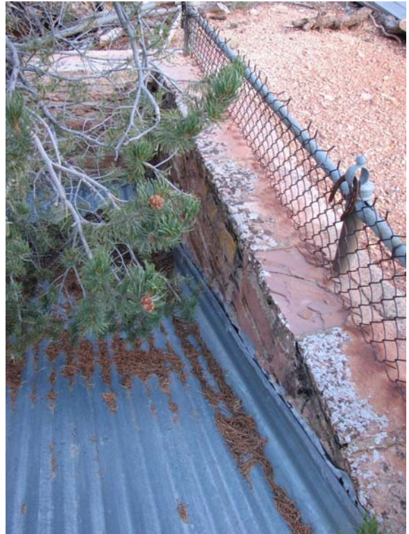
Roofing Attached to Stone Wall 0094 - 107
