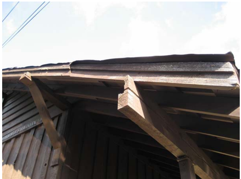
Porch Framing. Deteriorated Edge Beam and Rafters 0078-159
