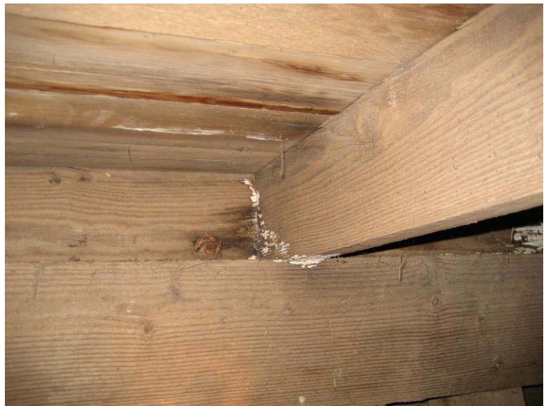
Rotting Porch Joist 0090 - 229
