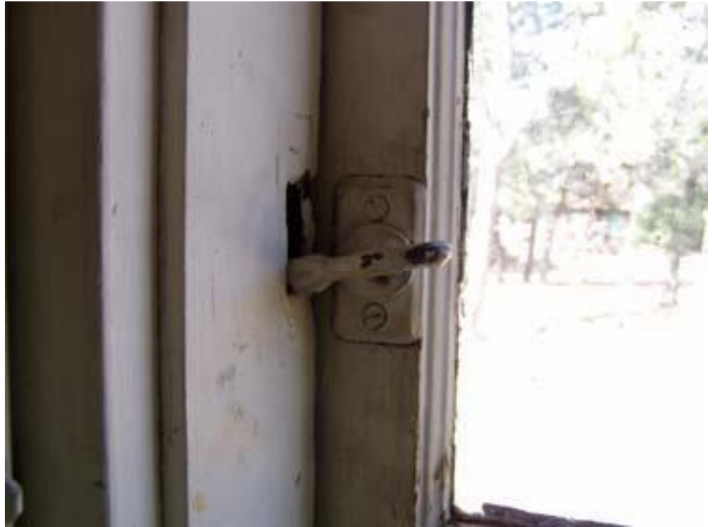
North Window Thumb Latch – (8) 0069-207
