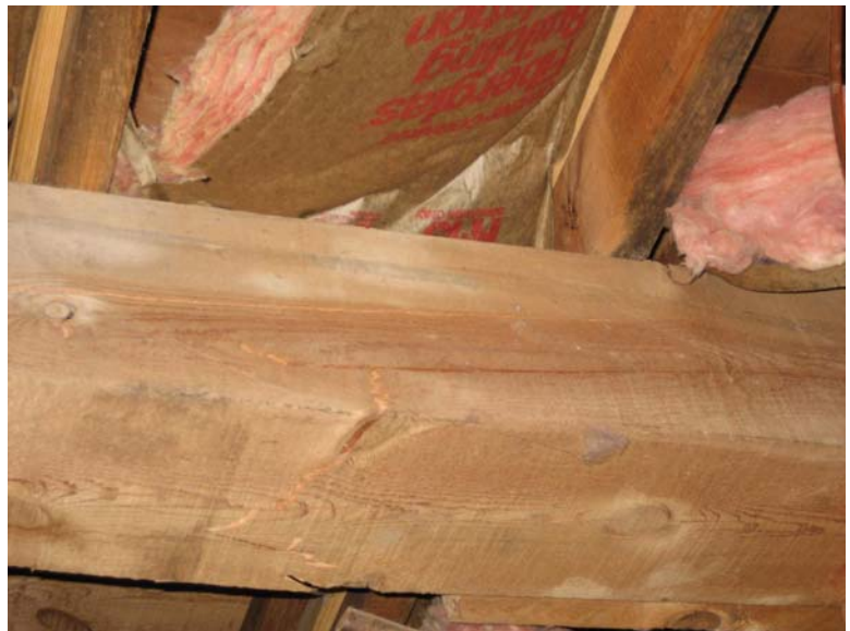
Failed First Floor Girder at Basement 0078-205
