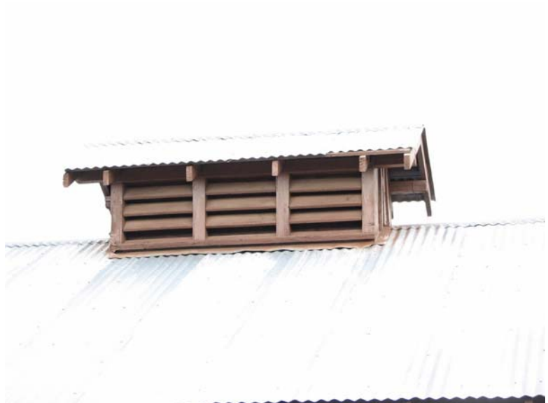
Wood Framed Louver Sections on Exterior of Cupola 0075-108
