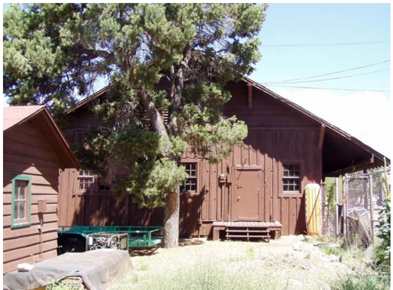
Board and Batten Siding at South Elevation 0078-115
