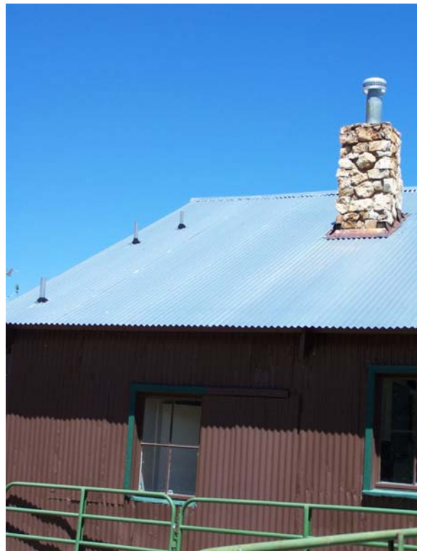
Corrugated, Galvanized Steel Sheet Metal Roofing 0080-106
