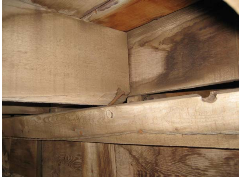
Failing Ledger at West Porch 0078-144
