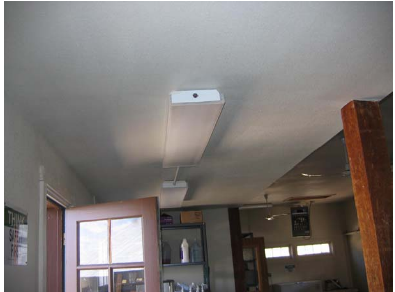
Surface-mounted Lensed Fluorescent Fixture 0090 - 247
