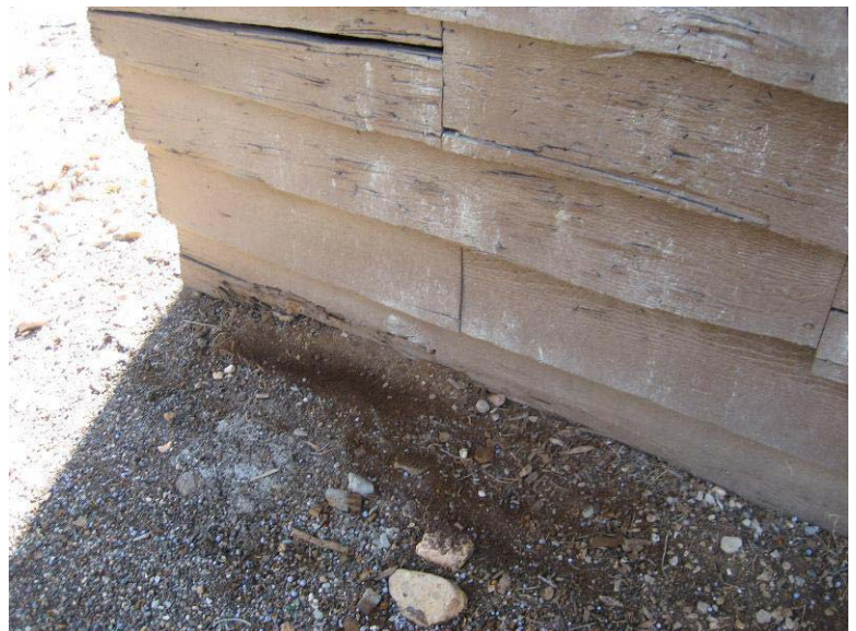
Deteriorated Wall Sheathing at East Wall 0099 - 122
