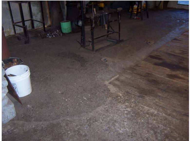
Asphalt Overlaying Conc. Floor; 2x12 Plank Floor 0075-205
