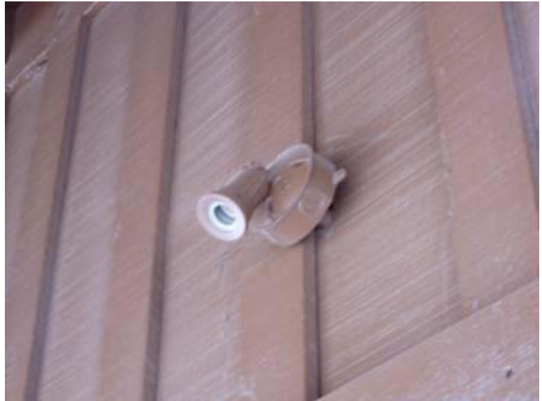
Floodlight on West Façade - No Lamp 0078-154
