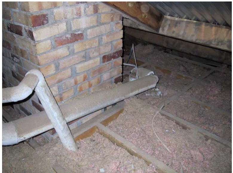
Abandoned Steam Piping in Attic 0080-237
