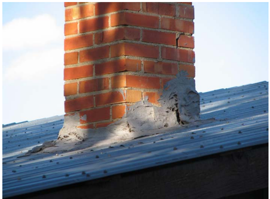
Sheet Metal Roof & Flashing at Chimney 0074-106
