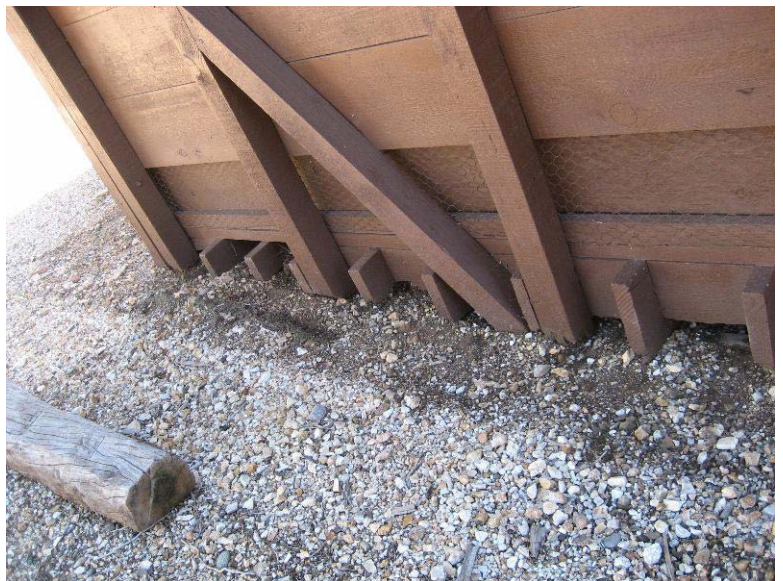
Southeast Corner: Framing Rotted by Soil Contact 0088-121
