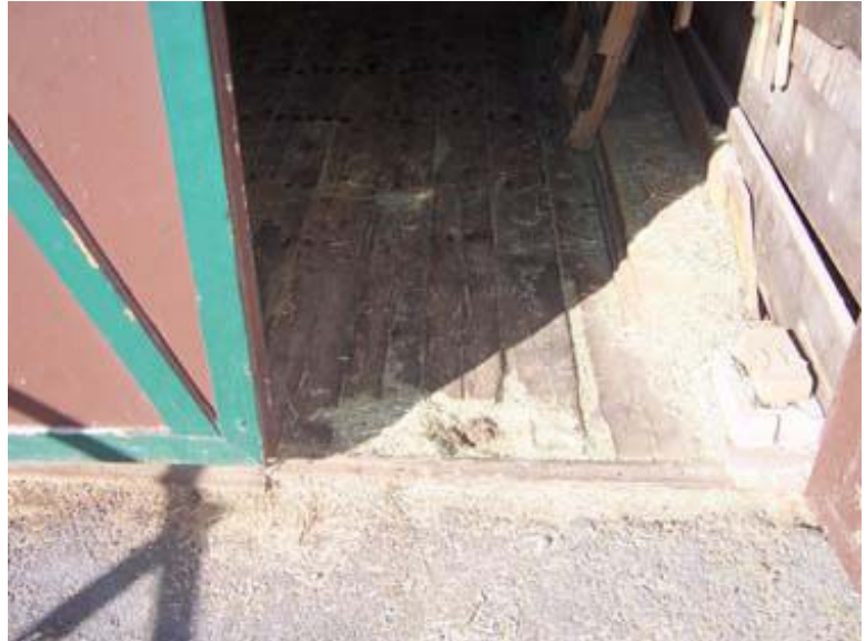
Damaged Wood Flooring at Threshold 0074-127
