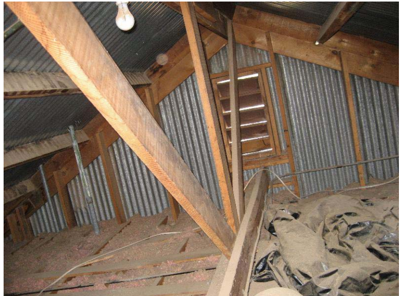
Transverse Truss and Ceiling at West Bay 0080-221
