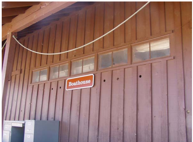
Vertical Board and Batten Siding 0078-113
