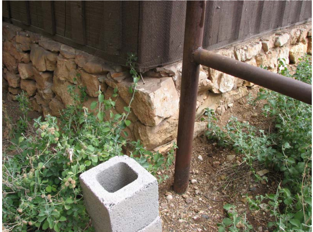
Stone Foundation at Southwest Corner 0074-113
