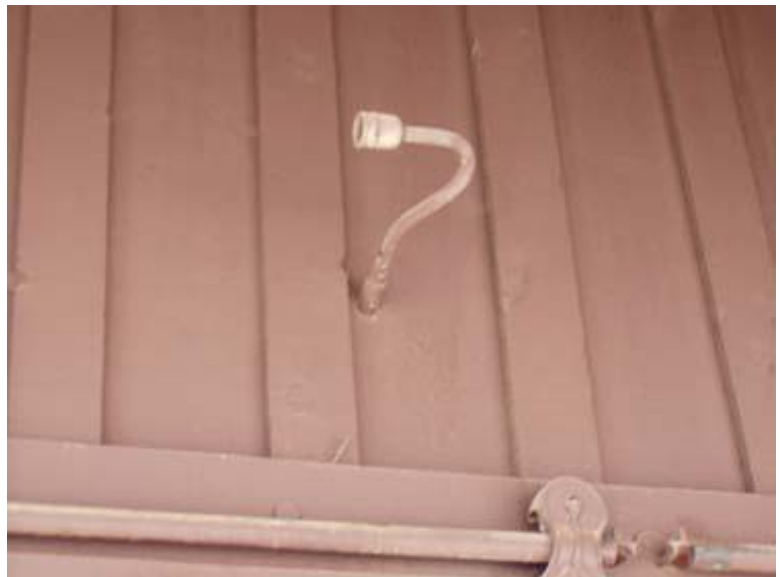
Gooseneck Arm at Loading Dock 0078-155
