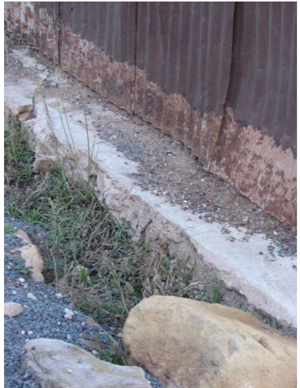
Siding Extends to the Top of the Concrete Ledge 0080-110
