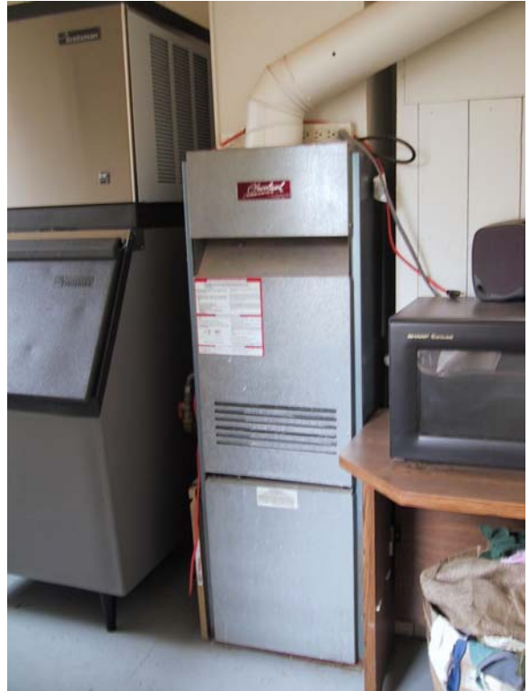
Propane Forced Air Furnace 0080-232
