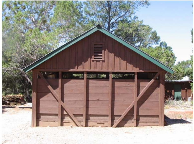
Cross-Braced 4x4s at the Tripled-Up 4x4 Corners 0088-112
