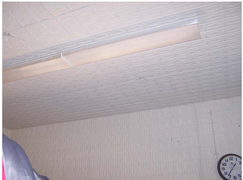
Stamped Tin at Walls and Ceiling 0080-207
