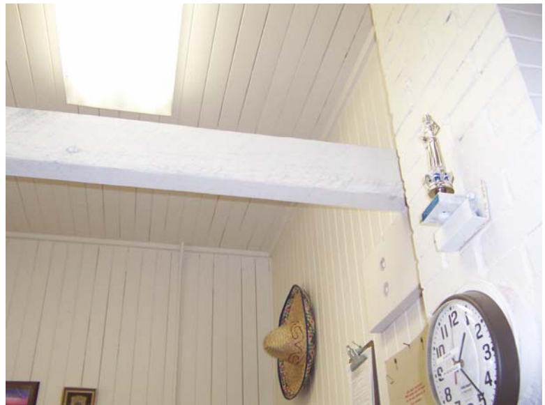
Tongue and Groove Walls and Ceiling 0090 - 207
