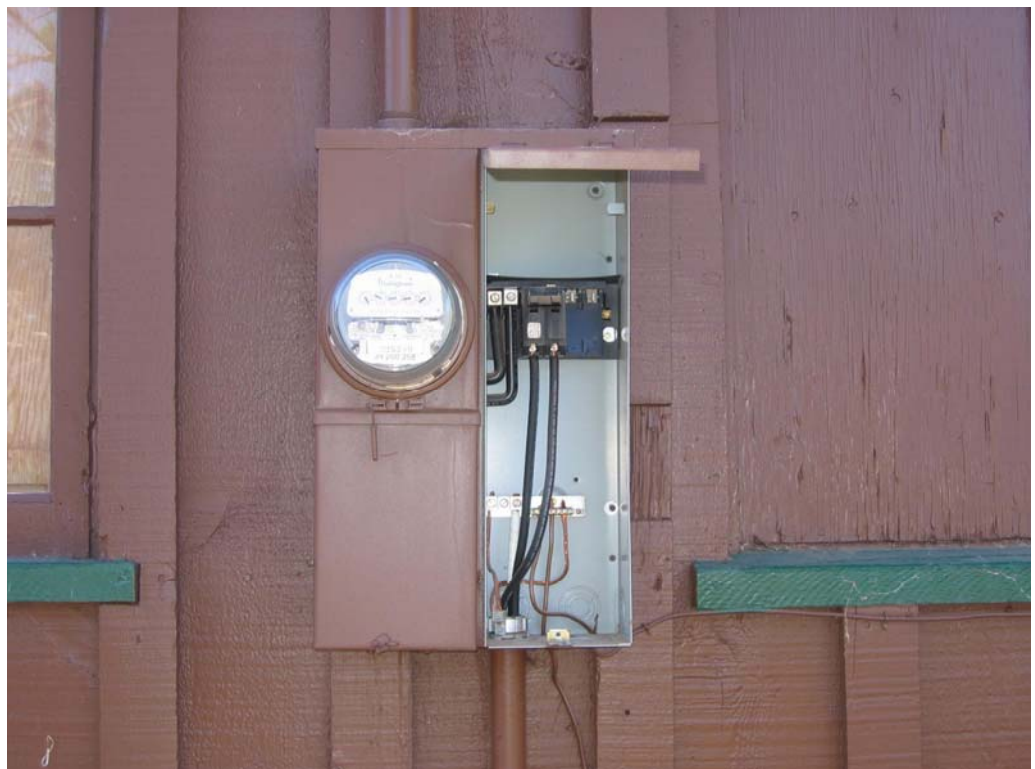
Electrical Service Disconnect 0069-133
