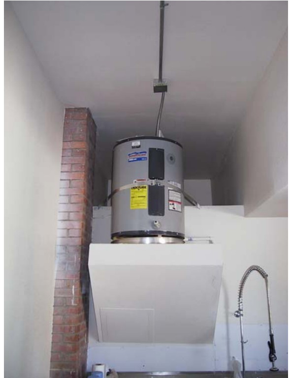
Electric Water Heater 0090 - 230
