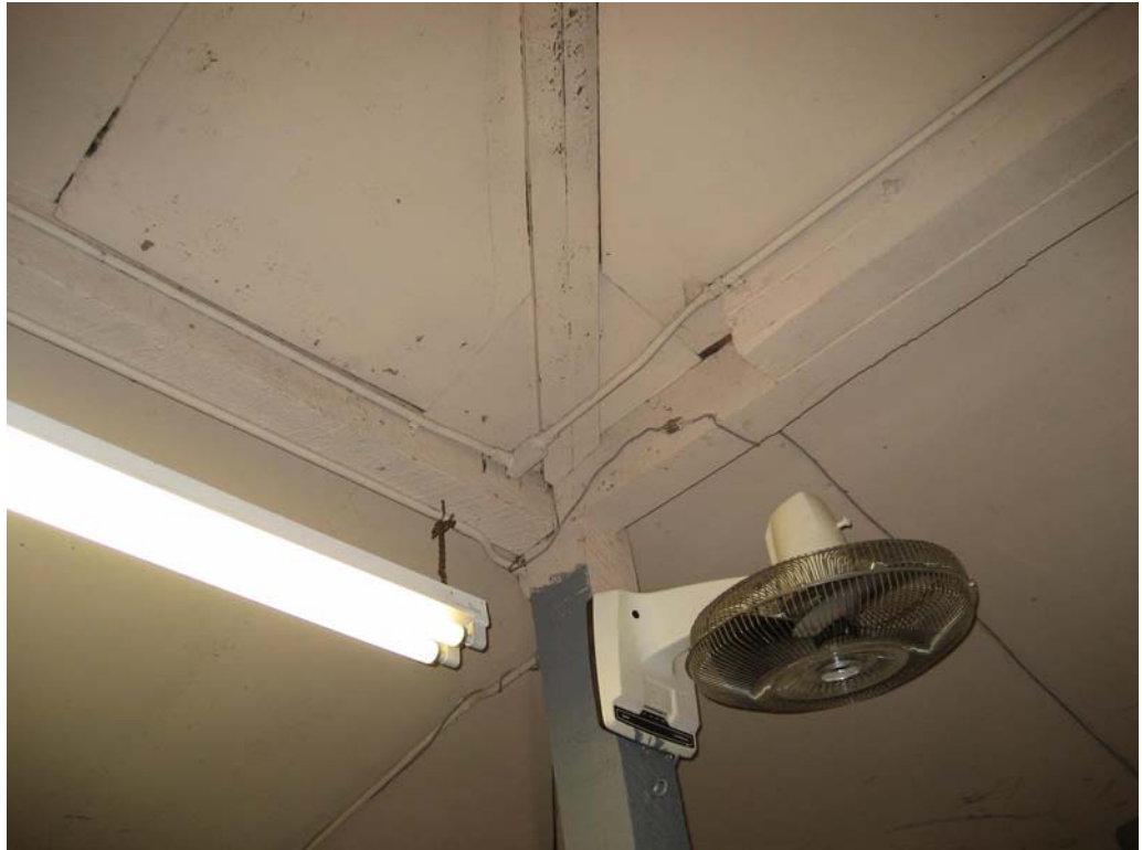
Typical Interior Ridge & Hip Beams 0069-201
