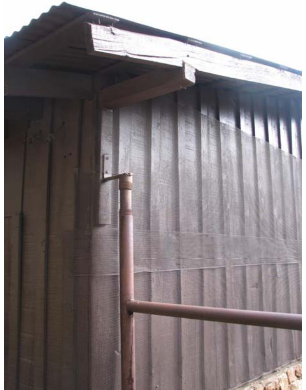
Bracket in Southwest Corner showing Missing Brace 0074-107
