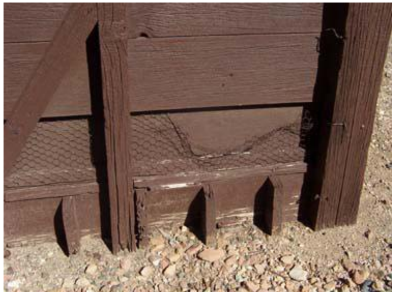
Plywood Over Chicken Wire at the Base of the Wall 0088-113
