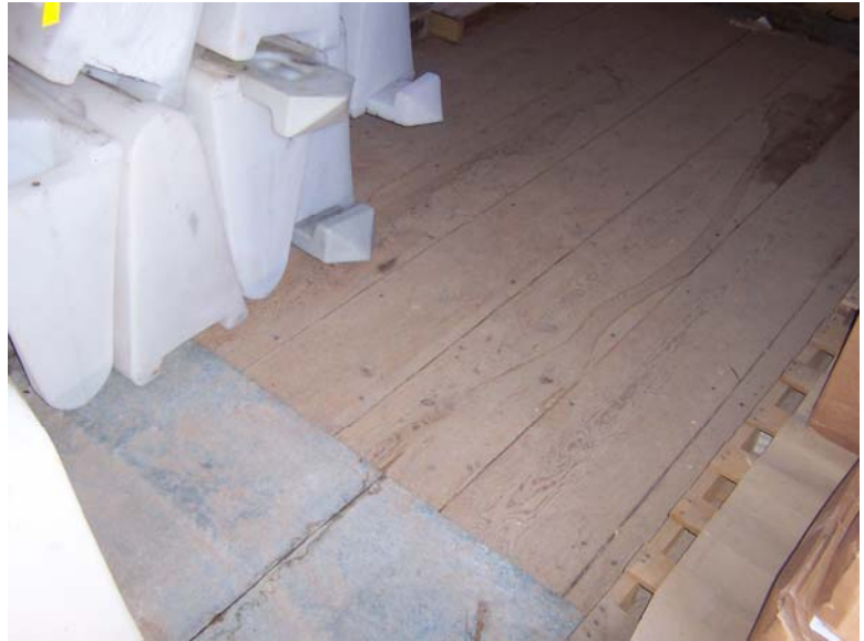
2x12 Flooring with Sheet Metal Overlay 0088-202
