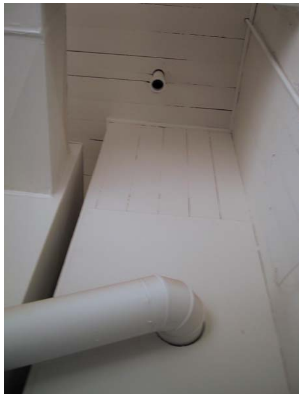
Furnace Flue 0080-233
