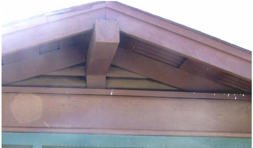
6x6 Beam End Cantilevering 0094 - 109
