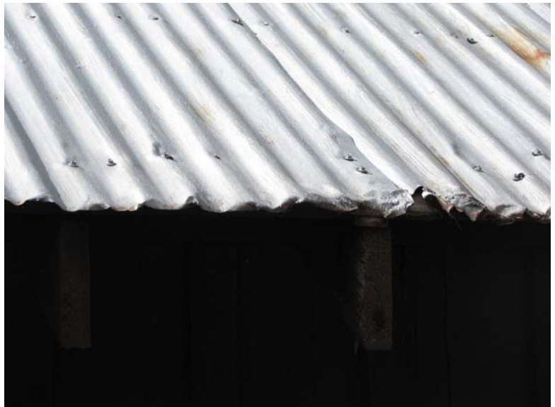
Damaged Edge of Sheet Metal Roofing 0078-108
