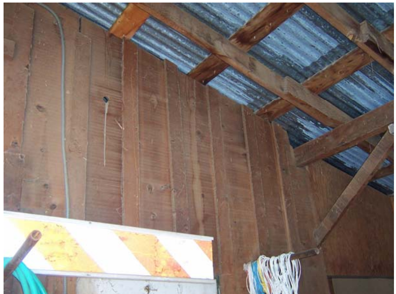
Planks with Battens 0074-212
