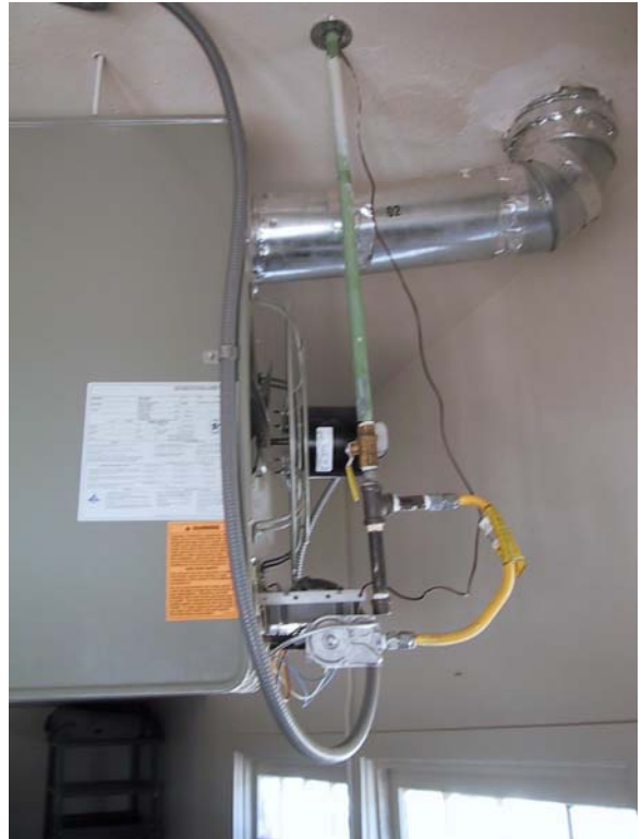
Unit Heater Flue and Gas Connections
