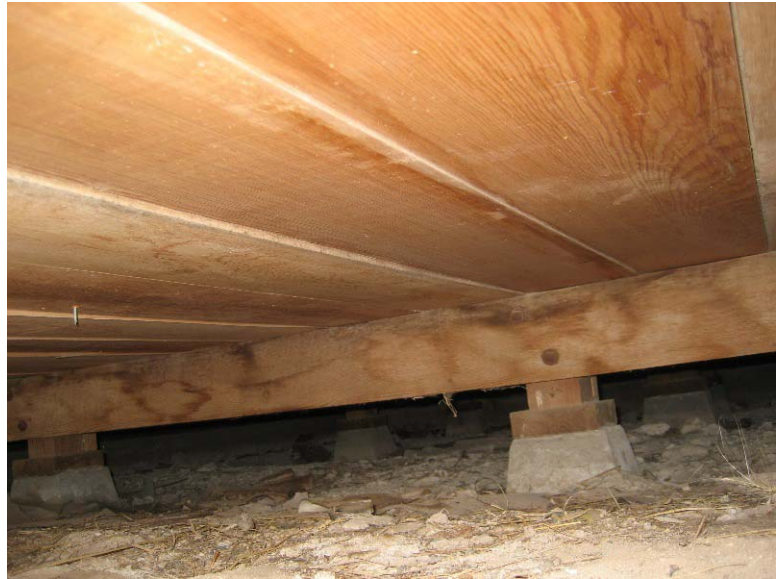
Typical Interior Floor Girders and Foundations 0094 - 137
