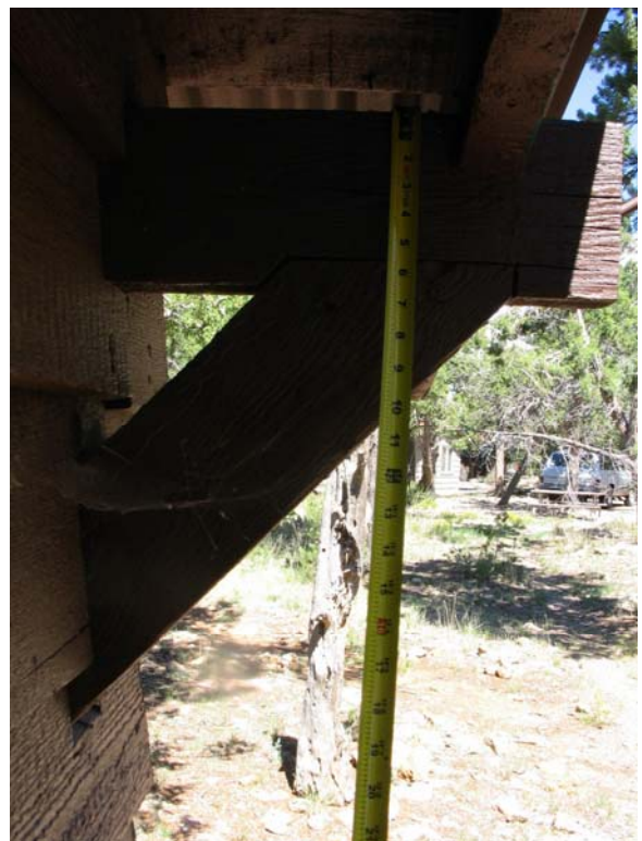
3x6 Beam Extensions and Braces 0099 - 106
