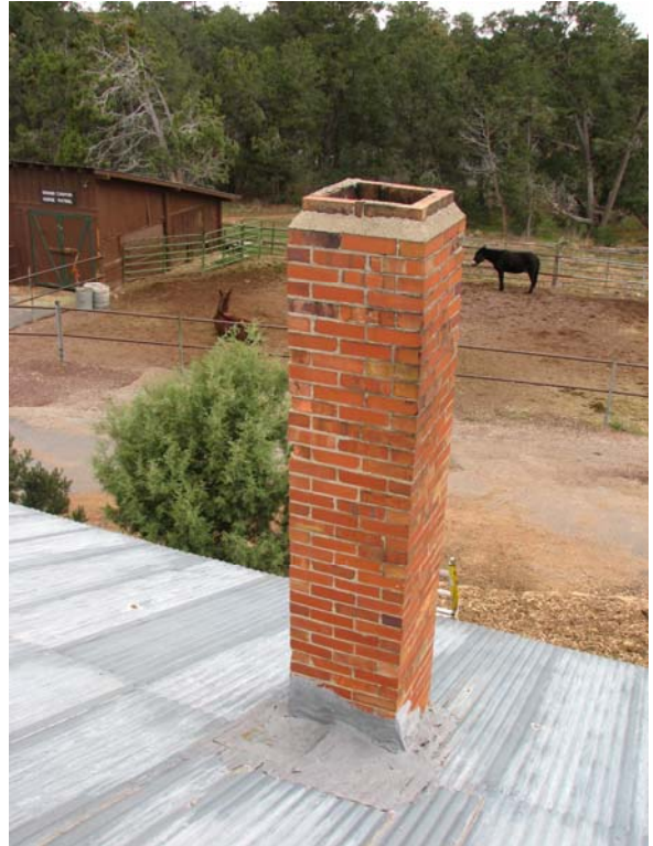
24"x24" Chimney with 12"x12" Un-lined Flue 0075-113
