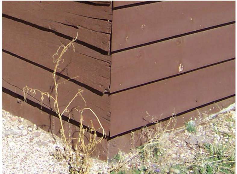
Split Siding at Mitered Corners 0079-111
