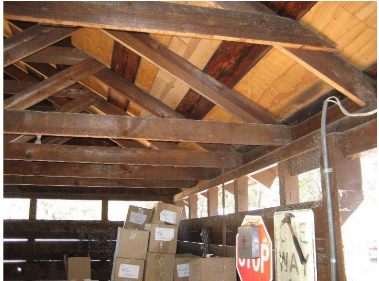
Typical Truss Bearing at Exterior Wall 0088-204
