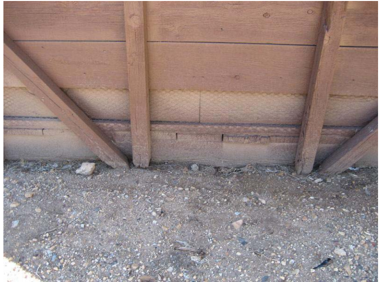
East Wall: Framing Rotted by Soil Contact 0088-122
