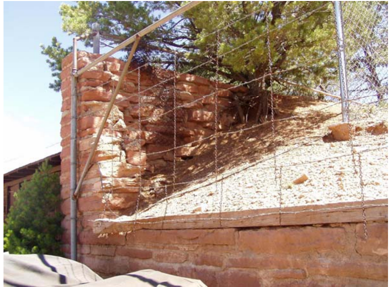
Random Ashlar, Red Sandstone Retaining Wall 0094 - 113
