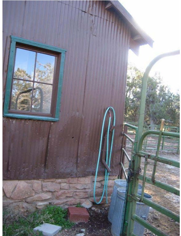
West Wall: Typical Perimeter Foundation 0080-226
