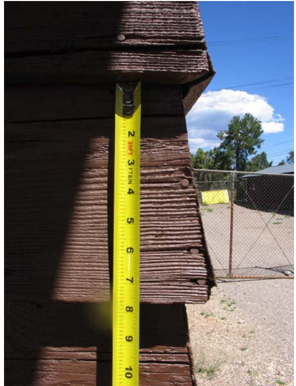
1x10 Lap Siding with Mitered Corners 0090 - 112
