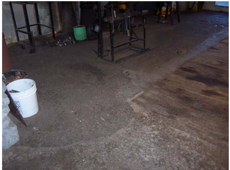
Asphalt Overlay at Concrete Slab Floor 0075-212
