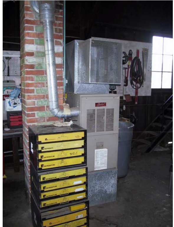
Propane Forced Air Furnace 0075-215
