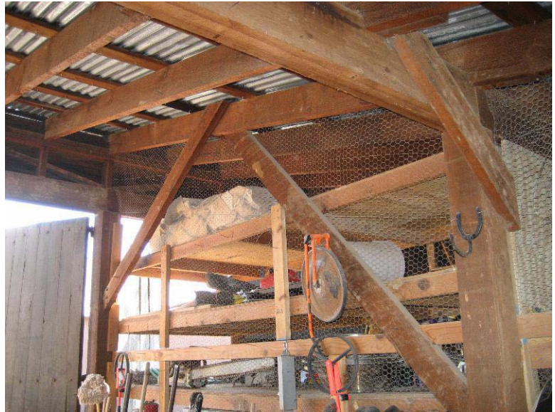
Bracing at Door Jamb Lines and Girder 0099 - 205
