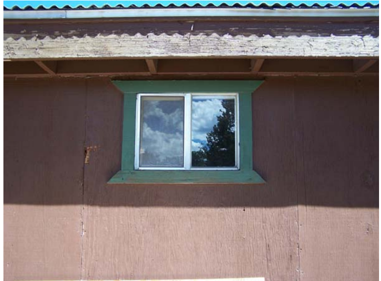
Plywood Siding on South Elevation 0087-109
