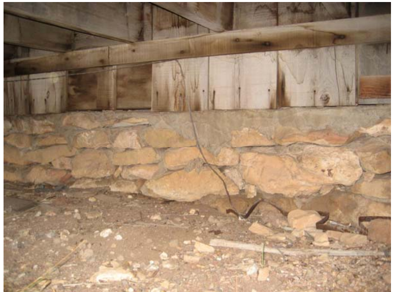
West Porch Ledger, Typical Perimeter Foundation 0078-143
