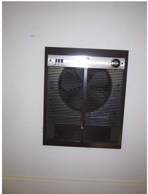
Restroom Ventilator
