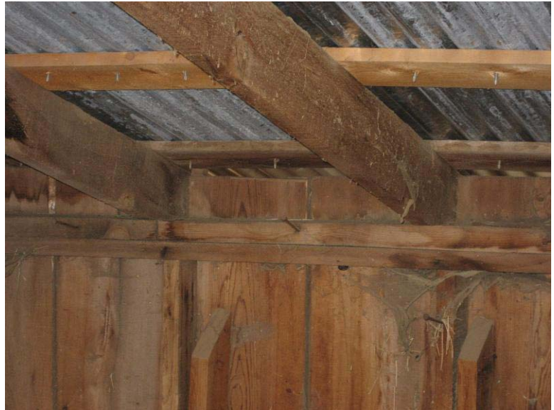
Typical Rafter Bearing on Wall Top Plate 0074-219
