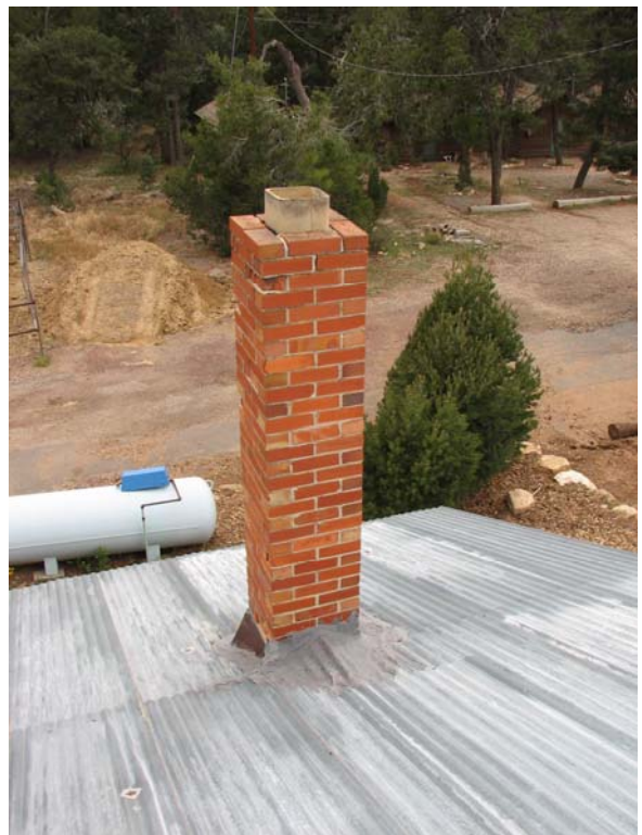
16"x16" Chimney with 8" Clay Flue Liner 0075-114
