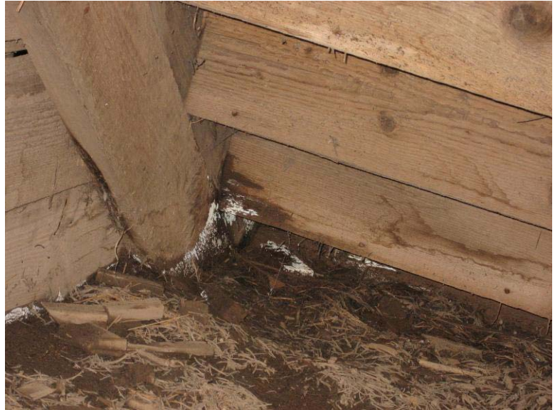
Rotting Stair Stringer at West End of Porch 0090 - 228
