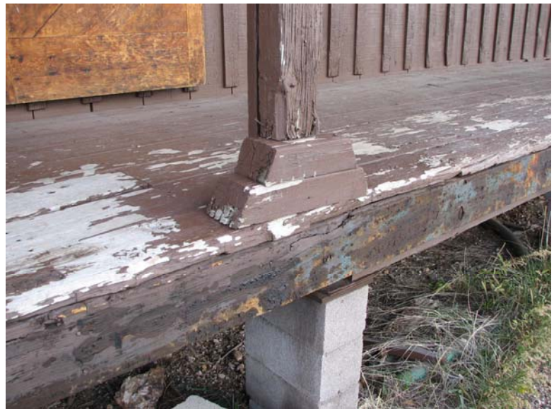
4x6 Posts Supporting Roof Overhead 0078-119
