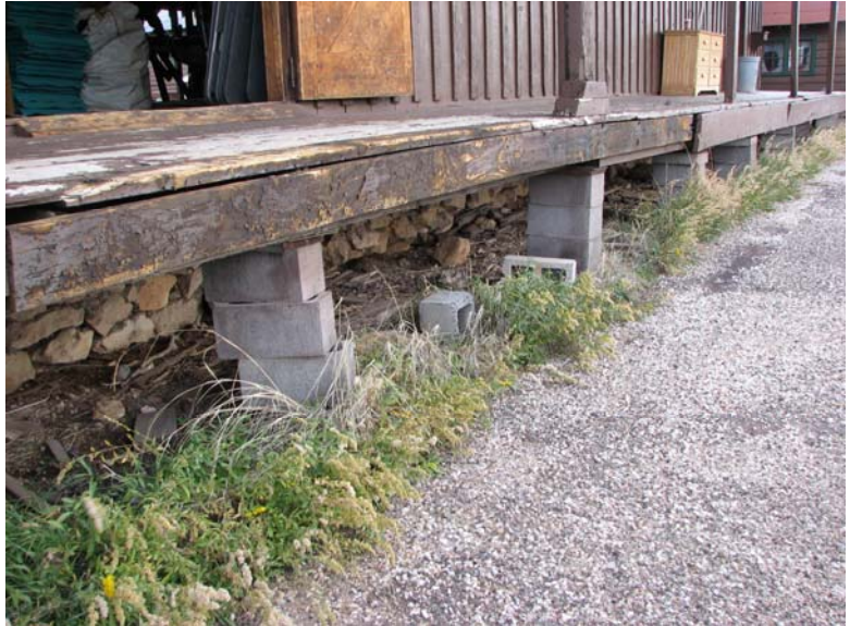
Porch Supported on Loosely Stacked 8x16" CMU 0078-118
