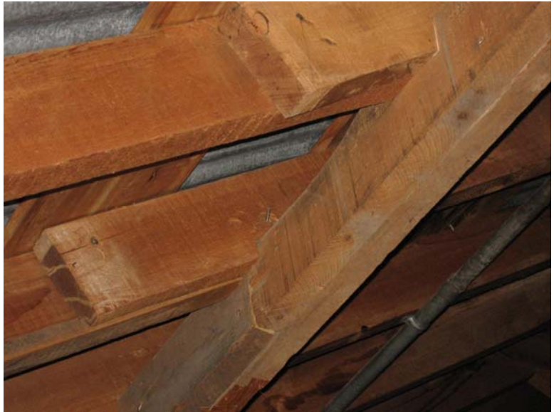
Rafter Bearing at Interior Girder Line 0078-258
