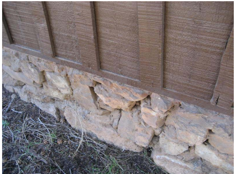
Typical Stone Perimeter Foundation 0074-130
