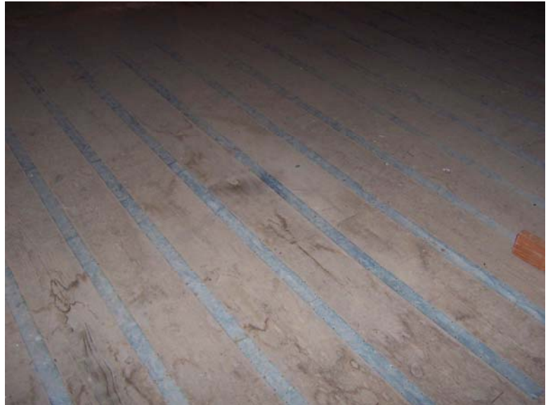
Plank Flooring with Metal Strips at Second Floor 0078-252
