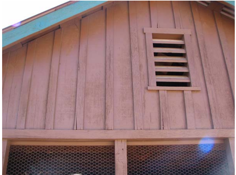
Vertical Board and Batten Gable Ends 0088-110
