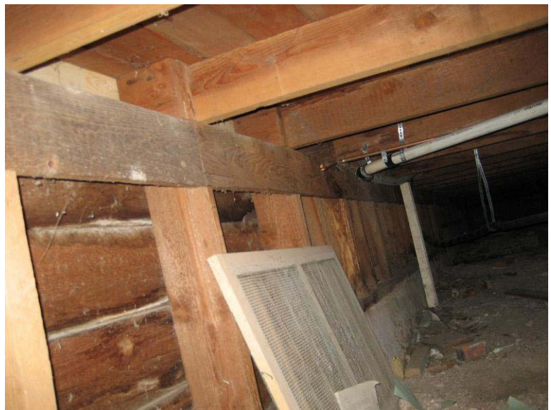
North Wall: Typical Framing Below First Floor 0090 - 221
