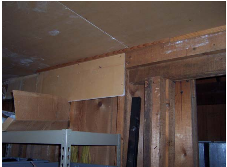
Unfinished Gypsum Board at Wall and Ceiling 0078-230
