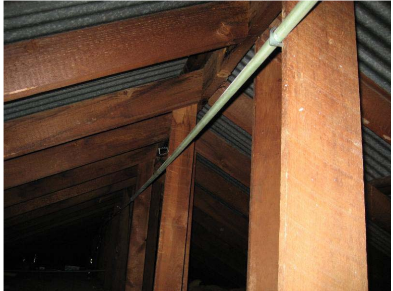
Typical Roof Framing at Ridge 0090 - 218
