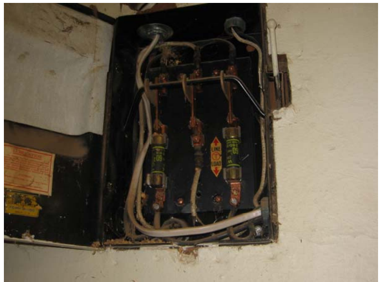
Electrical Service Disconnect 0074-224
