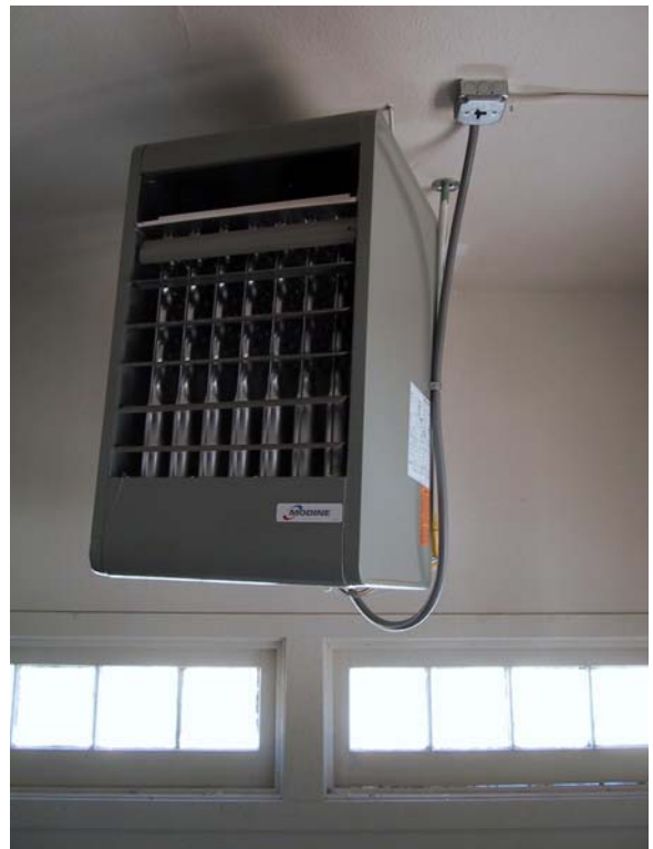
Forced Air Propane Unit Heater 0090 - 238
