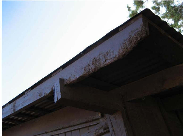
Livestock Damage to North Barge Rafter 0074-133
