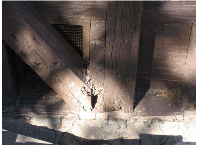
North wall: Brace and Post Rotted 0088-124
