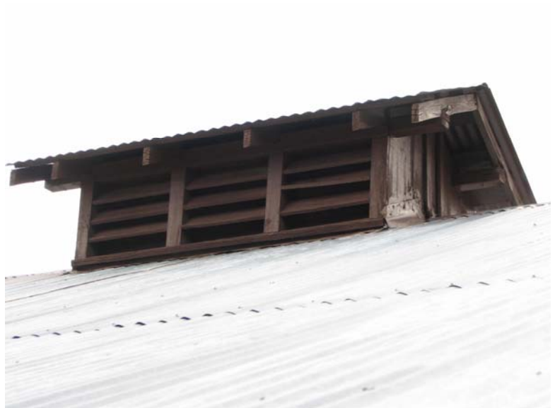
Louvered Cupola on Corrugated Sheet Metal Roofing 0075-106
