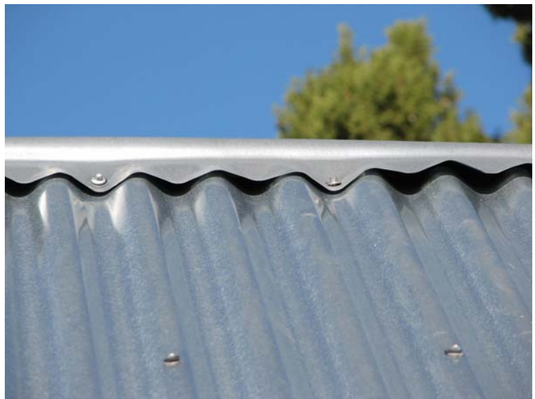
Round-Over Ridge Cap at the Ridge Line 0088-107
