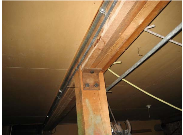
Interior Girder Supporting Second Floor Joists 0078-240
