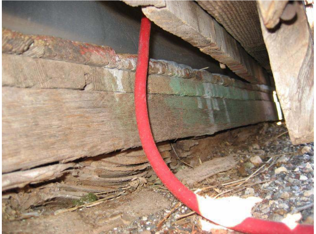
Deteriorated Rim Joist at South Wall
