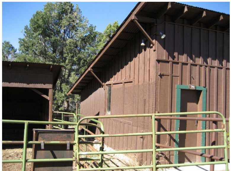
South Wall with Missing Kicker to Barge Rafter 0074-134
