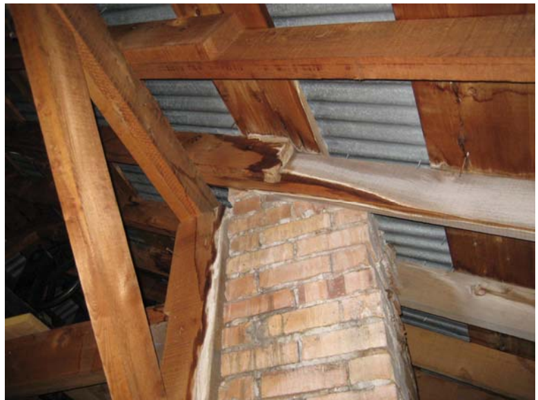
Water Damage Around North Chimney 0078-263
