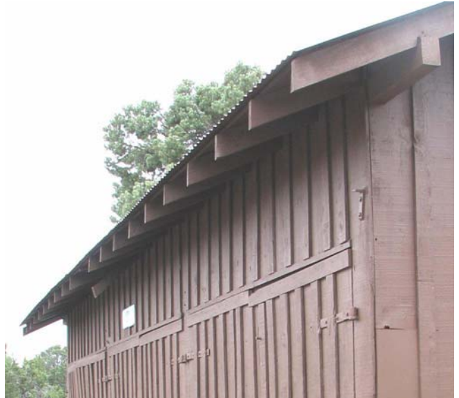
Exposed Rafter Tails on East Elevation 0075-109
