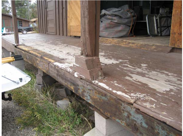
West Porch. Note Failing CMU Pier, Damaged Post 0078-142
