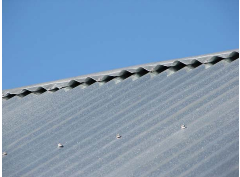
Corrugated, Galvanized Sheet Metal Roof 0088-106
