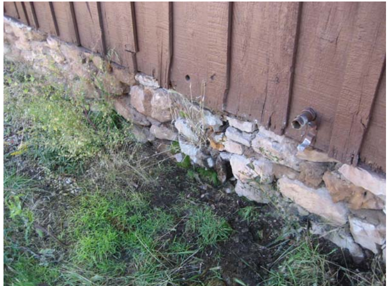
West Wall: Perimeter Foundation. Note Water Damage 0075-131
