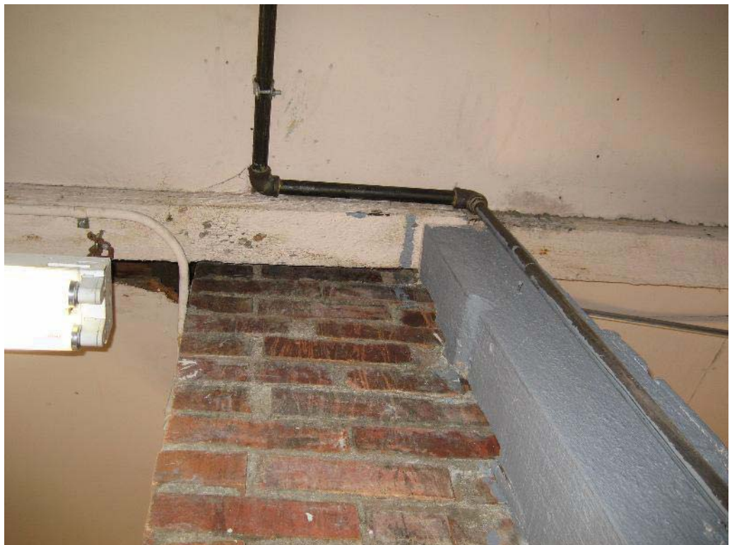
Deteriorated Wood Foundation Under East Side
