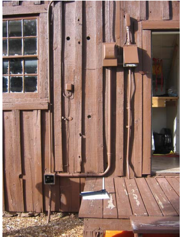
Exterior Panel and Service Disconnect 0078-146
