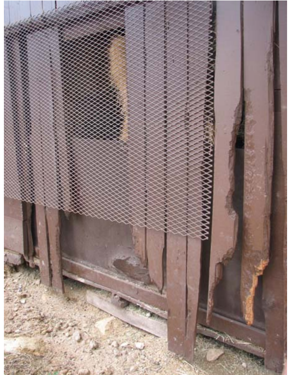
Board and Batten Siding with Hardware Cloth 0074-111
