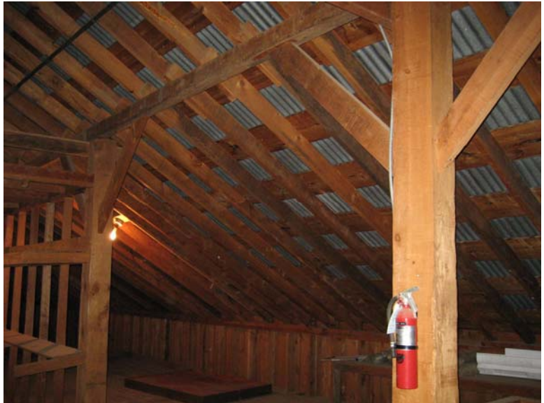
Interior Girder, Columns, Bracing 0078-260
