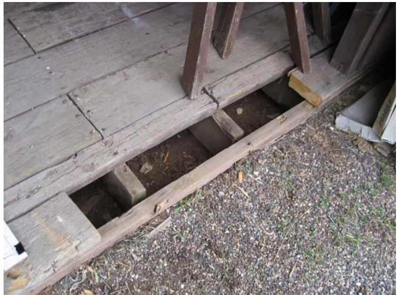
East Porch Missing Decking, Deteriorating Framing 0078-145
