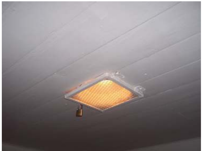
Incandescent Fixture with Grate 0087-225
