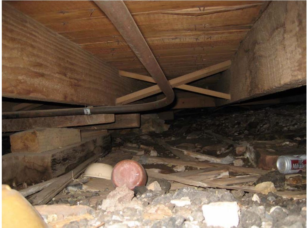
Deteriorated Wood Foundation Under East Side
