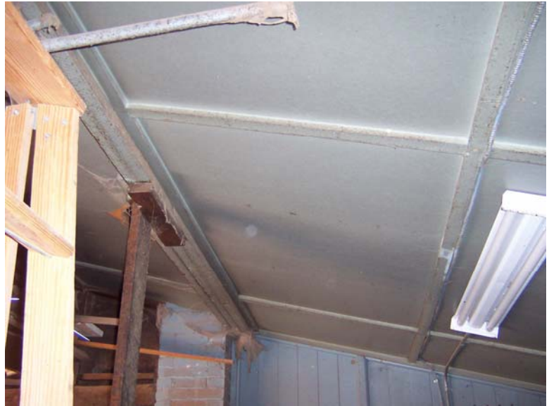
Fiberboard with Battens 0074-209
