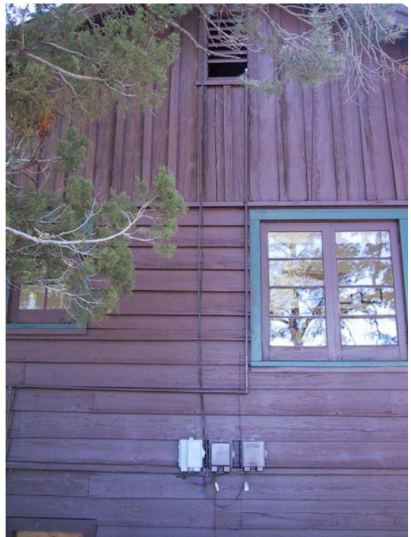
Propane Gas Piping Entering Building 0090 - 140
