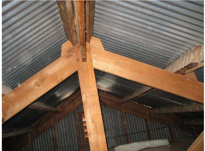
Typical Truss: at Ridge 0080-218
