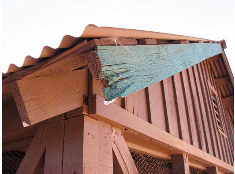
Exposed Rafter Tails at Roof Overhangs 0088-108
