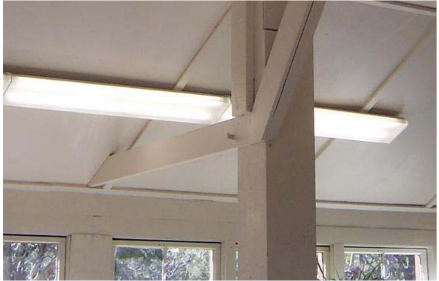
Surface-mounted Lensed Fixture
