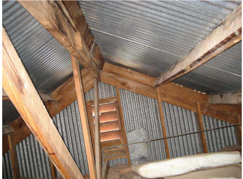
Transverse Truss at East Bay 0080-222
