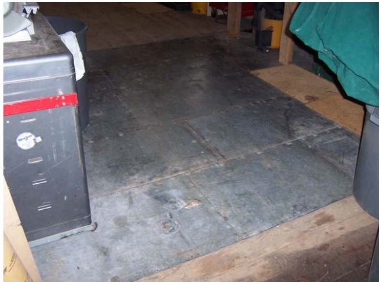
Wood Plank Flooring with Sheet Metal Overlay 0078-253
