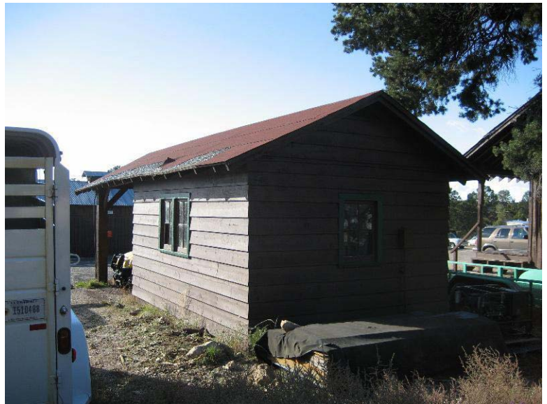
Southwest Elevation. Note Deflected Roof at Canopy 0079-126
