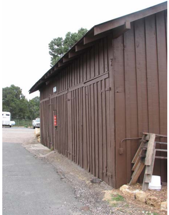
Vertical Board and Batten Siding 0075-111
