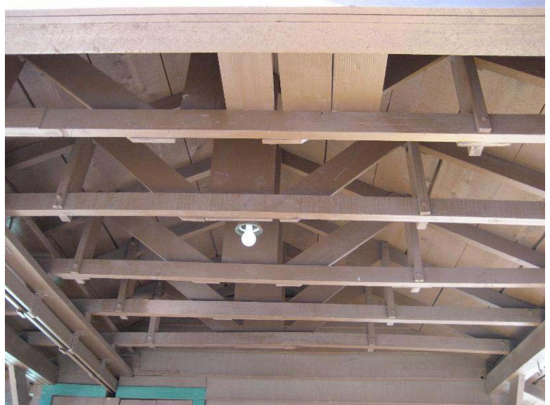
Typical Roof Truss 0079-123
