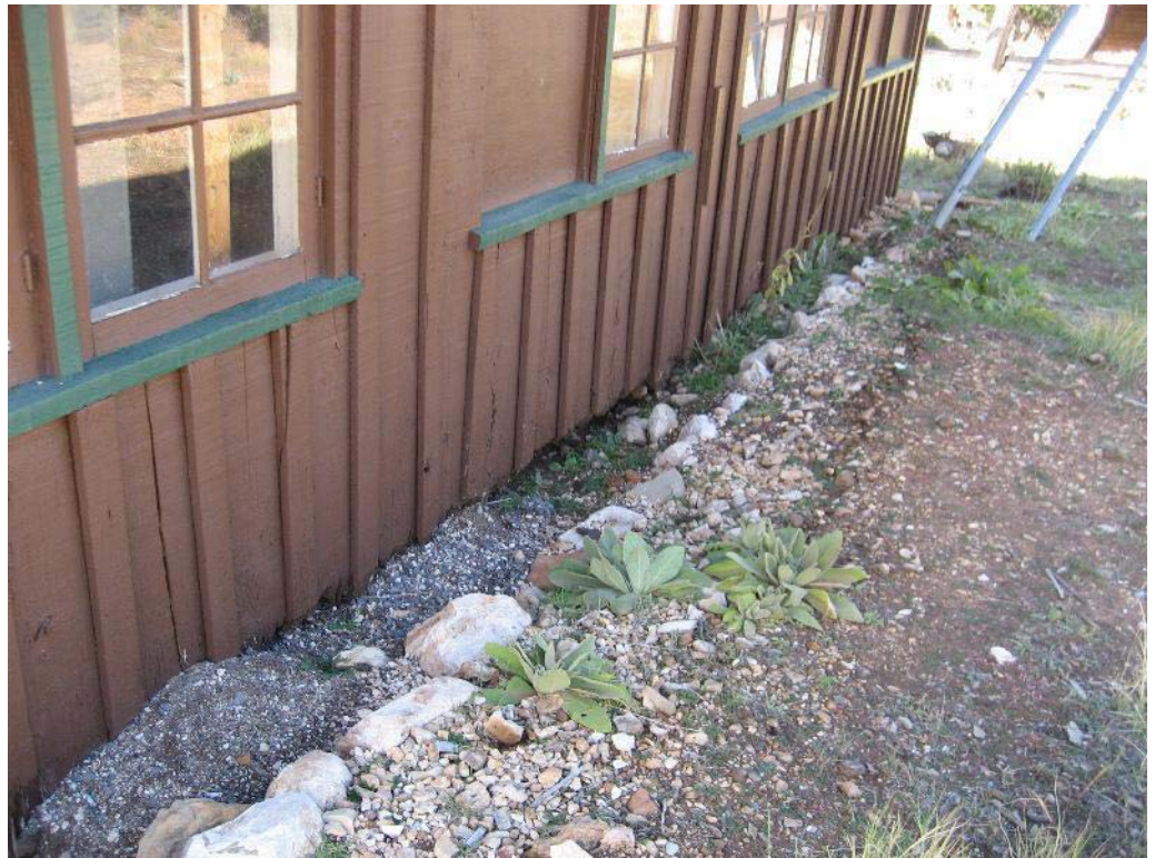
East Wall: Note Lack of Foundation 0069-130
