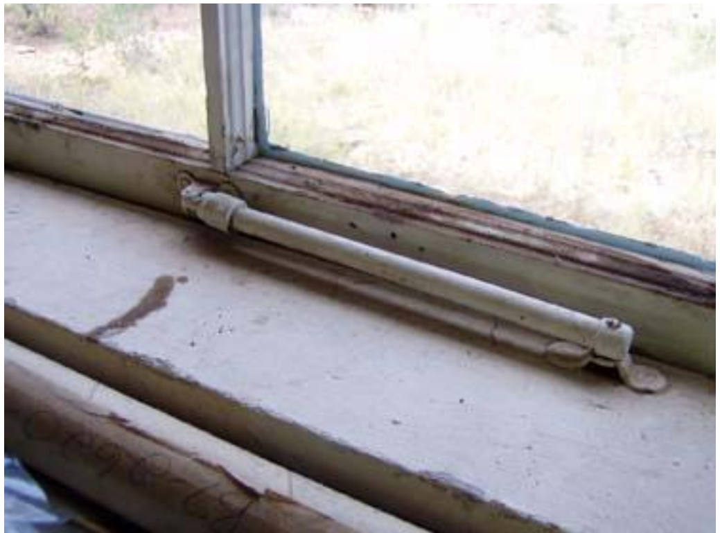
North Window Piston Hardware – (8) 0069-206
