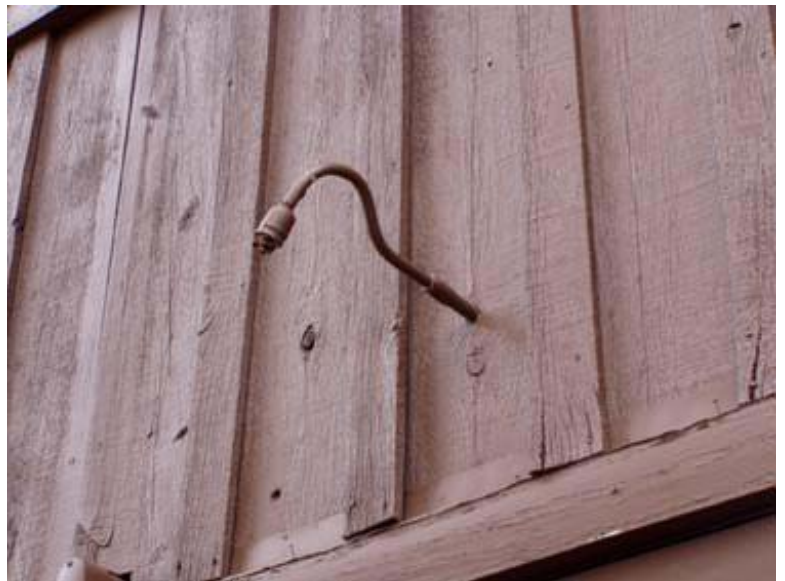
Gooseneck Arm on South Façade 0078-153
