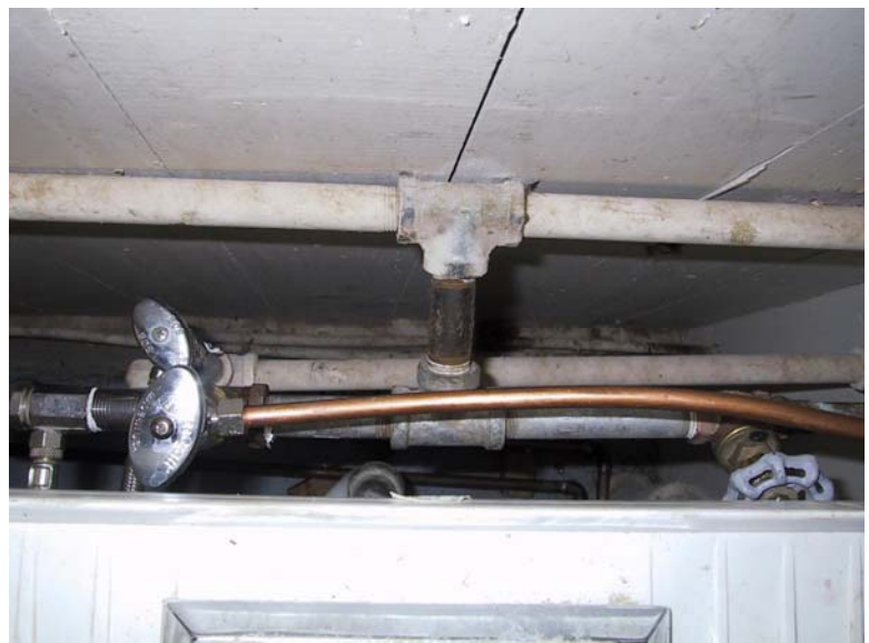
Typical Domestic Water Plumbing 0080-133
