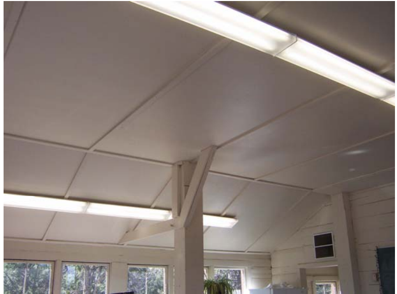
Gypsum Board with Battens 0080-206
