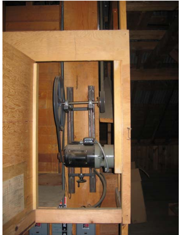
Elevator Hoist motor 0078-268
