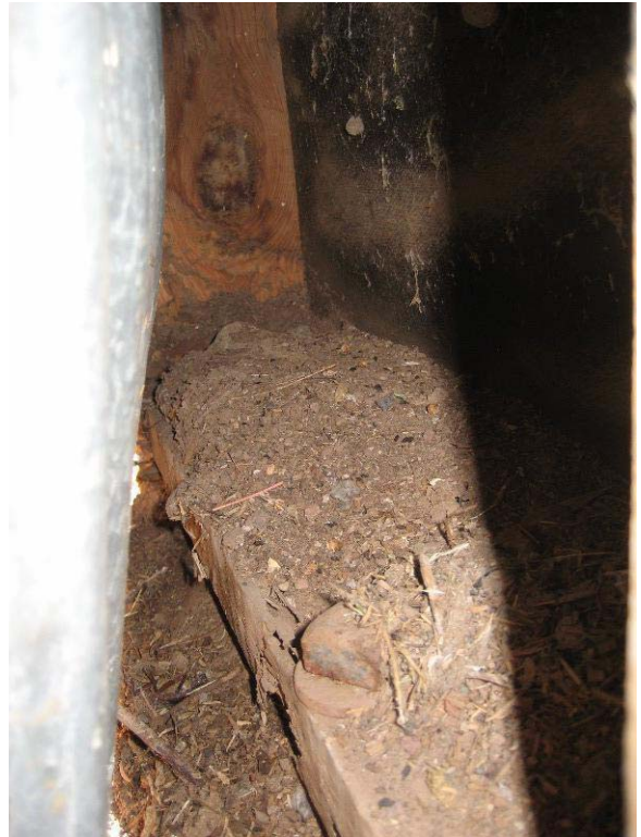
East Wall: Deteriorated Sill and Stud 0080-224
