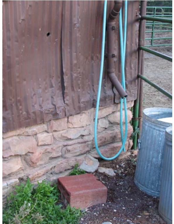
Siding Extends Over Stone Foundation 0080-109
