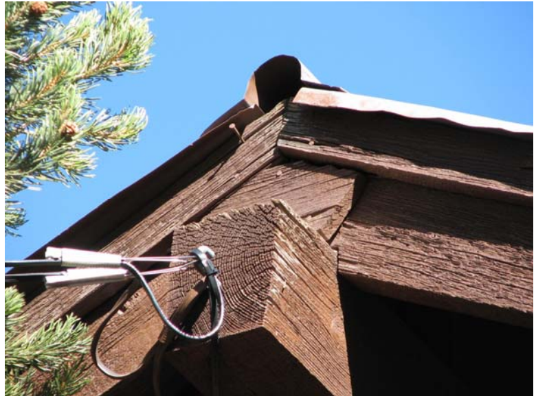
Round-Over Cap Flashing Along Ridge 0090 - 107
