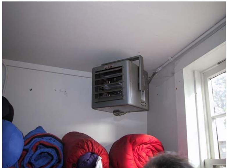
Electric Unit Heater 0078-245
