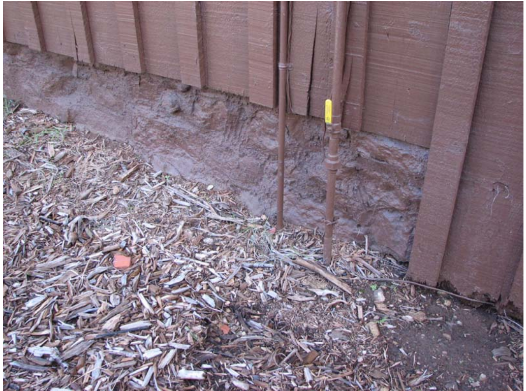
Painted Stone Foundations on North Side 0069-114
