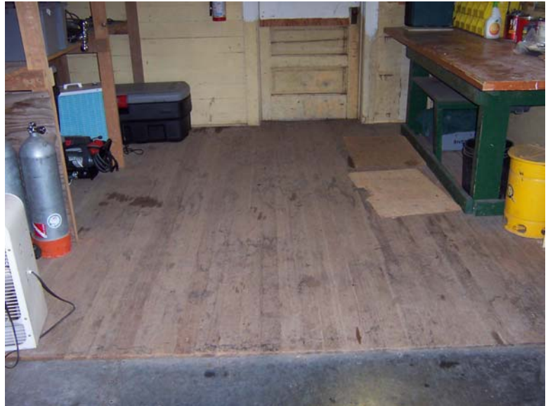
1x3 Tongue and Groove Wood Flooring 0078-235
