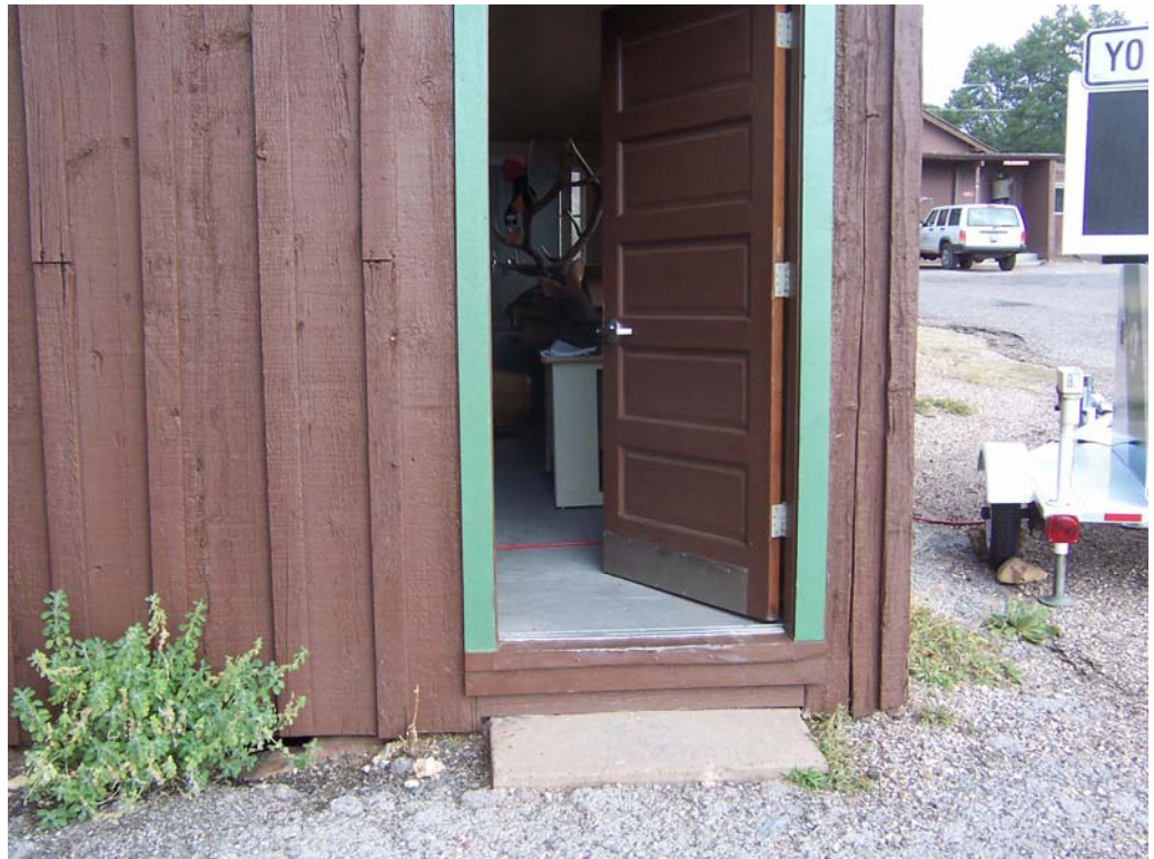
Step and Stop at Exterior Door (A) 0069-128
