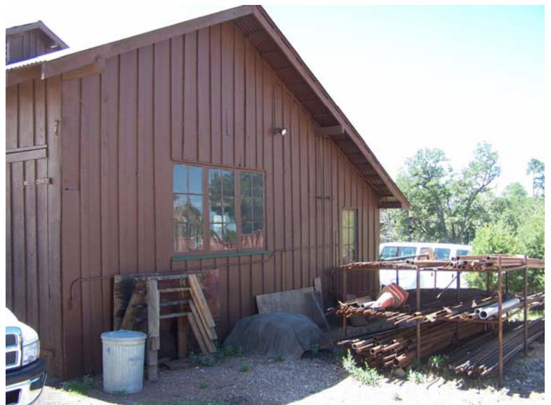
Board and Batten Siding on North Elevation 0075-112
