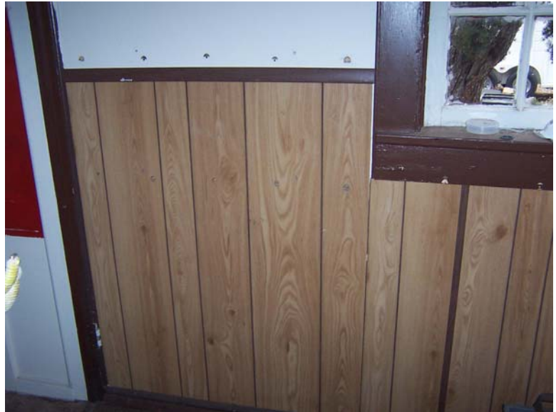
Finished Gypsum Board Above Modern Wood Paneling 0078-233
