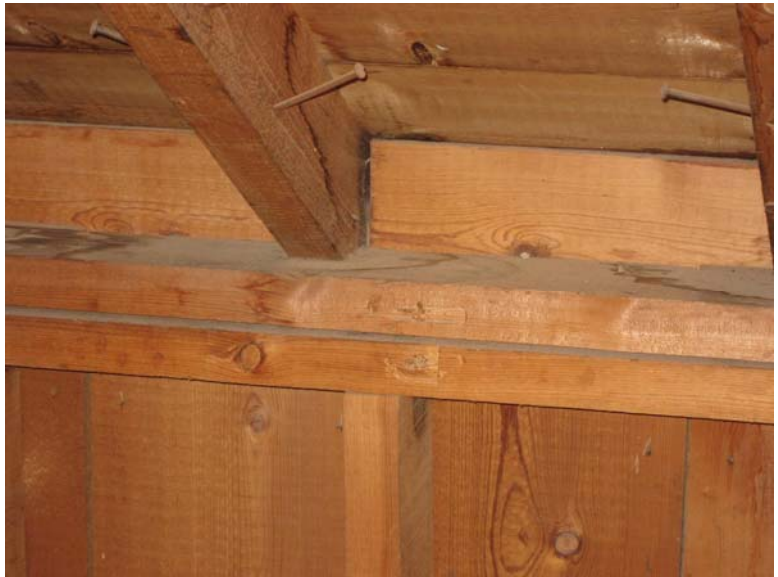
Typical Rafter Bearing at Exterior Wall 0078-259
