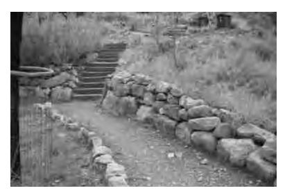
**Photograph 45.** Stone edging, stone walls, and wire mesh tree cages. (JMA 2002)
