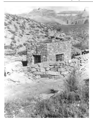
**Figure 54.** General view of rock masonry wall constructed around upstream side of the lower [Rehandling] Pump House, 1965, looking north. (Grand Canyon National Park Museum Collection #4705k)
