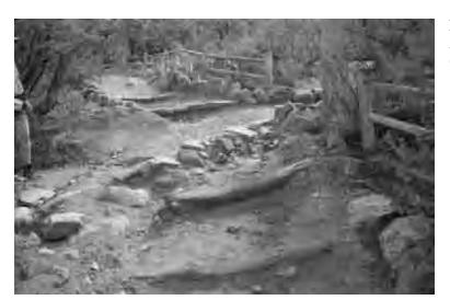
**Photograph 14.** Erosion around Bright Angel Trail log risers. (JMA 2002)
