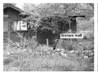
**Figure 71.** Repair the Caretaker's Residence/SAR Cache terrace by stabilizing the wall and removing unwanted vegetation growing through and over the stones. (History Matters 2002)
