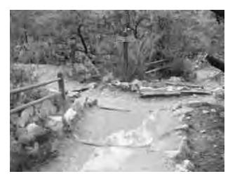
**Figure 60.** Portions of trails that puddle during wet weather should have low spots filled during trail maintenance. Assess the causes of puddling to prevent recurrence.
