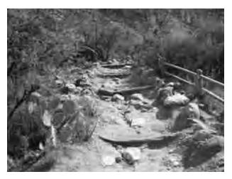
**Figure 61.** Eroded places around log risers should be backfilled and and the trail tread resurfaced during trail maintenance. Repairs should be made so that water is diverted away from the trail tread, rather than trapped.
