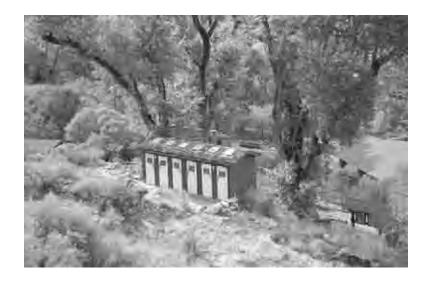
**Photograph 91.** Concrete cistern located at site of perennial spring. (JMA 2002)
