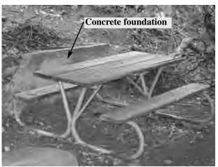
**Figure 73.** Determine the original purpose of the foundation and remove it if it is not historic, serves no purpose, and will not be re-used.
