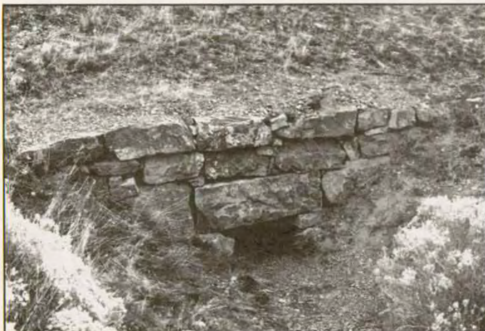
Figure 36. Detail of stabilized stone culvert in CP grade – west slope. Source: HRA 2000.
