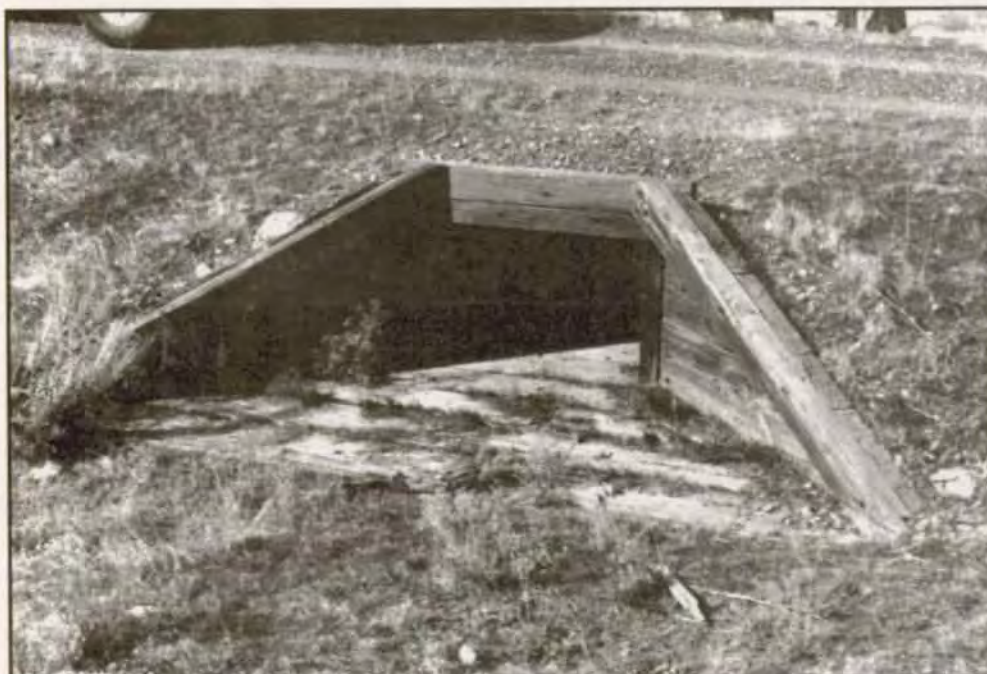
Figure 37. Detail of wood culvert in CP grade – west slope. Source: HRA 2000.
