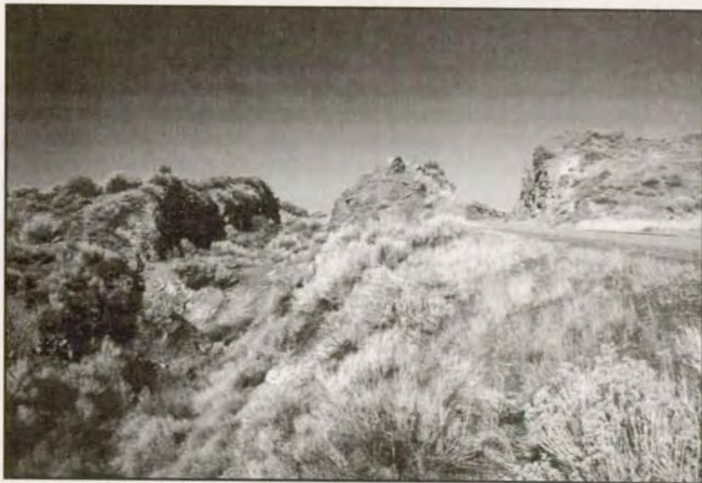
Figure 45. View to the west of the parallel grades of the CP (right) and the UP (left), west slope. Unfinished UP grade shows stair-step cut. Source: HRA 2000.
